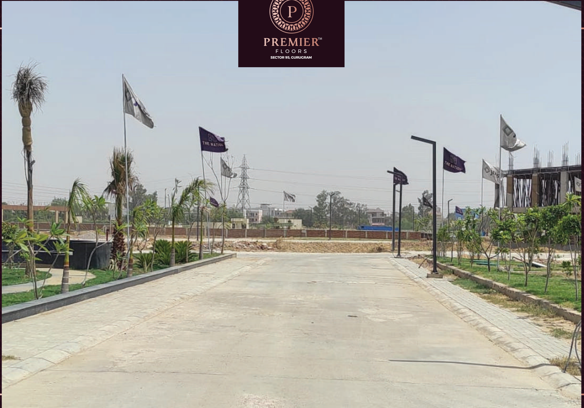
Pathway Development Work In Progress
