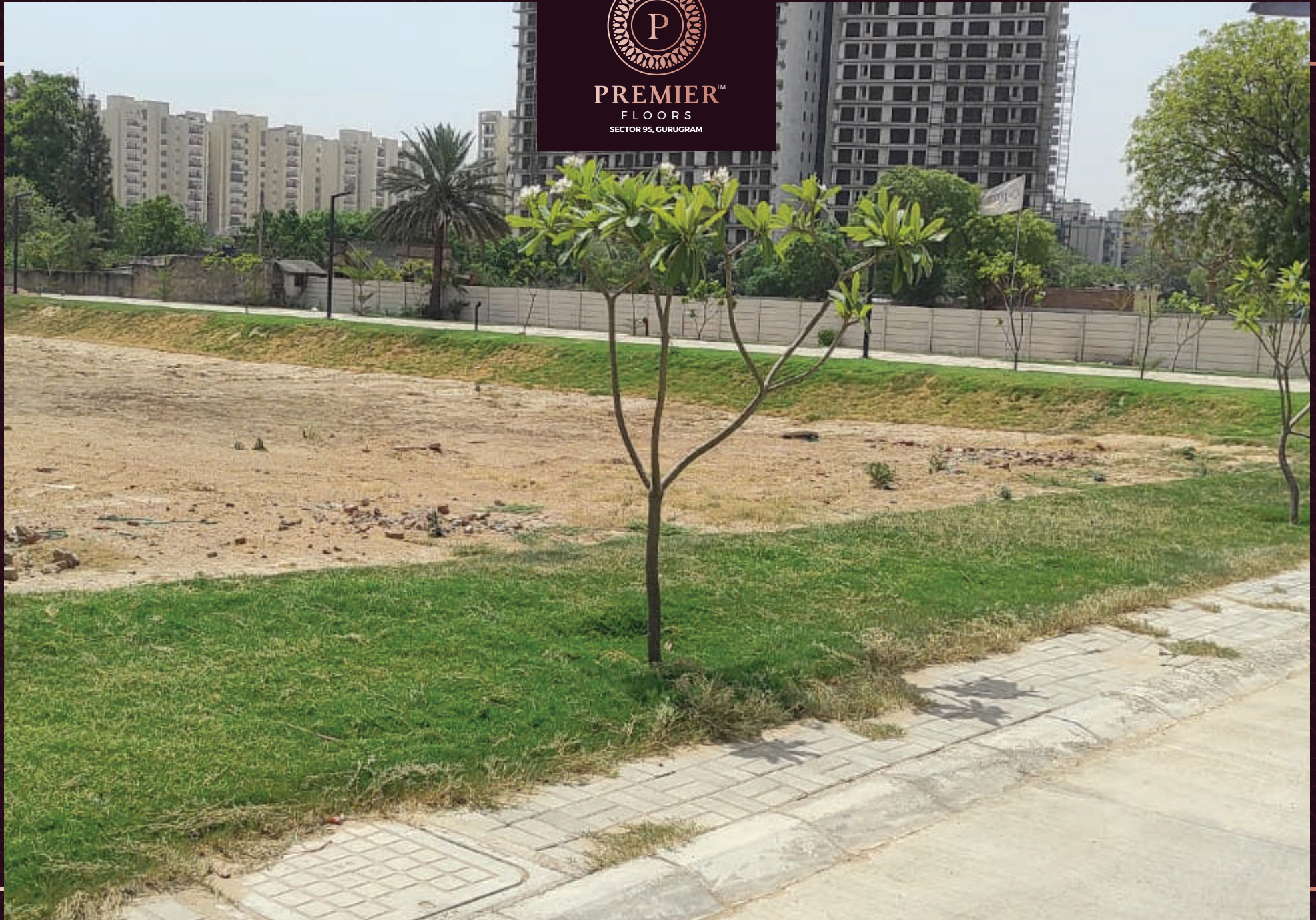
Pathway Development Work In Progress
