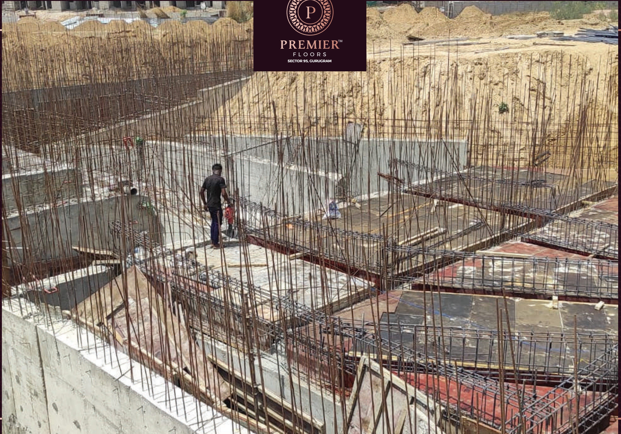
STP Construction Work In Progress
