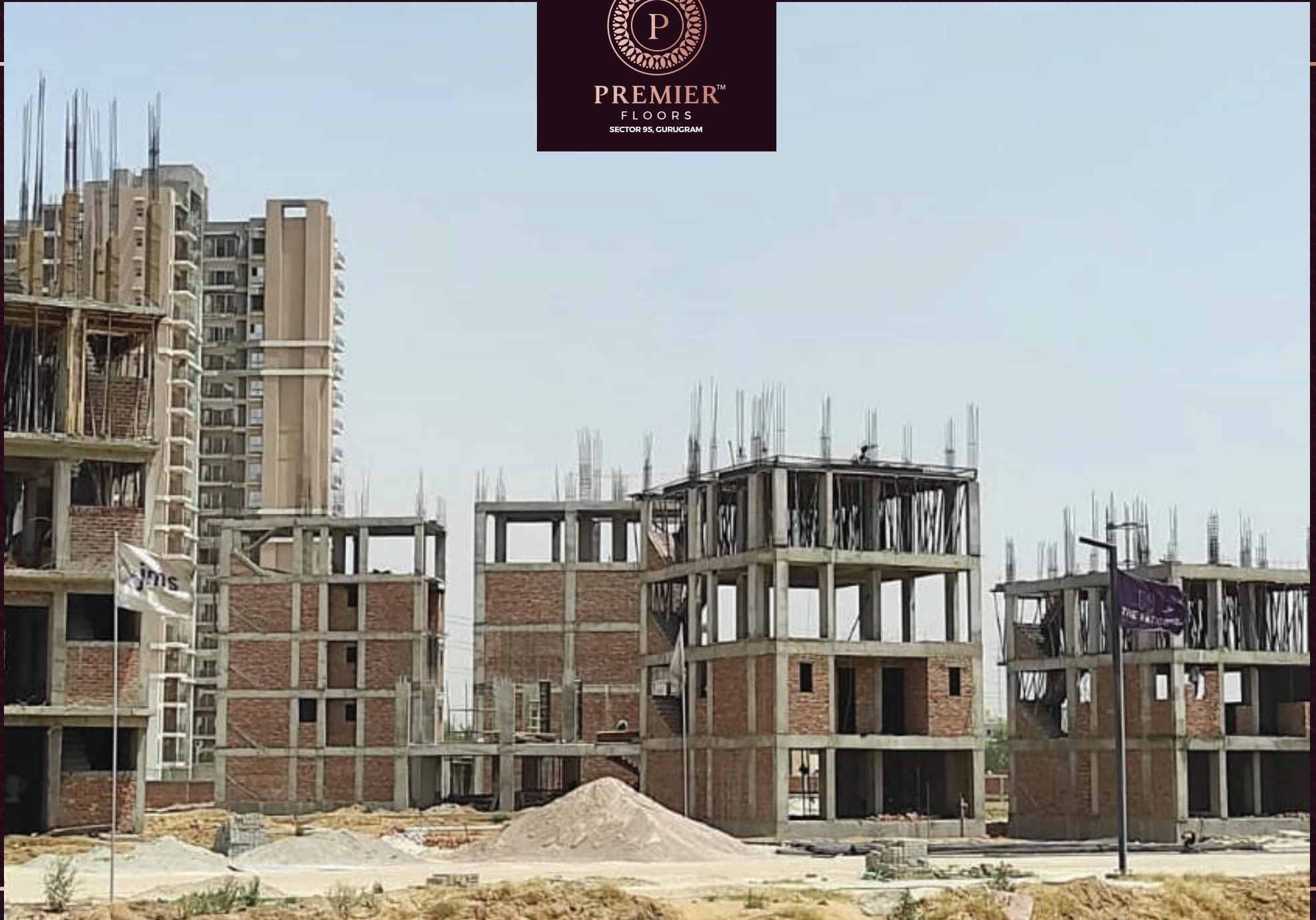
Floors Construction Work In Progress
