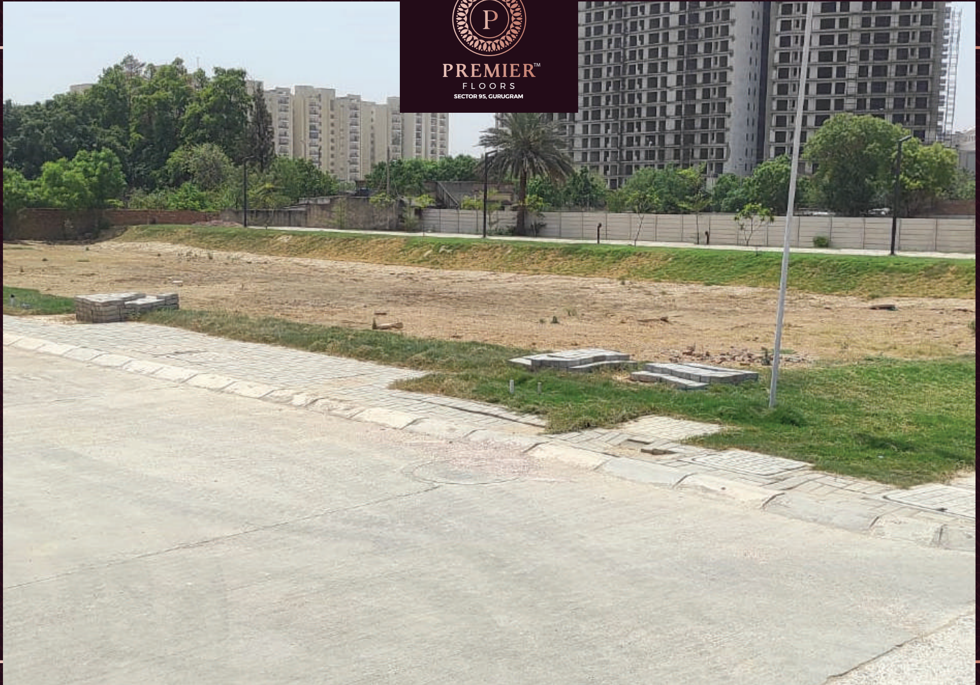
Pathway Development Work In Progress
