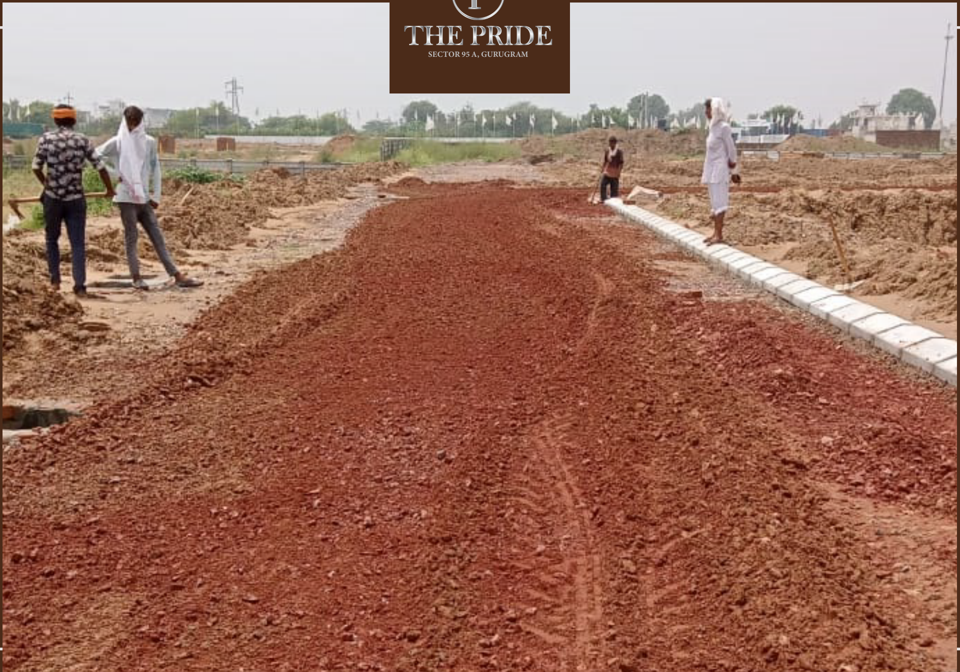
BALANCE ROAD WBM WORK IN PROGRESS
