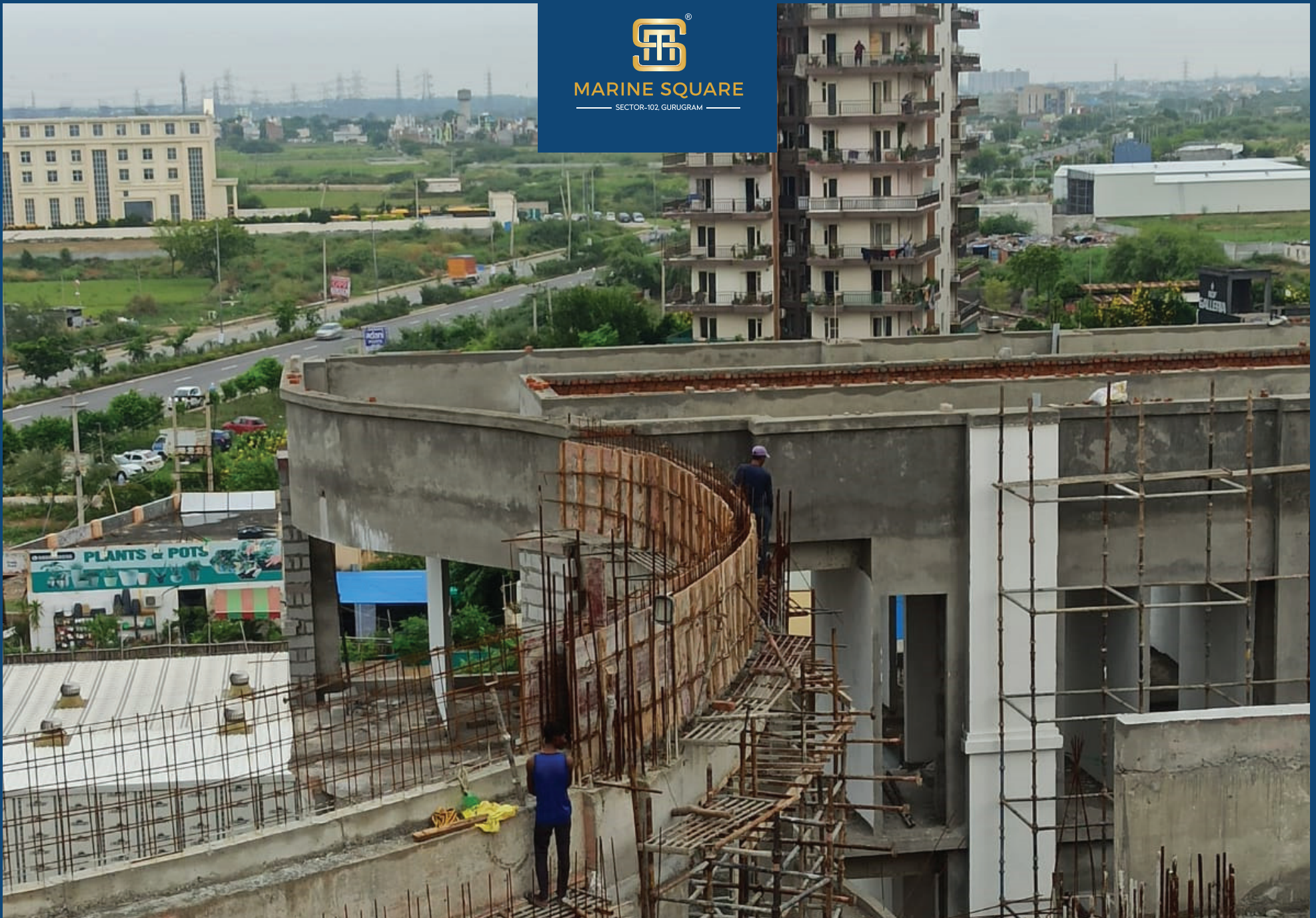
Parapet Wall Shuttering Work In Progress
