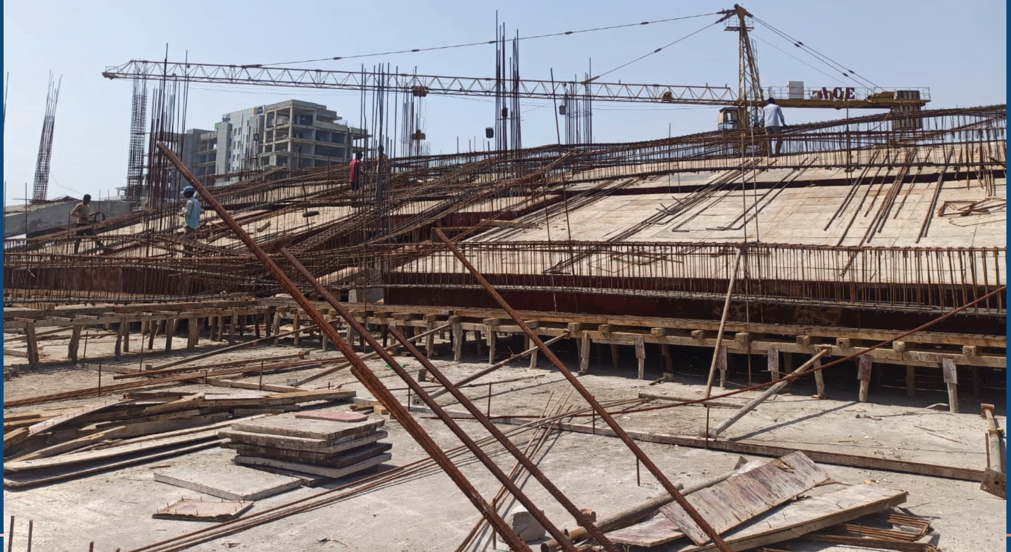
Multiplex Slab Shuttering
