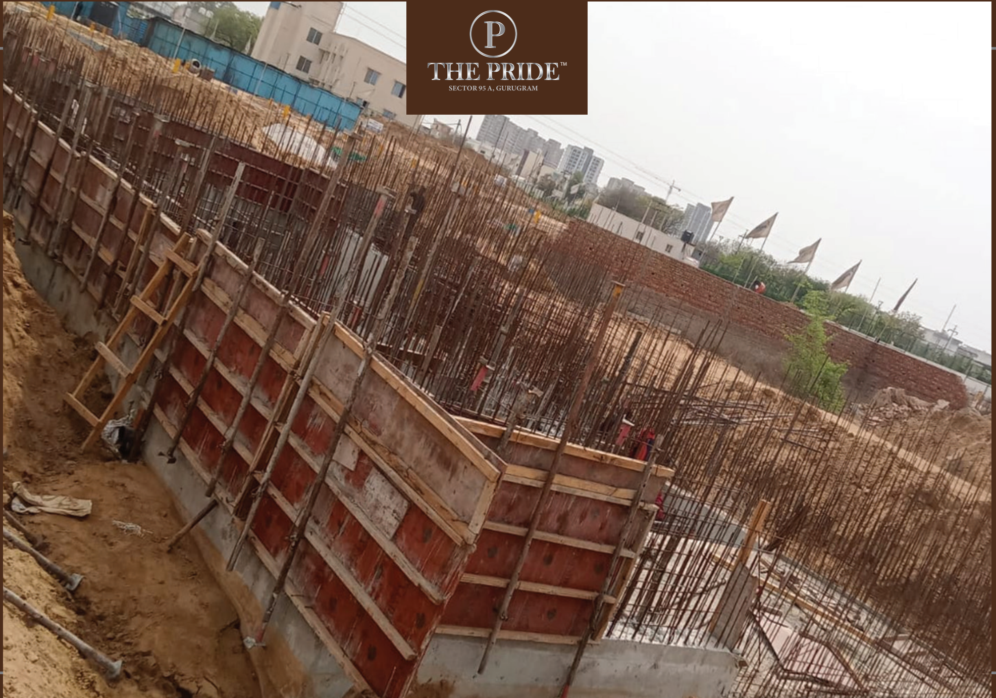
STP Tank Work In Progress
