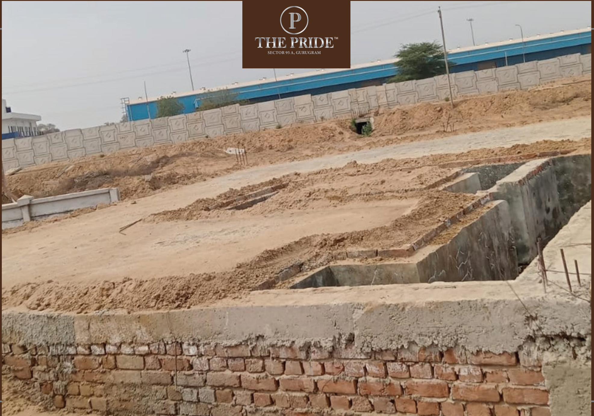
Green Area & CSS Foundation Work In Progress
