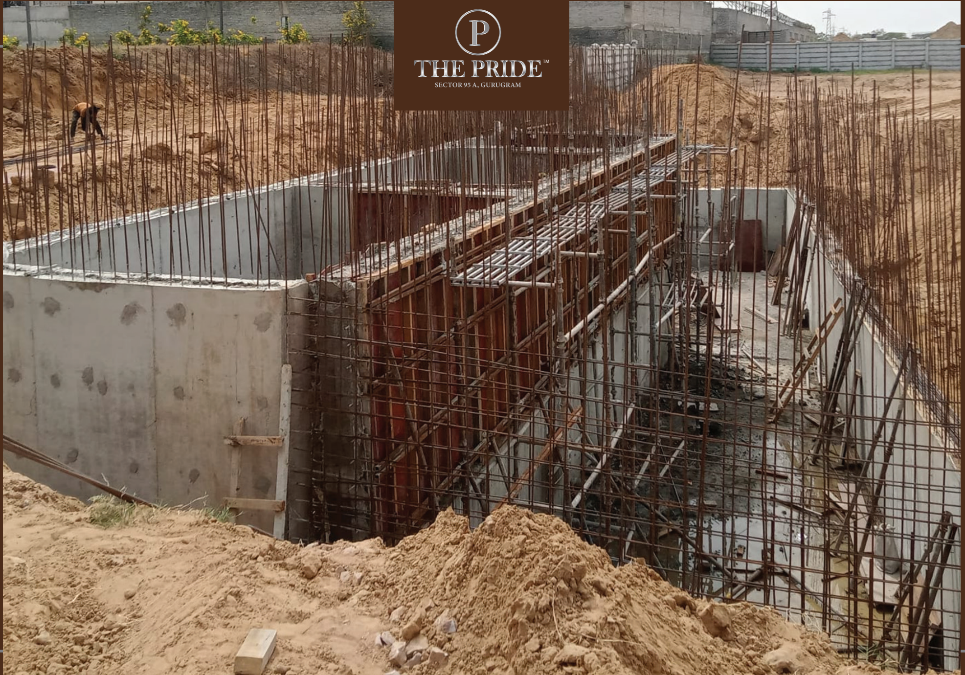
UG Tank Construction Work In Progress
