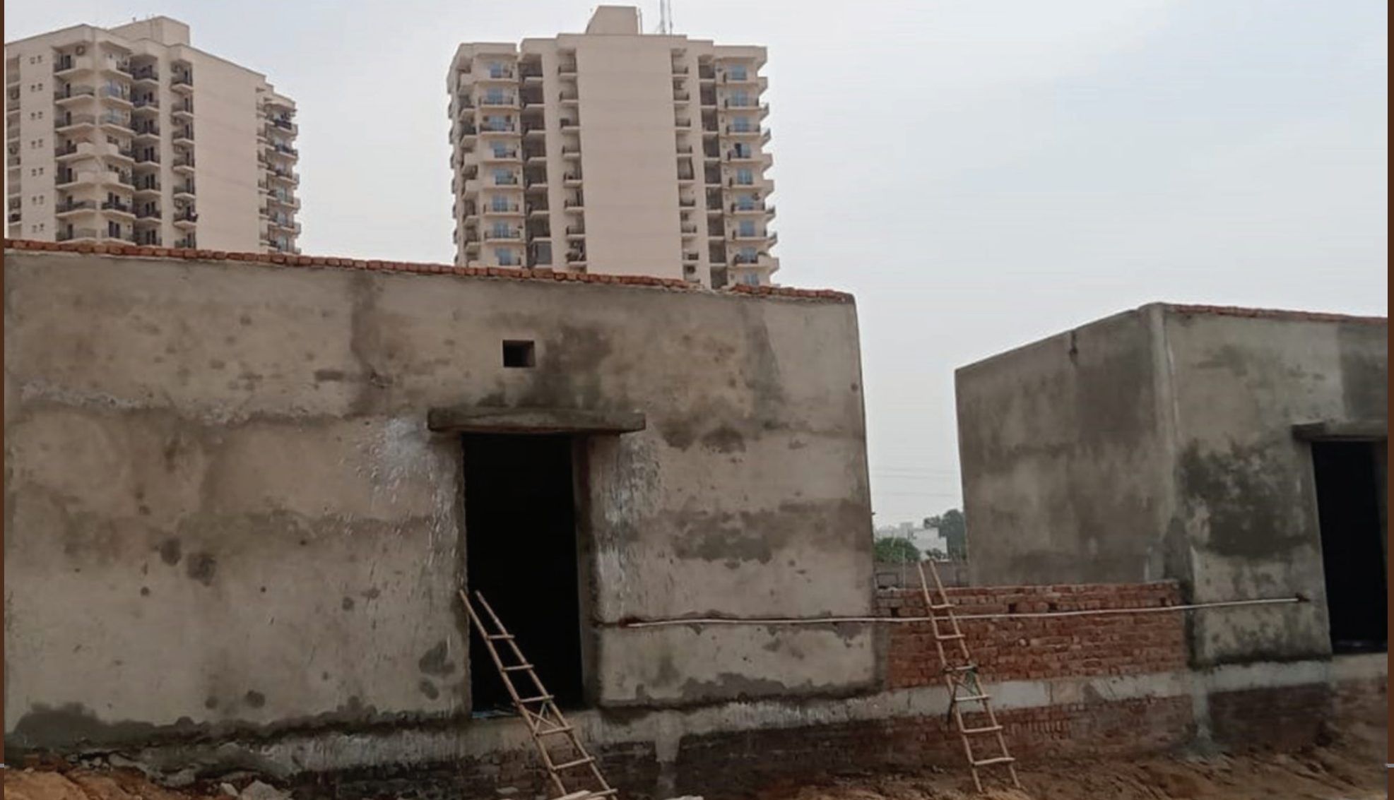
HT & VCB Room Work In Progress
