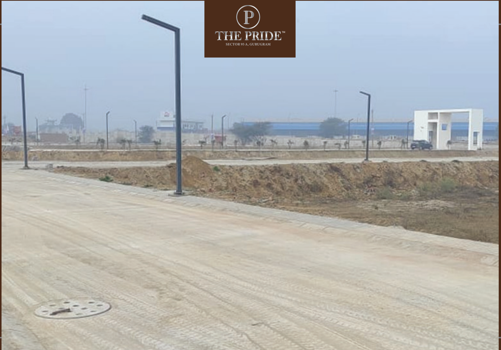
Electrical Light Poles & Paver Path Work Completed
