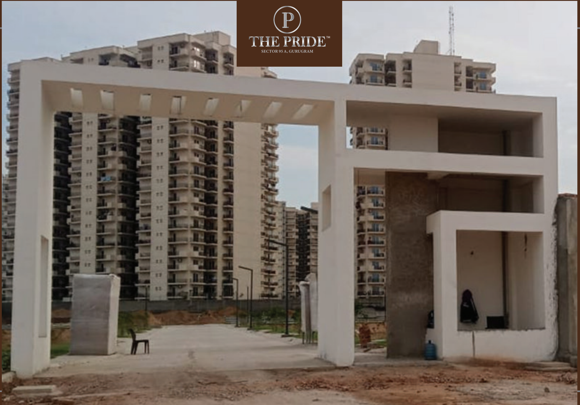
Entry Gate Finishing Work In Progress
