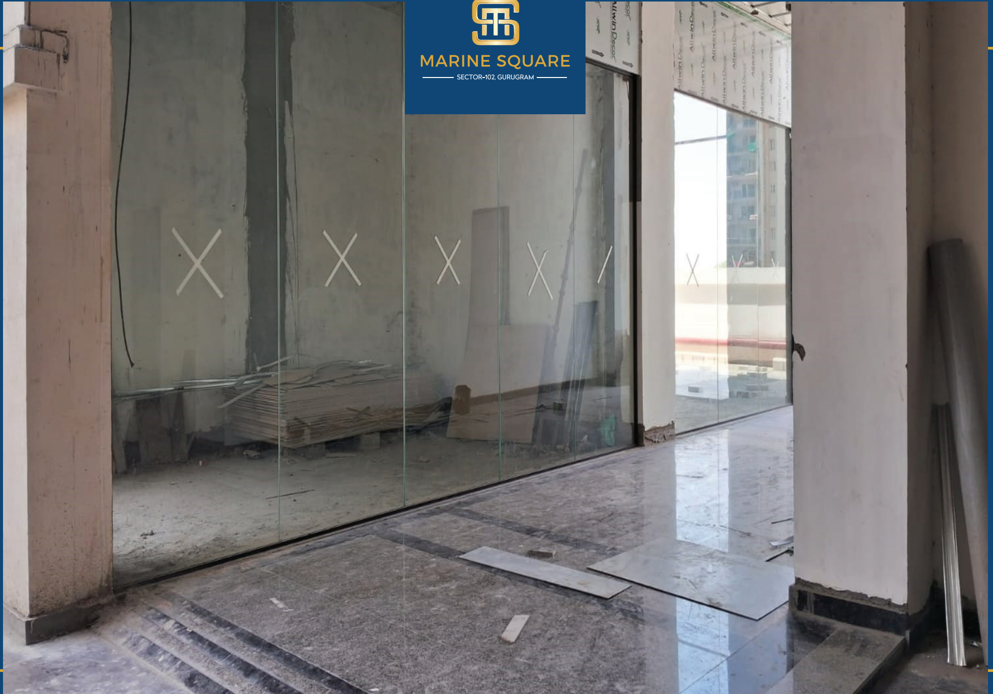
Glass Fixing Work In Progress
