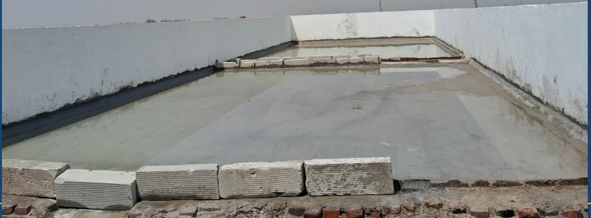
Terrace Waterproofing Work In Progress
