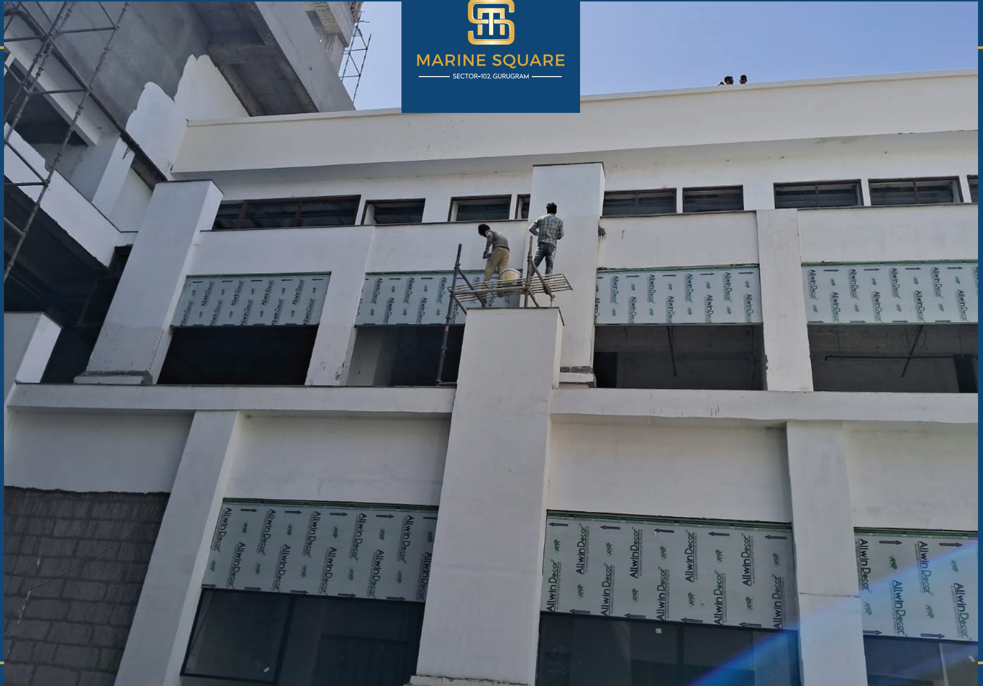
External Paint Work In Progress
