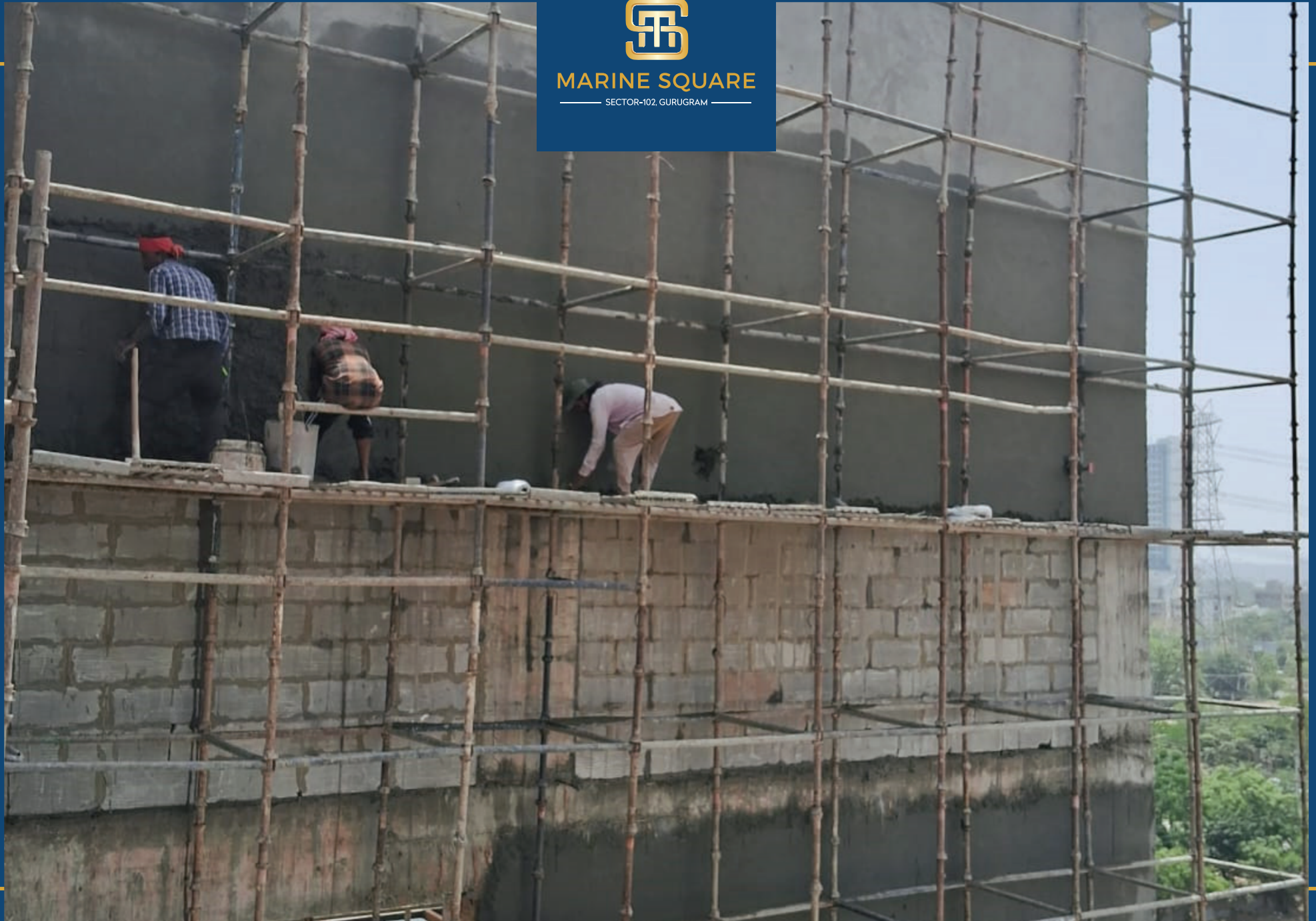
Outer Plaster Work In Progress
