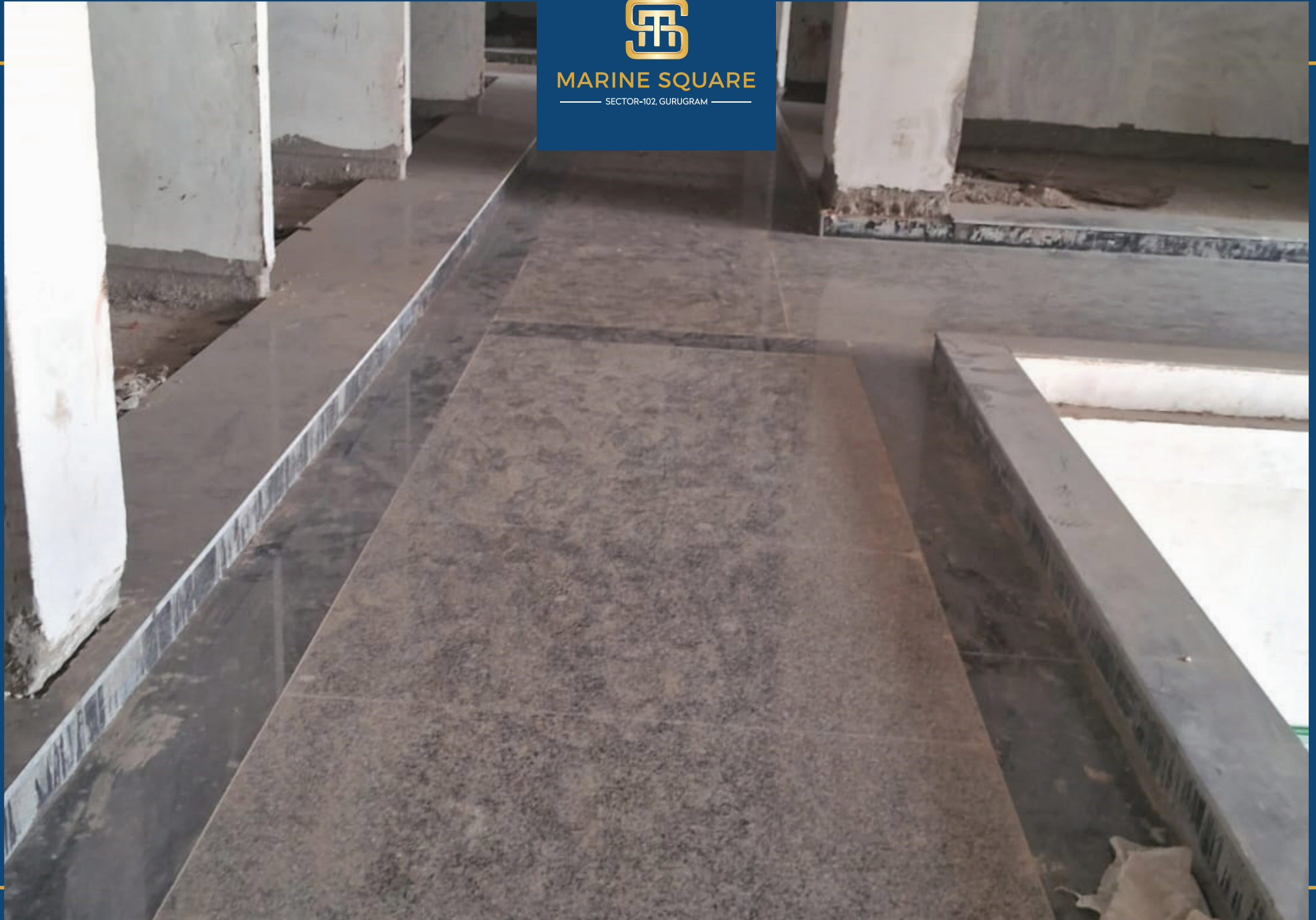
Granite Work In Progress
