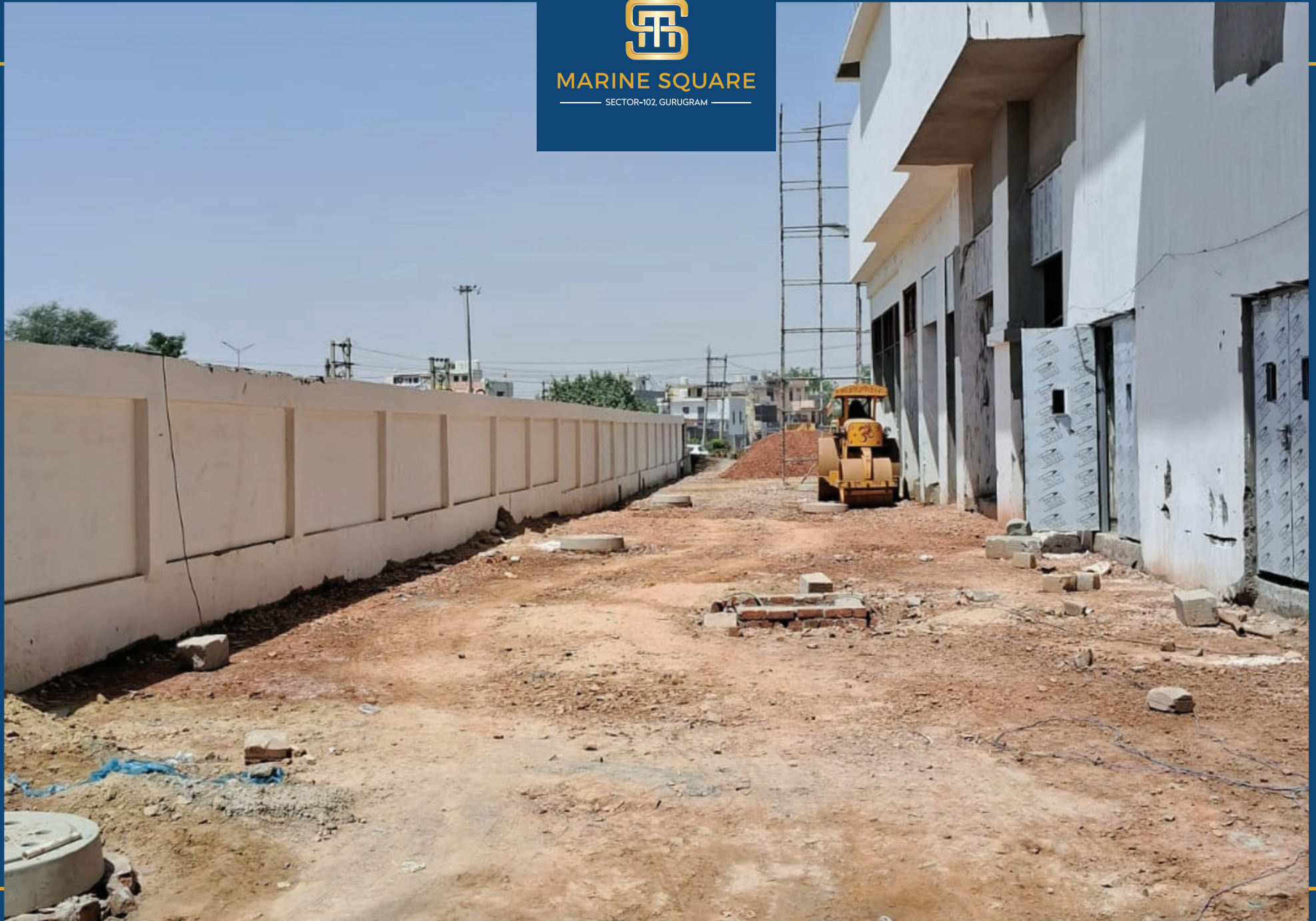
Road Construction Work In Progress
