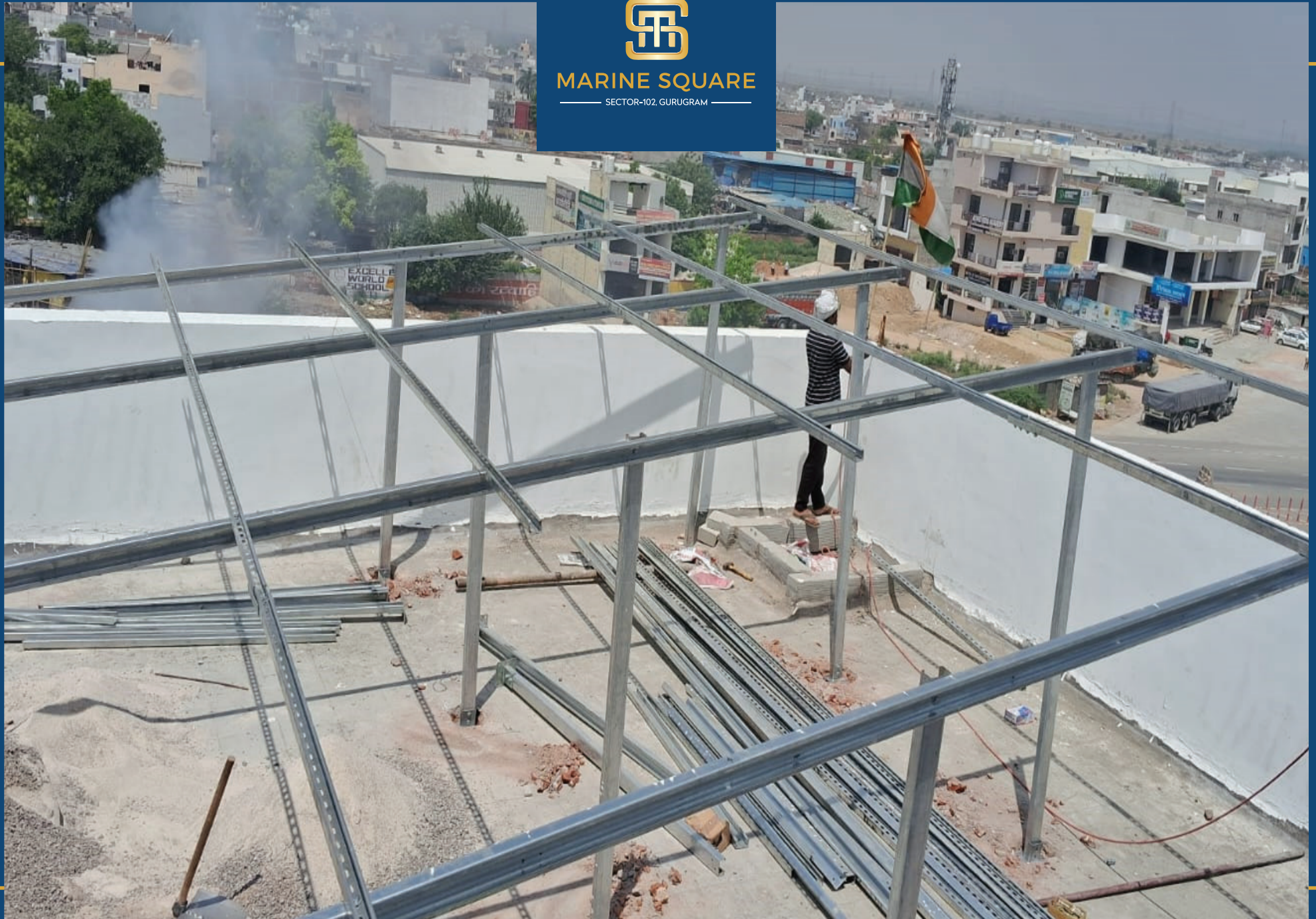
Solar Panel Frame Fixing Work In Progress
