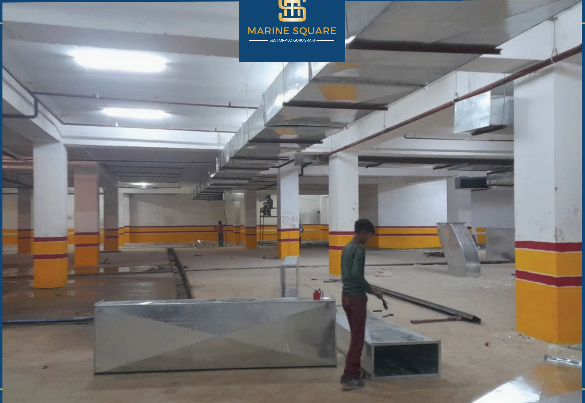
Ducting Work In Progress
