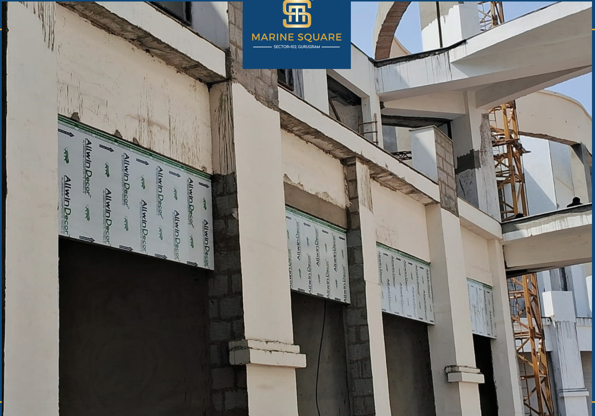
ACP Sheet Fixing Work For Glass Door
