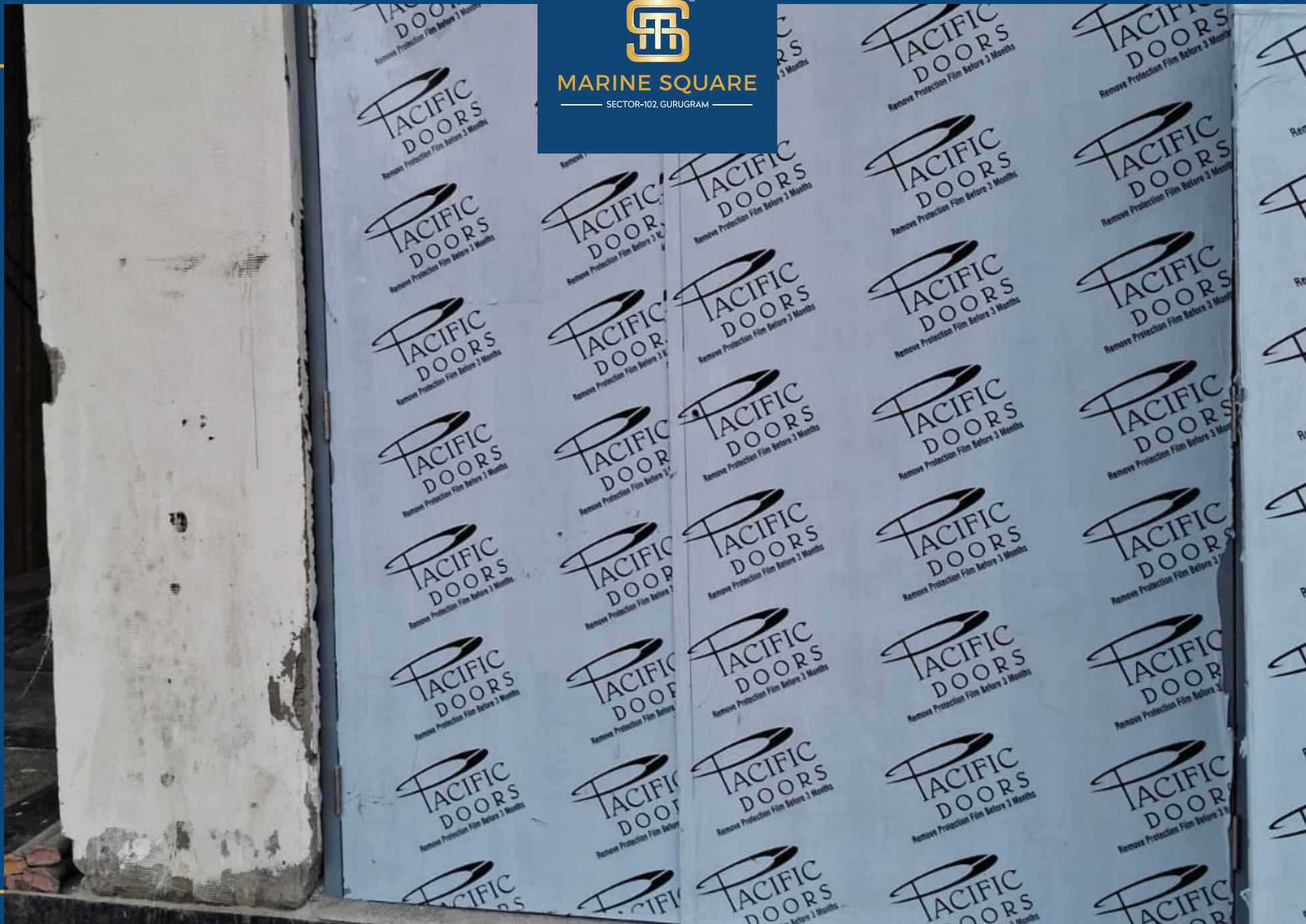
File Door Work In Progress
