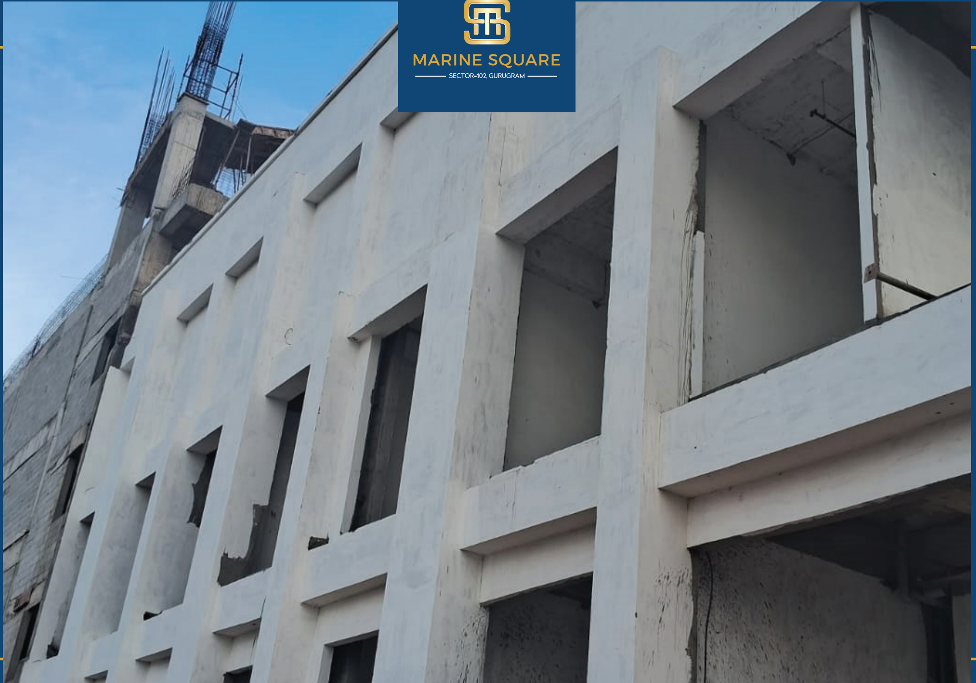
External Paint Work In Progress
