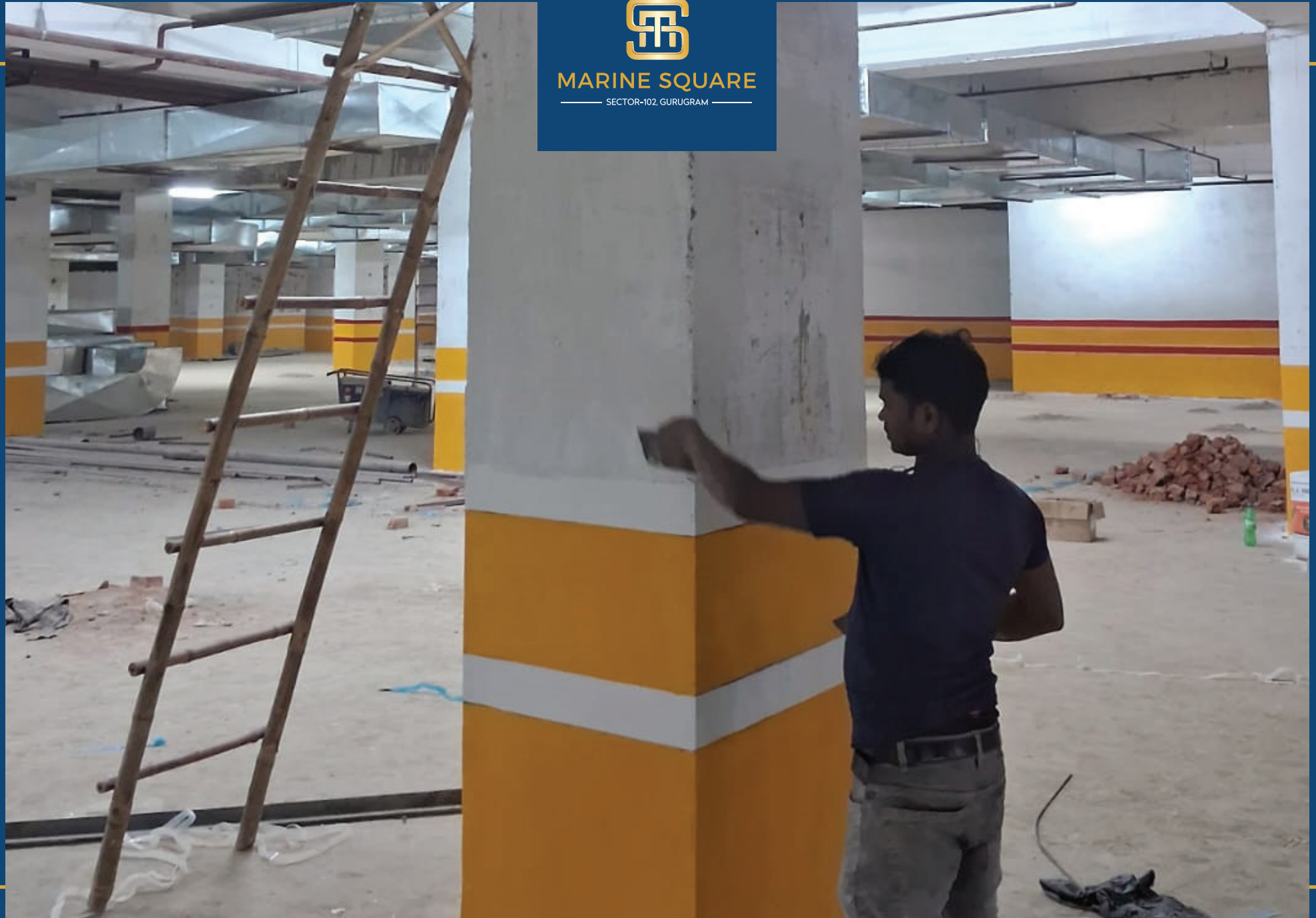
Basement Parking Paint Work In Progress
