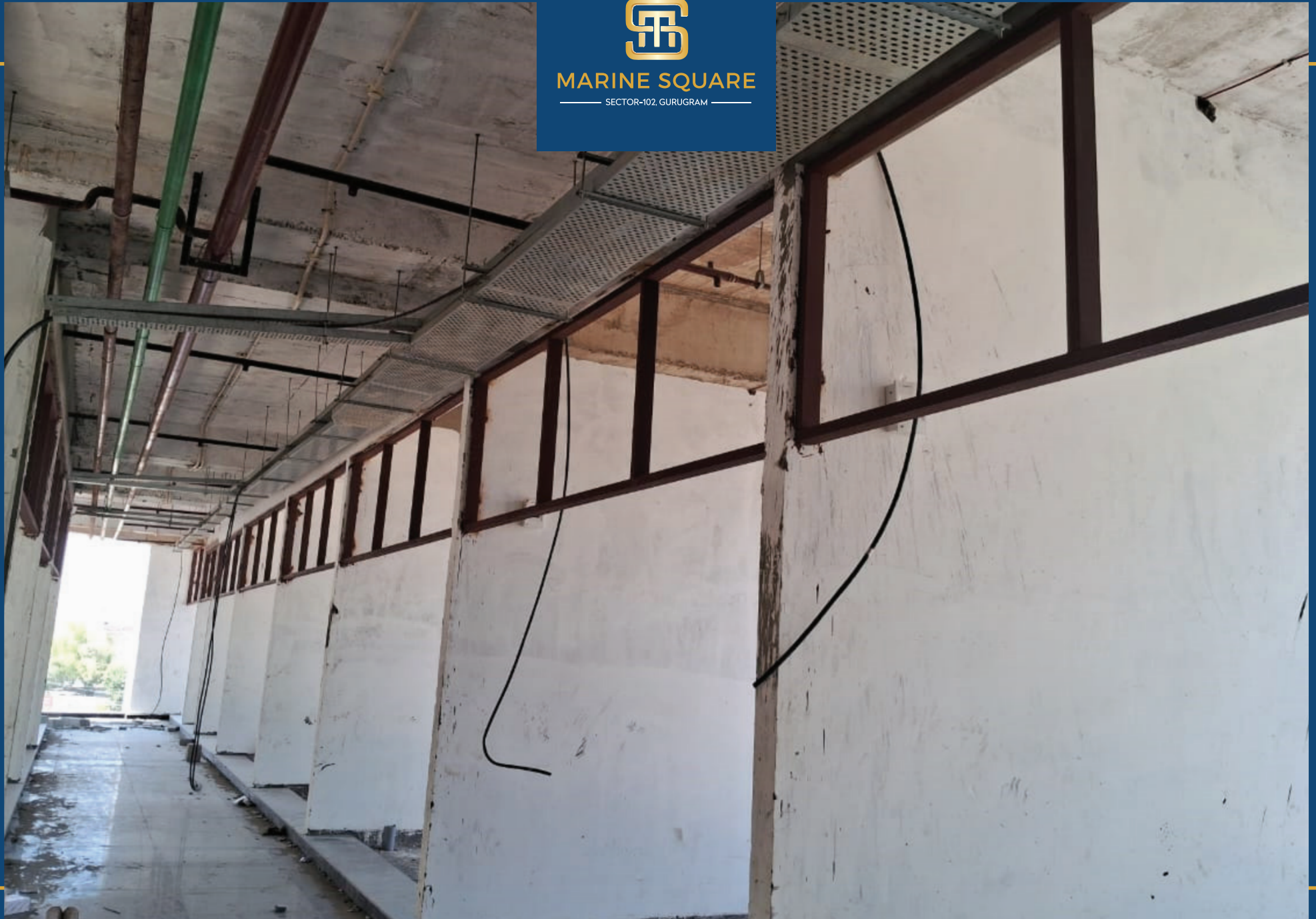
MS Shop Frame Work In Progress
