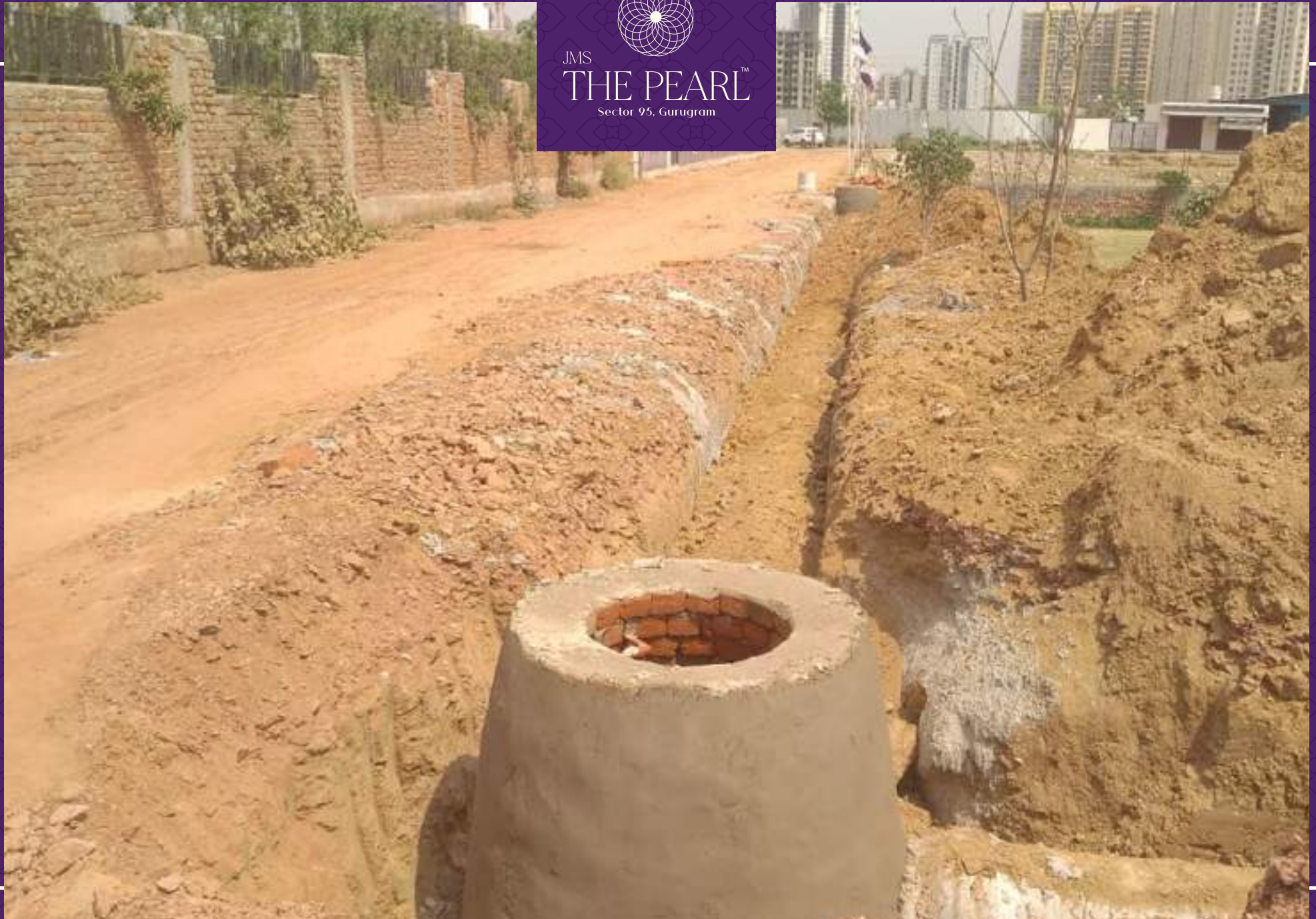
Sewer Line Laying Work In Progress
