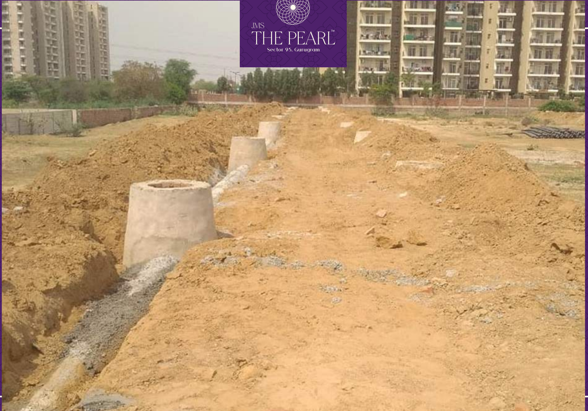
Storm Line Laying Work In Progress
