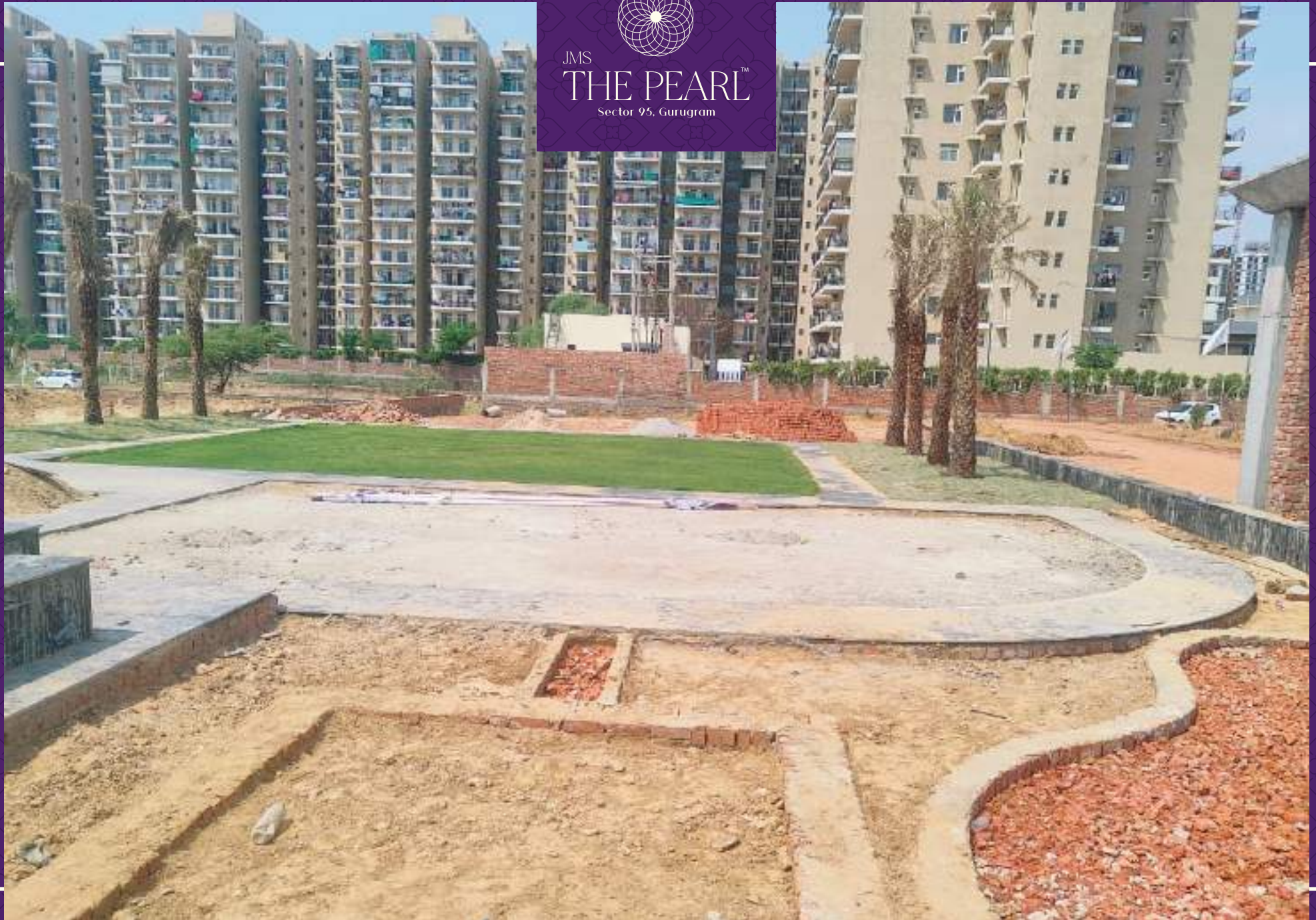
Park Area Work In Progress
