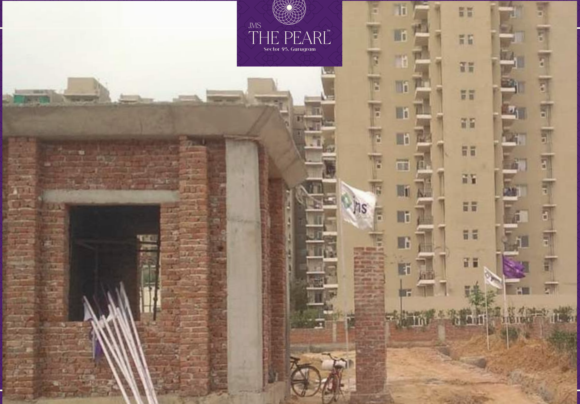
Entry Gate Work In Progress
