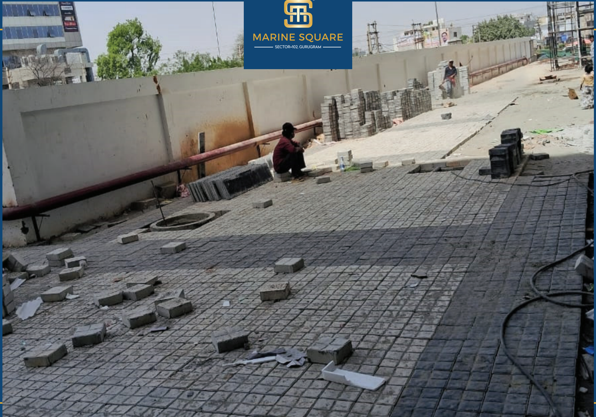
Pavour Block Work In Progress
