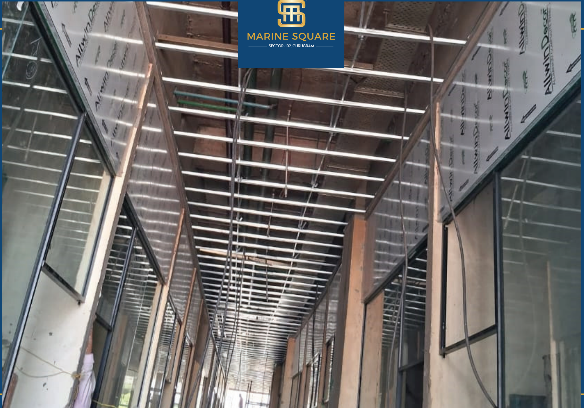
False Ceiling Framework In Progress
