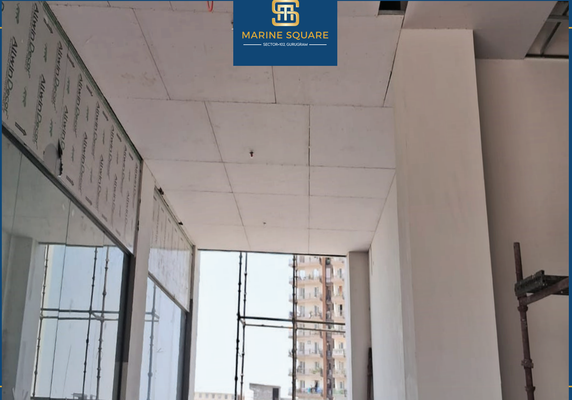
False Ceiling Work In Progress on Ground Floor
