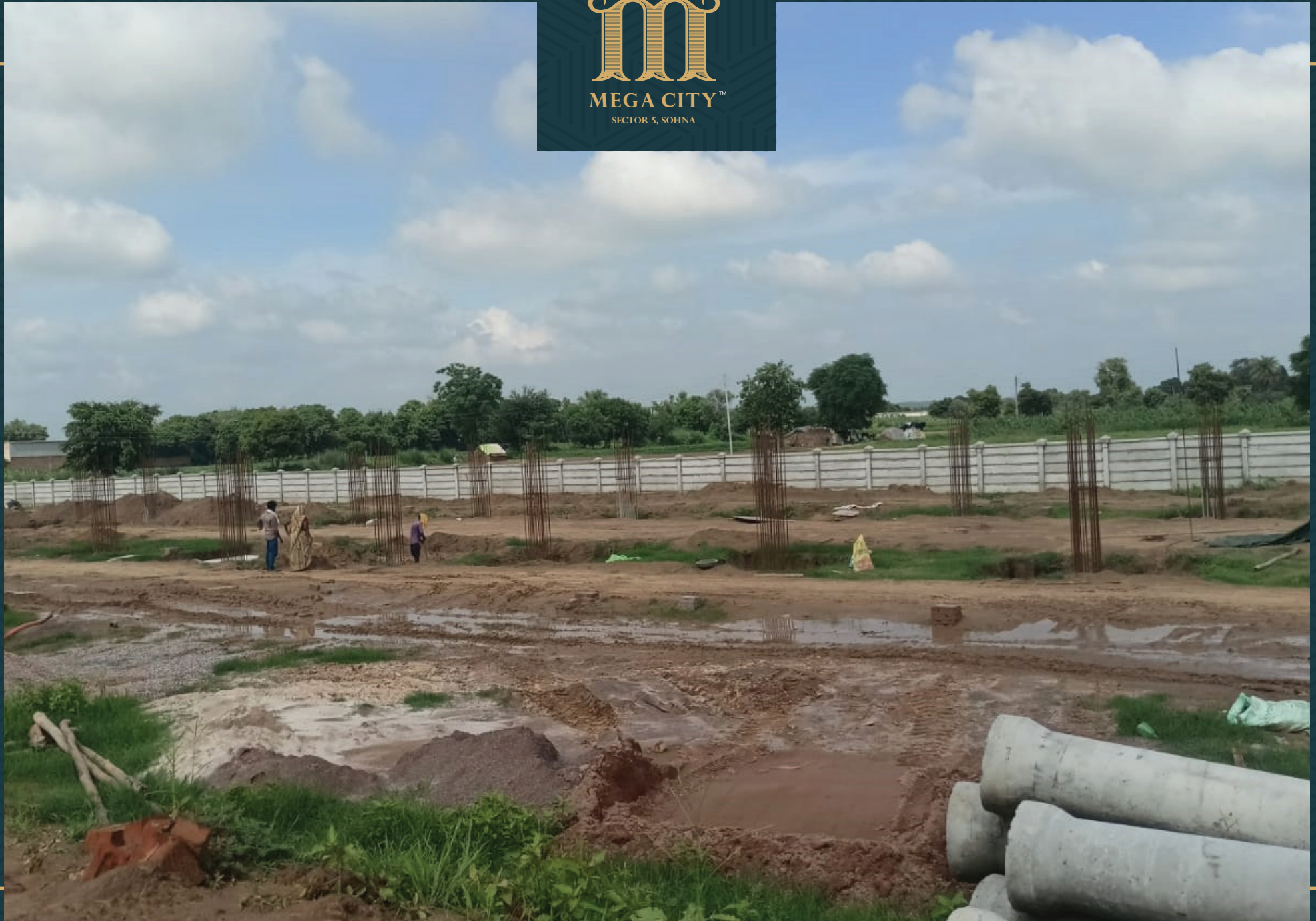
Club Building and Swimming Pool Foundation Work In Progress
