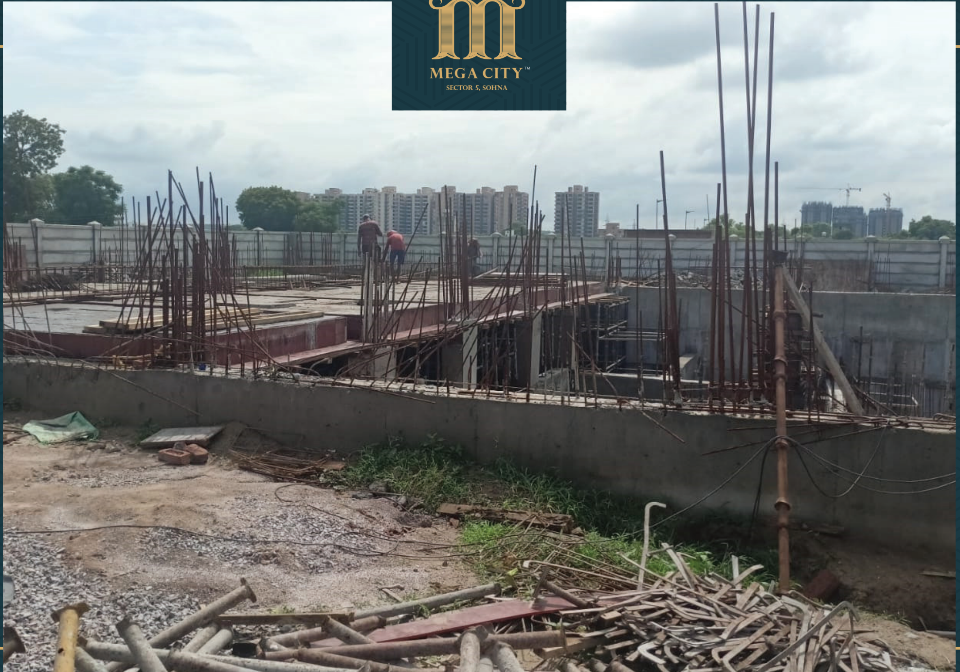
STP Slab Shuttering and Reinforcement In Progress
