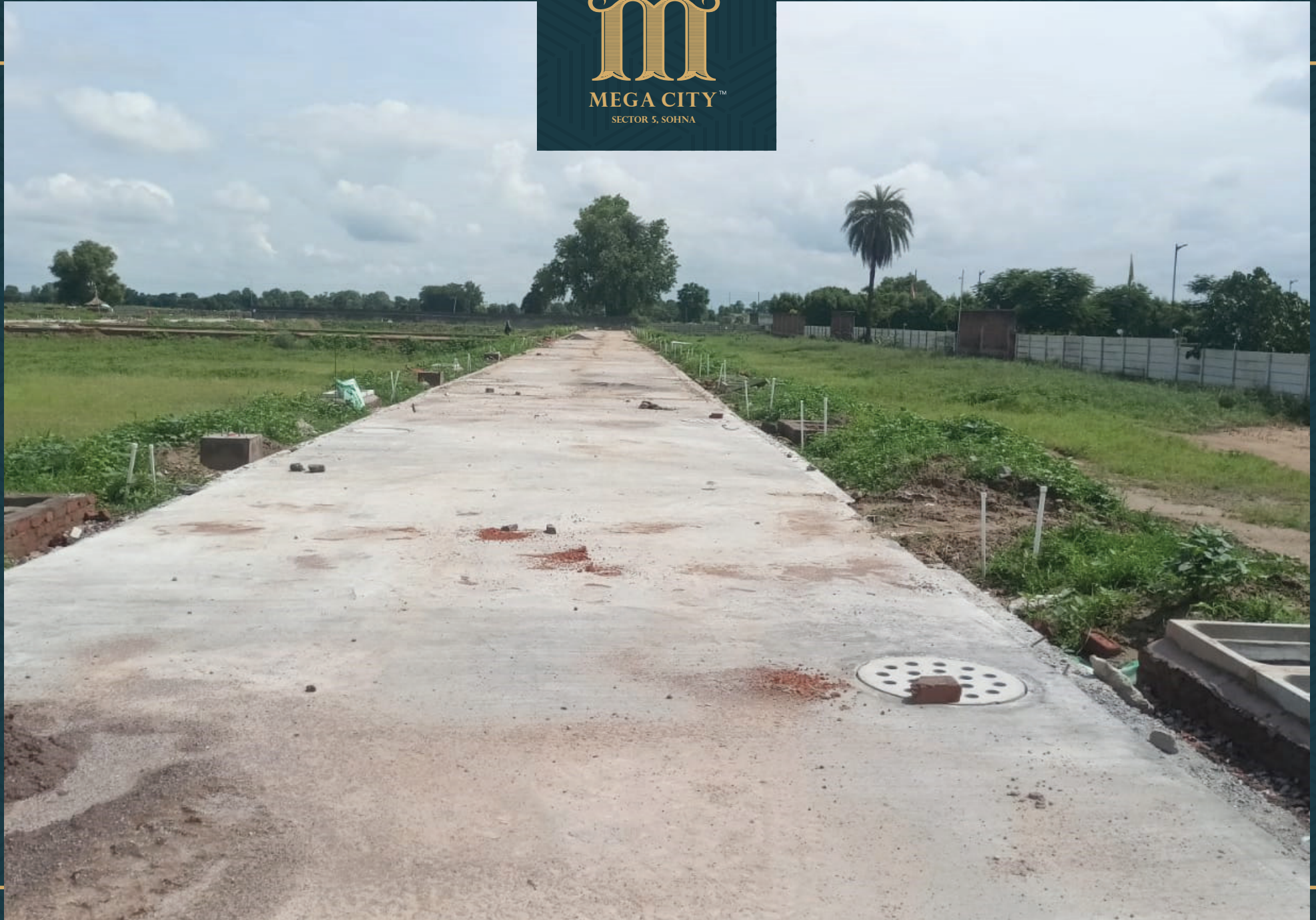
Road no 1 Water Supply, Sewerage, Road Trimix, Street Lights Foundation Completed
