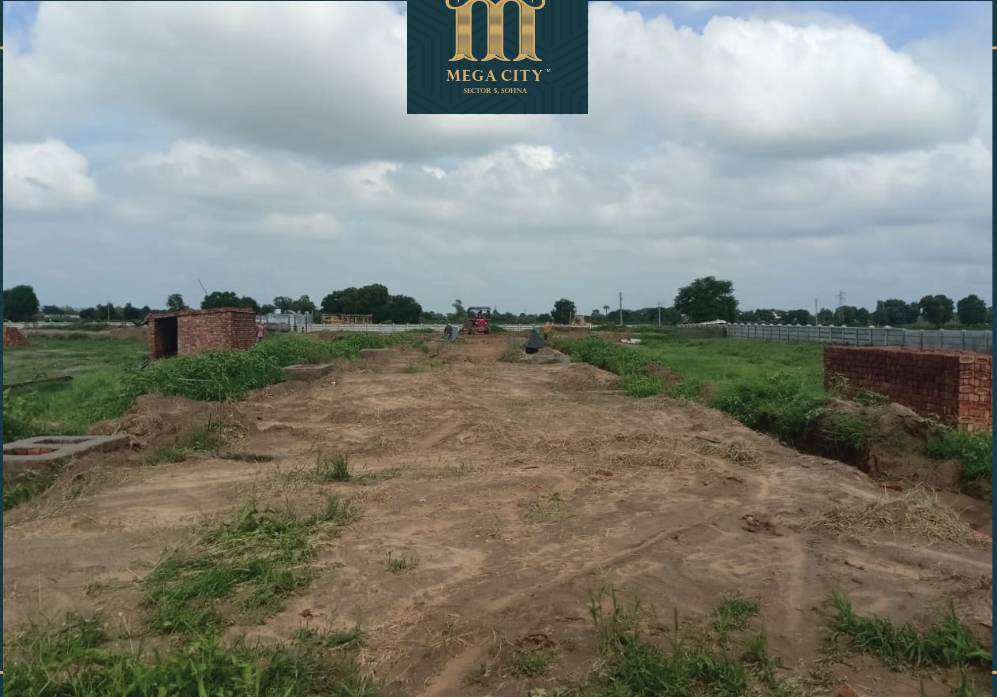
Road no 8 Road Subgrade and Electrical Chambers Work In Progress
