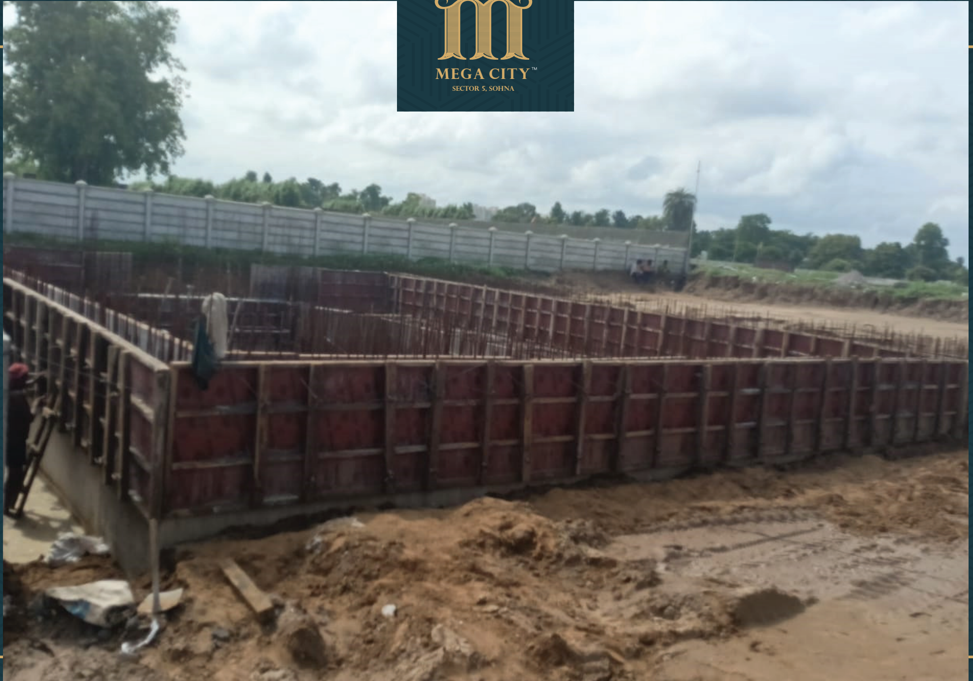
UGT Walls In Progress
