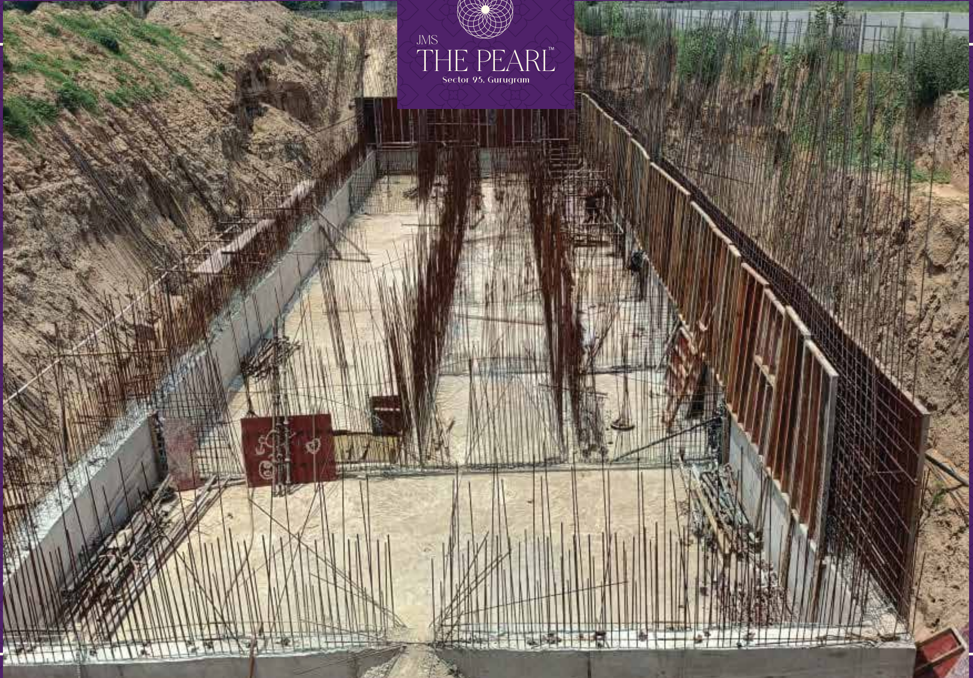
STP Construction Work In Progress
