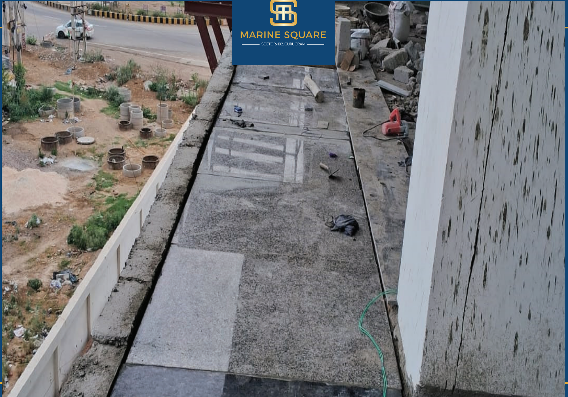
Granite Floor Work In Progress
