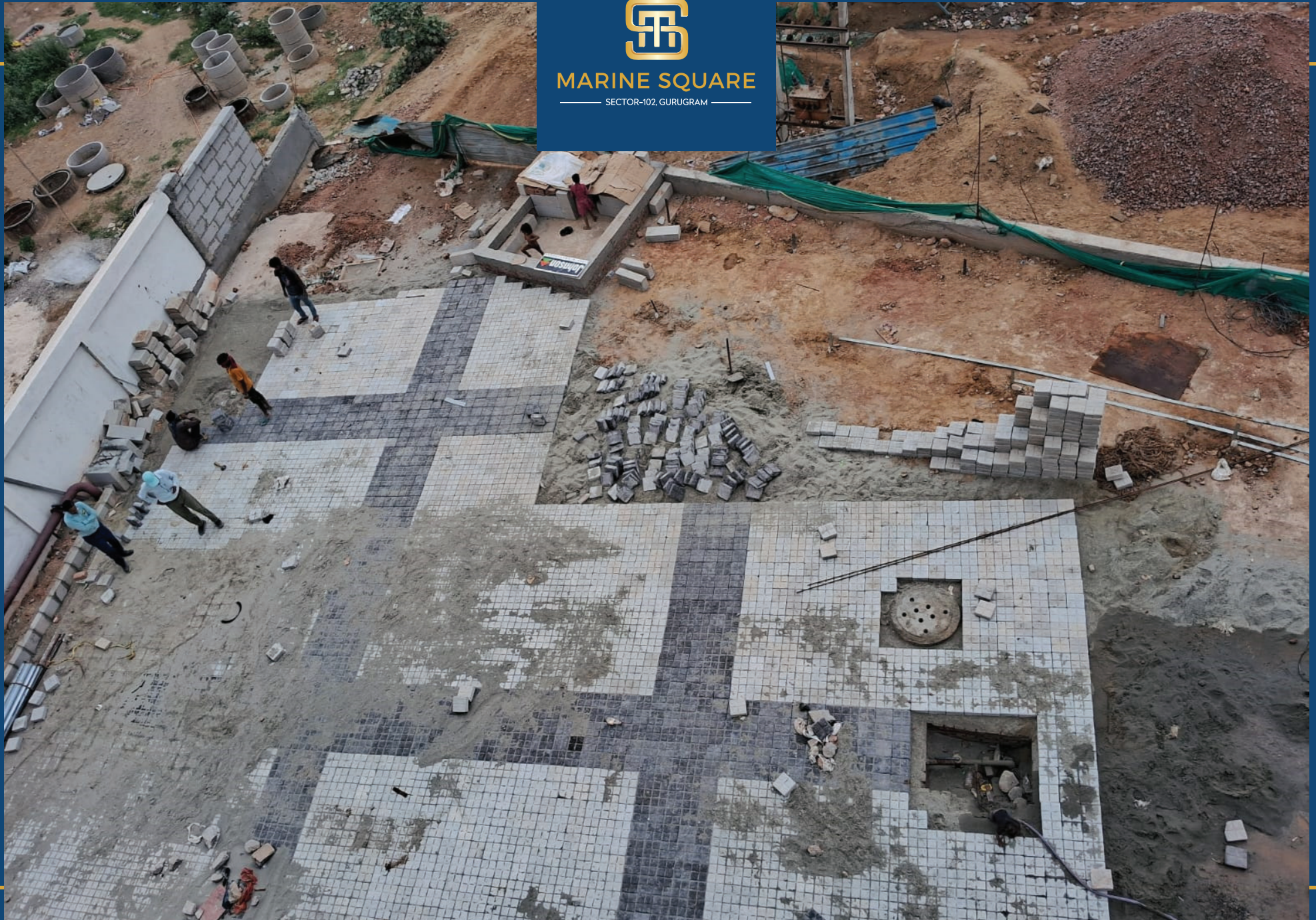
Road Paviour Block Work In Progress
