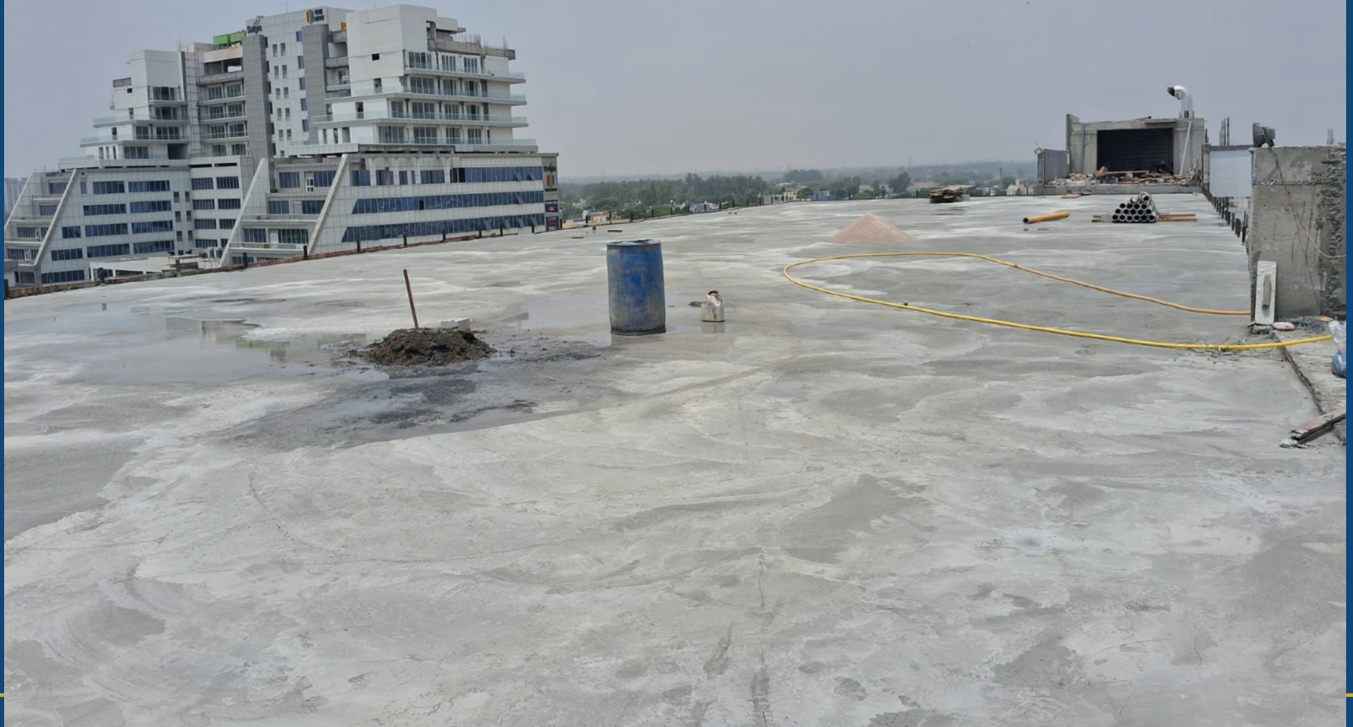
Multiplex Roof Slab Casted
