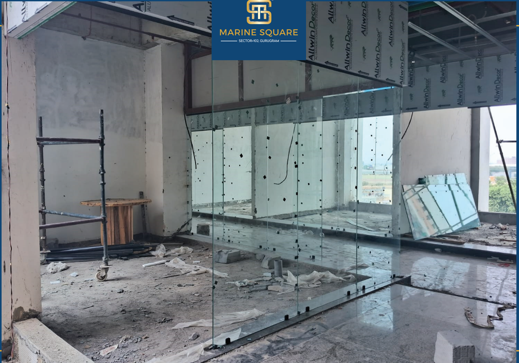
First Floor Glass Work In Progress
