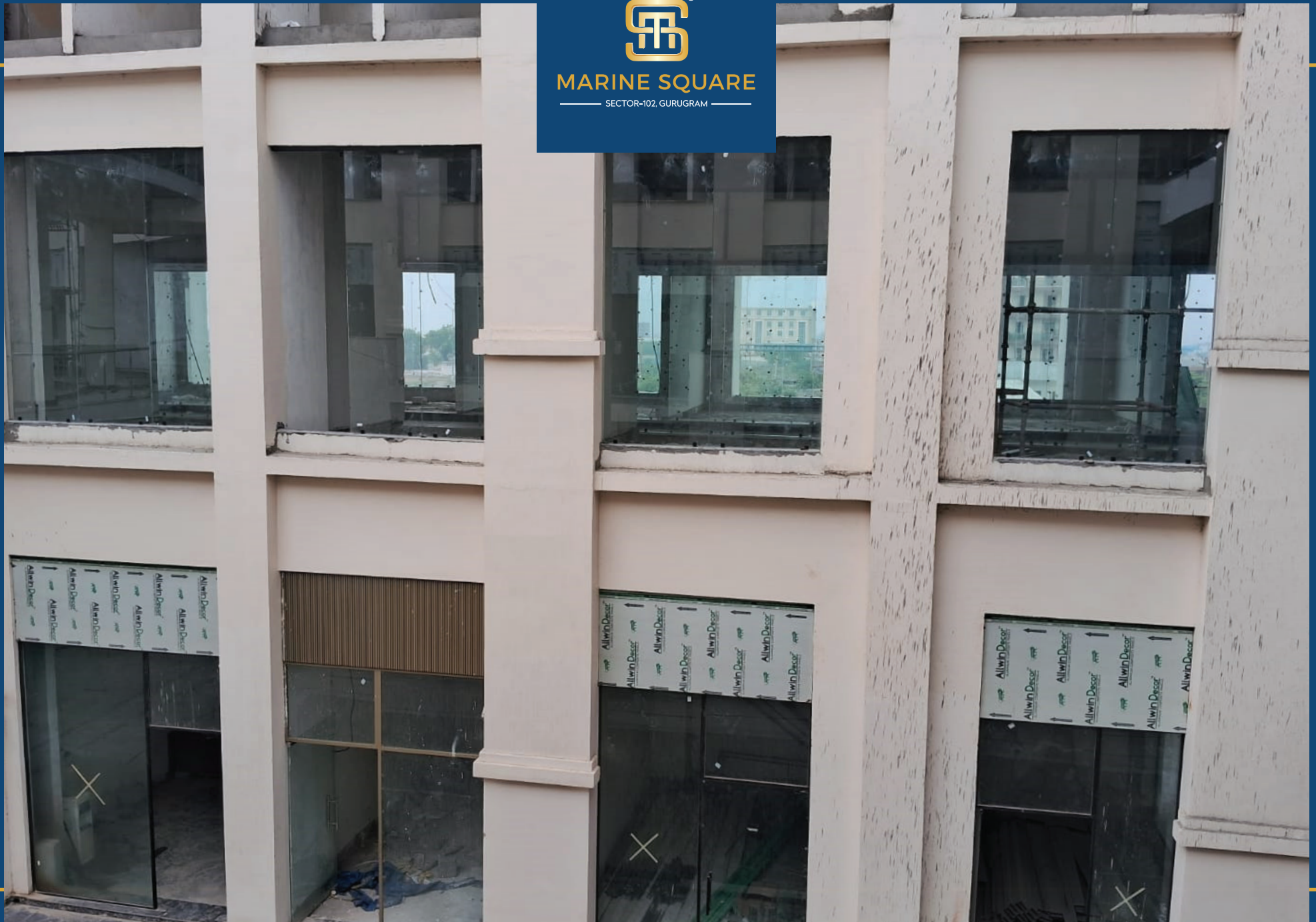
External Glass Work In Progress
