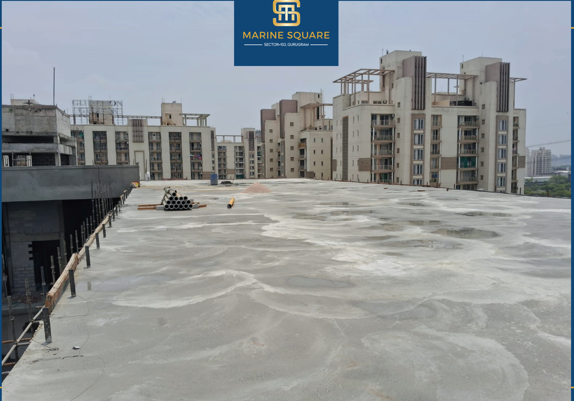
Multiplex Roof Slab Casted
