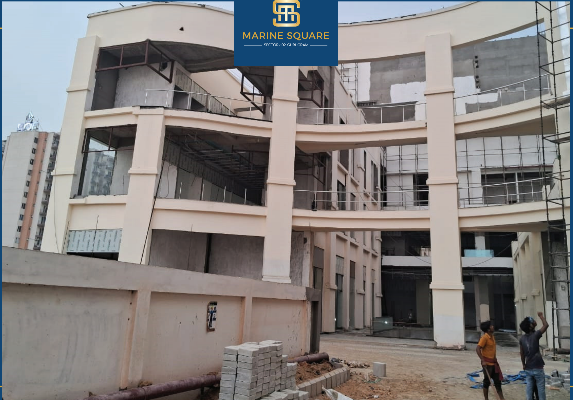
External Glass Work In Progress
