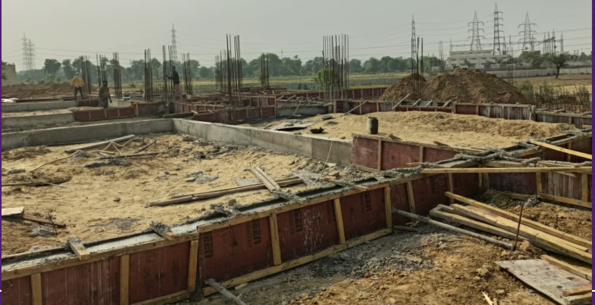
Clubhouse area plinth beam work in progress
