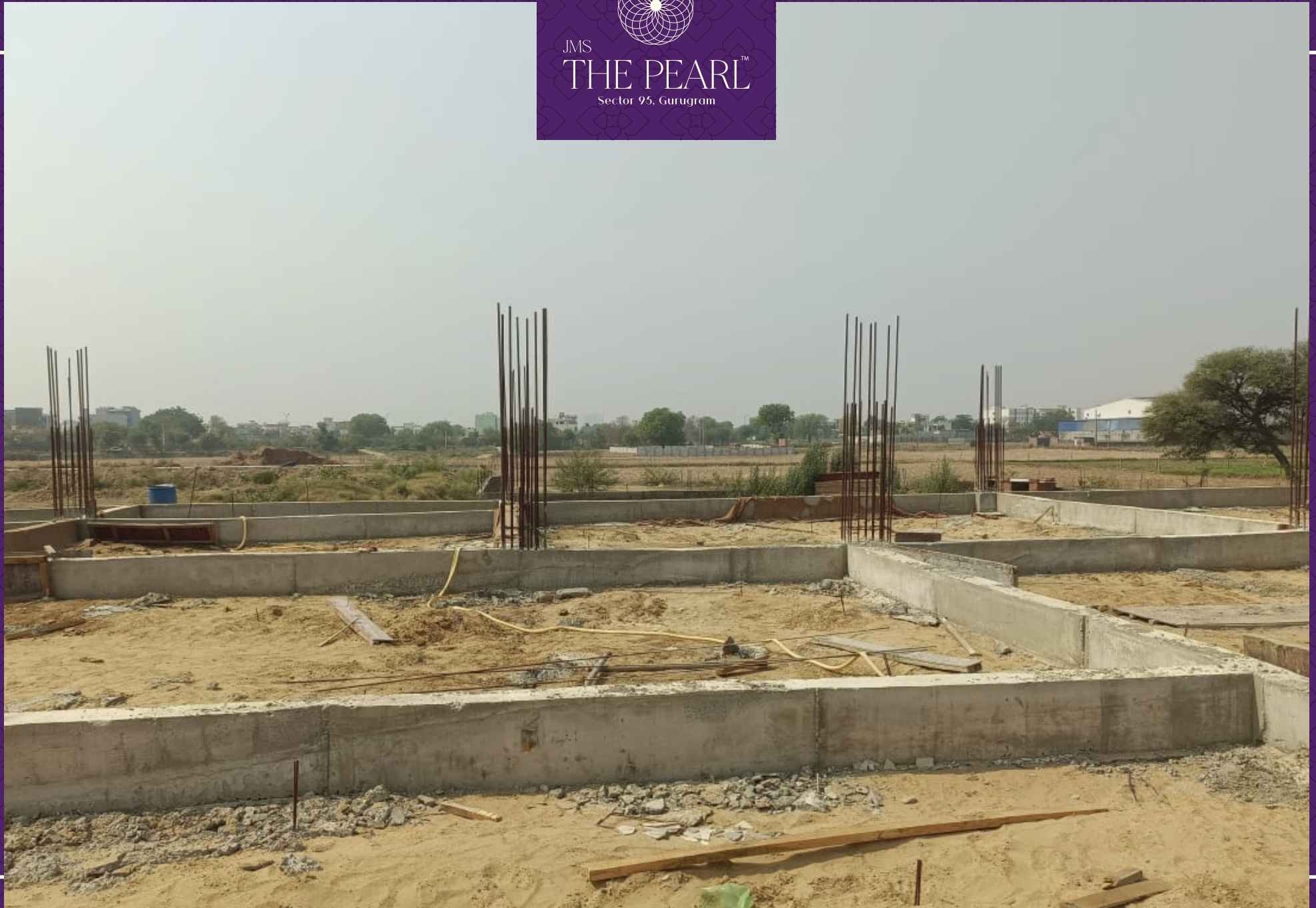
Clubhouse area plinth beam work in progress
