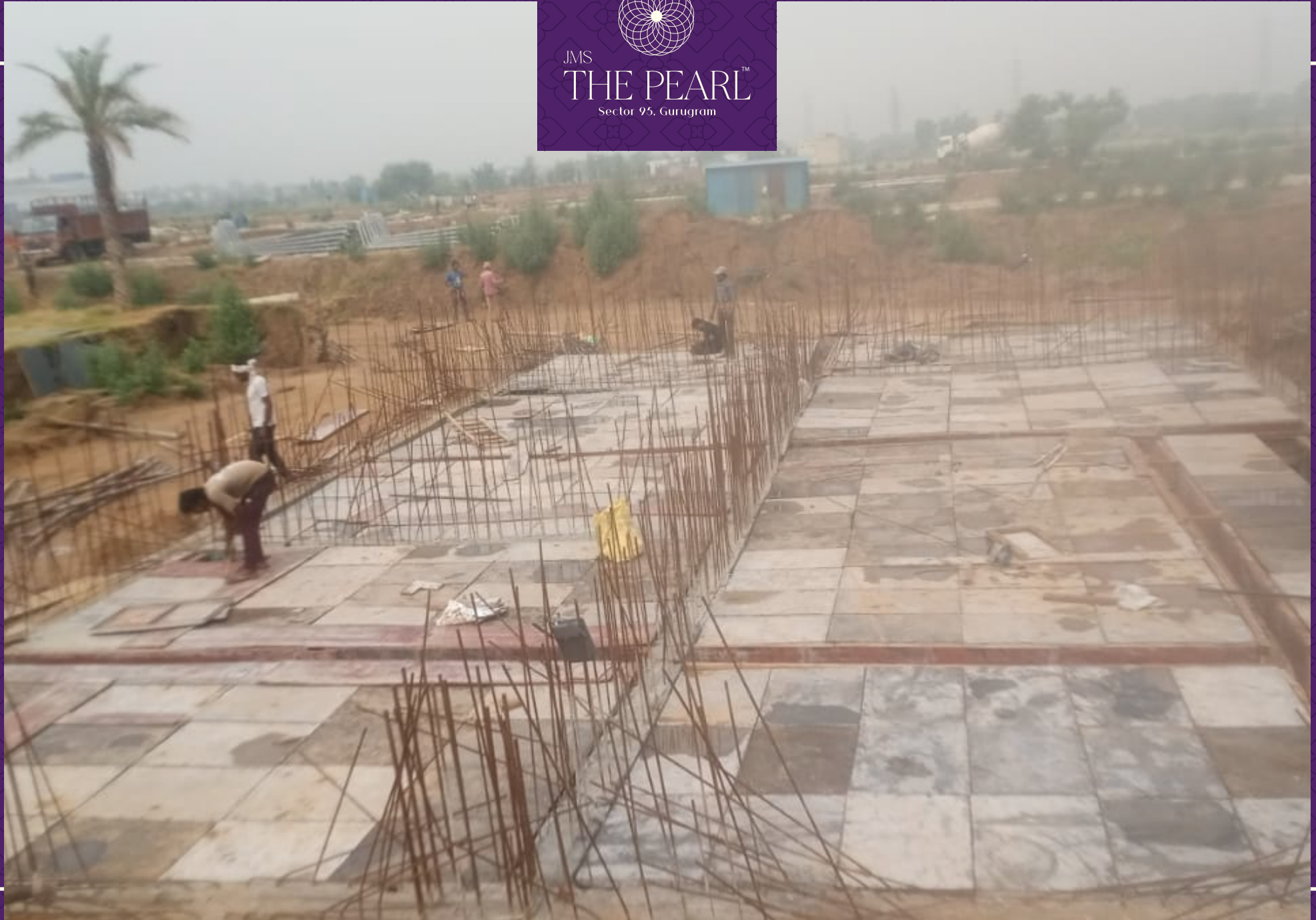
UG Tank slab work in progress
