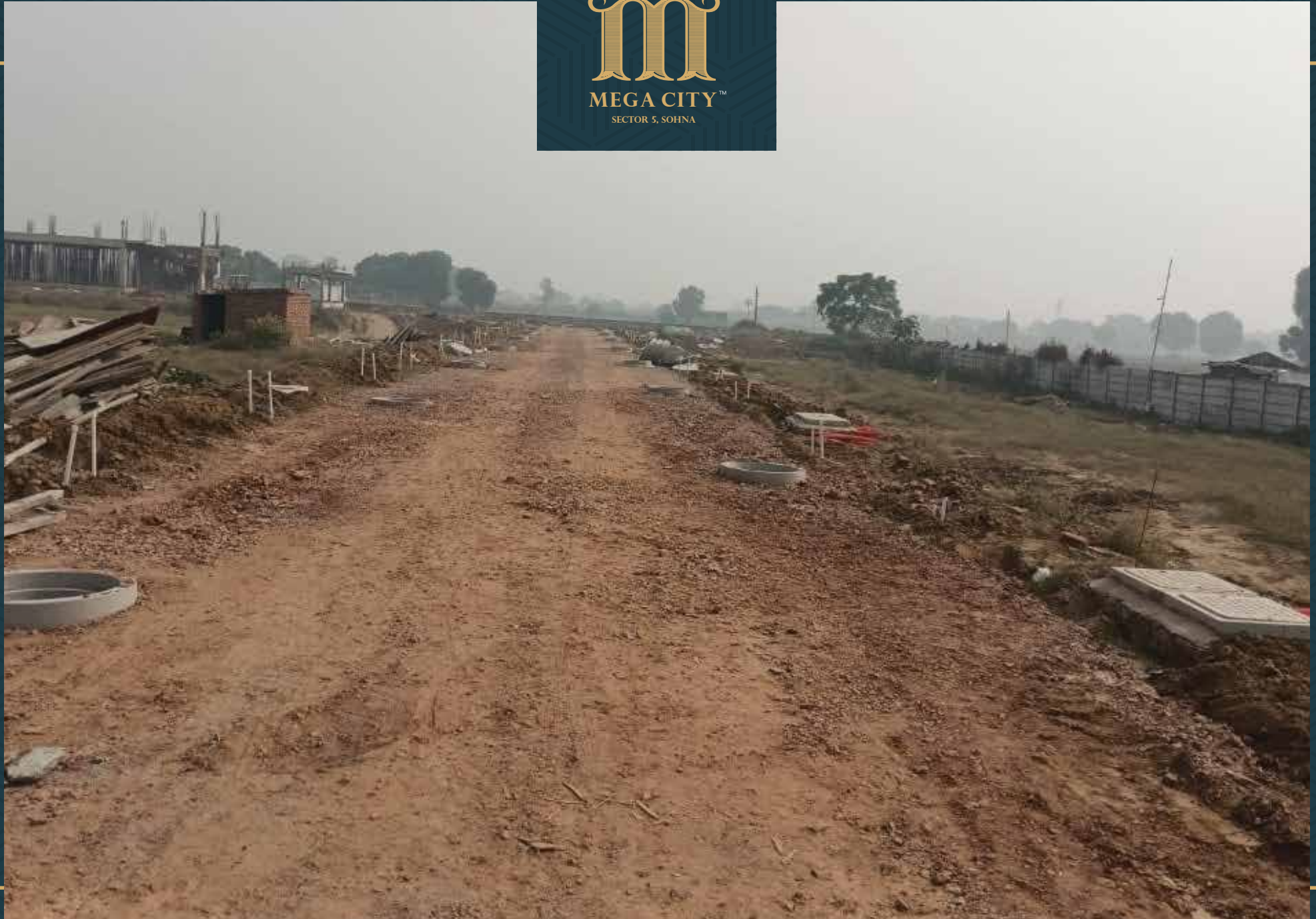
Road no 8. Sewer and storm water lines, water supply lines, electrical cables pipe ducts and road WBM completed. Footpath and Trimix (road finish layer) preparation in progress.
