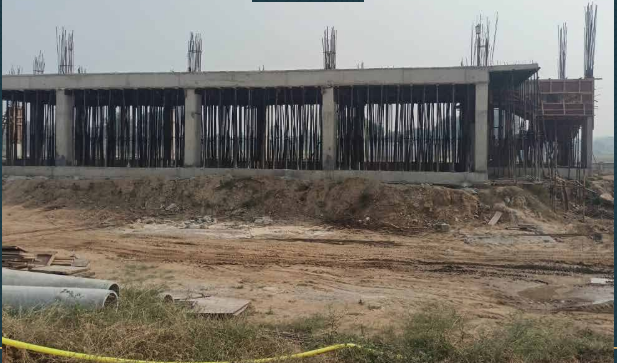
Club and swimming pool structure work in progress. Foundation completed and Ground Floor slab 50% casted
