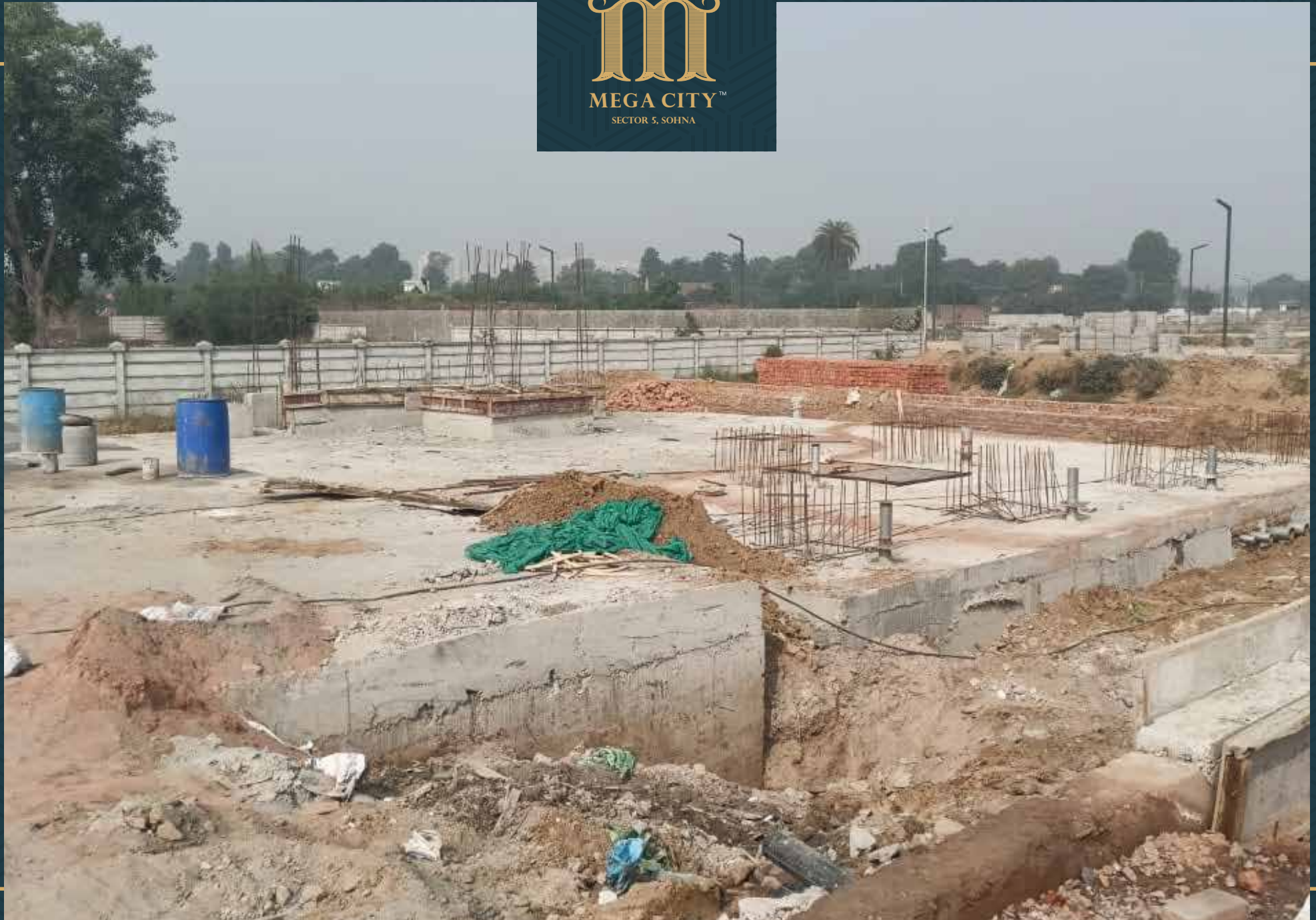
STP and UGT structure work completed and finishing work in progress.
