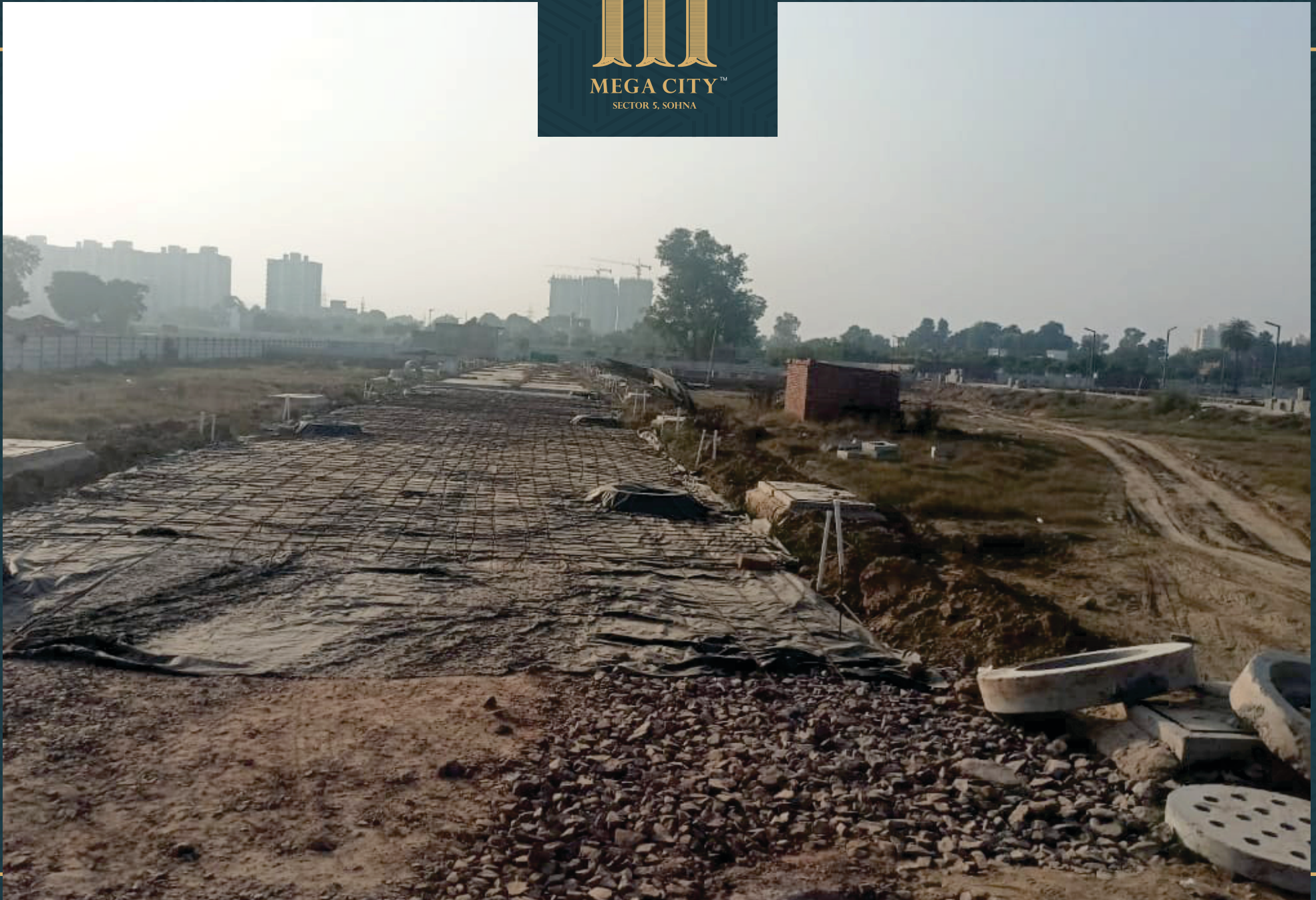
Road no.8 Water supply, sewerage, rain water harvesting, electrical cables, duct pipes and road base completed. Trimix and footpath work in progress
