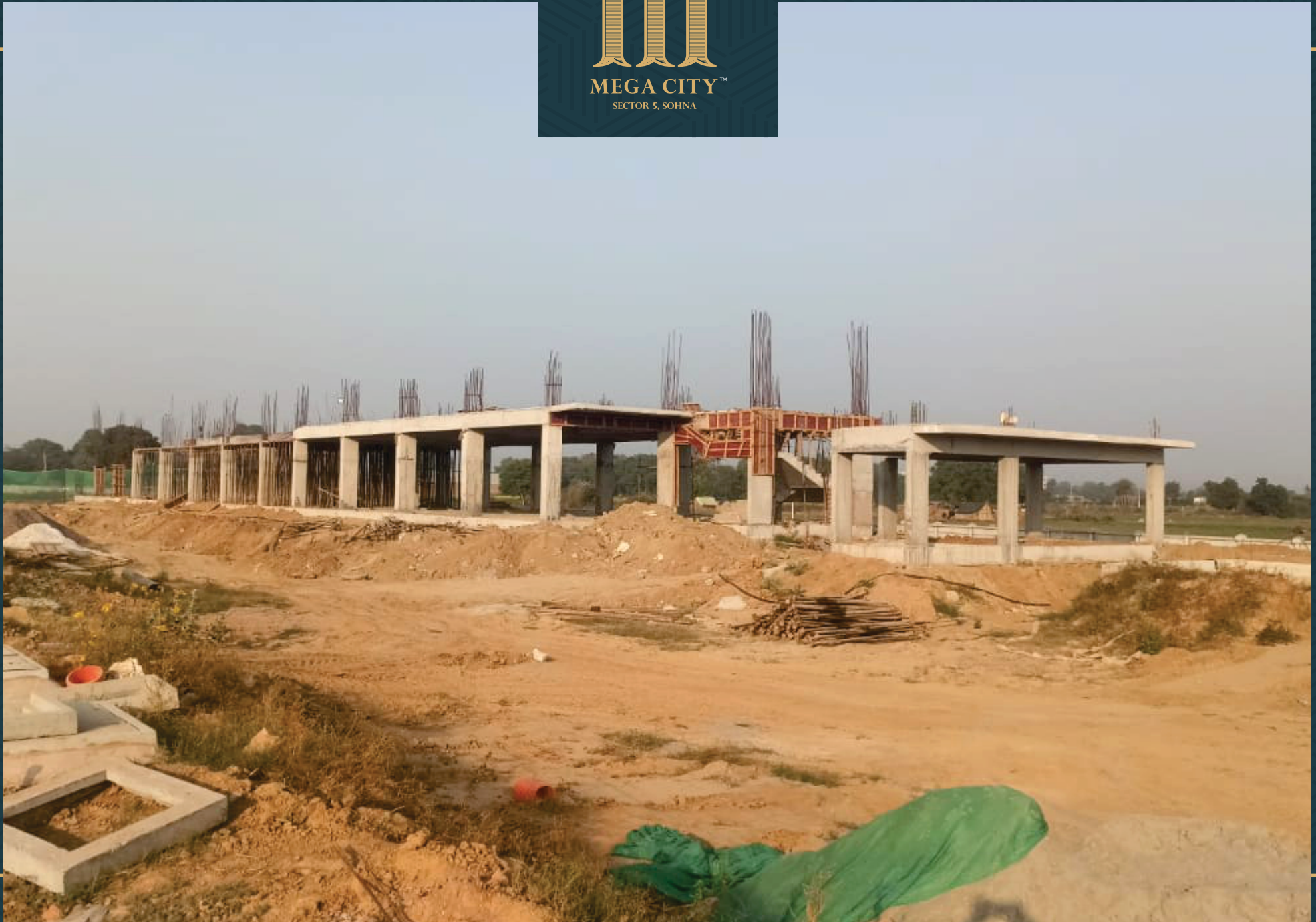
Ground Floor slab for Club & swimming area - 60% completed
