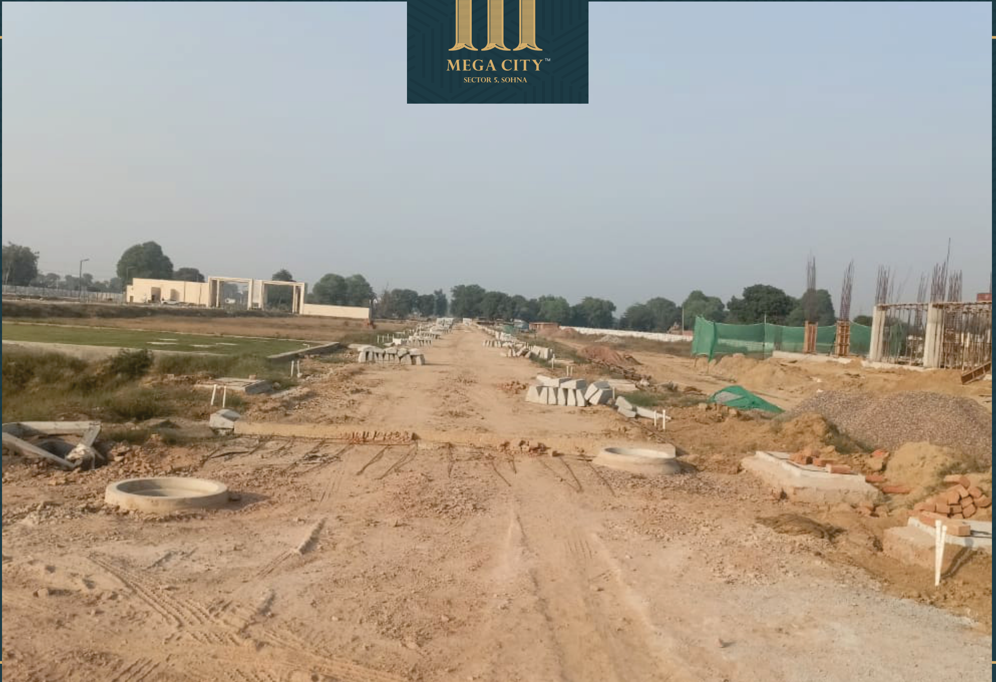
Road no.5 Water supply, sewerage, rain water harvesting, electrical cables, duct pipes and road base completed. Trimix and footpath work in progress
