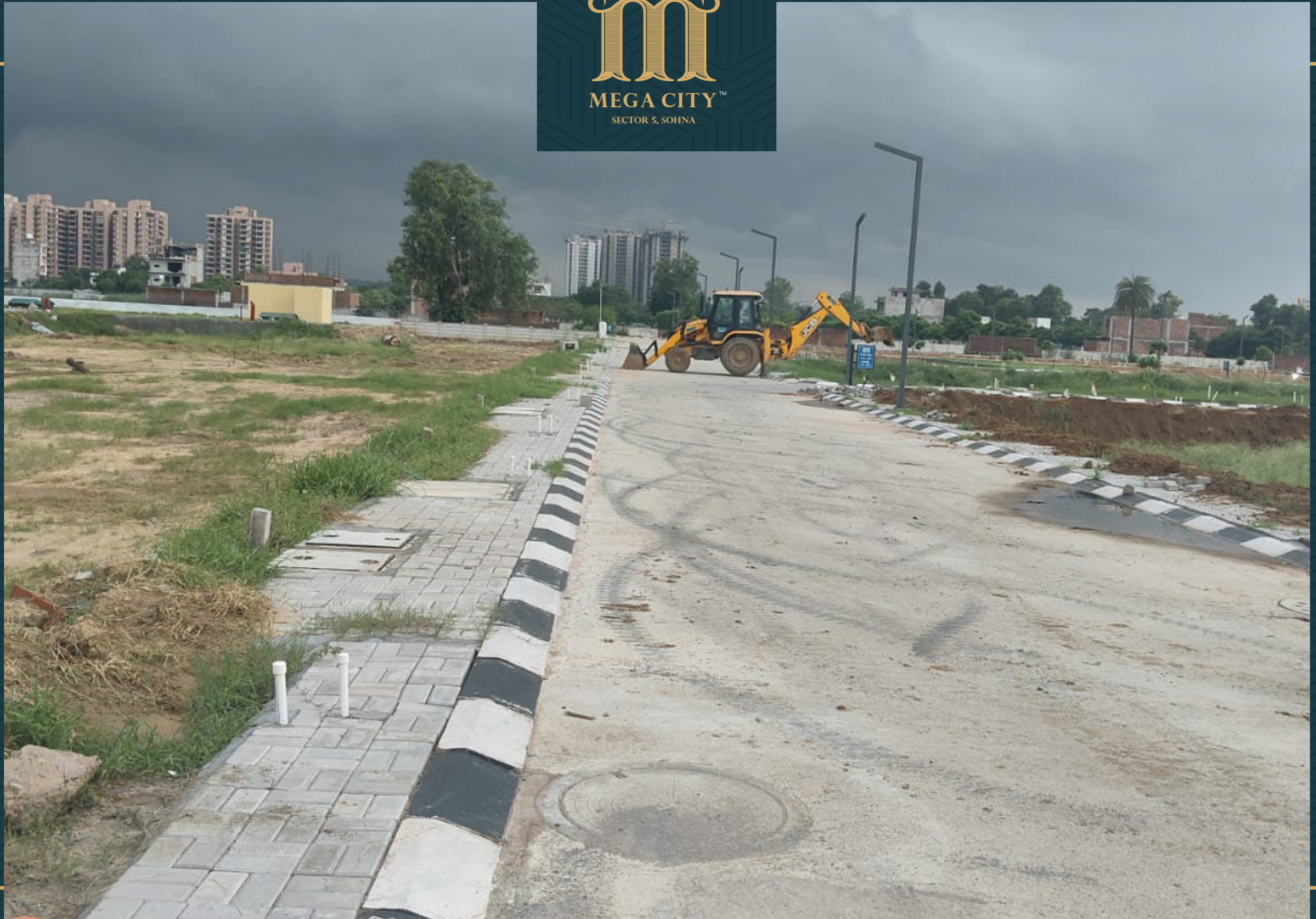
Road No. 7 Electrical cable laying work in progress
