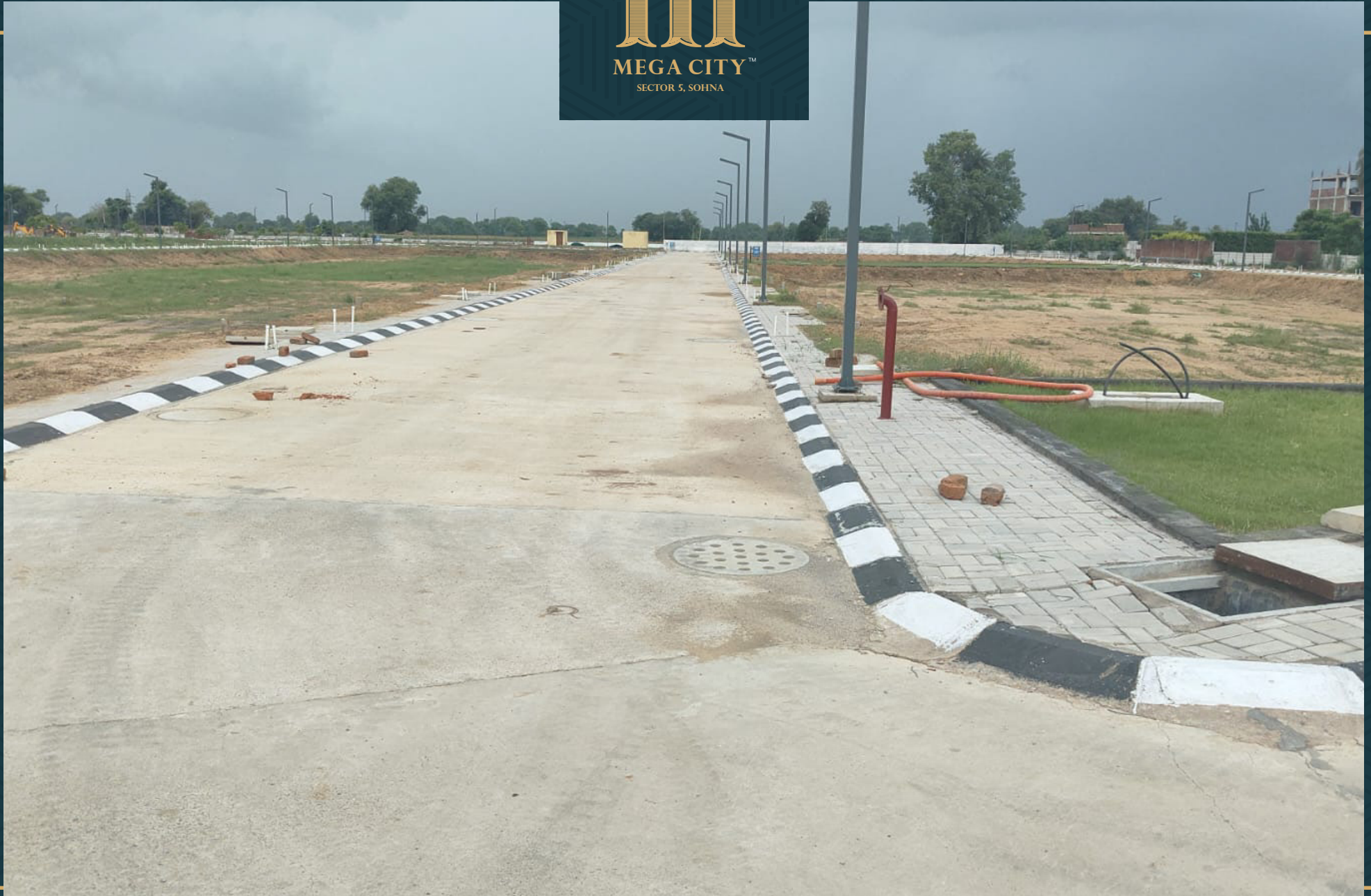
Road No. 2 Electrical cable laying work in progress
