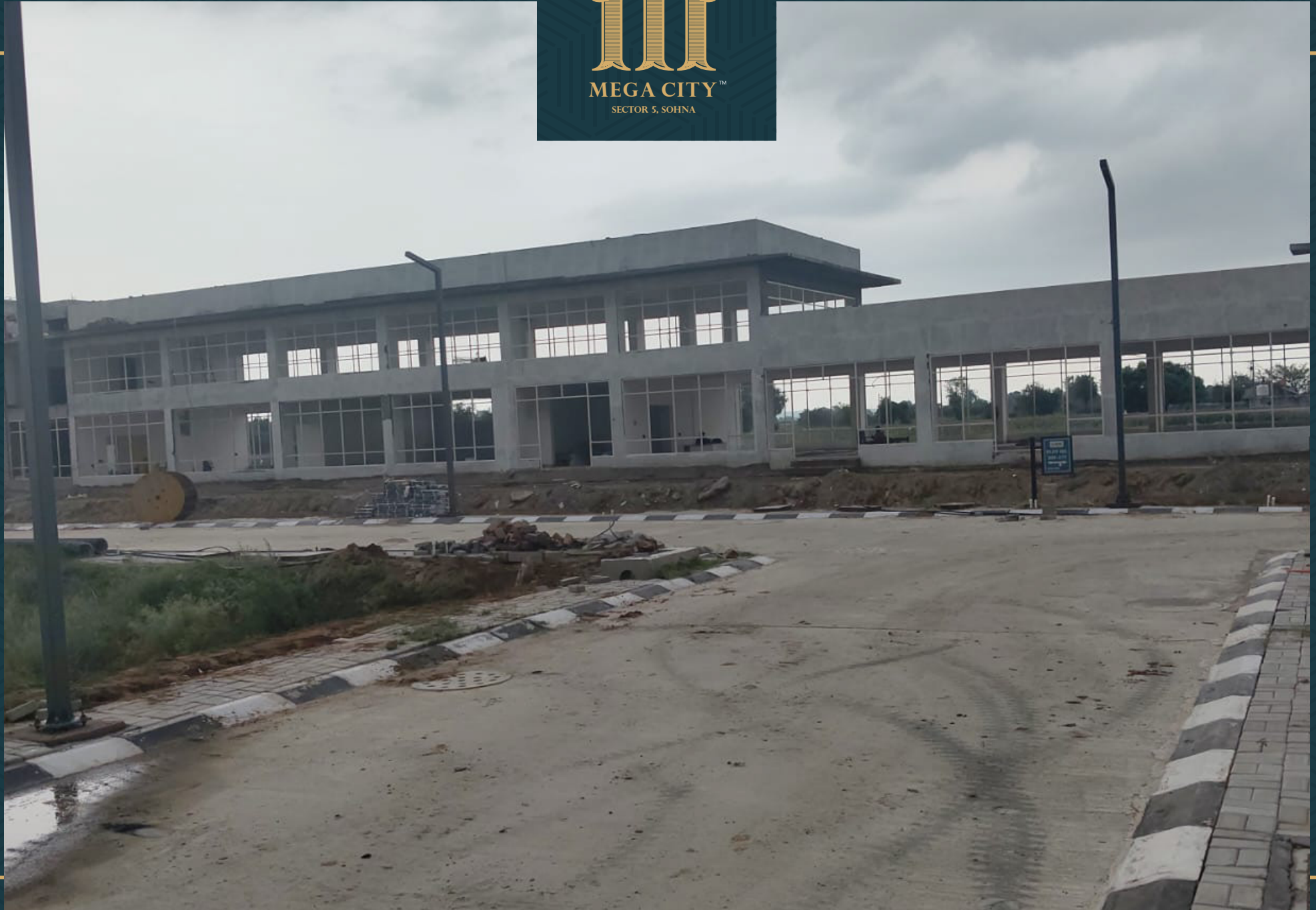
Club House work - 80% completed
