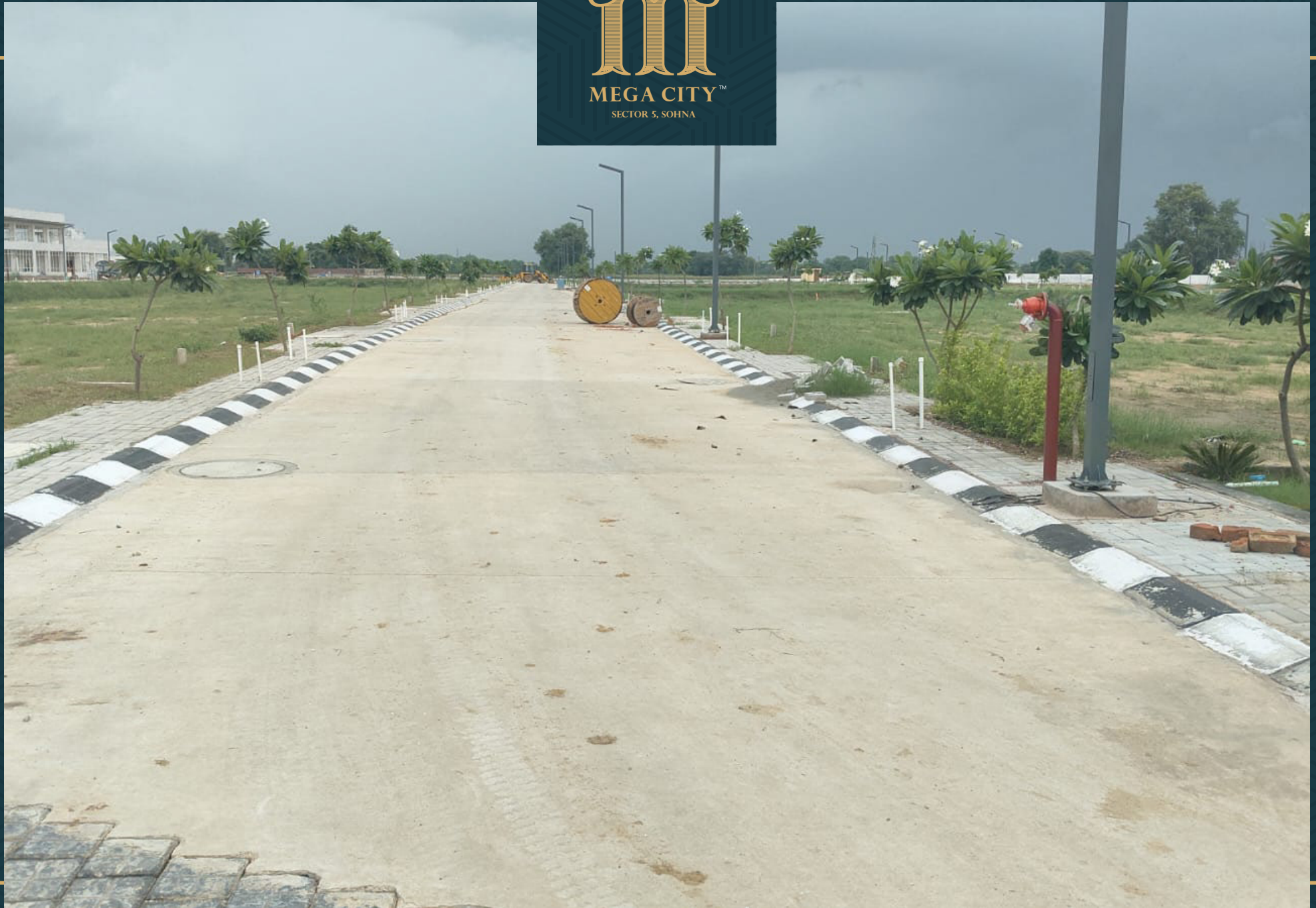
Road No. 4 Electrical cable laying work in progress
