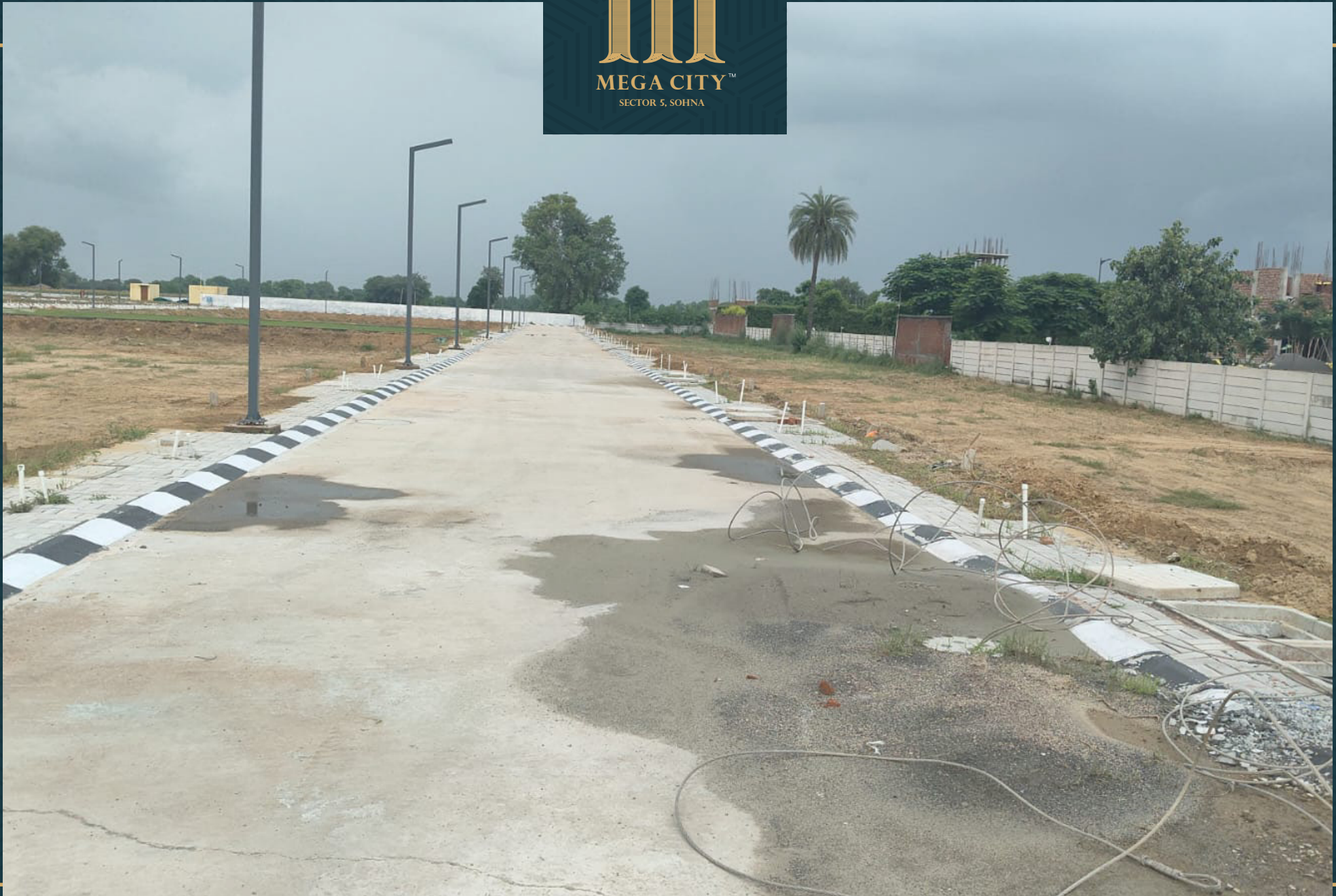
Road No. 1 Electrical cable laying work in progress
