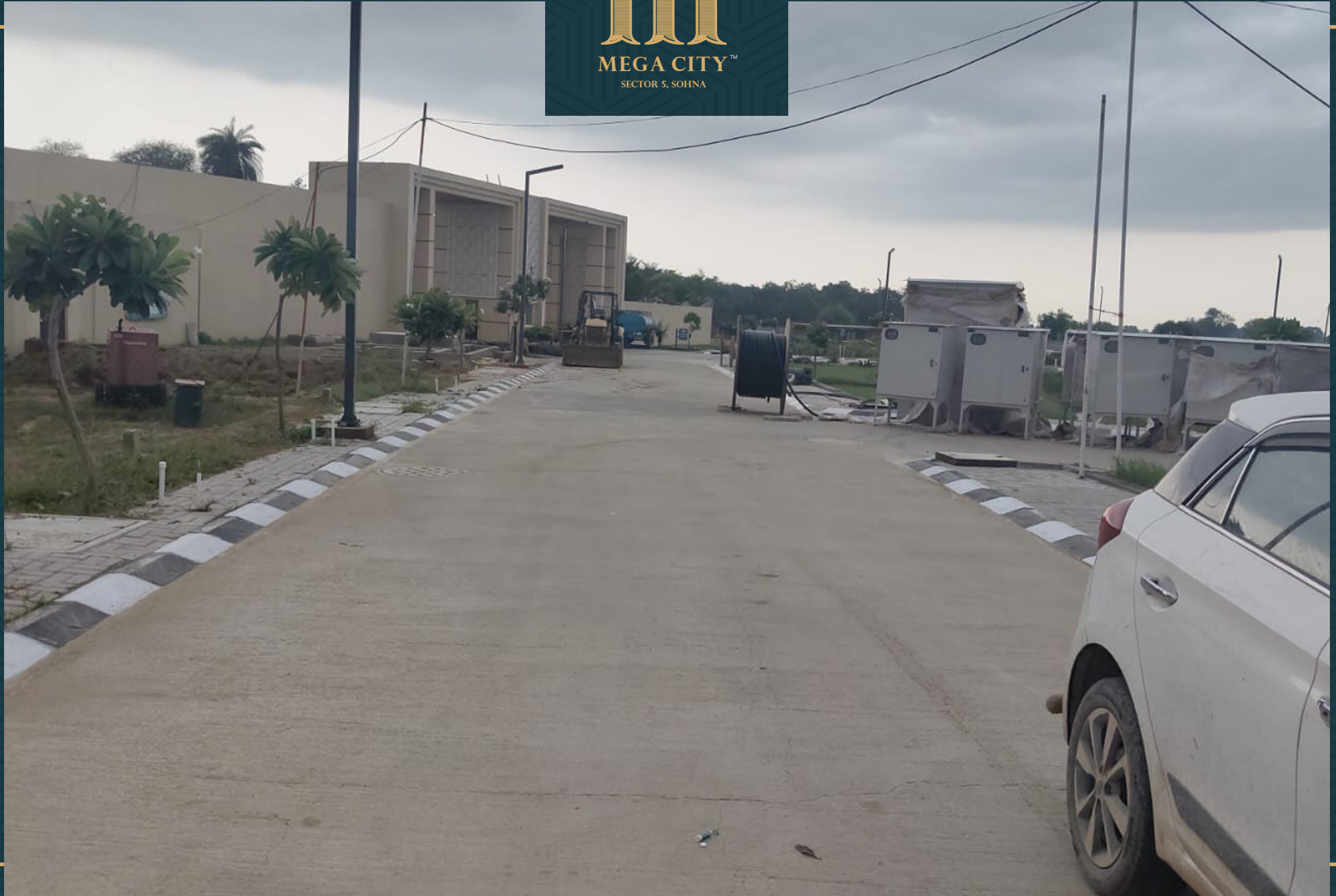
Road No. 6 Electrical cable laying work in progress
