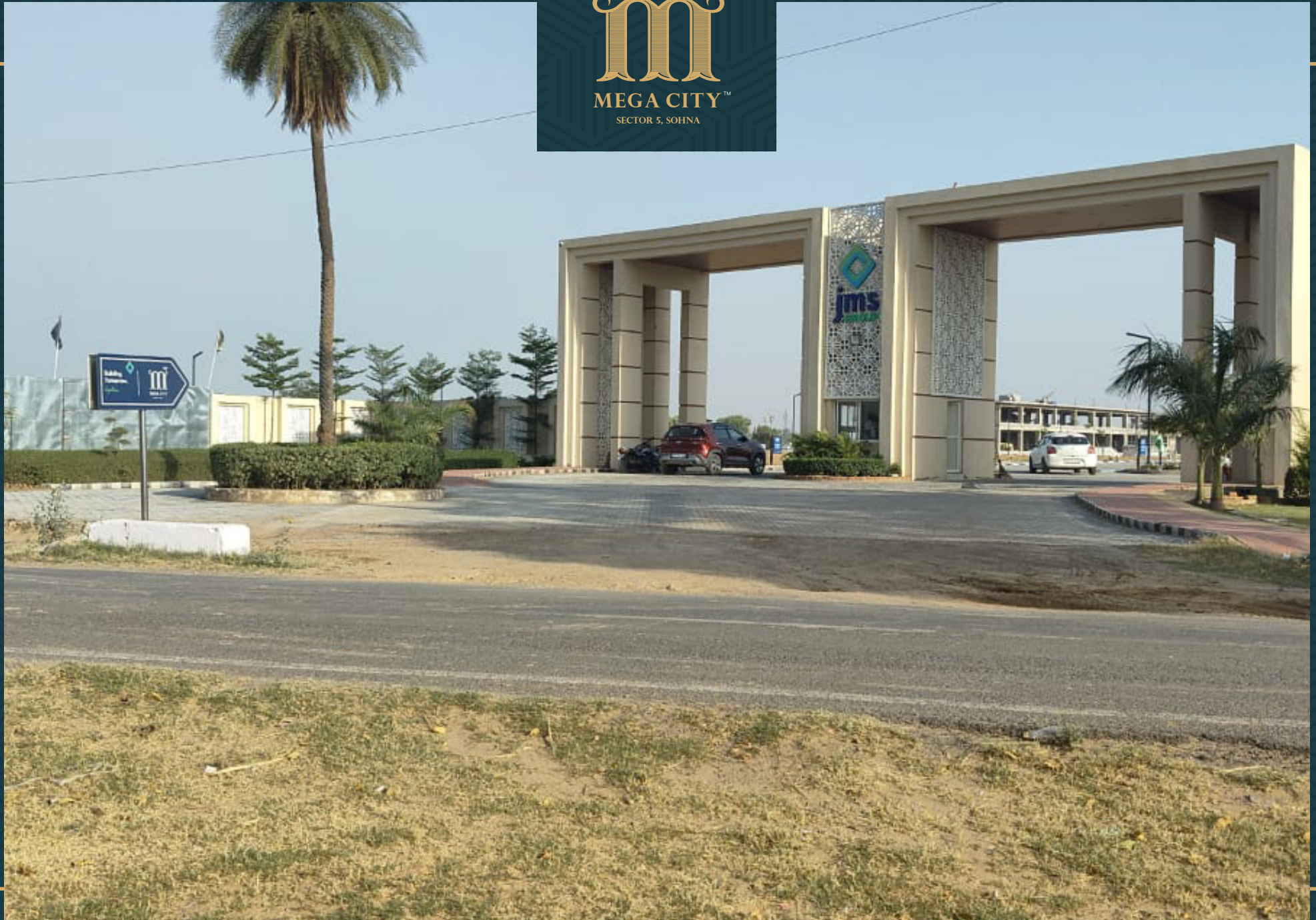
Entry Gate work completed
