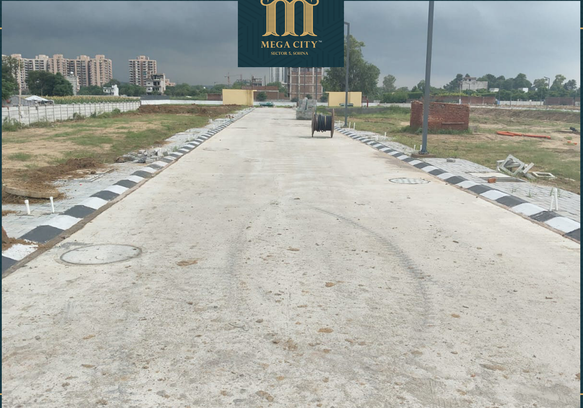
Road No. 8 Electrical cable laying work in progress
