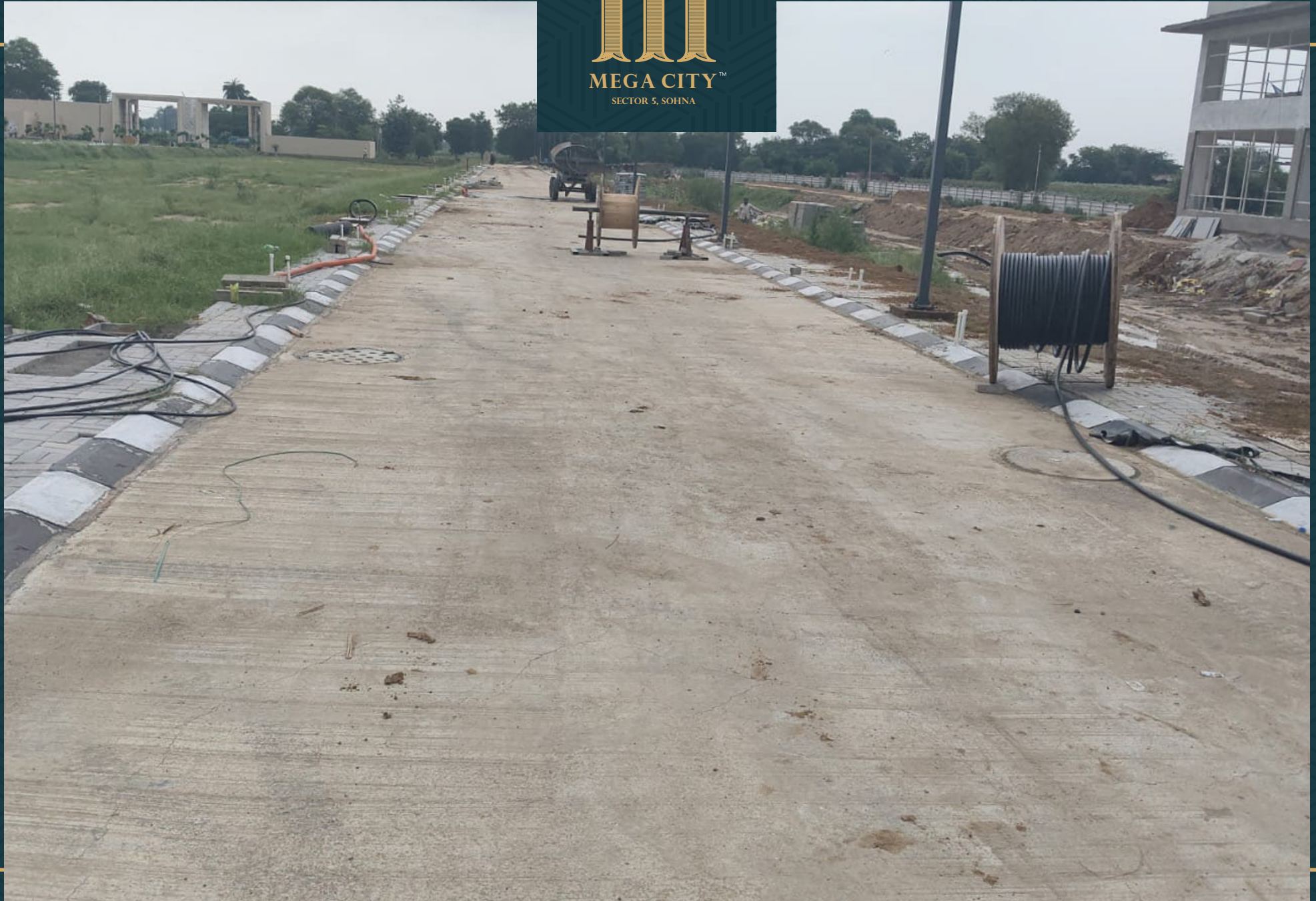
Road No. 5 Electrical cable laying work in progress
