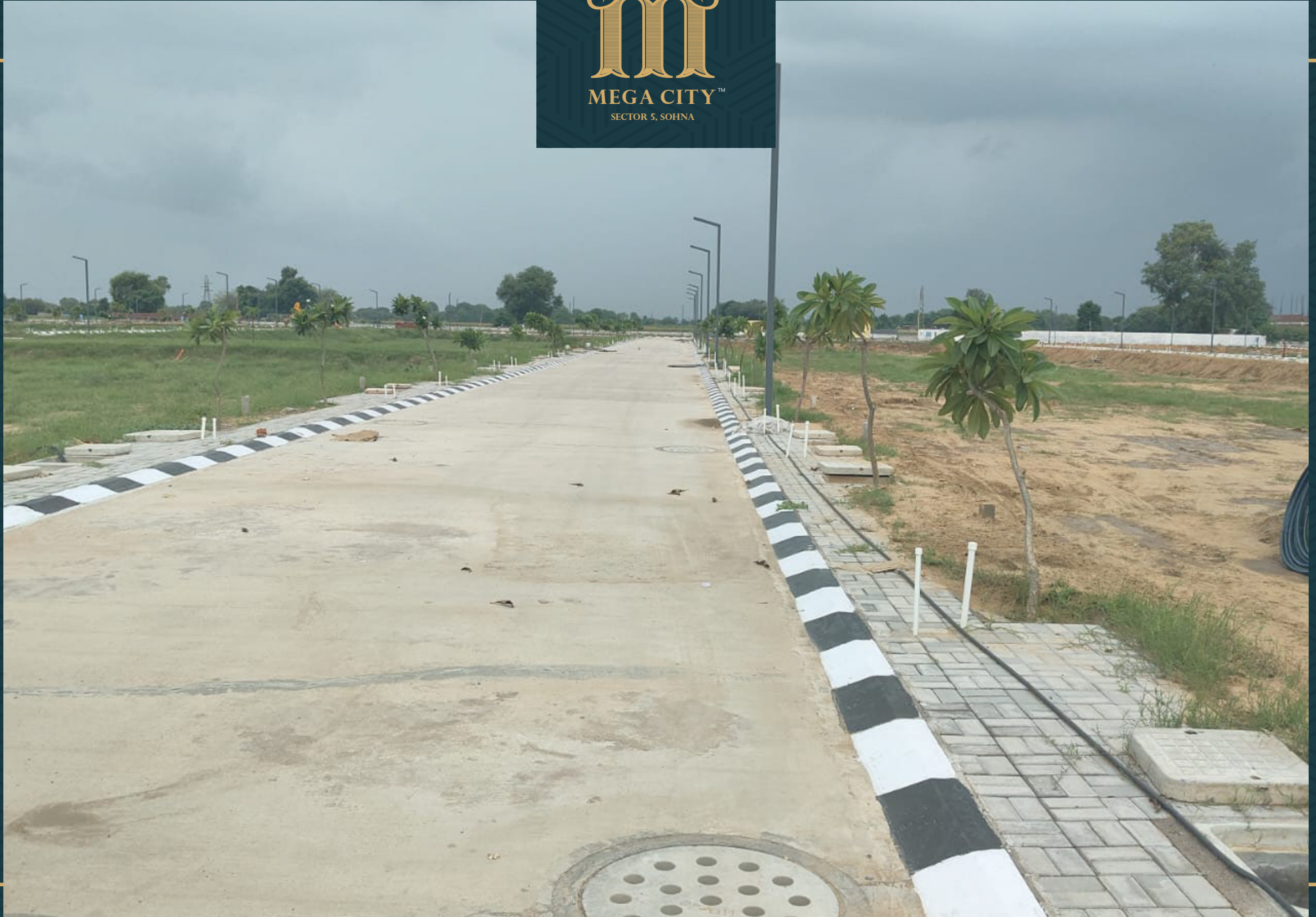
Road No. 3 Electrical cable laying work in progress
