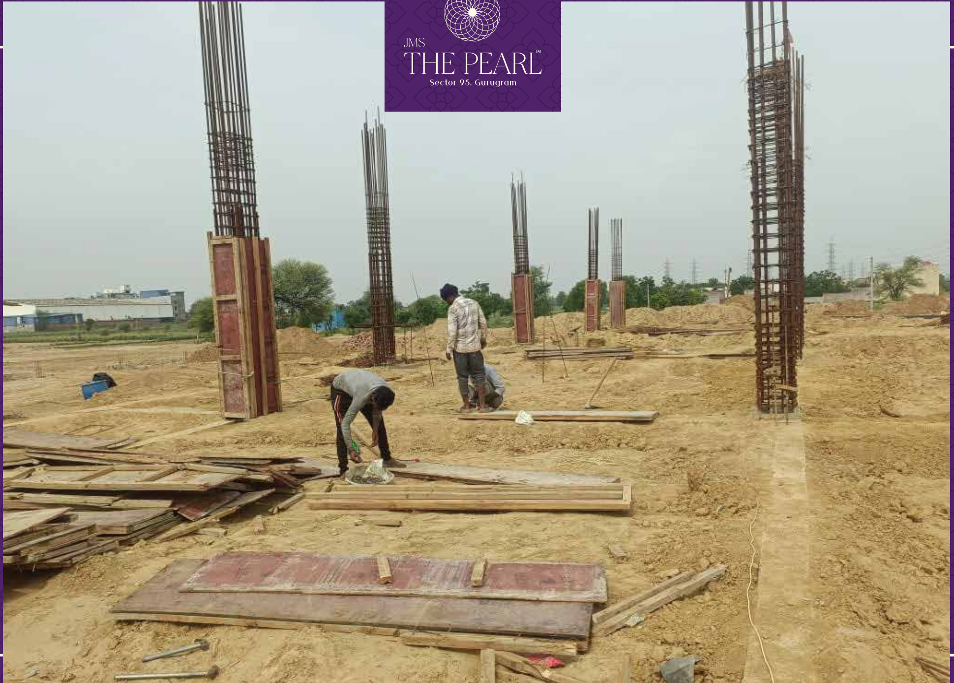
Clubhouse Construction work in progress
