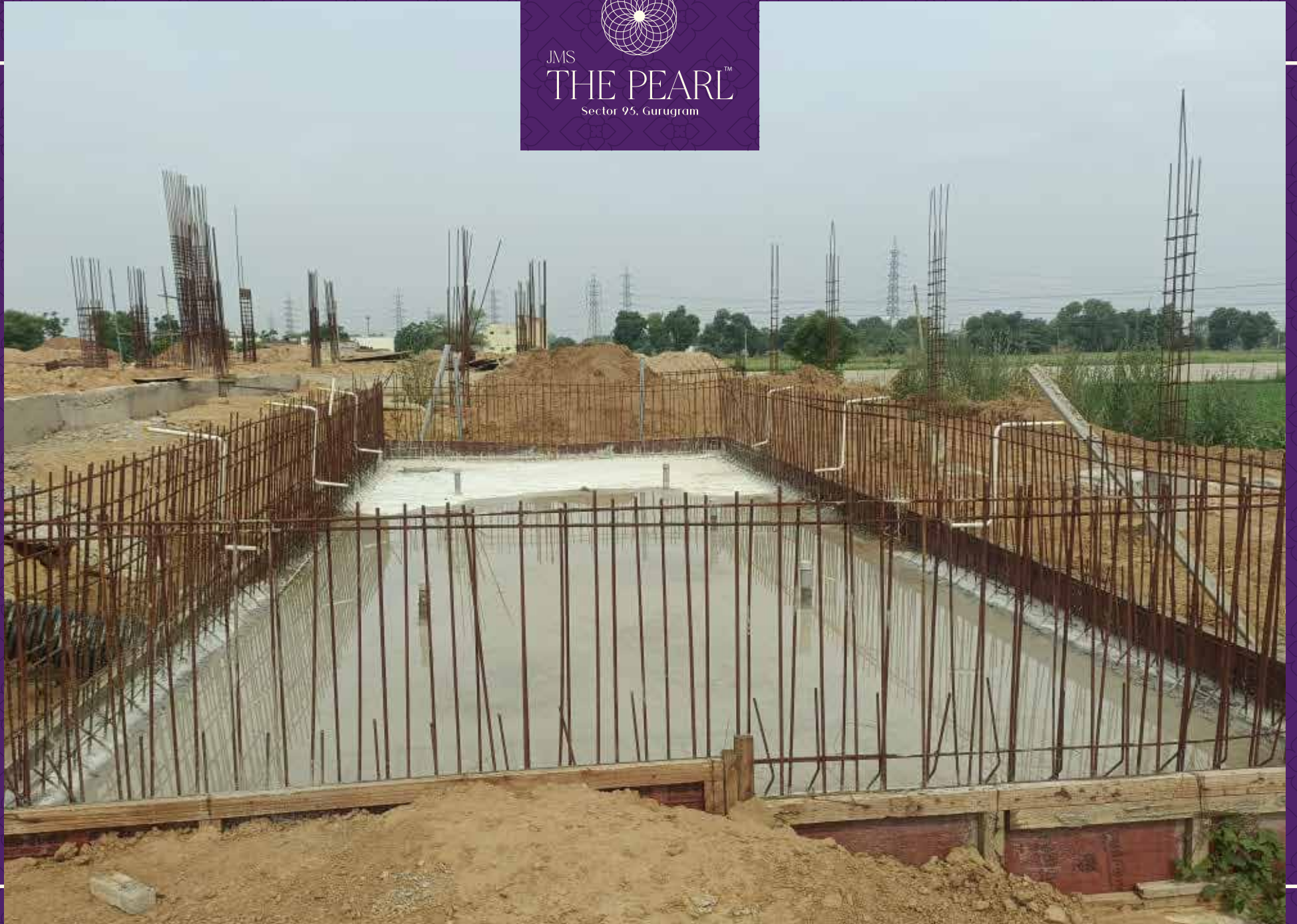
Clubhouse Construction work in progress
