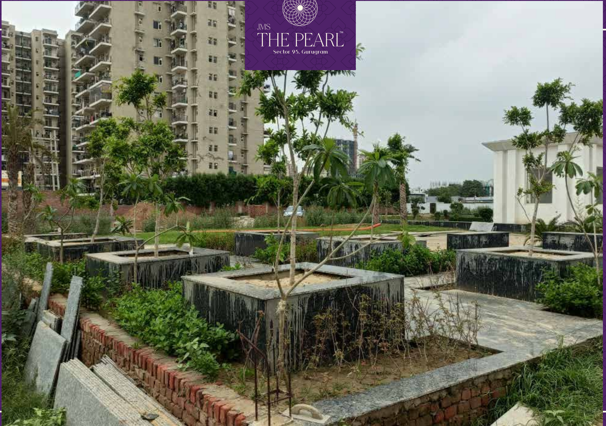
Green Area development work in progress
