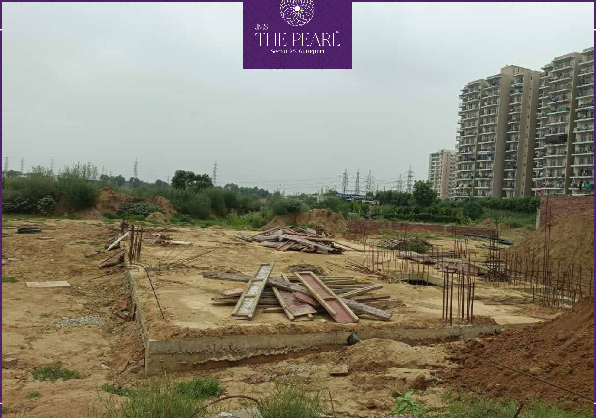
STP Construction work in progress
