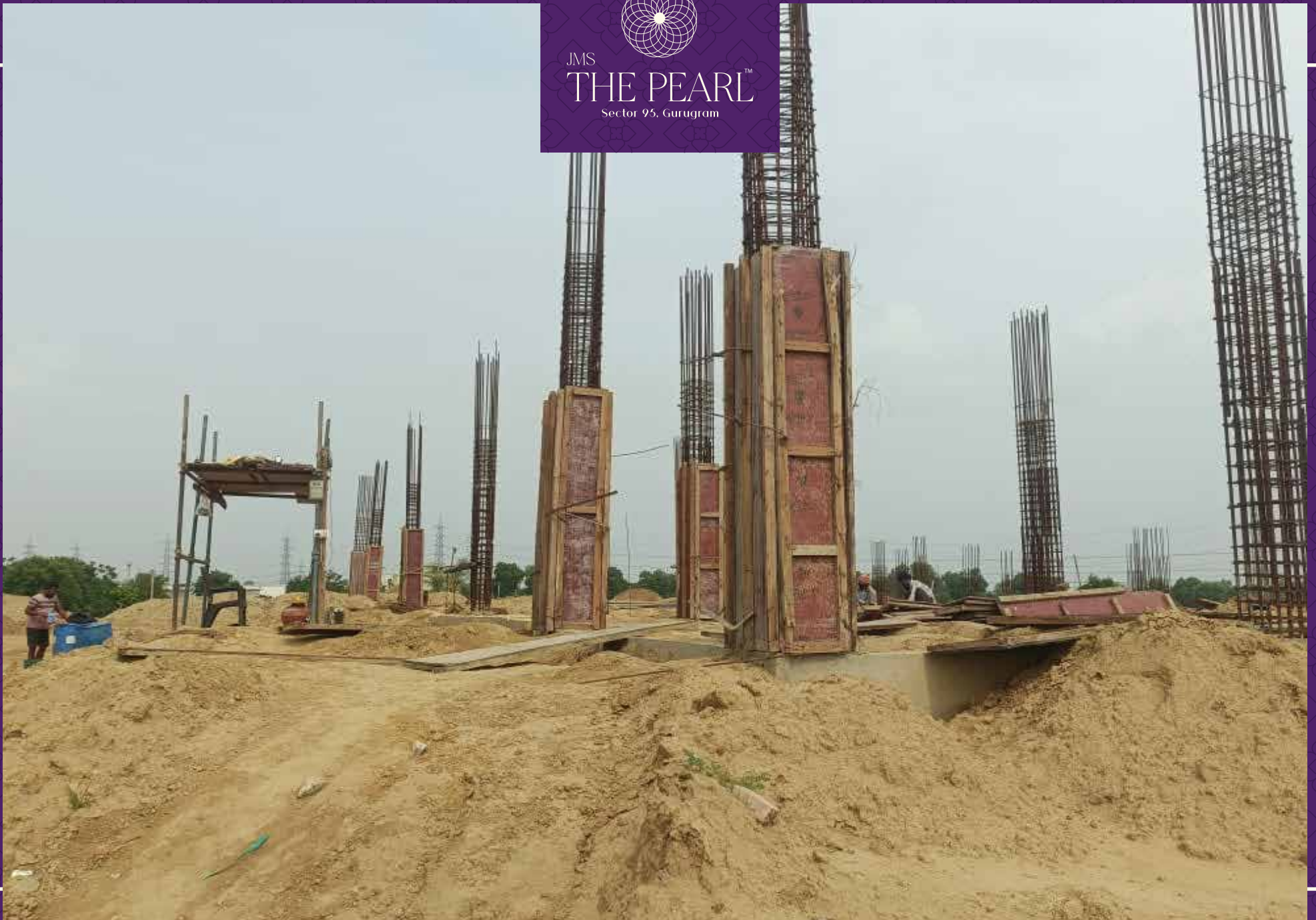
Clubhouse Construction work in progress
