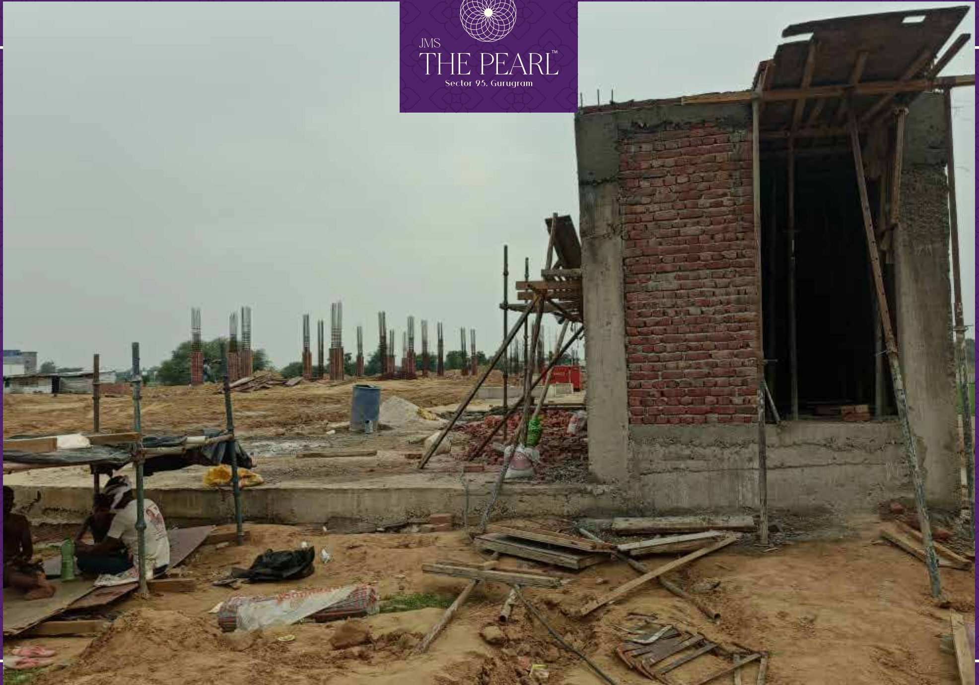
STP Construction work in progress
