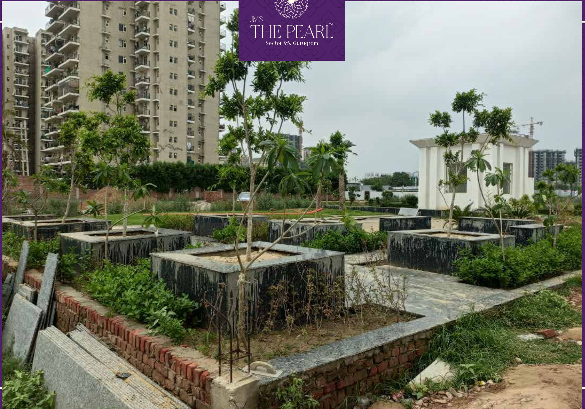
Green Area development work in progress
