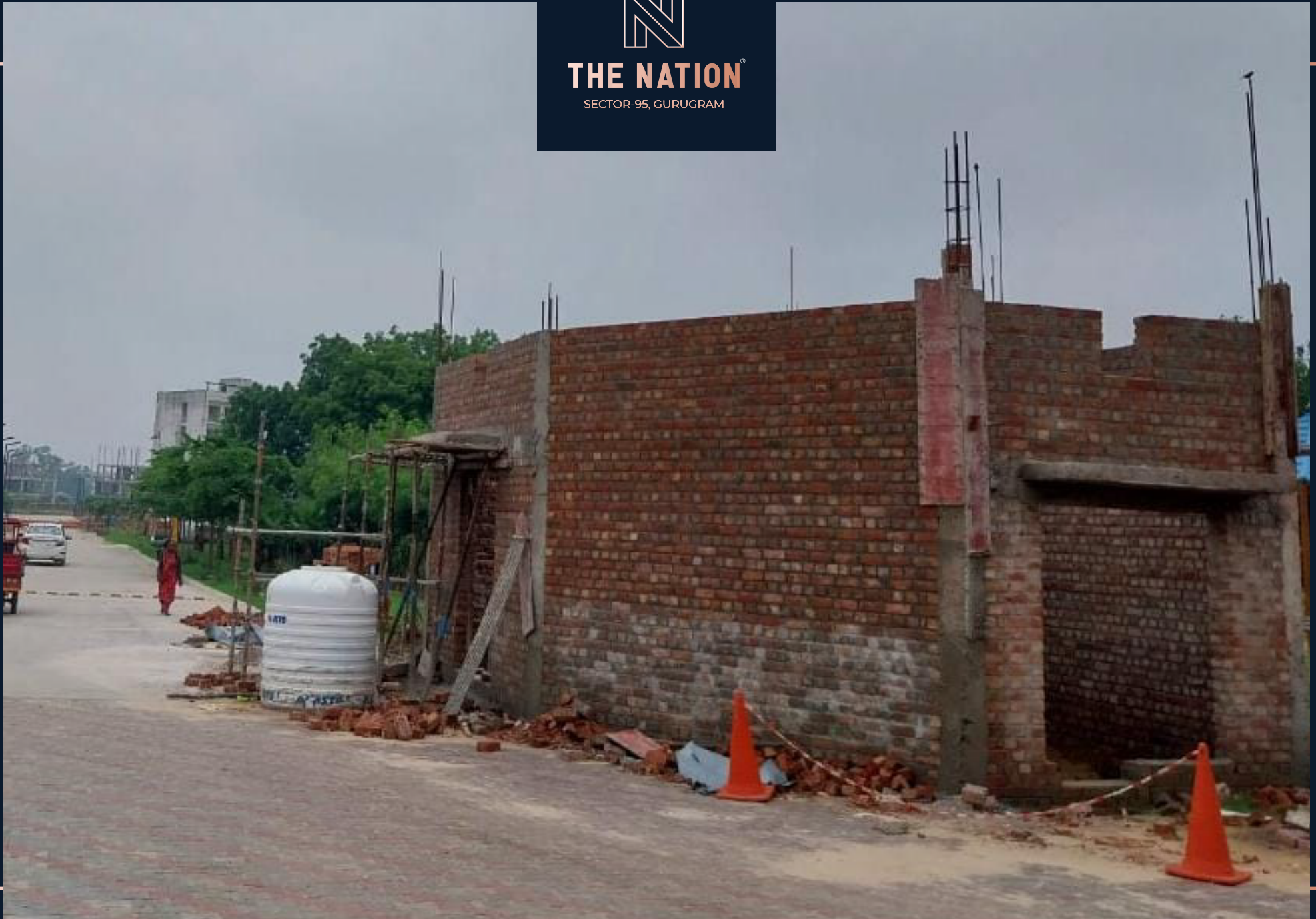
Electrical room construction work in progress
