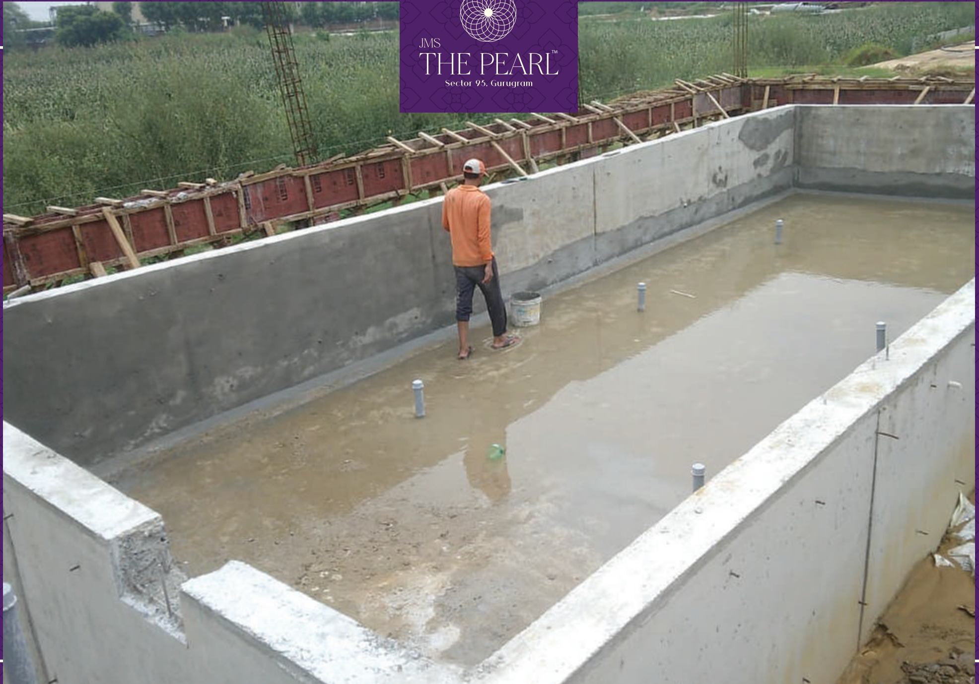
Club House construction work in progress
