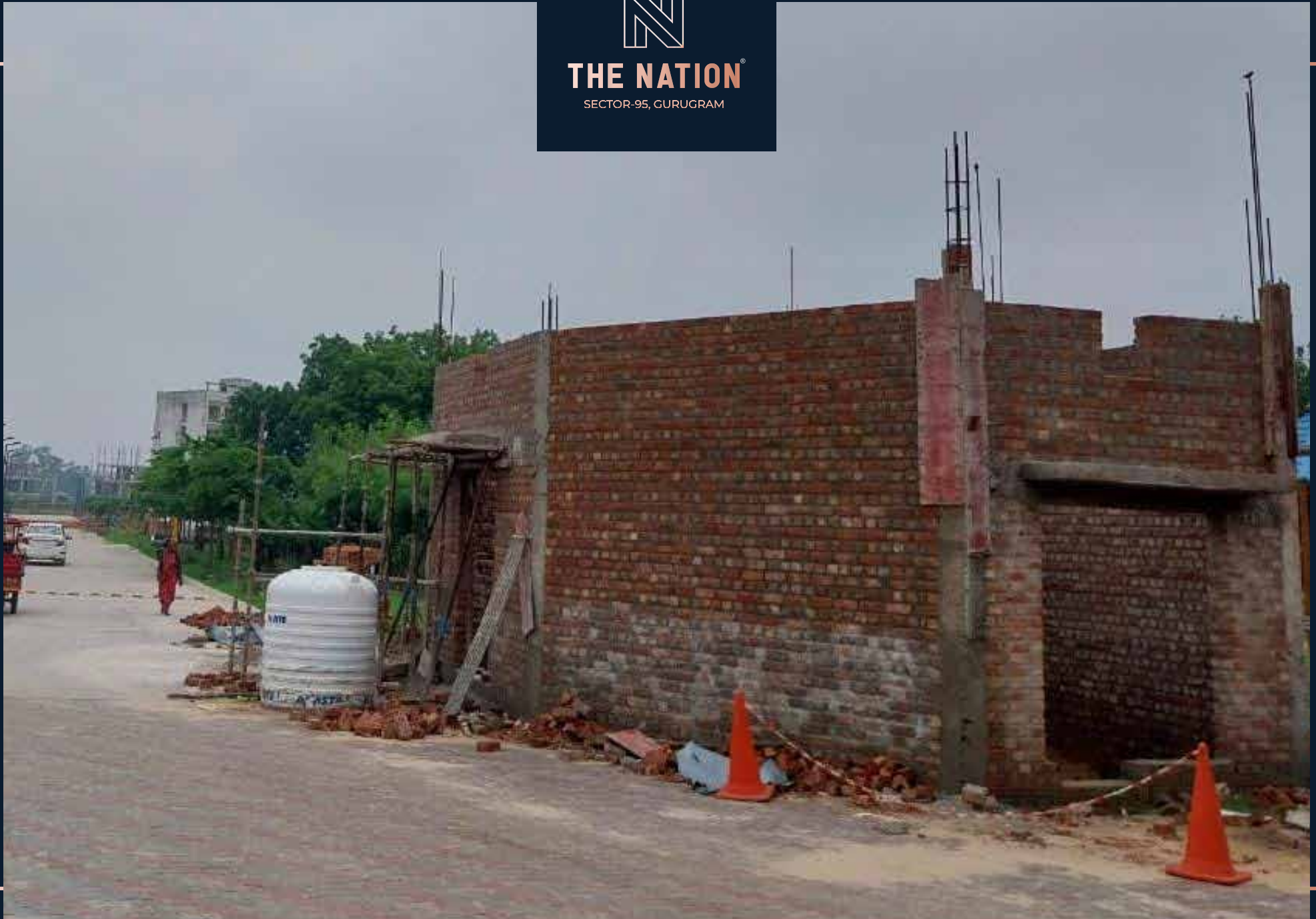
Electrical room construction work in progress
