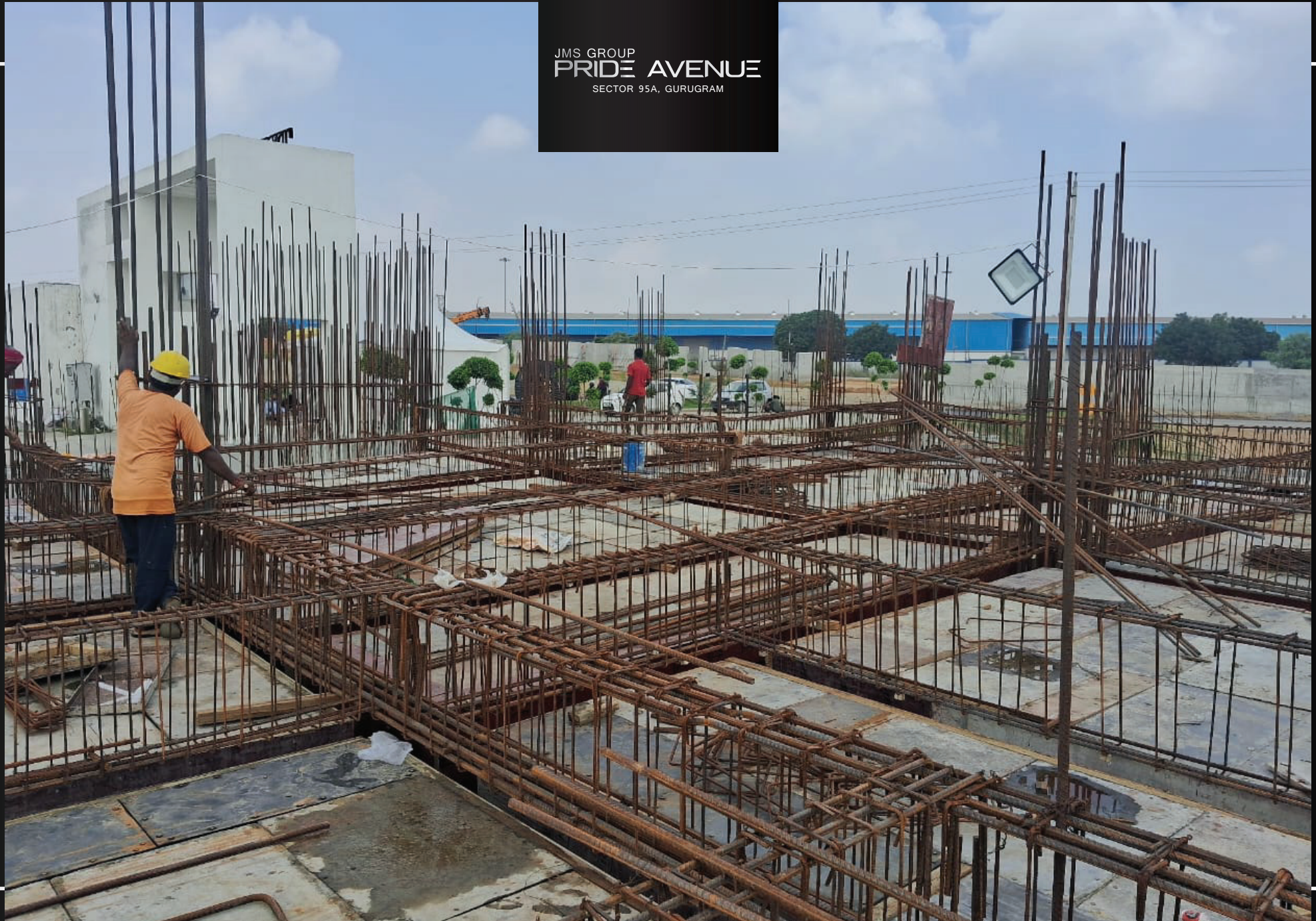
Ground floor slab beam reinforcement work in progress
