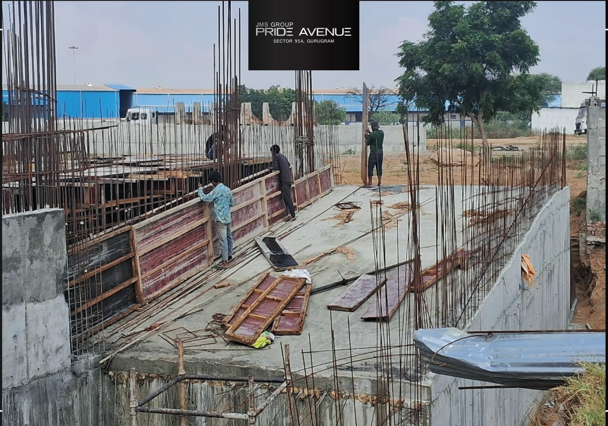
Ramp casted from ground floor to basement
