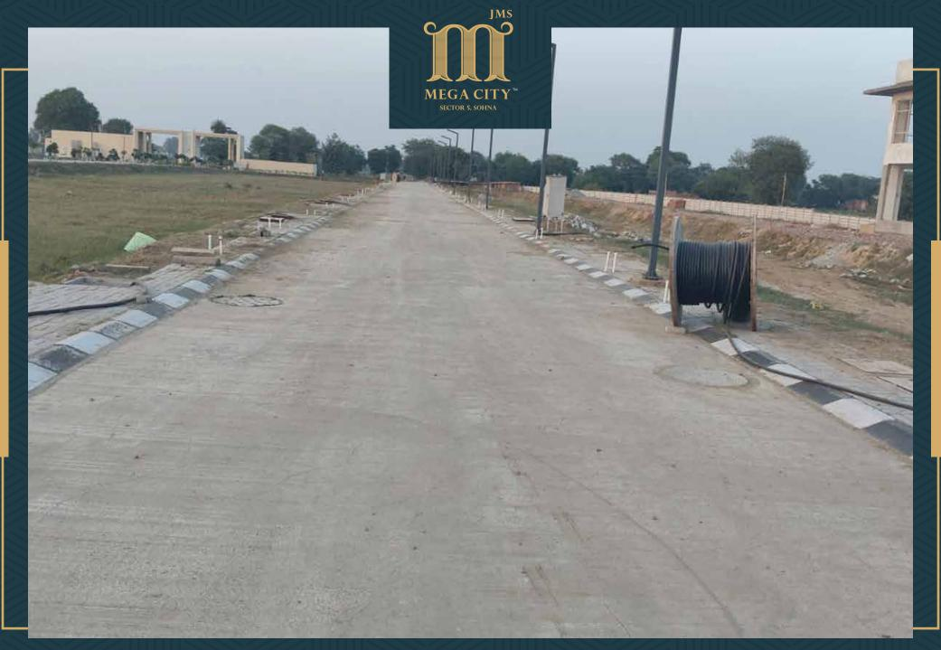
Road no. 5 civil development work, sewer, rainwater harvesting lines, water supply lines, road footpath pavers completed, electrical cable line and plantation work in progress
