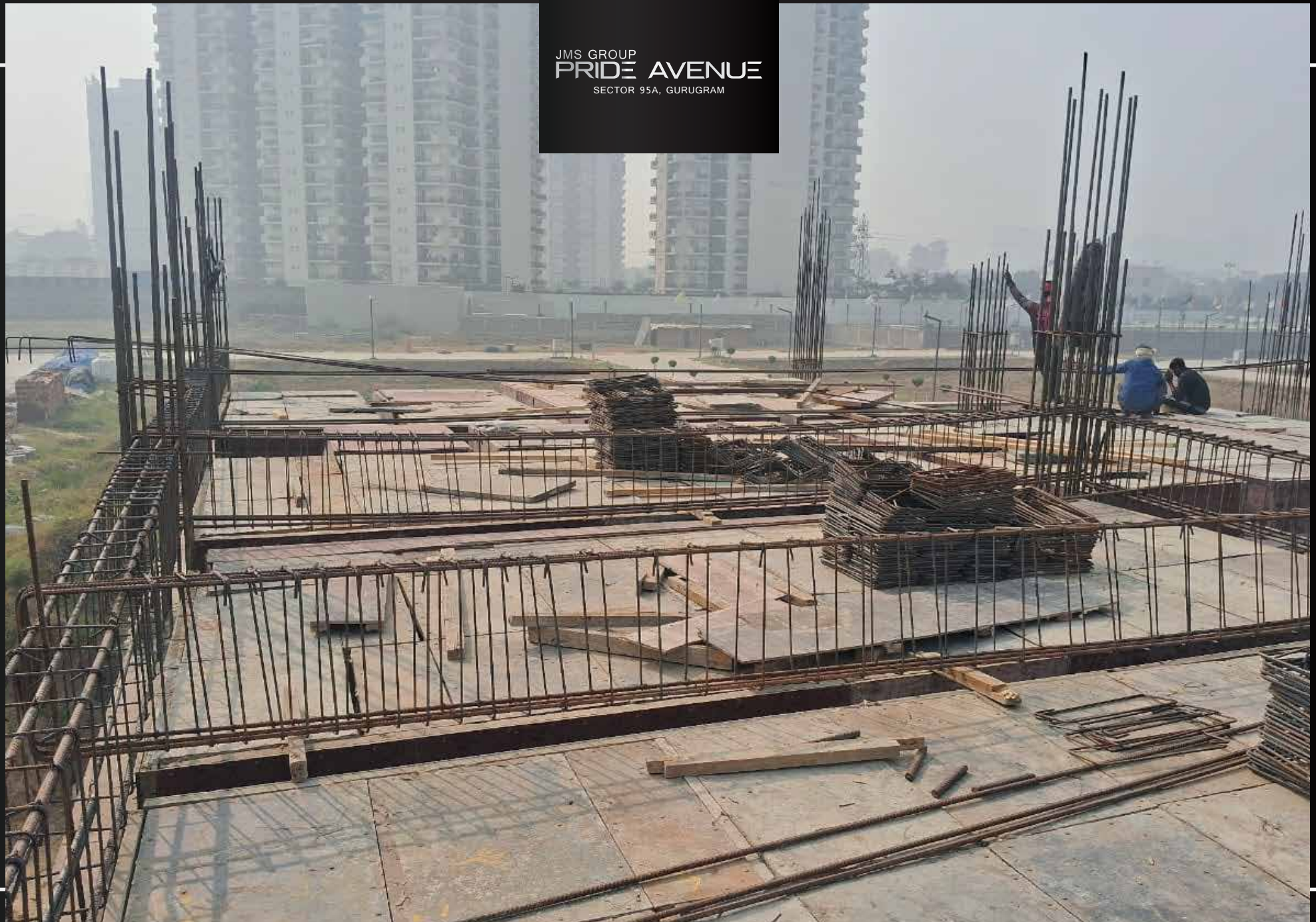
First floor slab beam reinforcement work in progress
