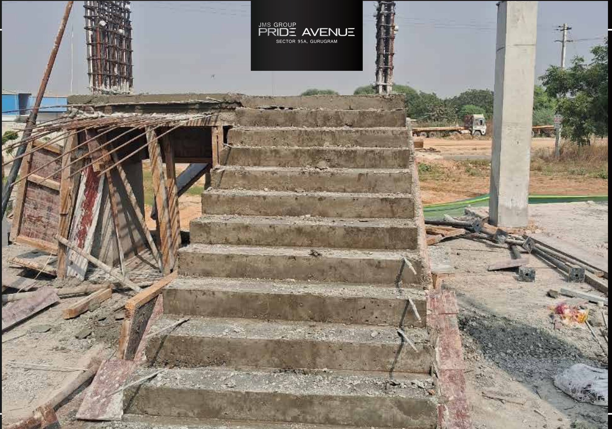
Staircase and column deshuttering work in progress
