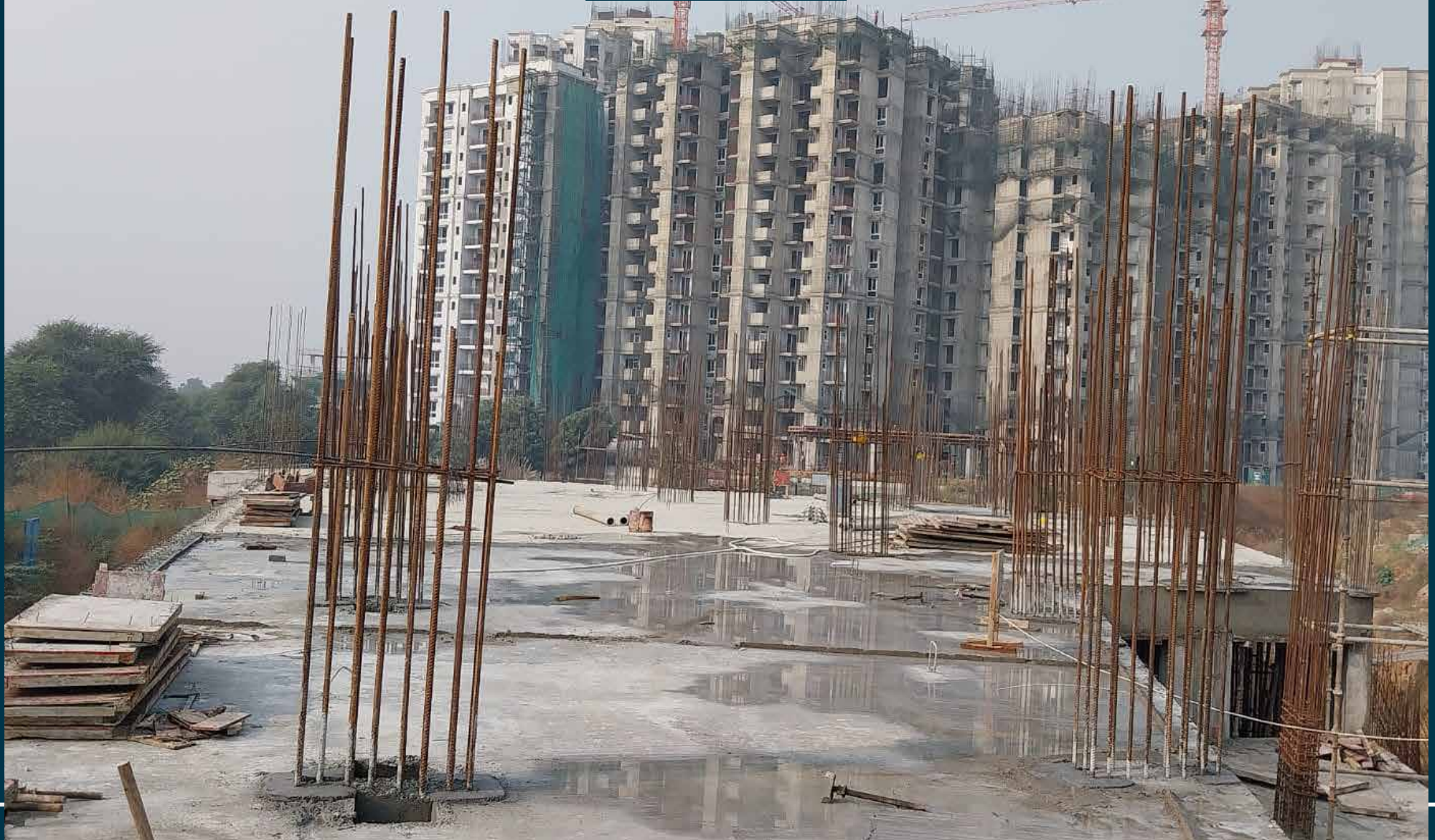
Underground floor slab casted
