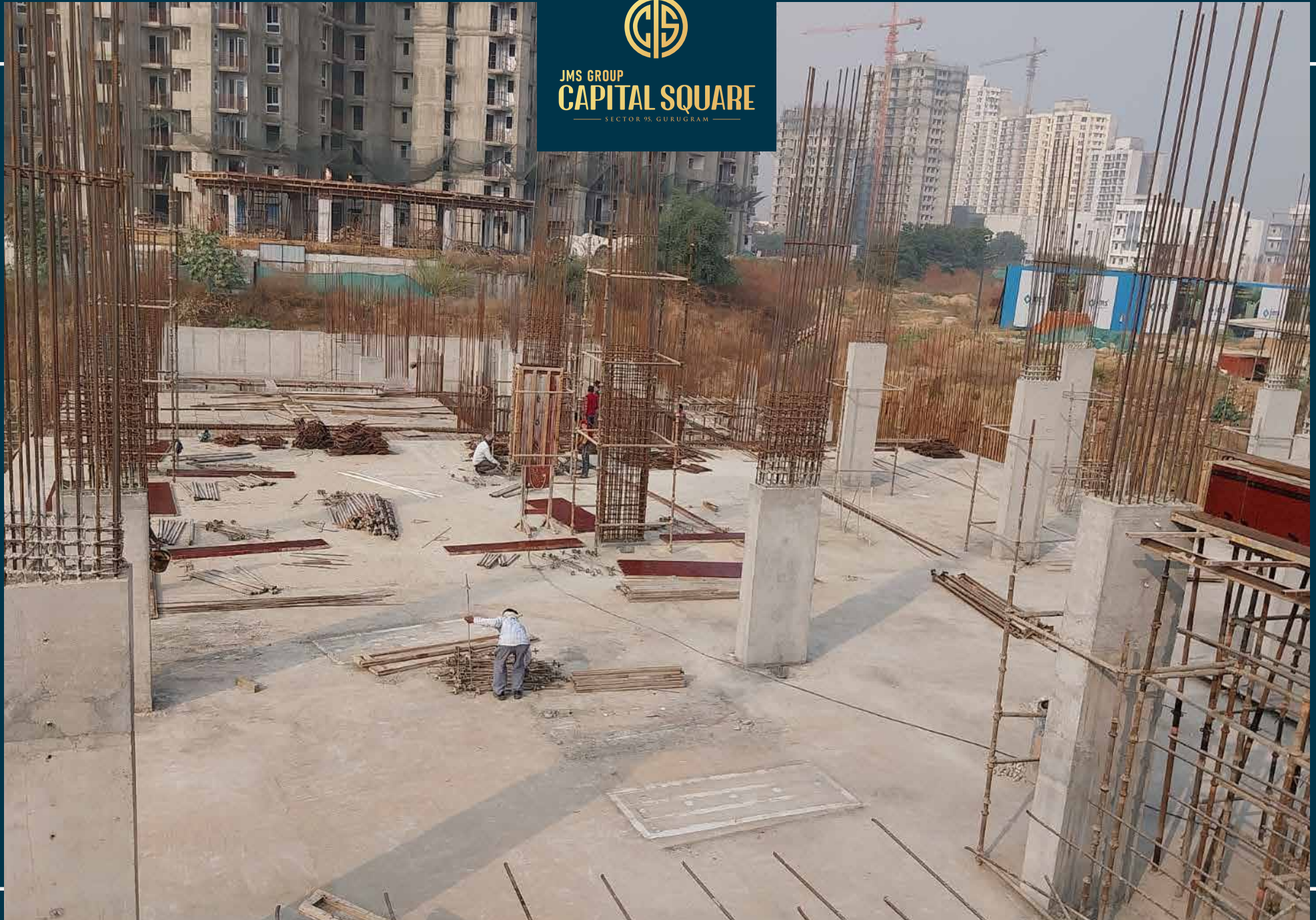
Underground floor slab casted
