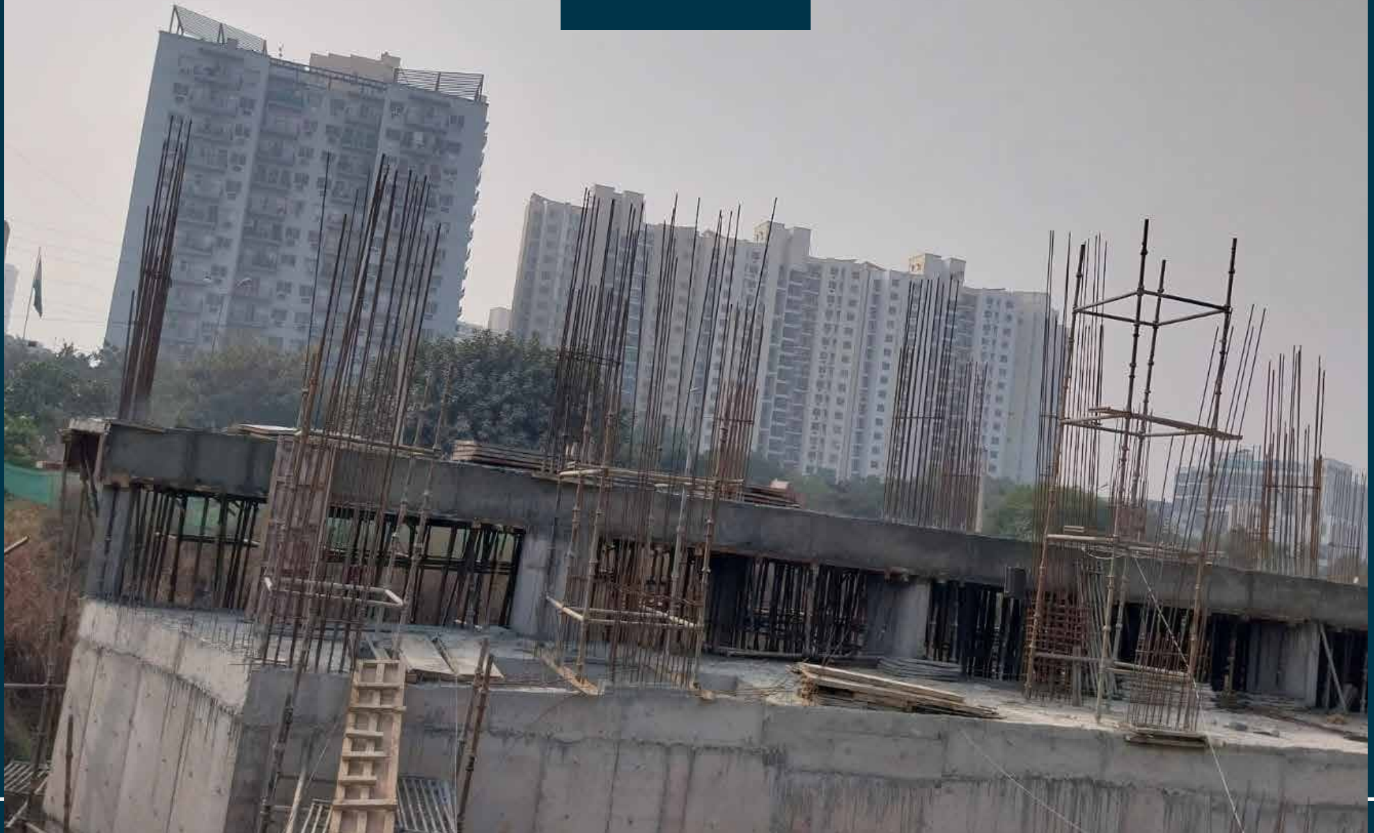
Underground floor slab casted
