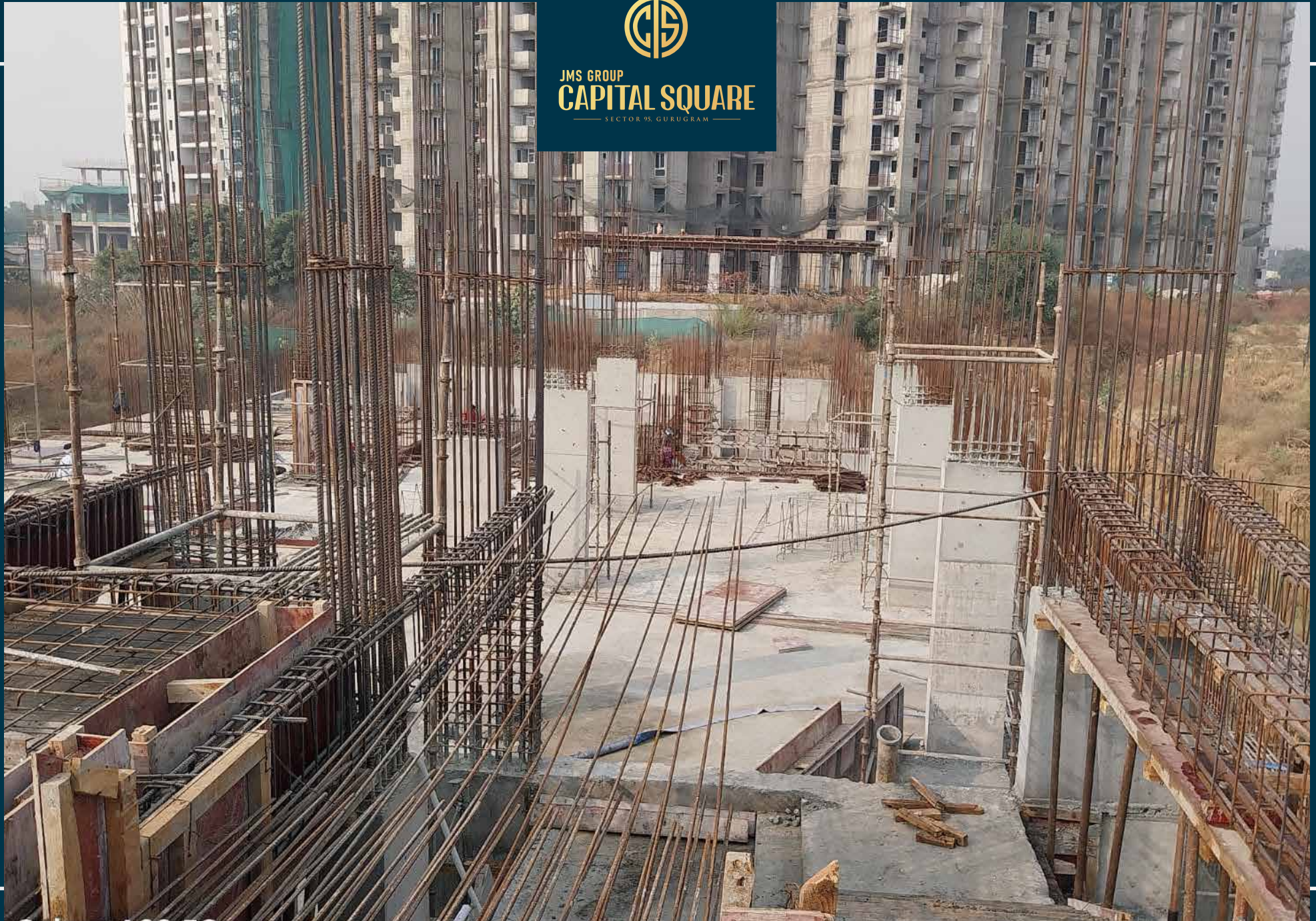
Underground floor slab casted
