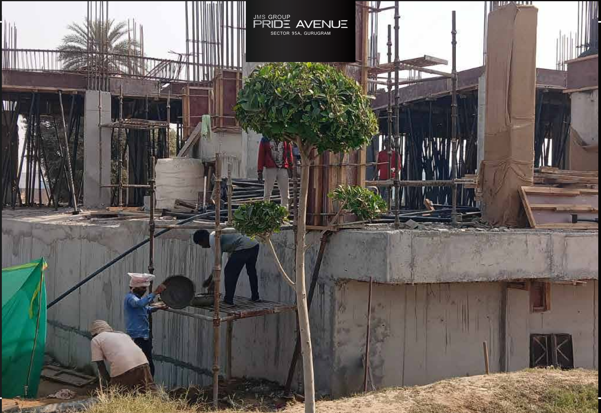
Ground floor slab casted
