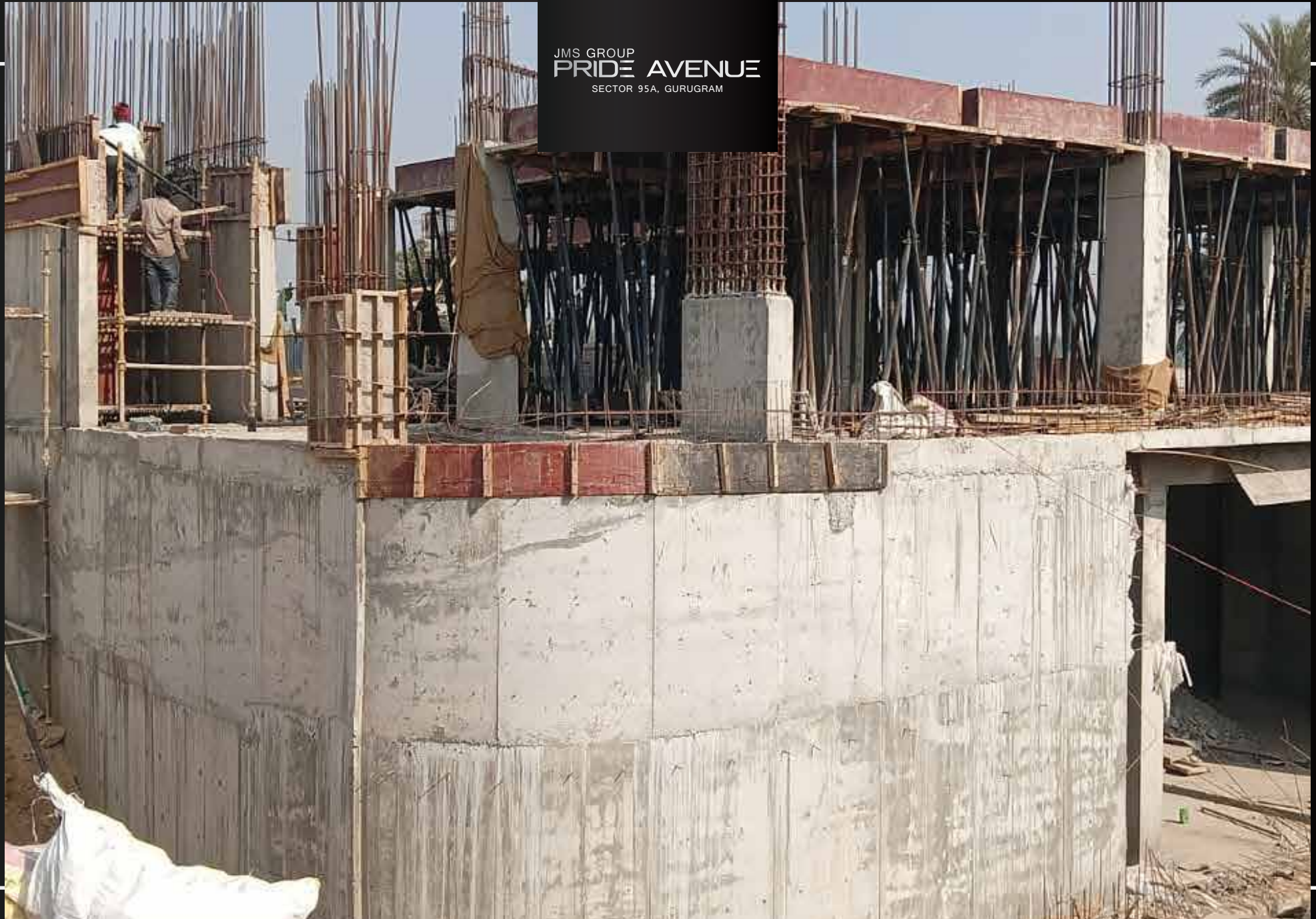
Ground floor slab casted
