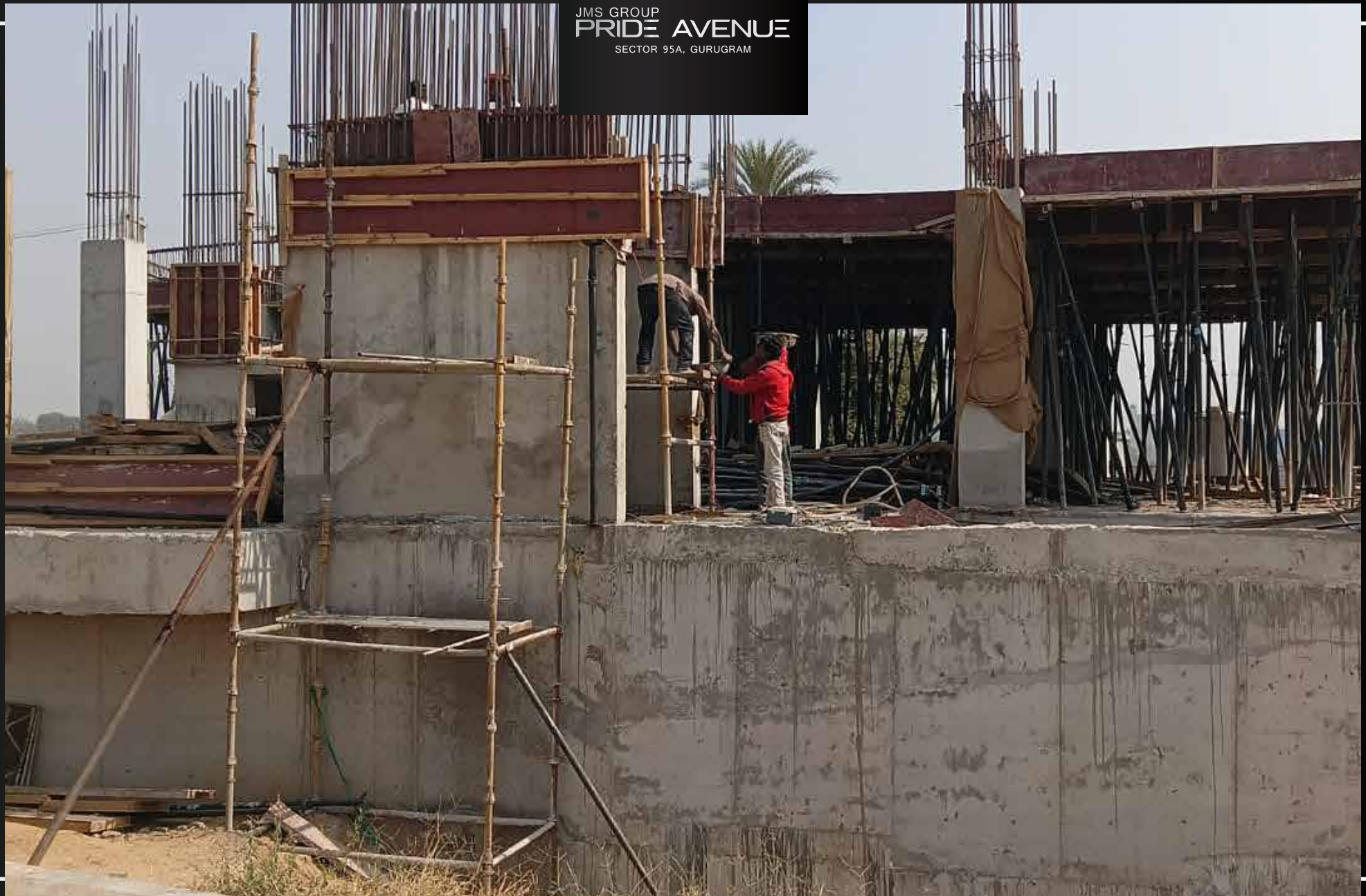
Ground floor slab casted
