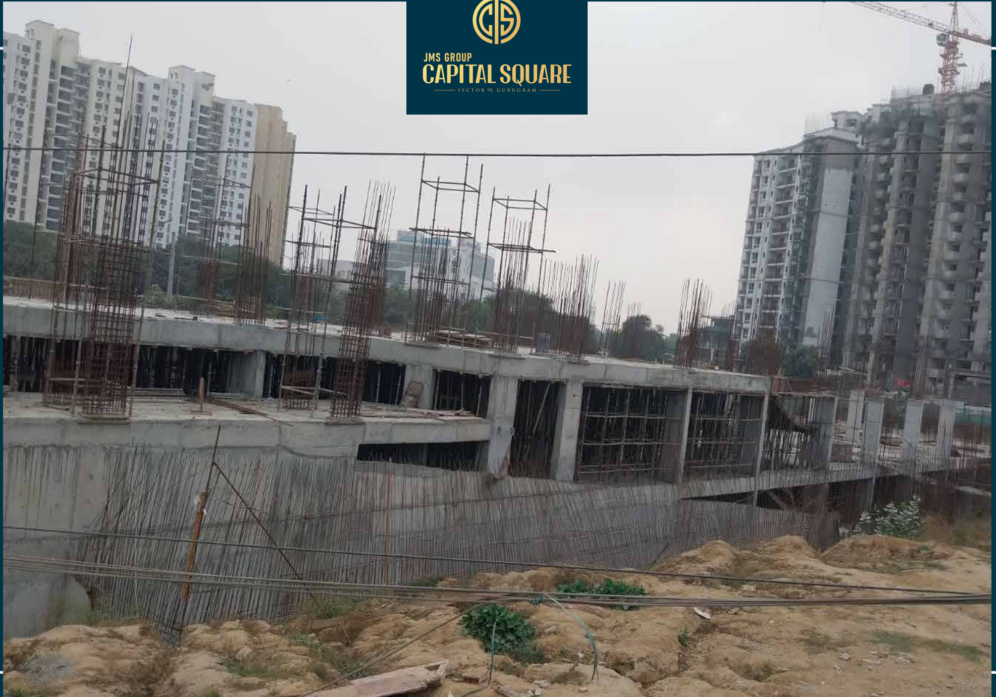
Underground floor slab casting work in progress
