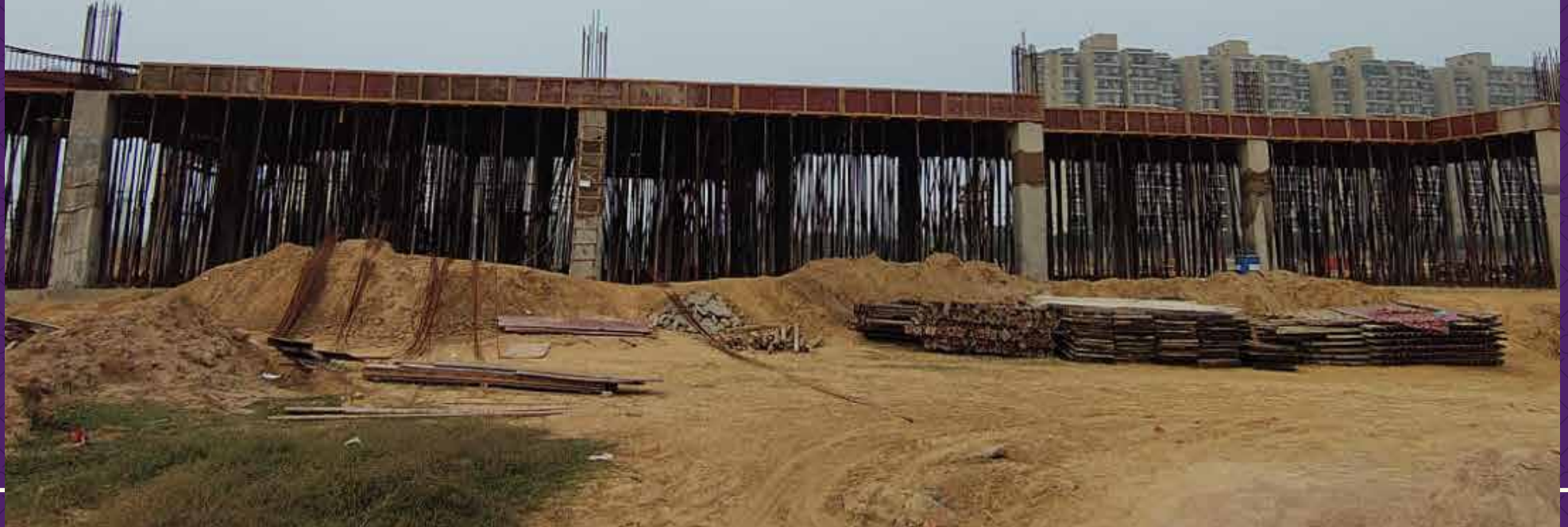
Slab shuttering work in progress
