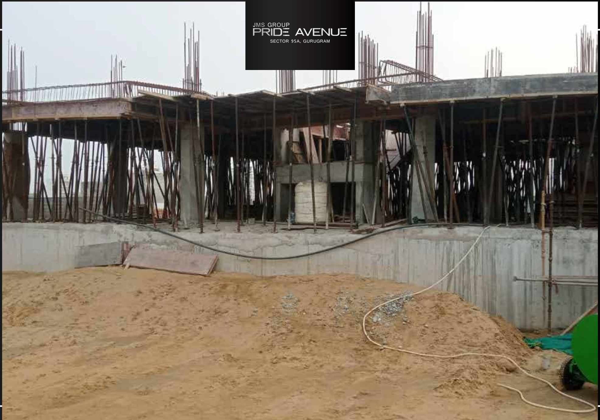
First floor level slab work in progress
