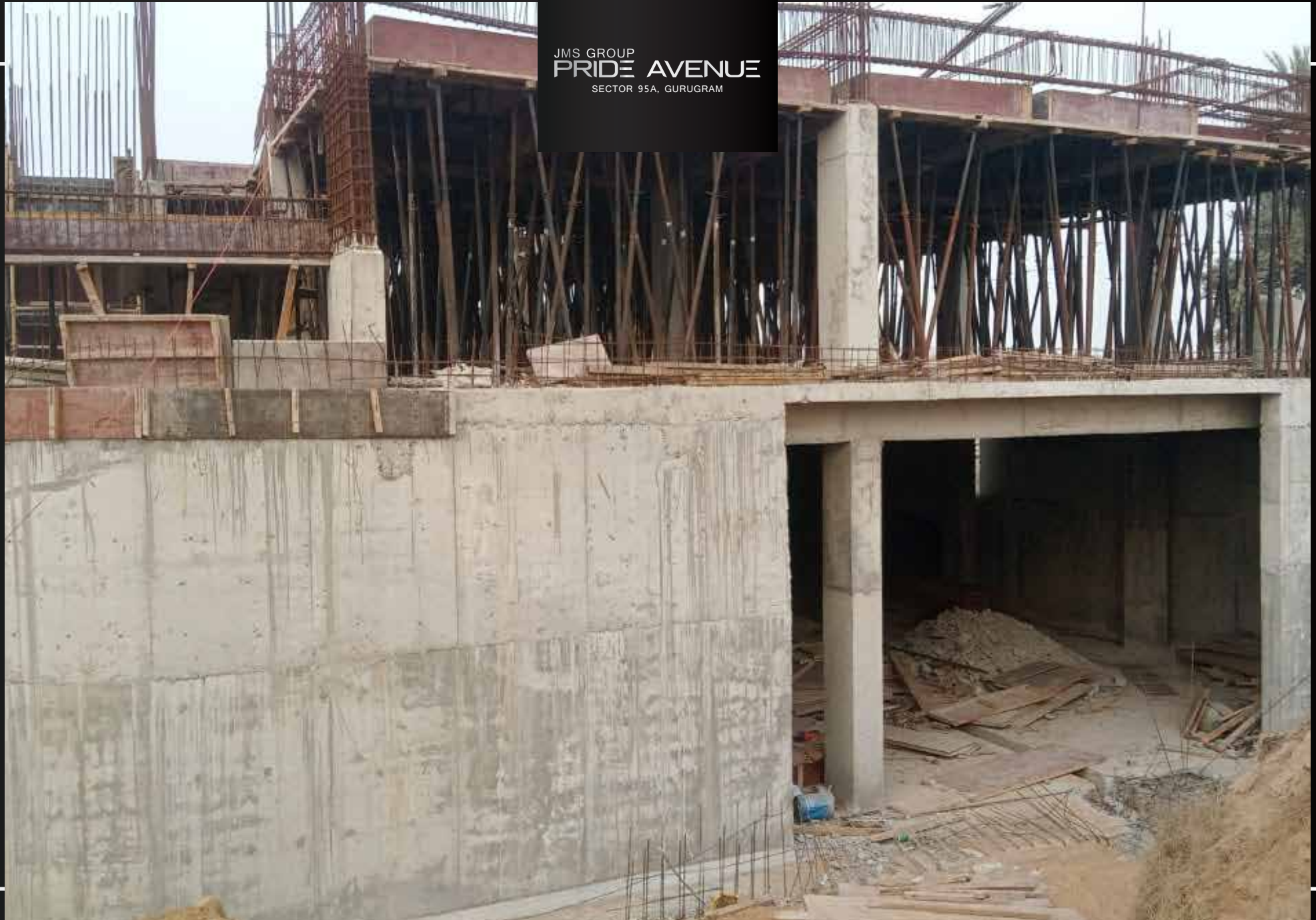
First floor level slab work in progress
