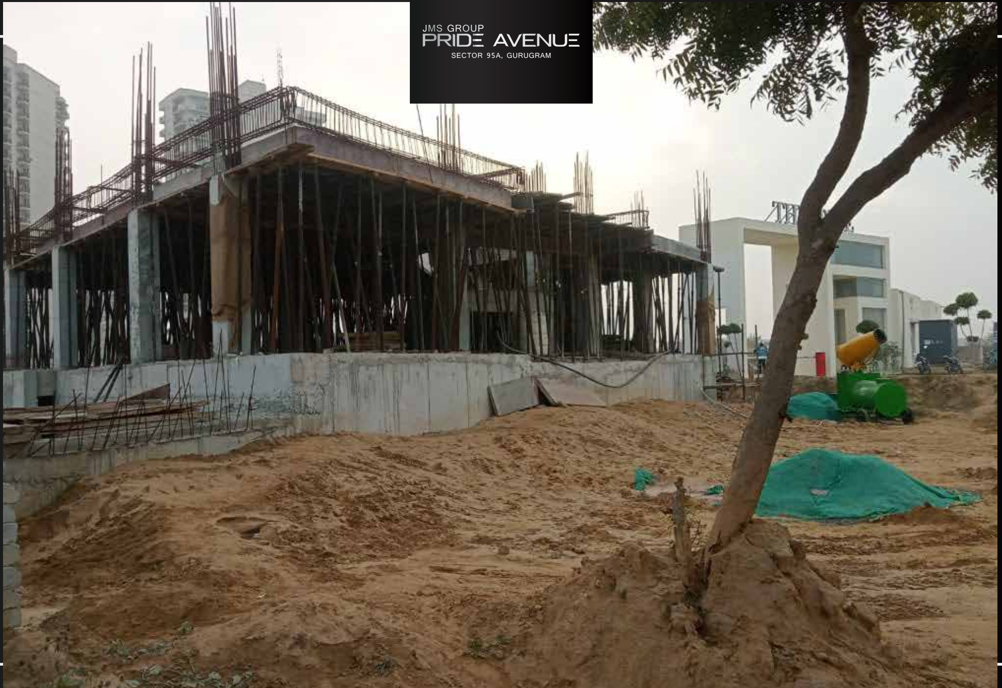
First floor level slab work in progress
