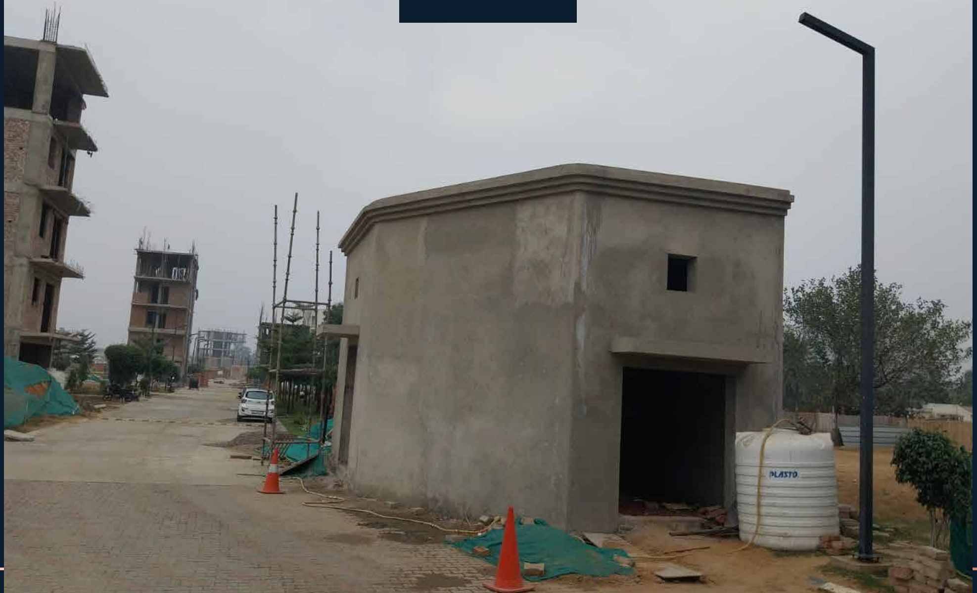
Electrical room work in progress
