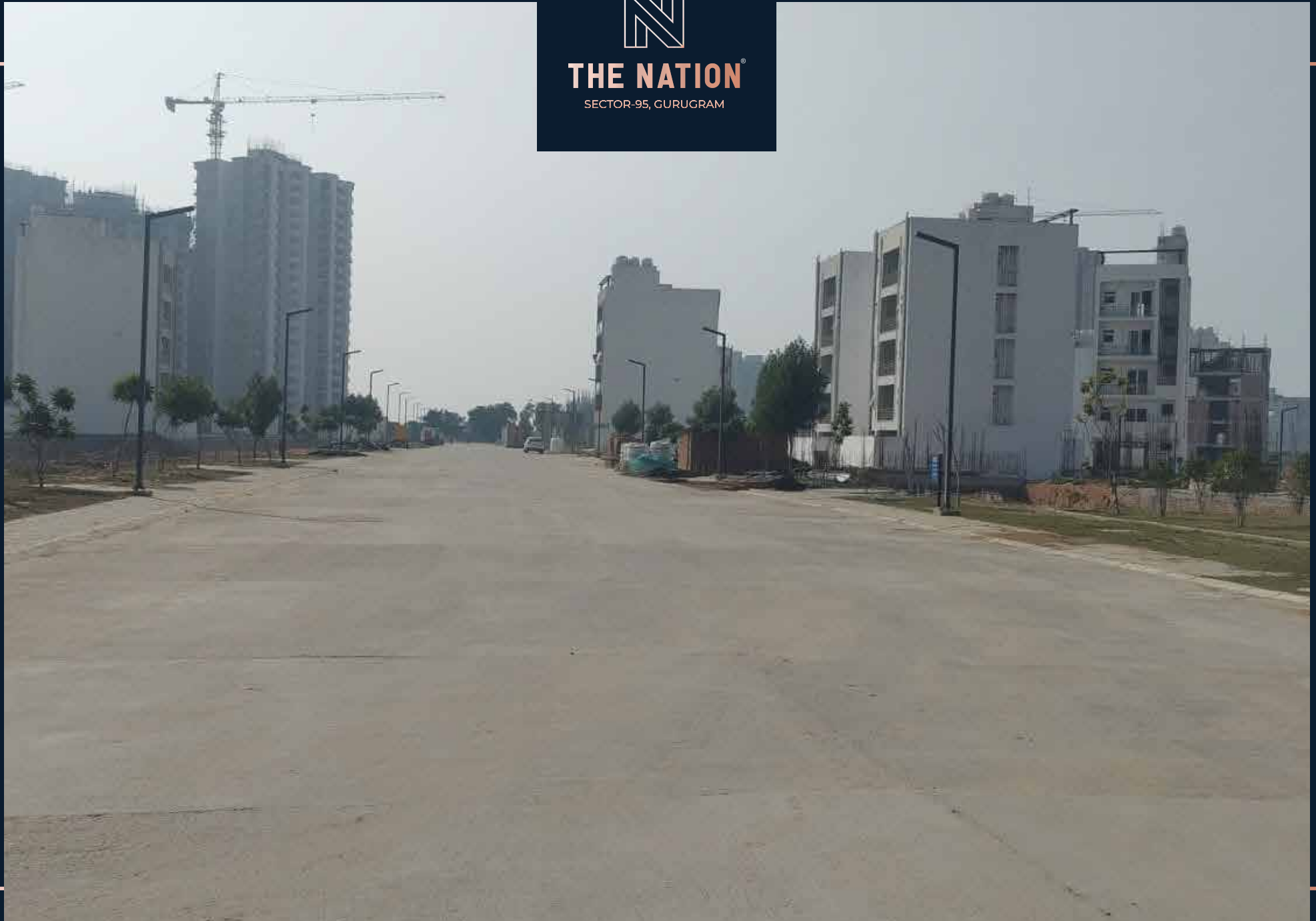
Construction of 24 meter road completed
