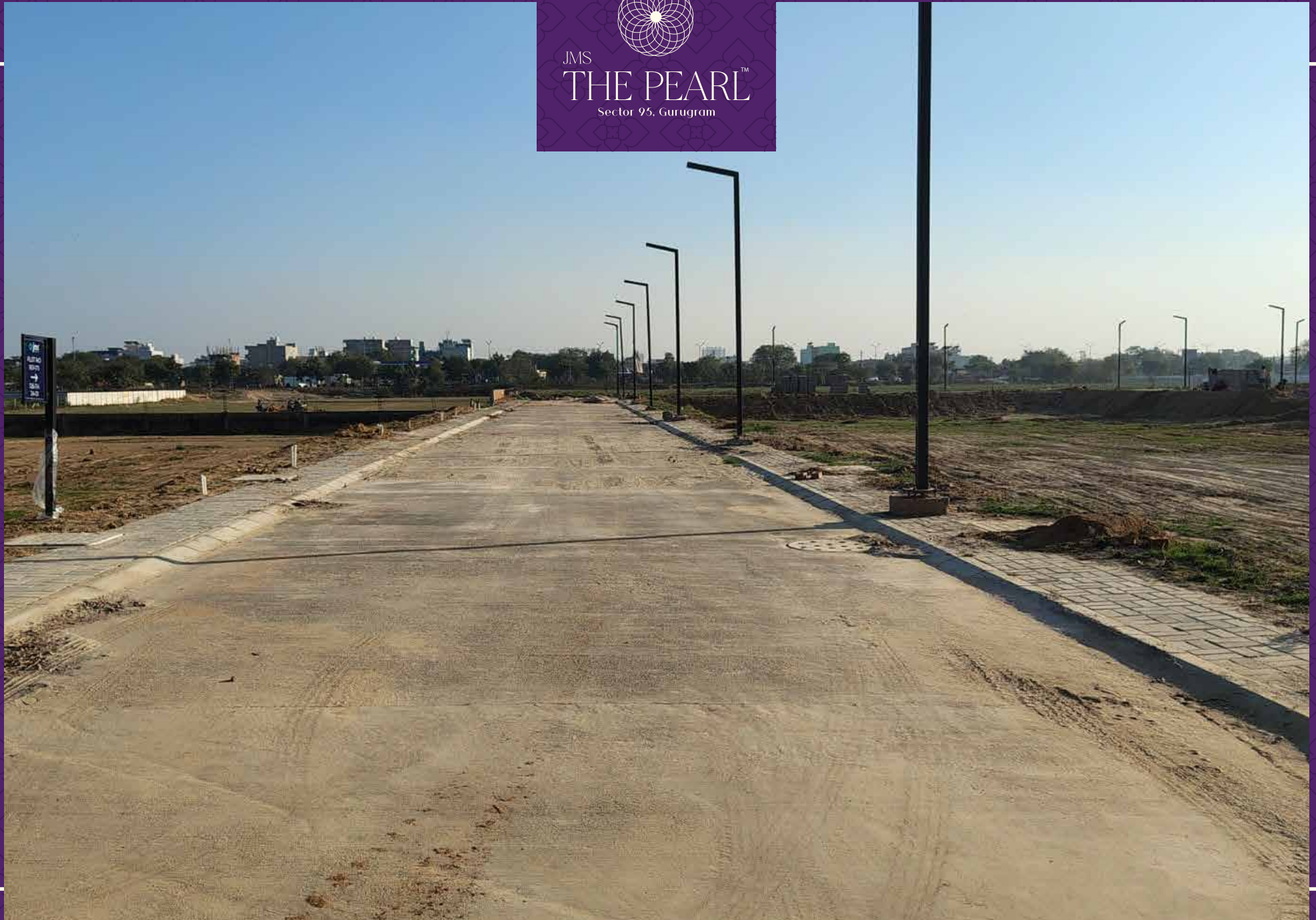
24 meter road construction in progress
