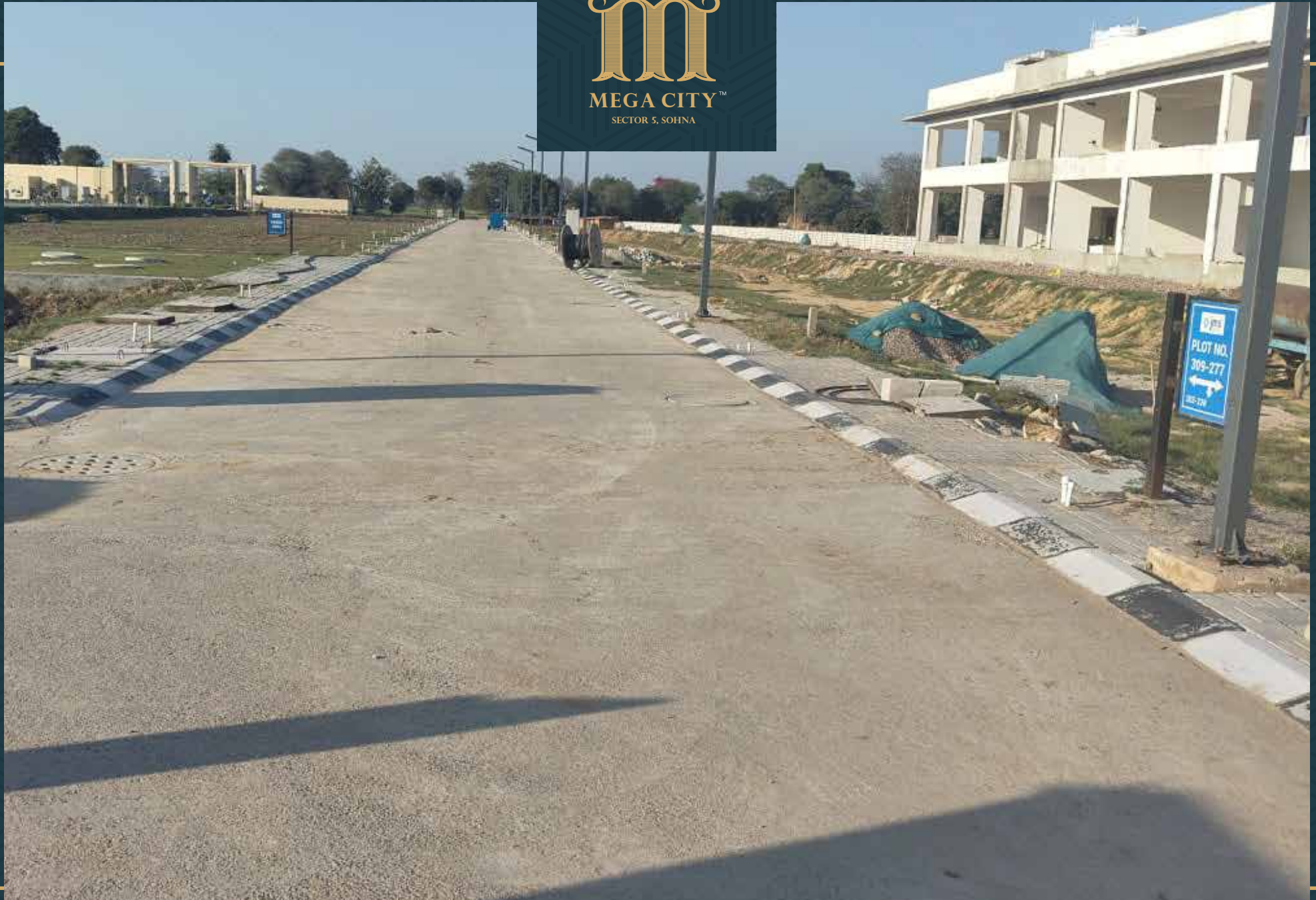
Road no. 5 work completed and electrical cable line work in progress
