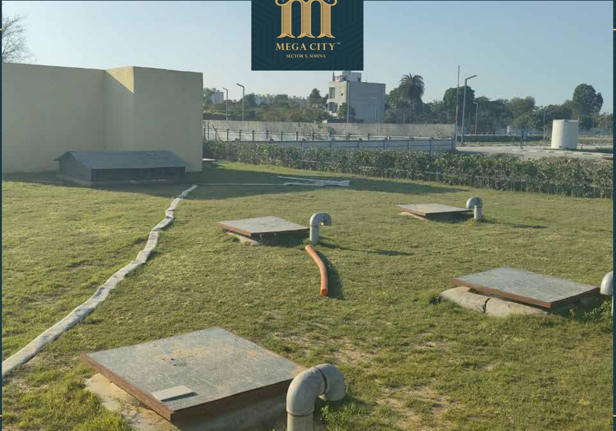
UGT construction completed
