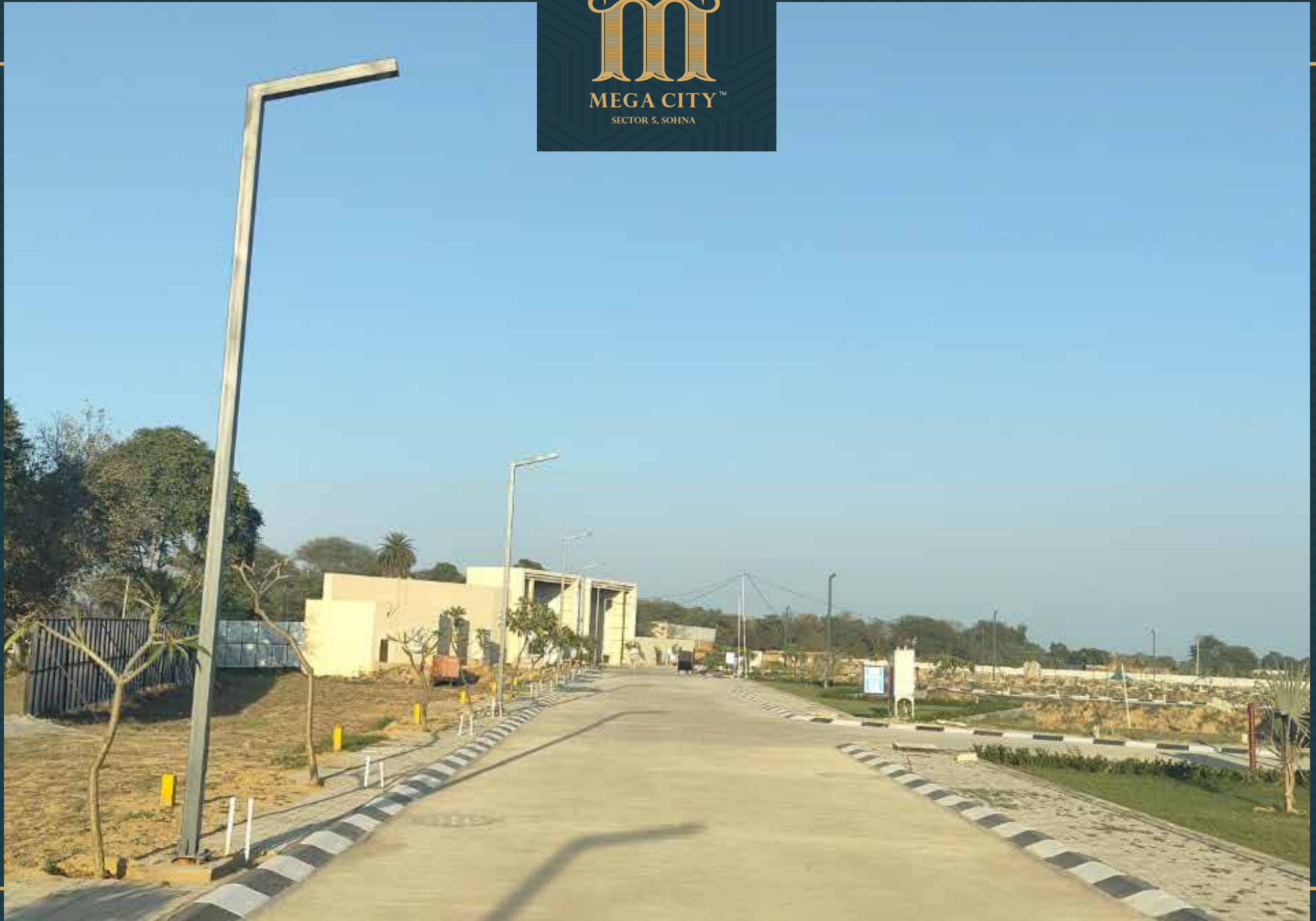
Road no. 6 work completed and electrical cable line work in progress
