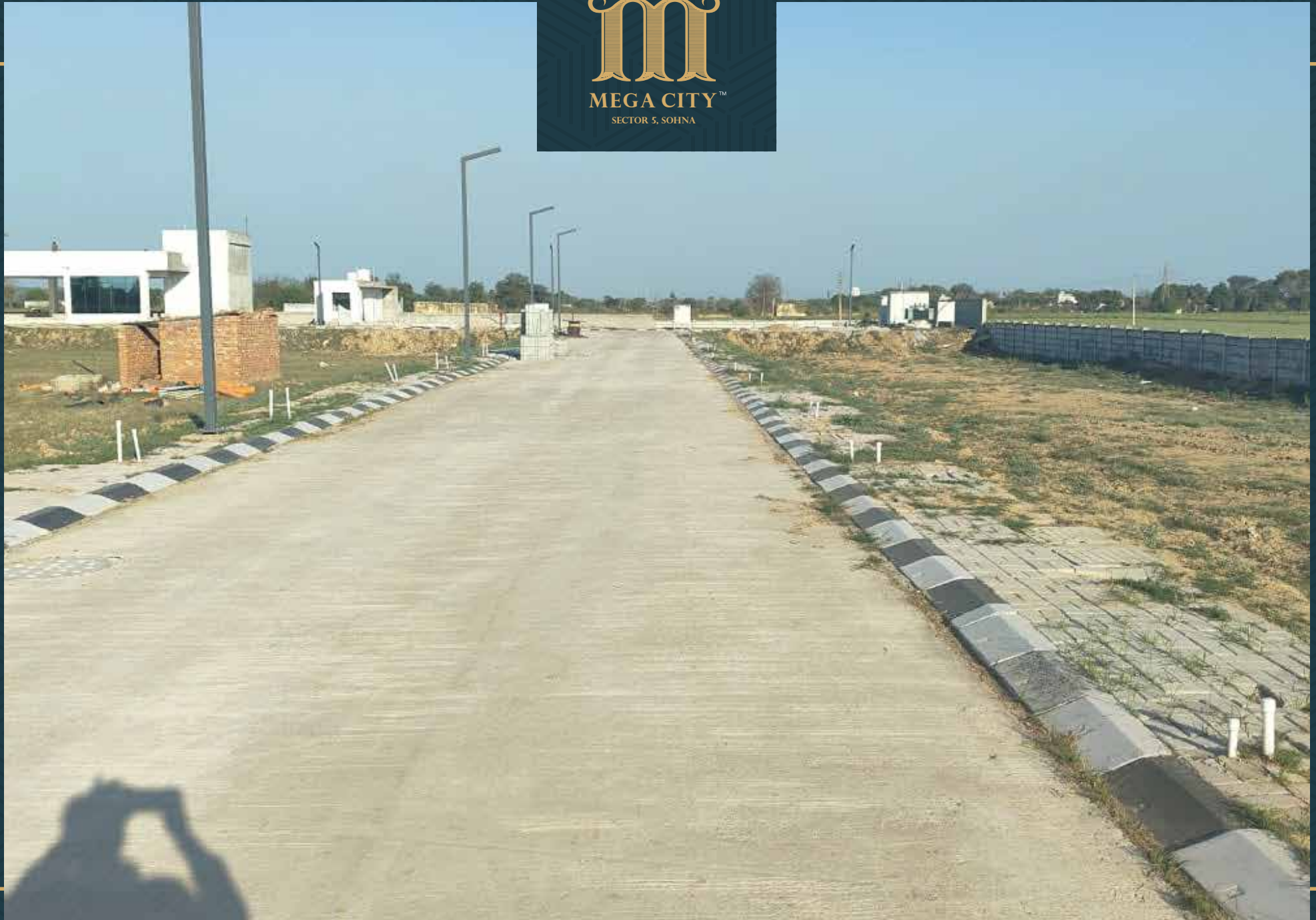
Road no. 8 work completed and electrical cable line work in progress
