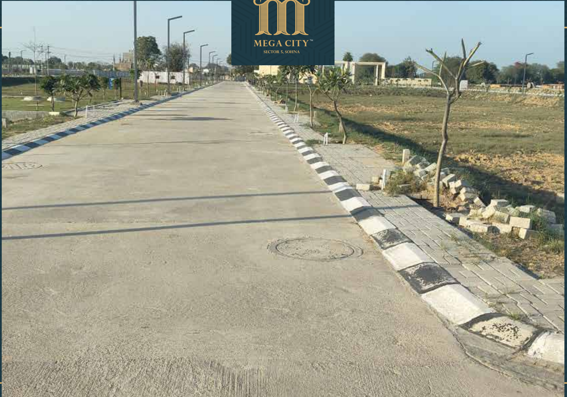
Road no. 3 work completed and electrical cable line work in progress
