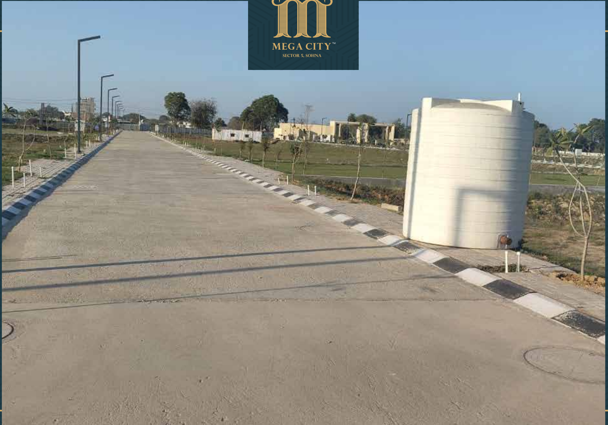
Road no. 2 work completed and electrical cable line work in progress
