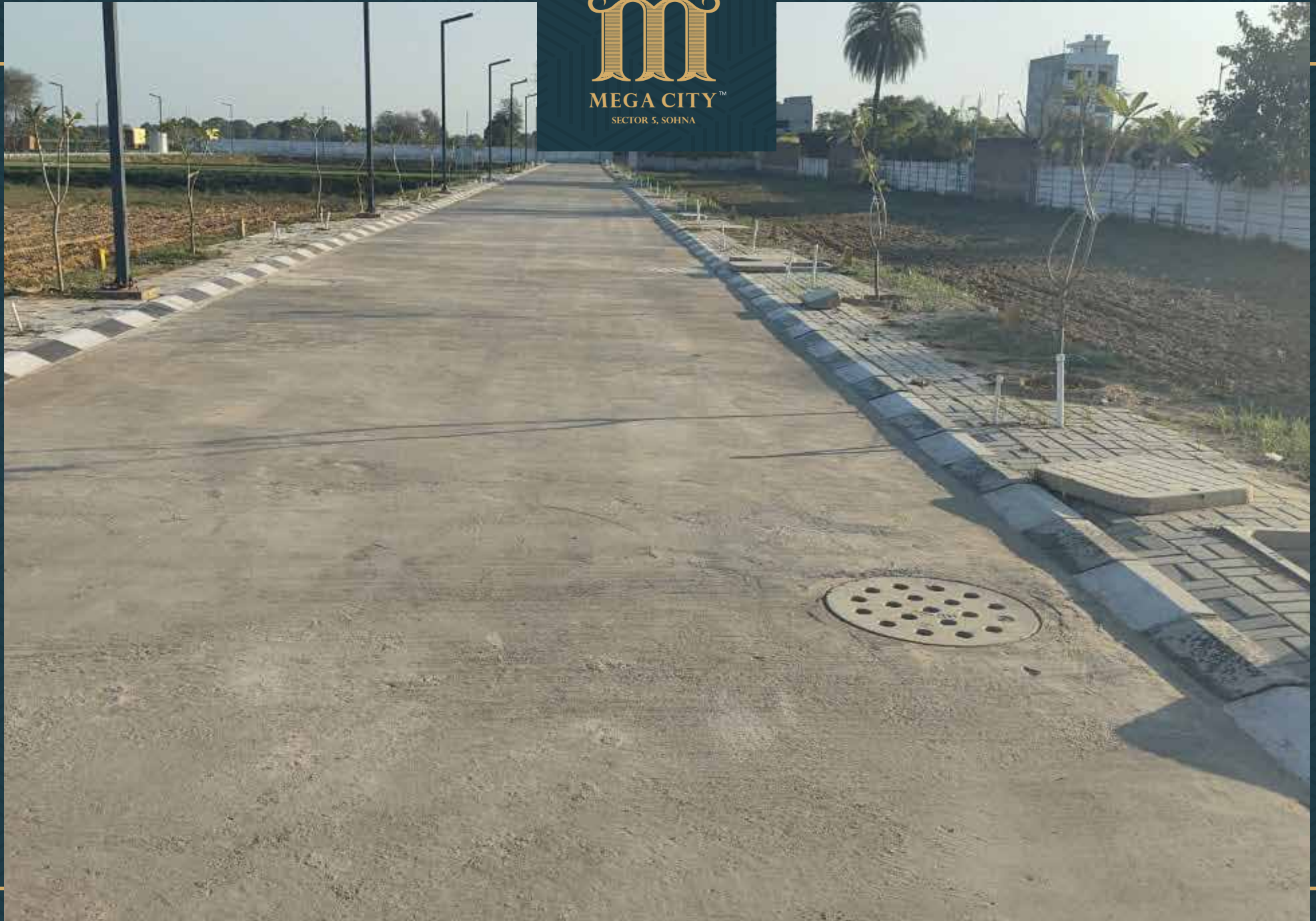
Road no. 1 work completed and electrical cable line work in progress
