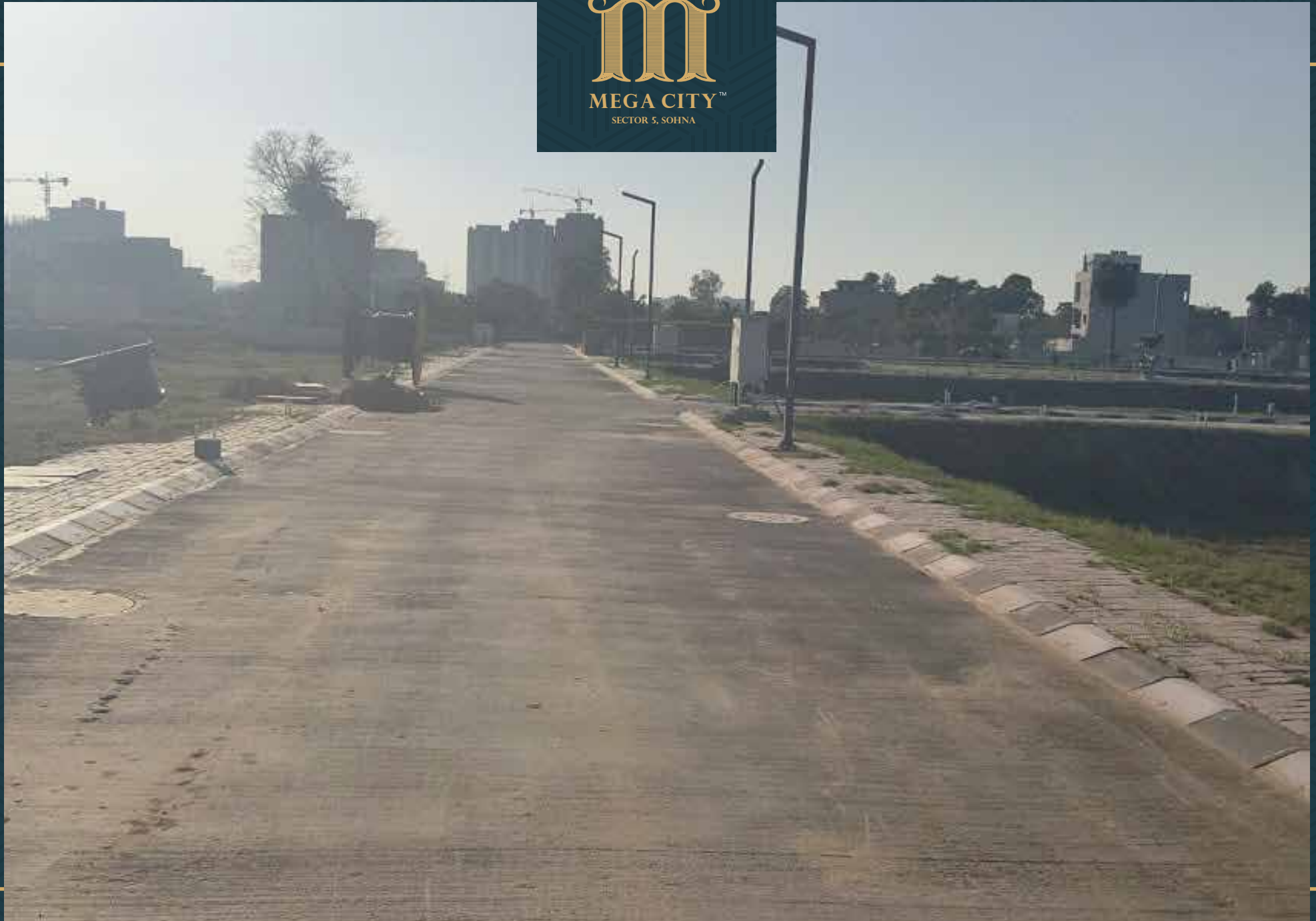
Road no. 7 work completed and electrical cable line work in progress
