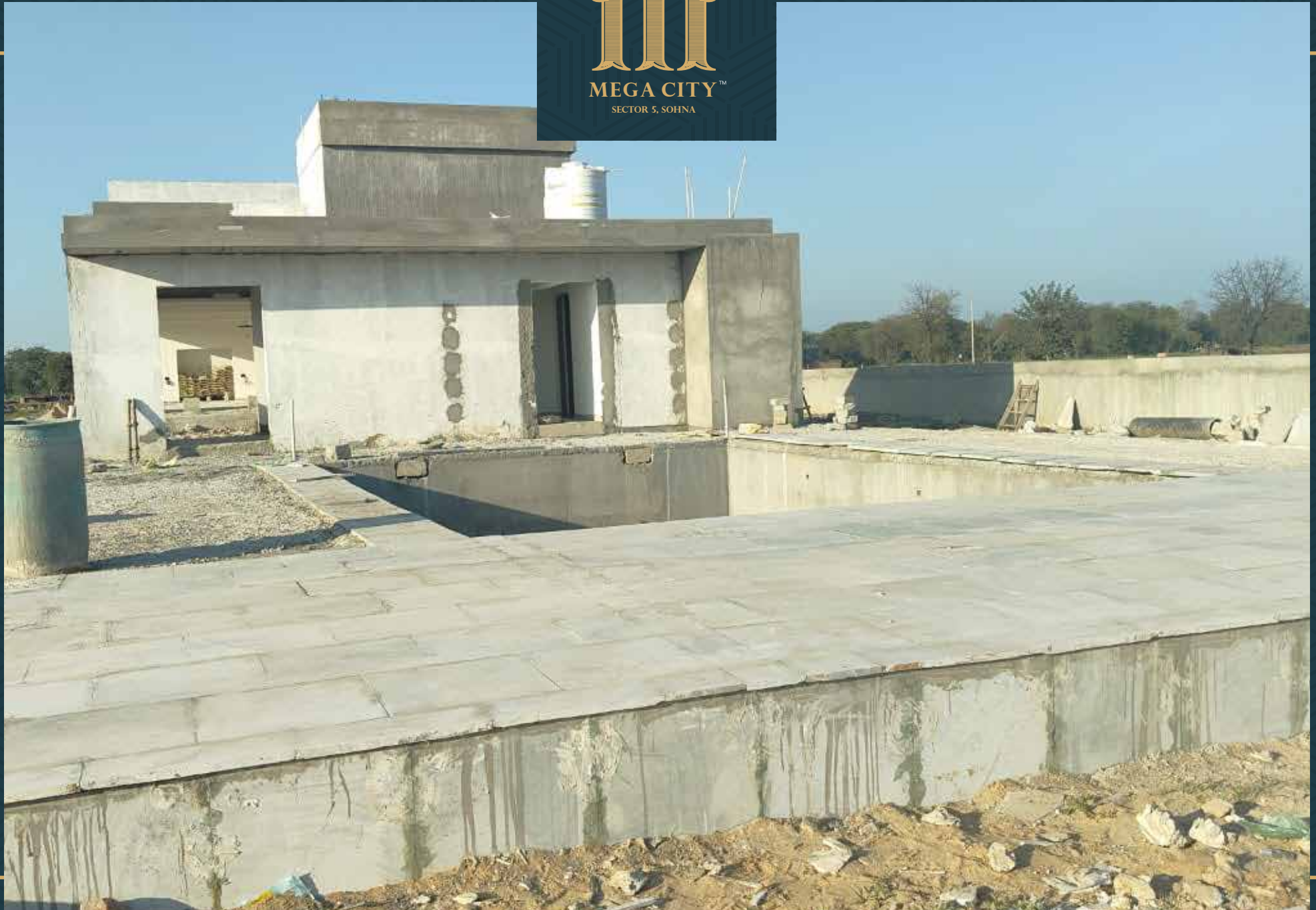
Swimming pool structure completed and finishing work in progress
