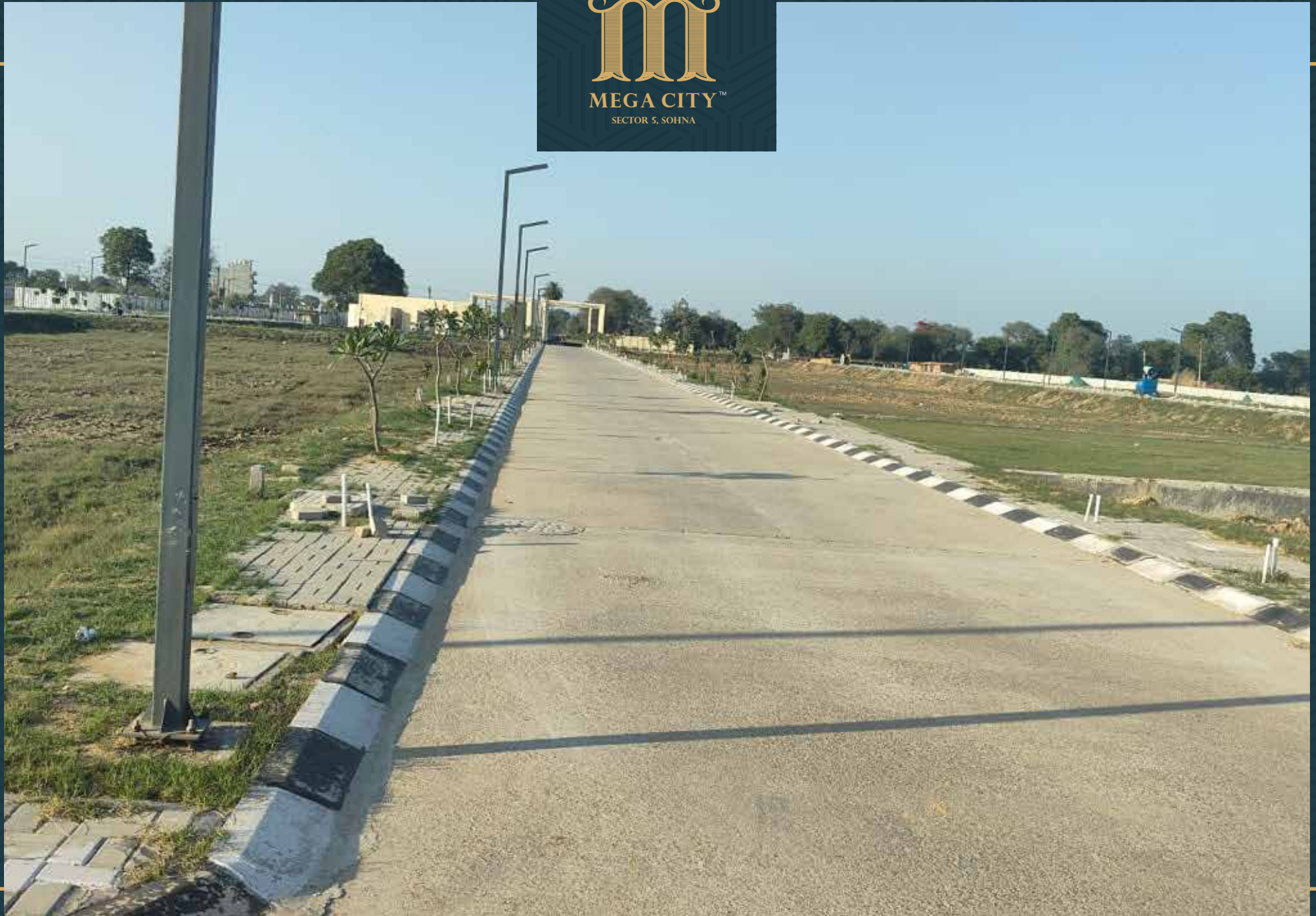
Road no. 4 work completed and electrical cable line work in progress
