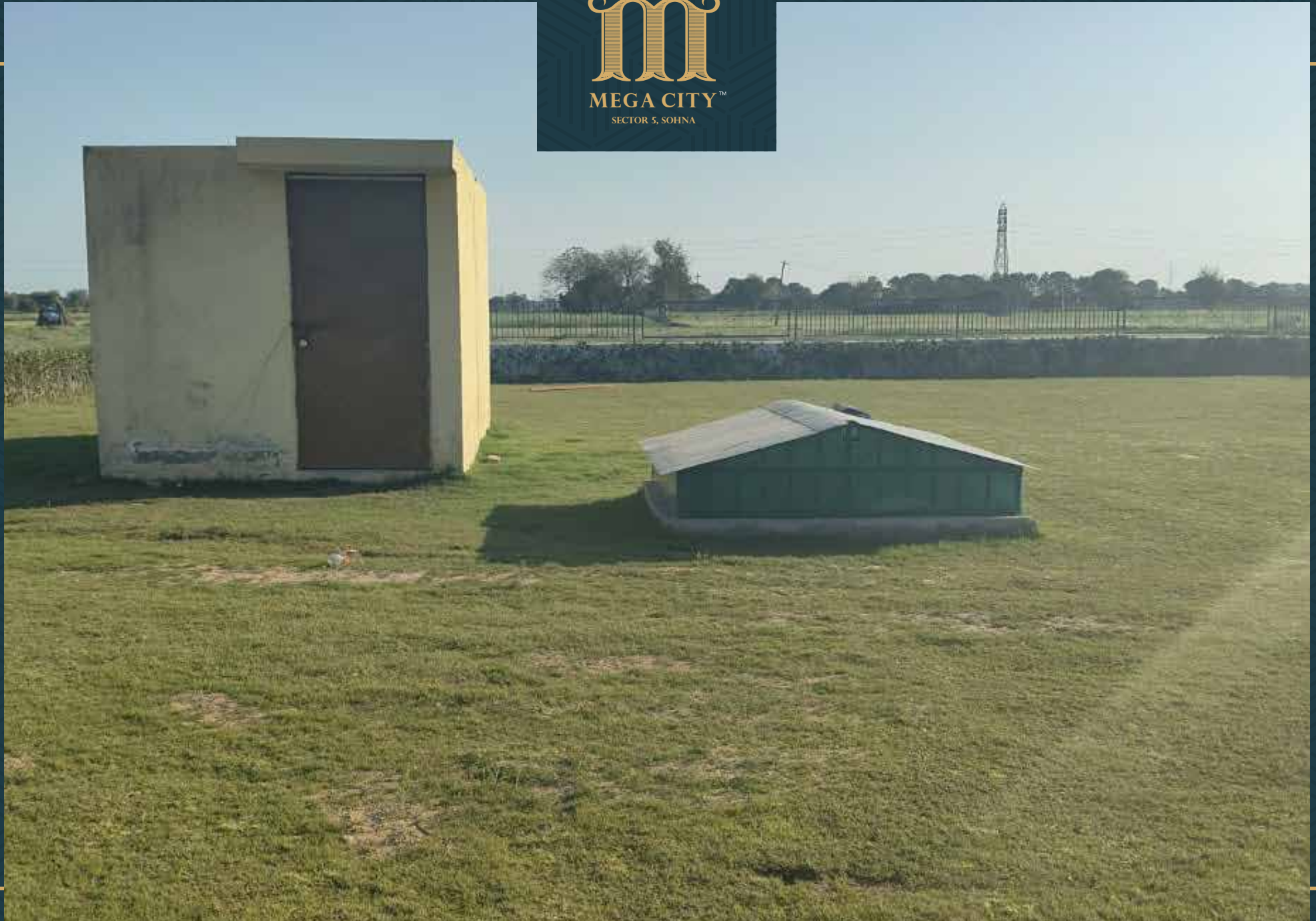
STP installation completed
