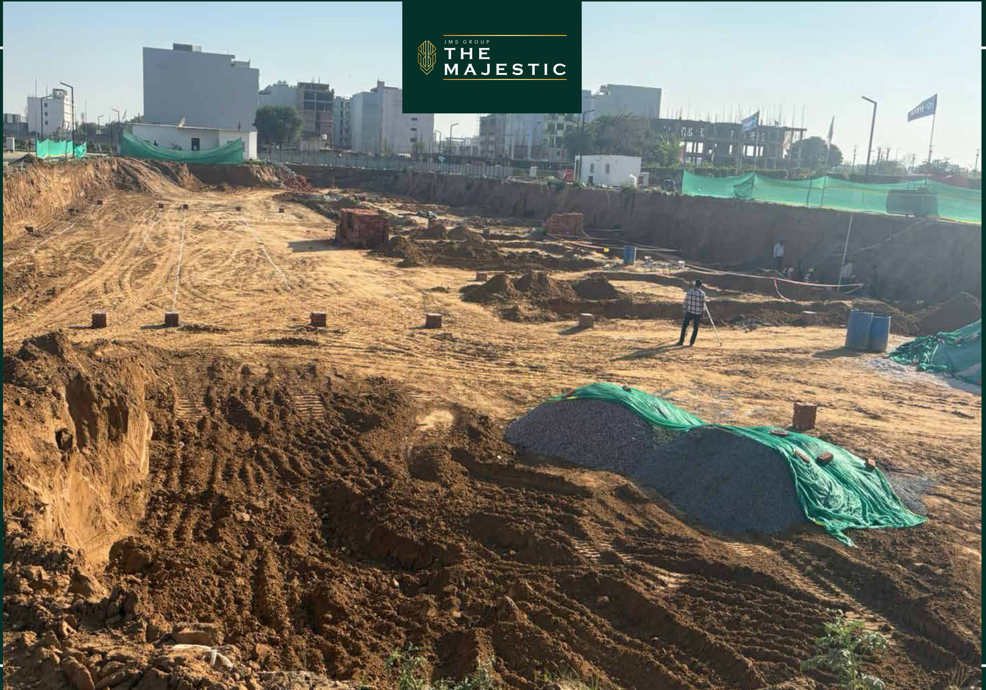
Plot no. 298 to 305 Foundation brick work in progress
