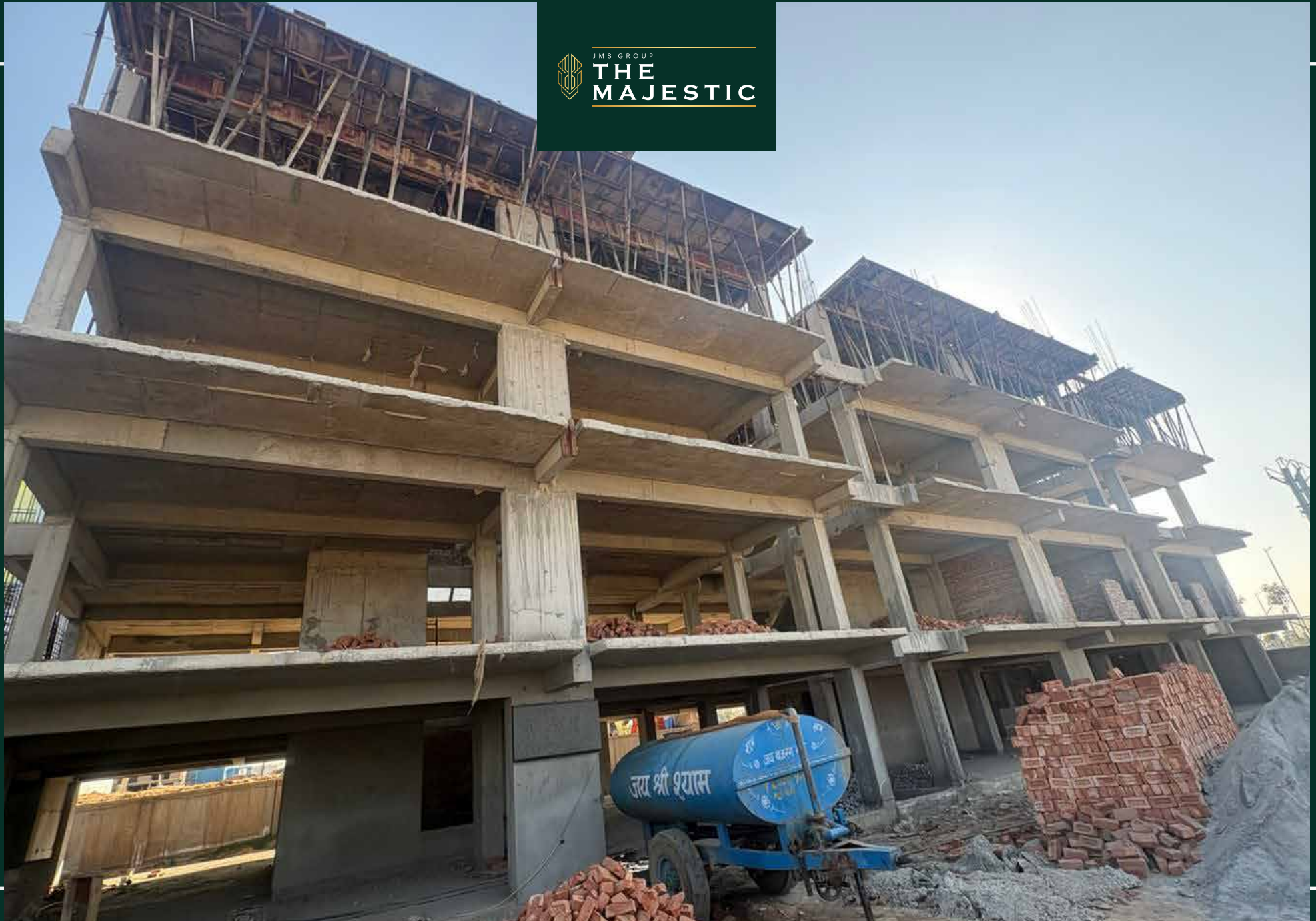
Plot no. 374 to 378 4th floor steel fixing work in progress
