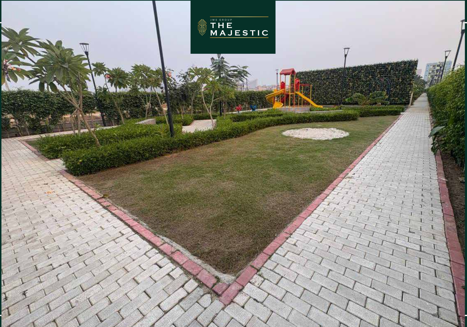
Park development work completed
