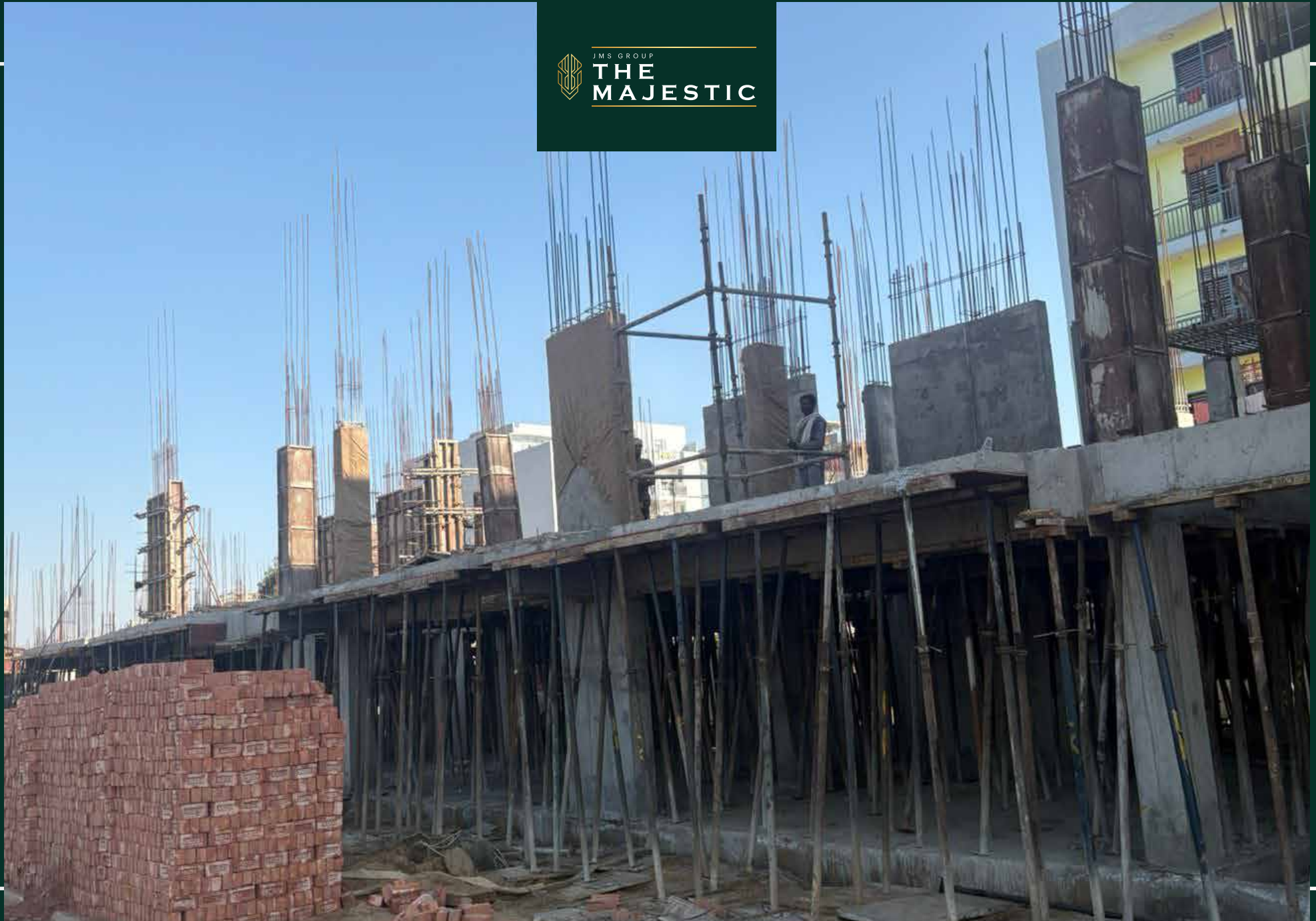
Plot no. 370 to 373 1st floor column casting work in progress
