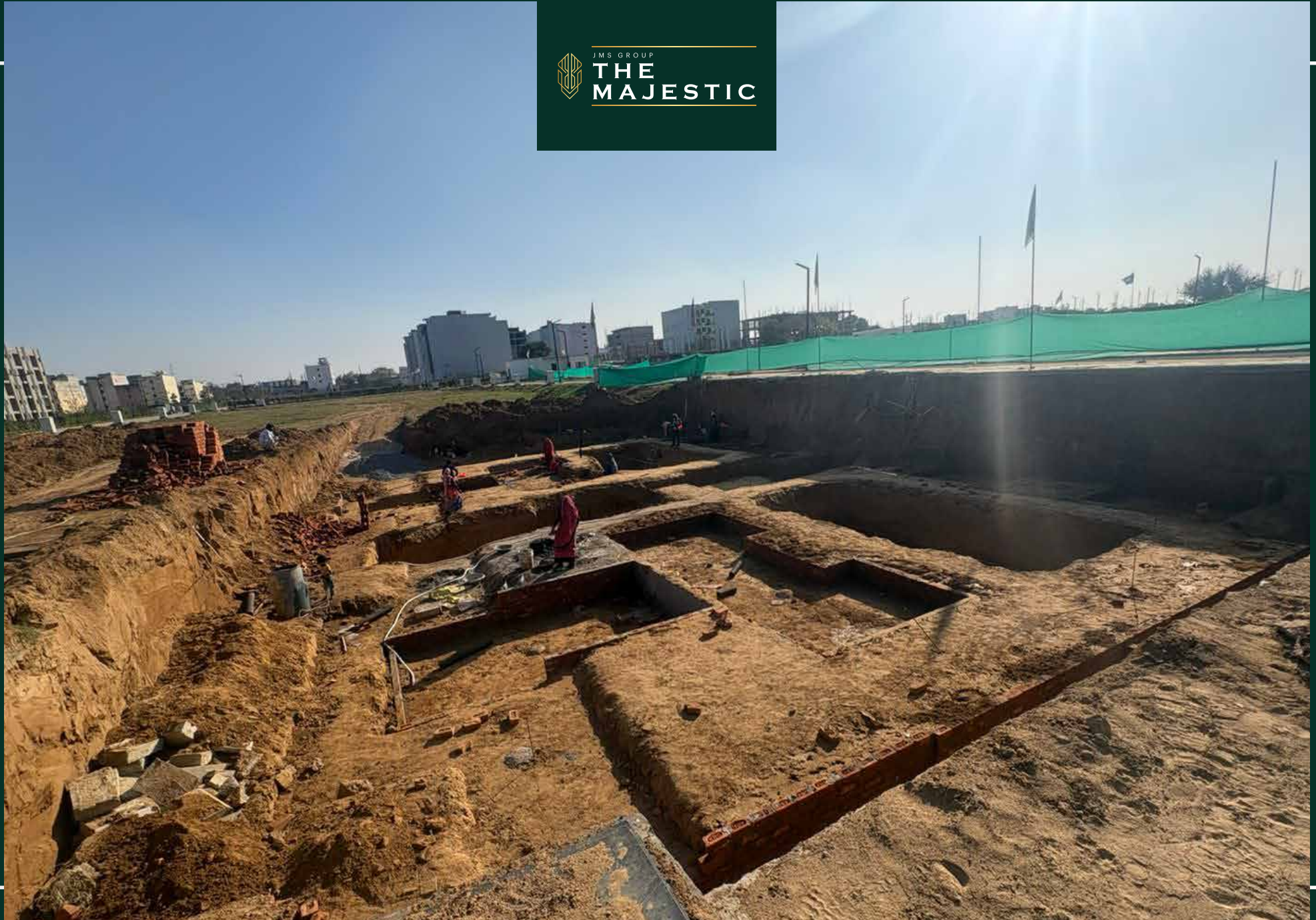
Plot no. 37 to 40 Foundation brick work in progress
