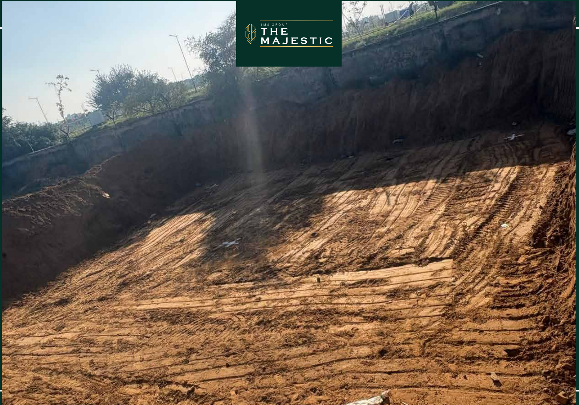
Plot no. 341 to 349 & Plot no. 350 to 360 Excavation work in progress
