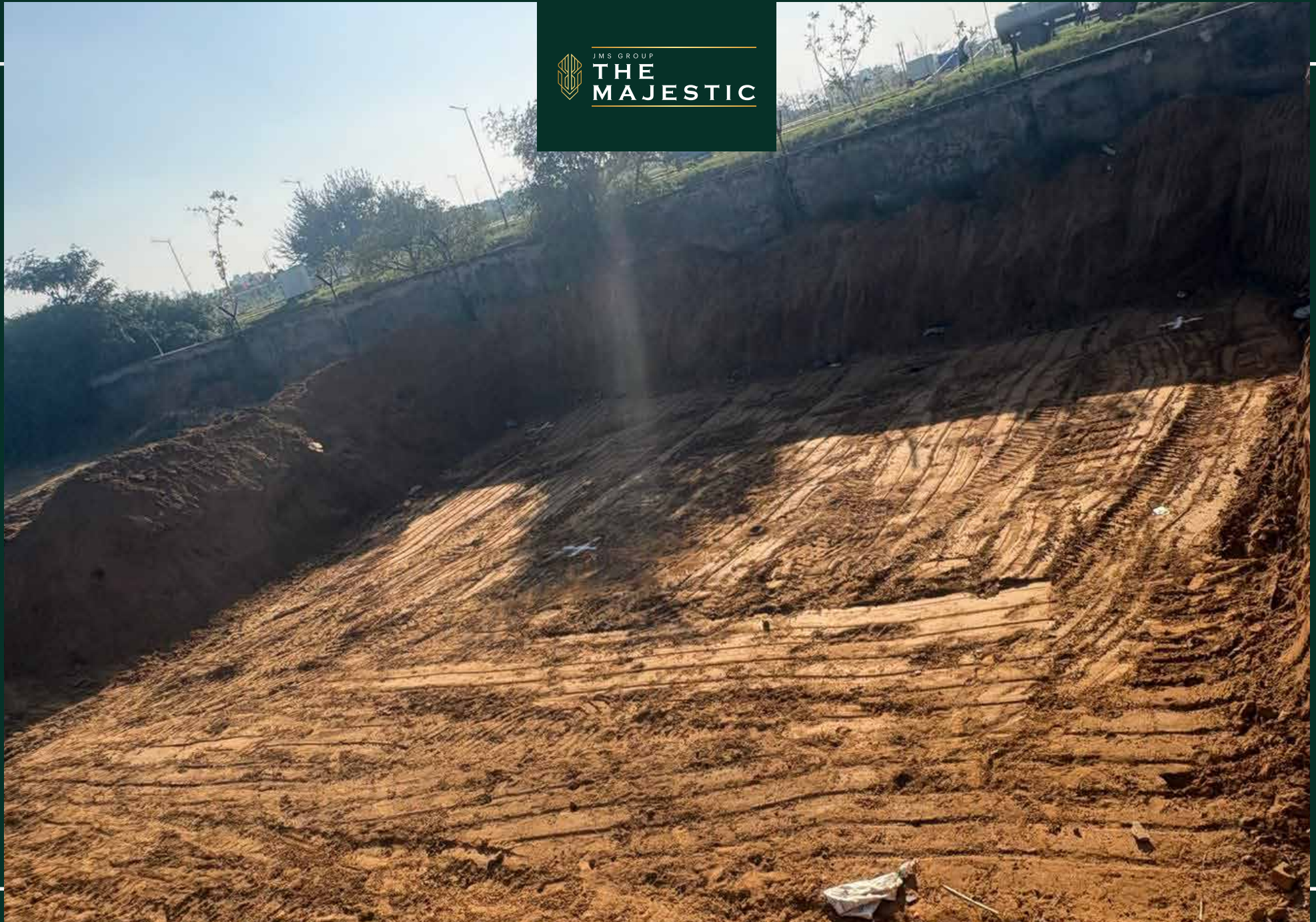
Plot no. 337, 339 & 340 Excavation work in progress
