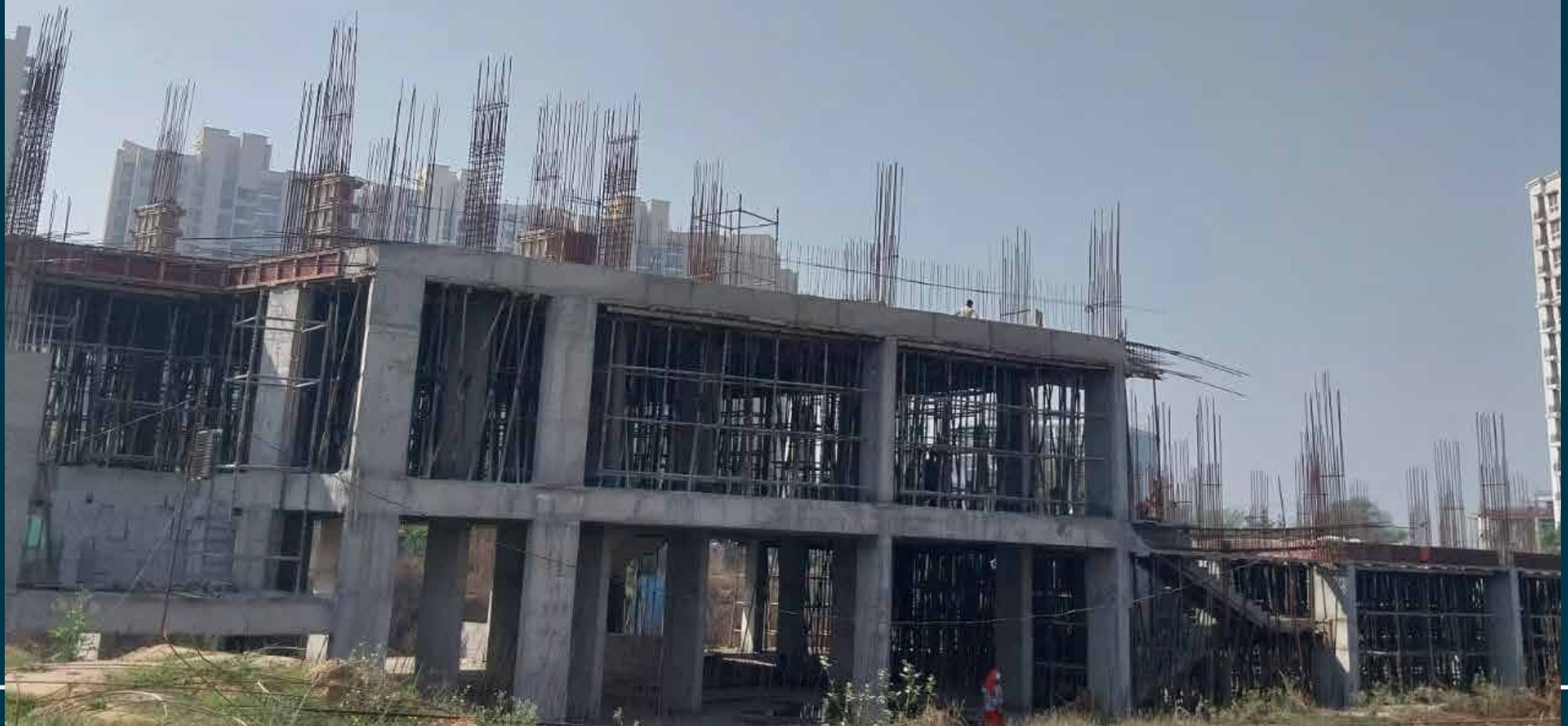
Underground floor and First floor slab casting work in progress
