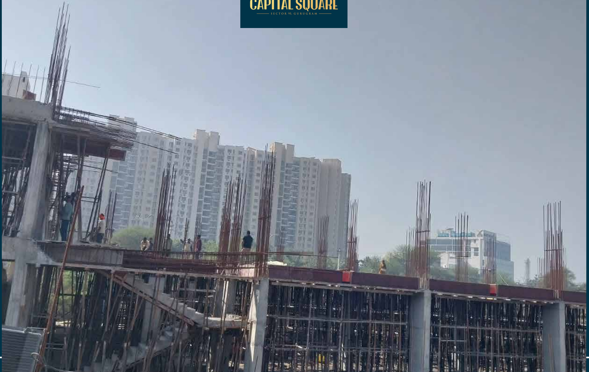
Underground floor and First floor slab casting work in progress
