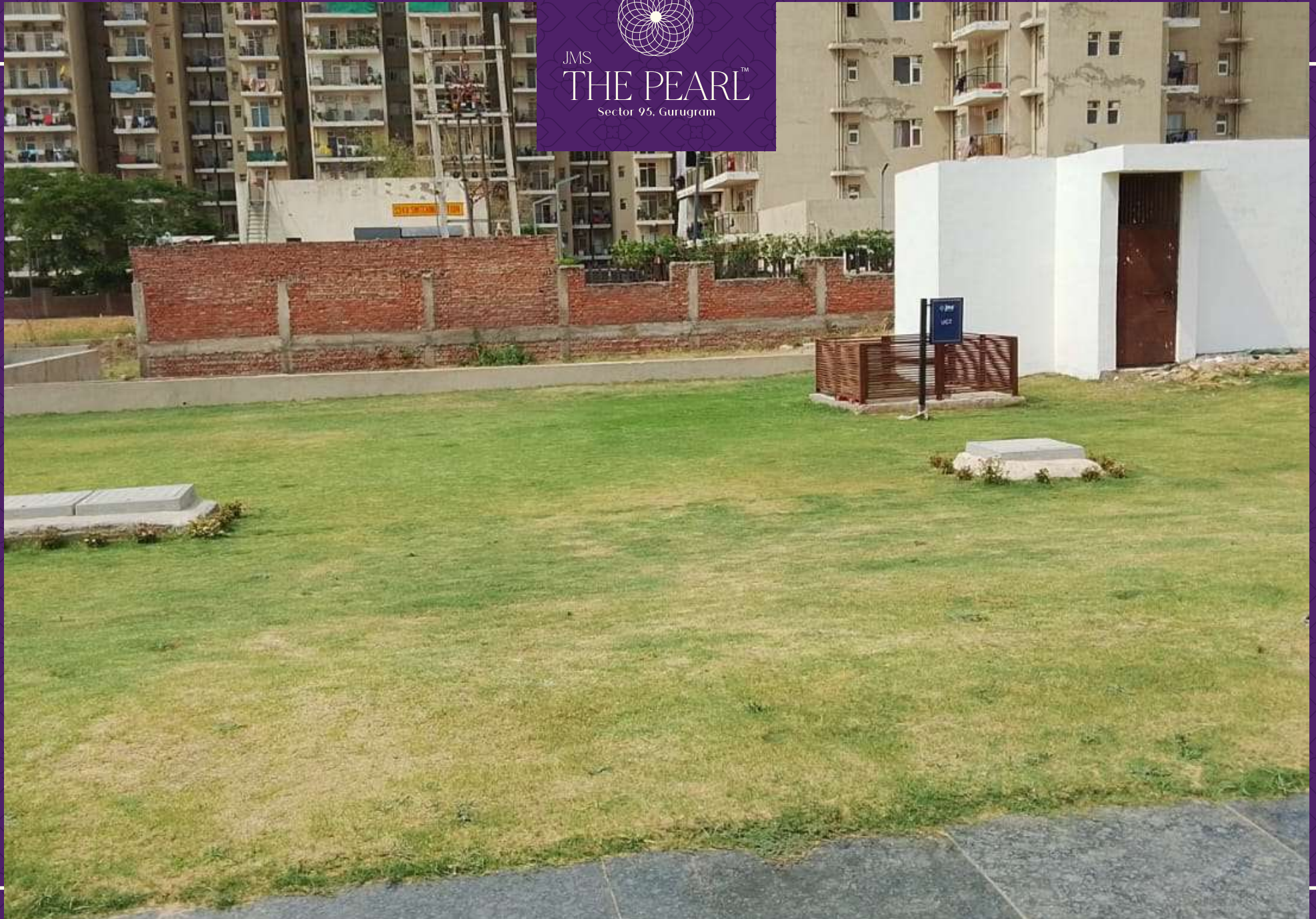
UGT construction in-progress
