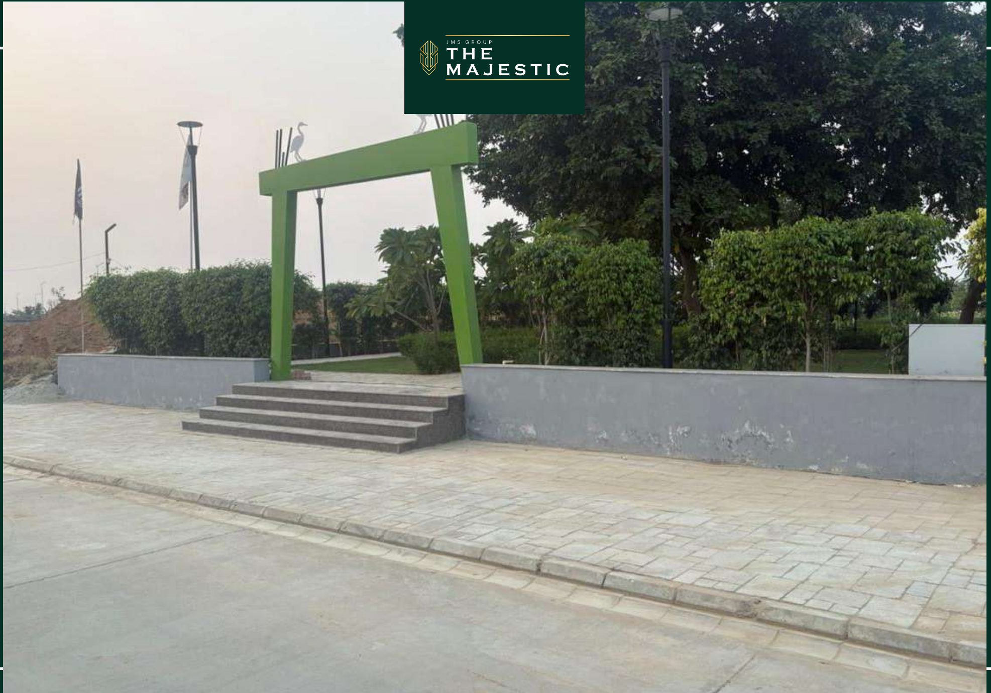
Park development work completed
