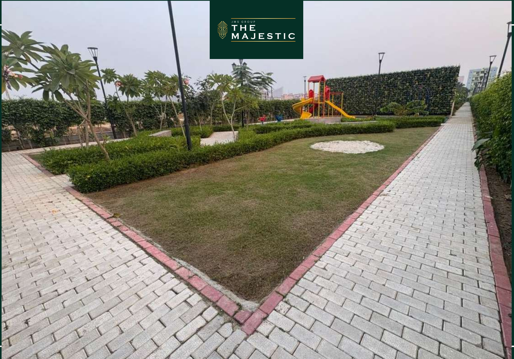
Park development work completed
