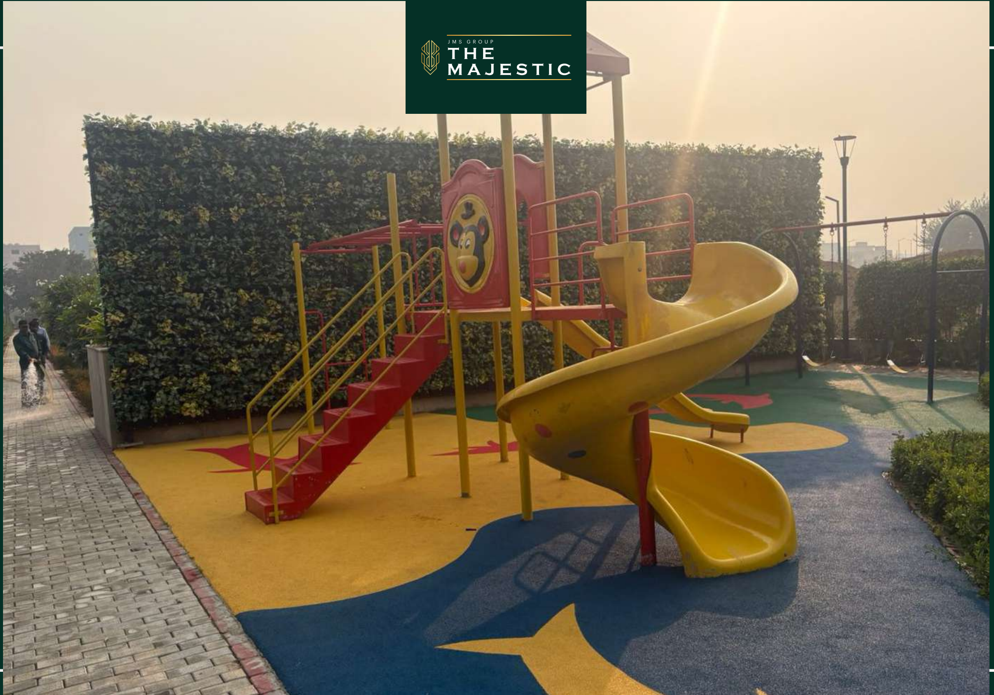
Kids play area work completed
