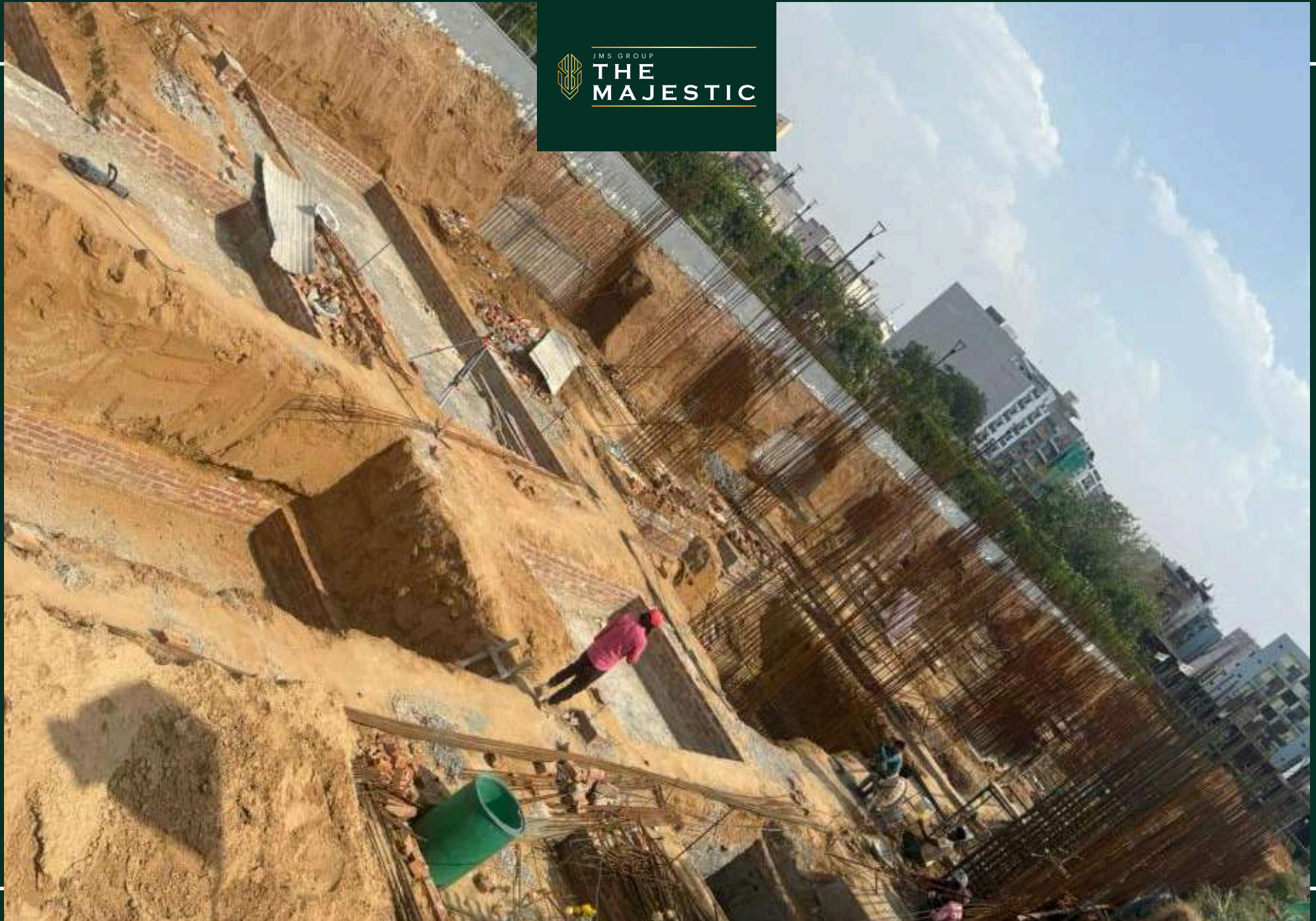
Plot 341-357 Retaining and footing work 90% completed
