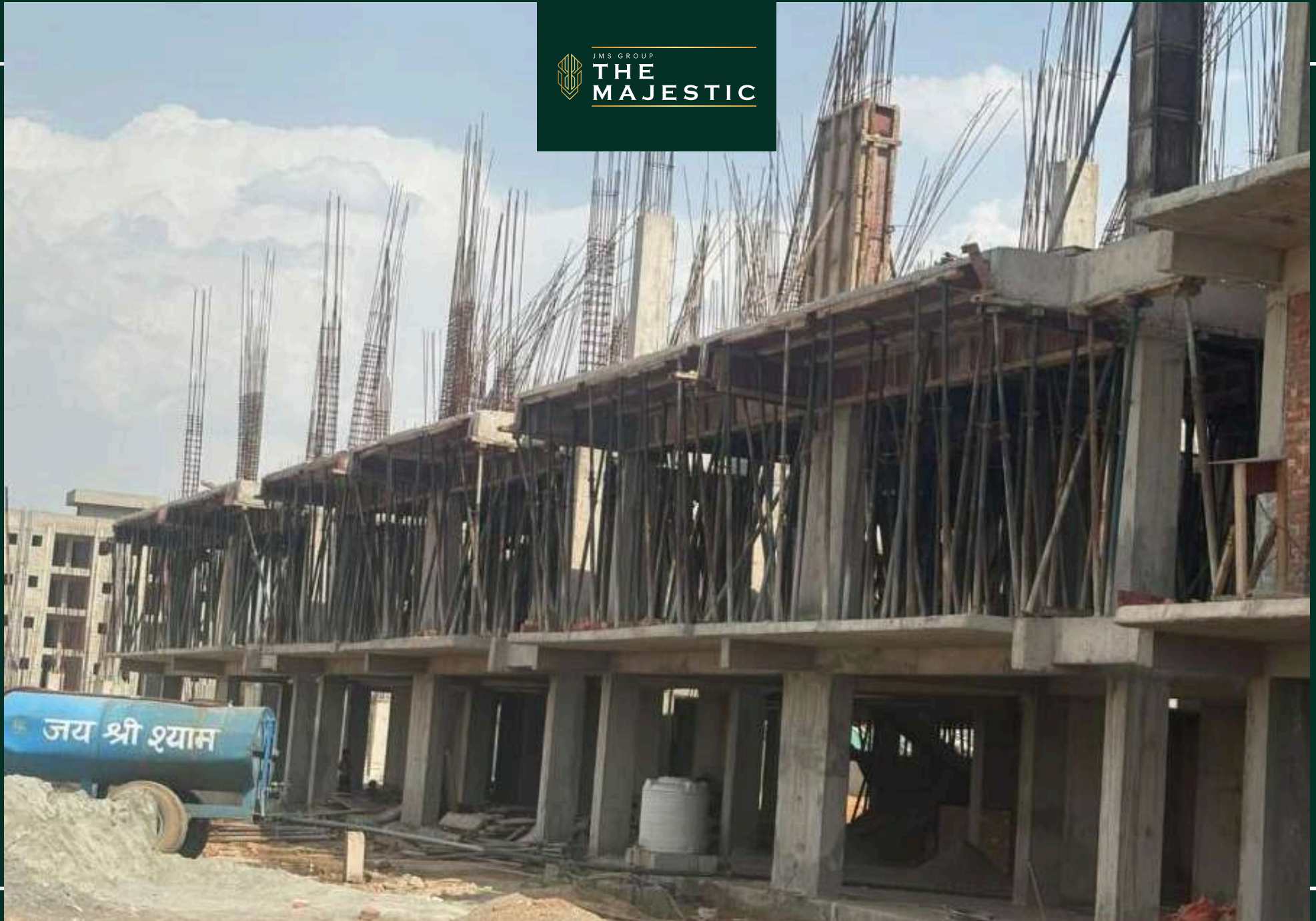
Plot 368-373 Above 2nd floor column shuttering work in progress
