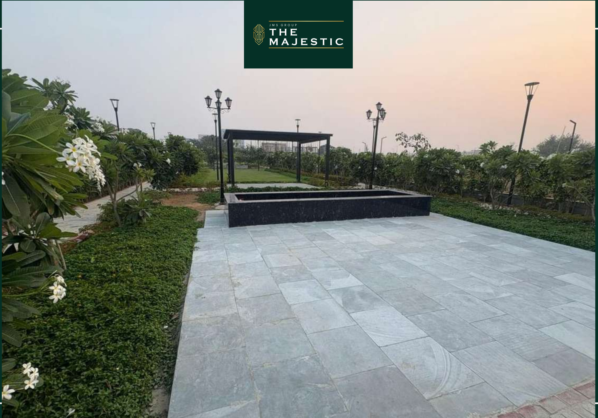
Park development work completed
