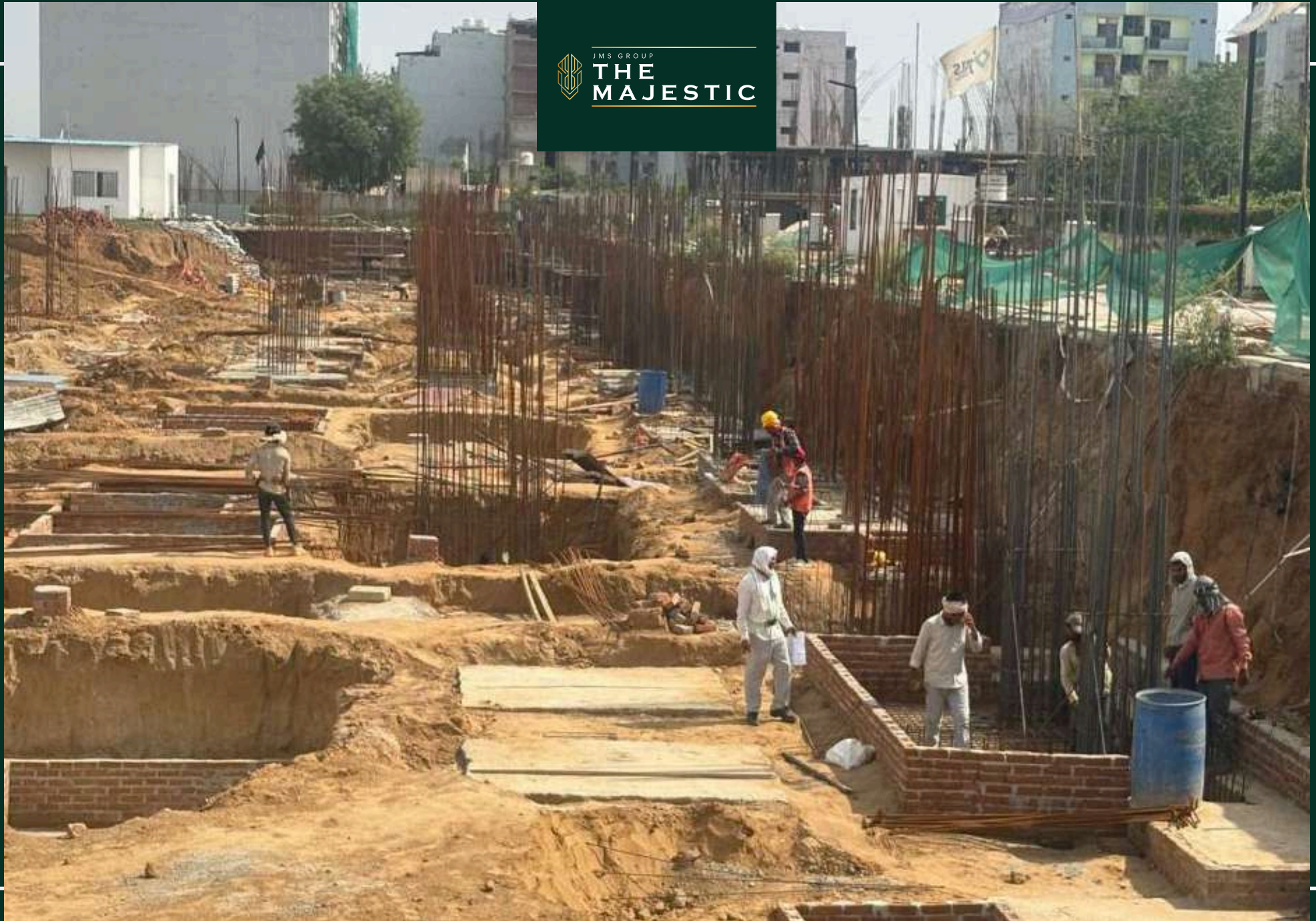
Plot 237-240 Retaining wall and RCC casting completed
