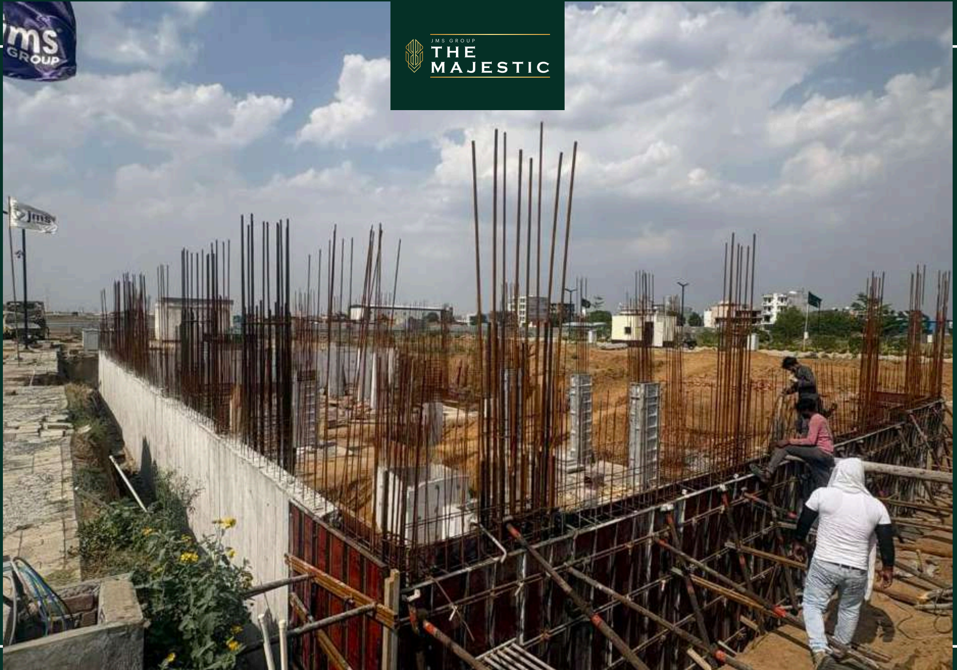
Plot 298-318 Retaining wall completed & Plot 301-318 retaining and shuttering work in progress
