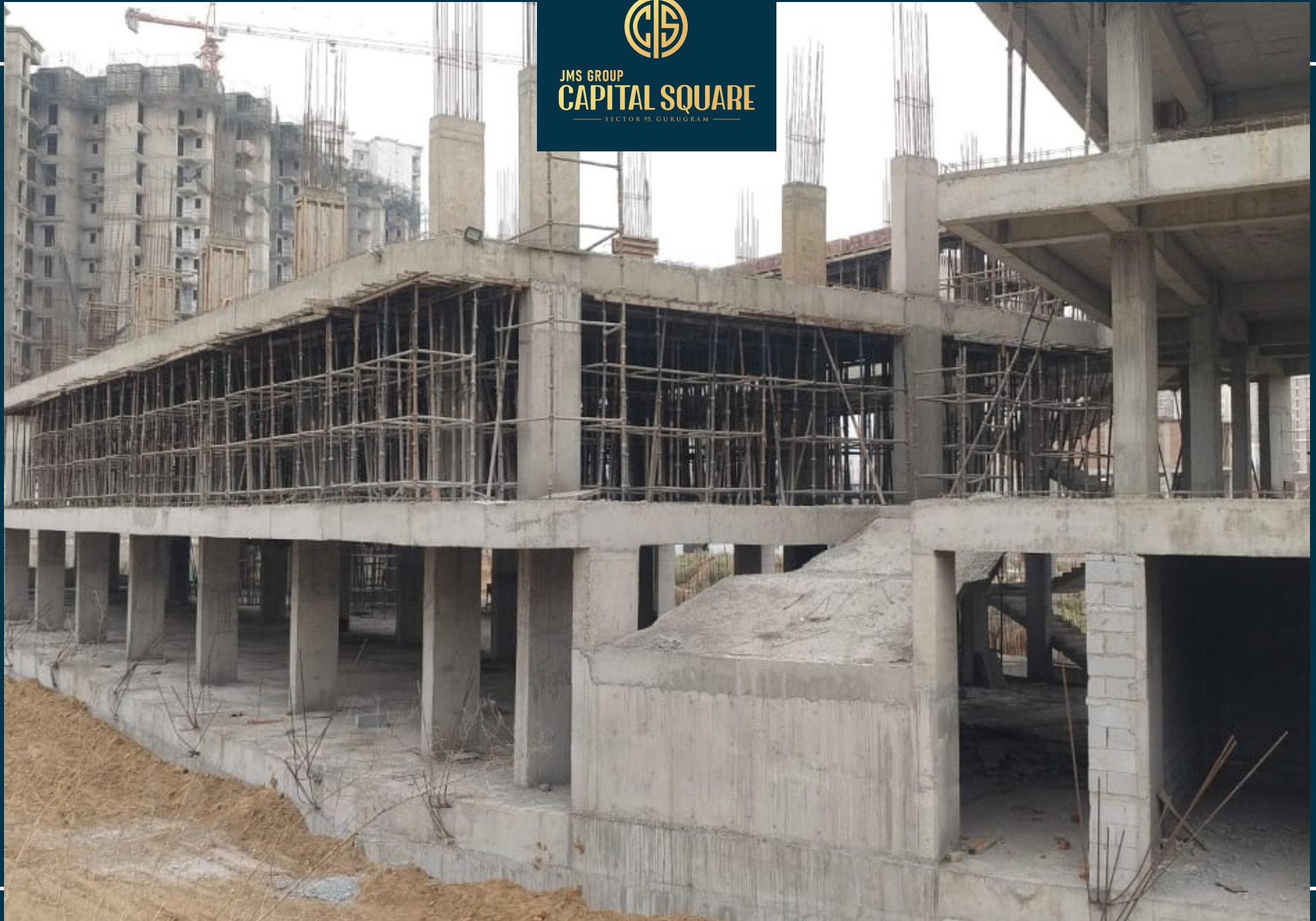
1st floor slab pouring work is in progress
