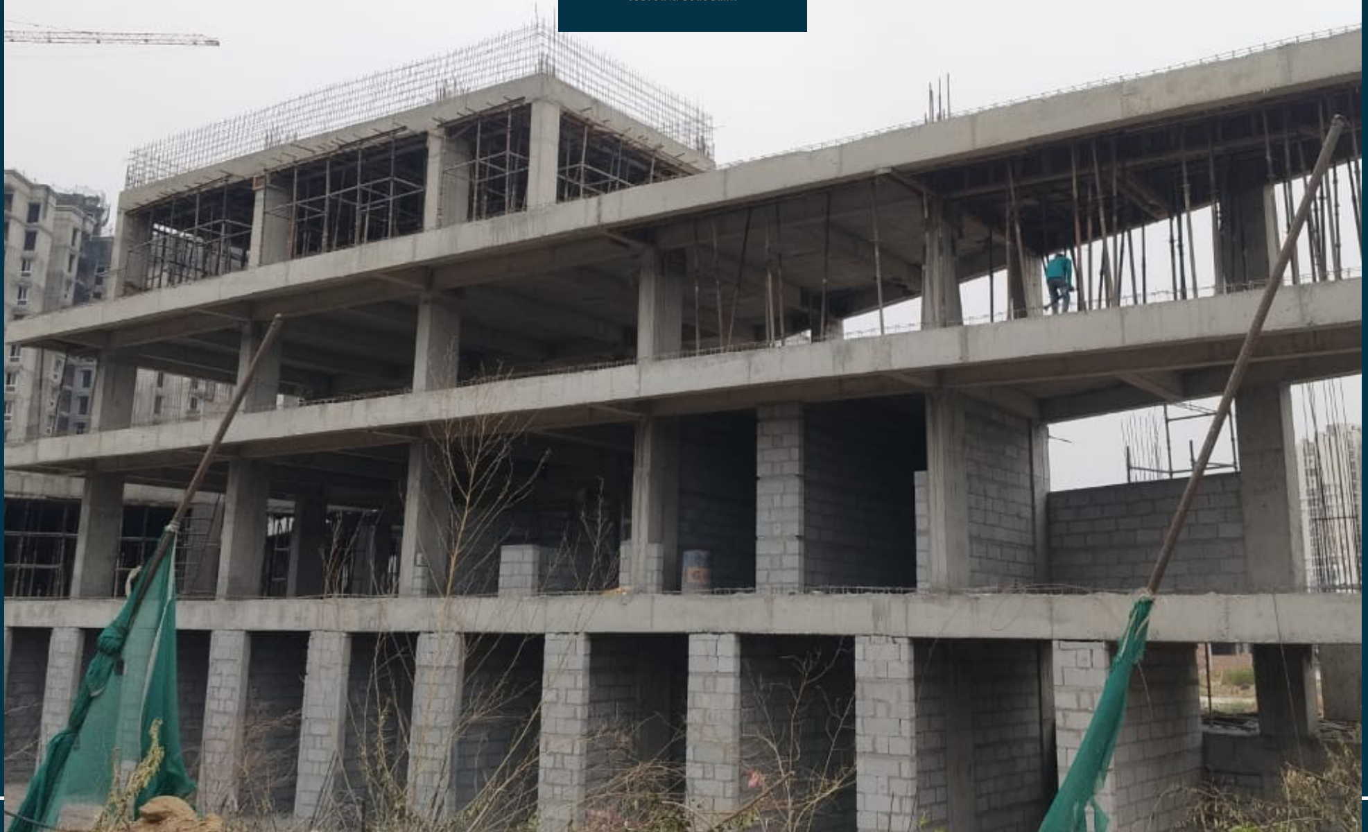
Block work is in progress
