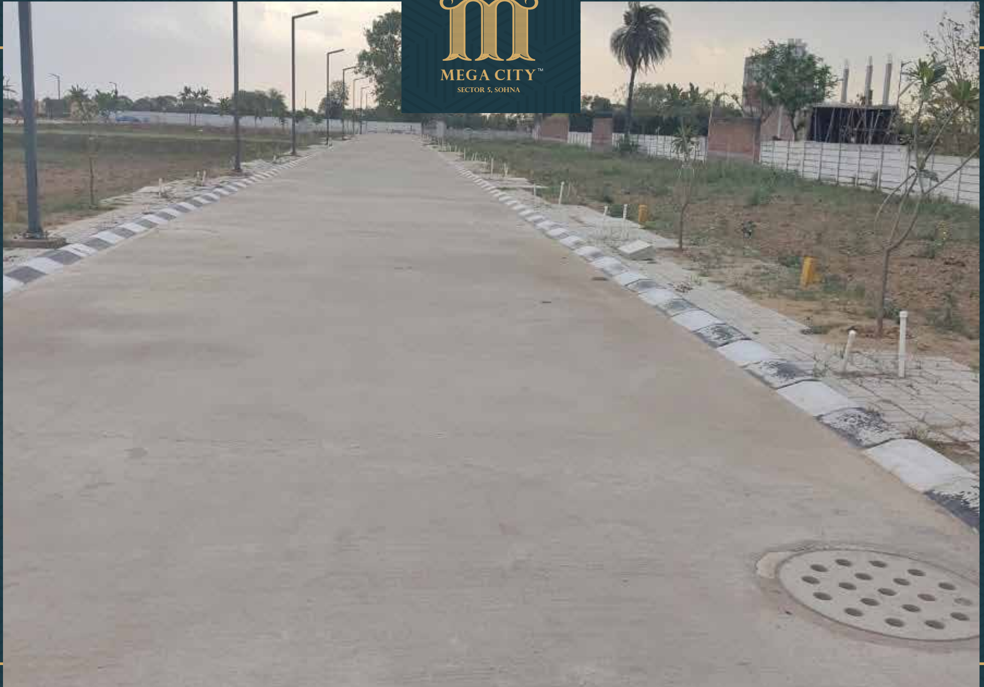
Road no. 1 development work completed including electrical cable lines
