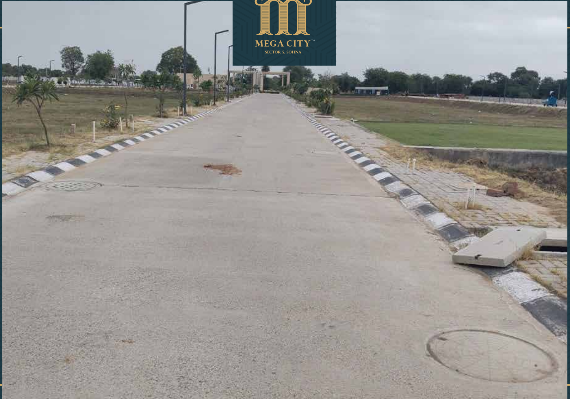
Road no. 4 development work completed including electrical cable lines
