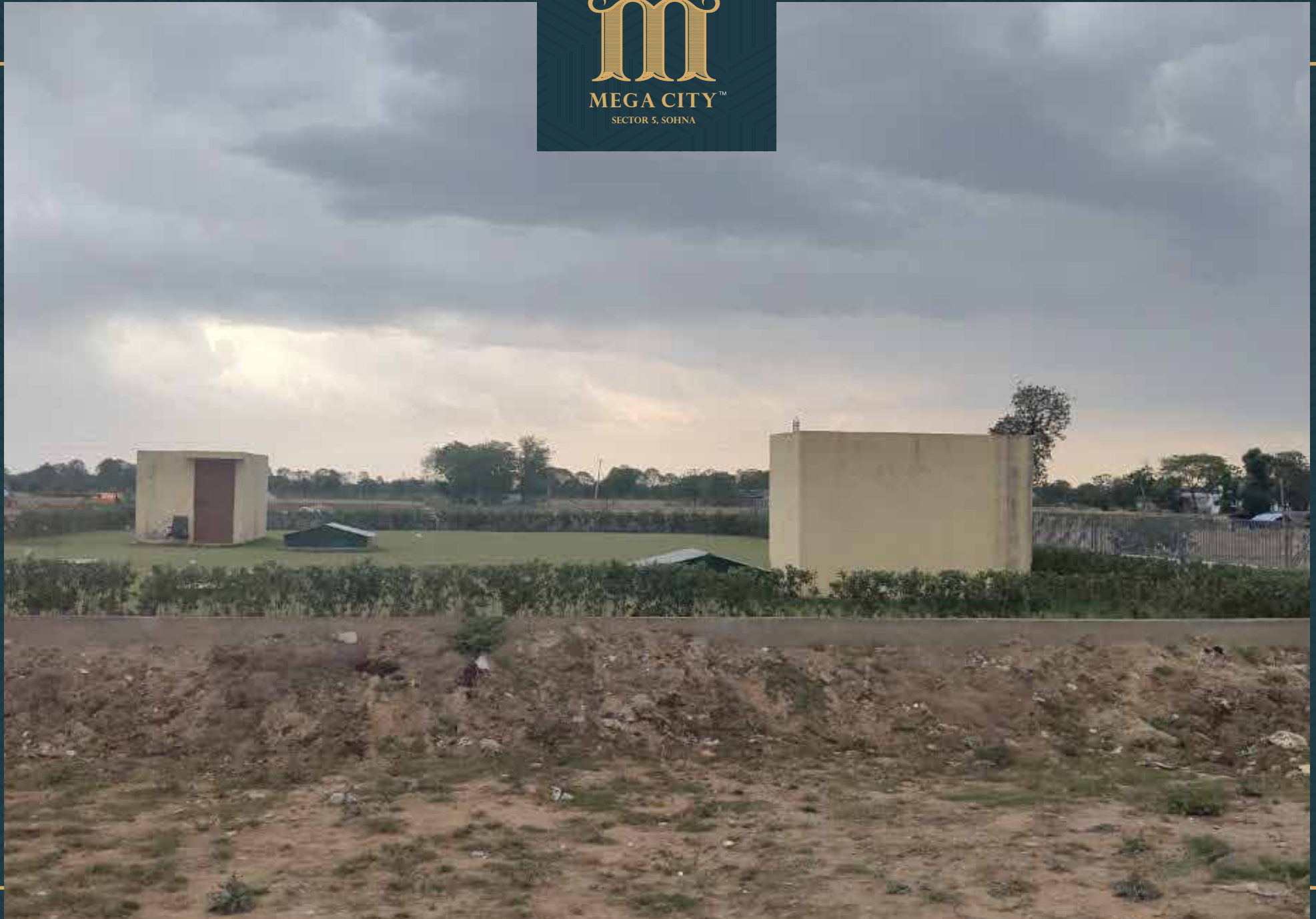
STP and UGT work completed
