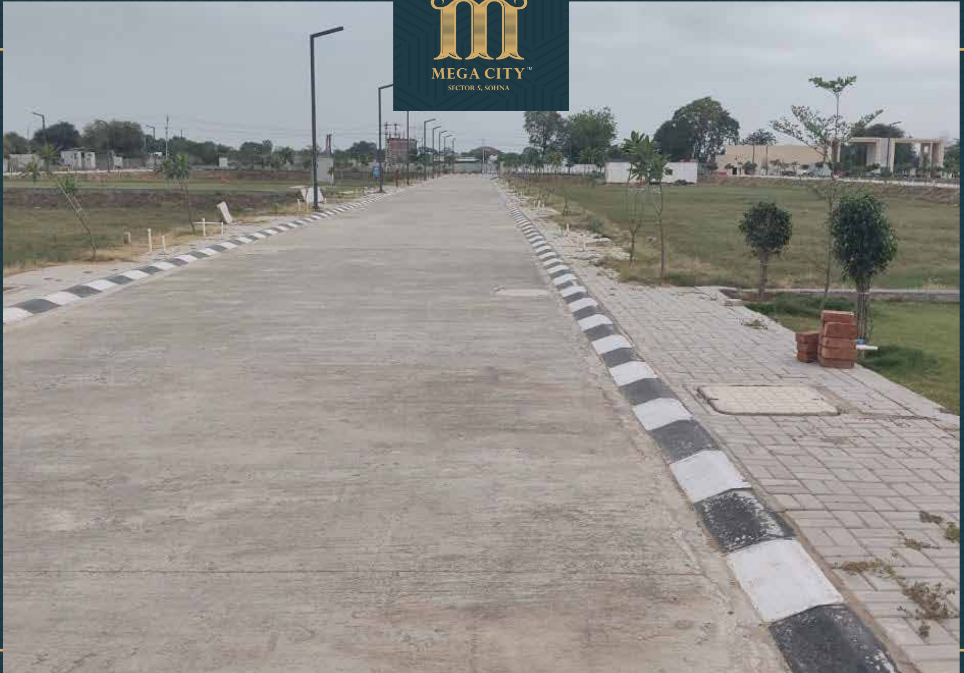
Road no. 2 development work completed including electrical cable lines
