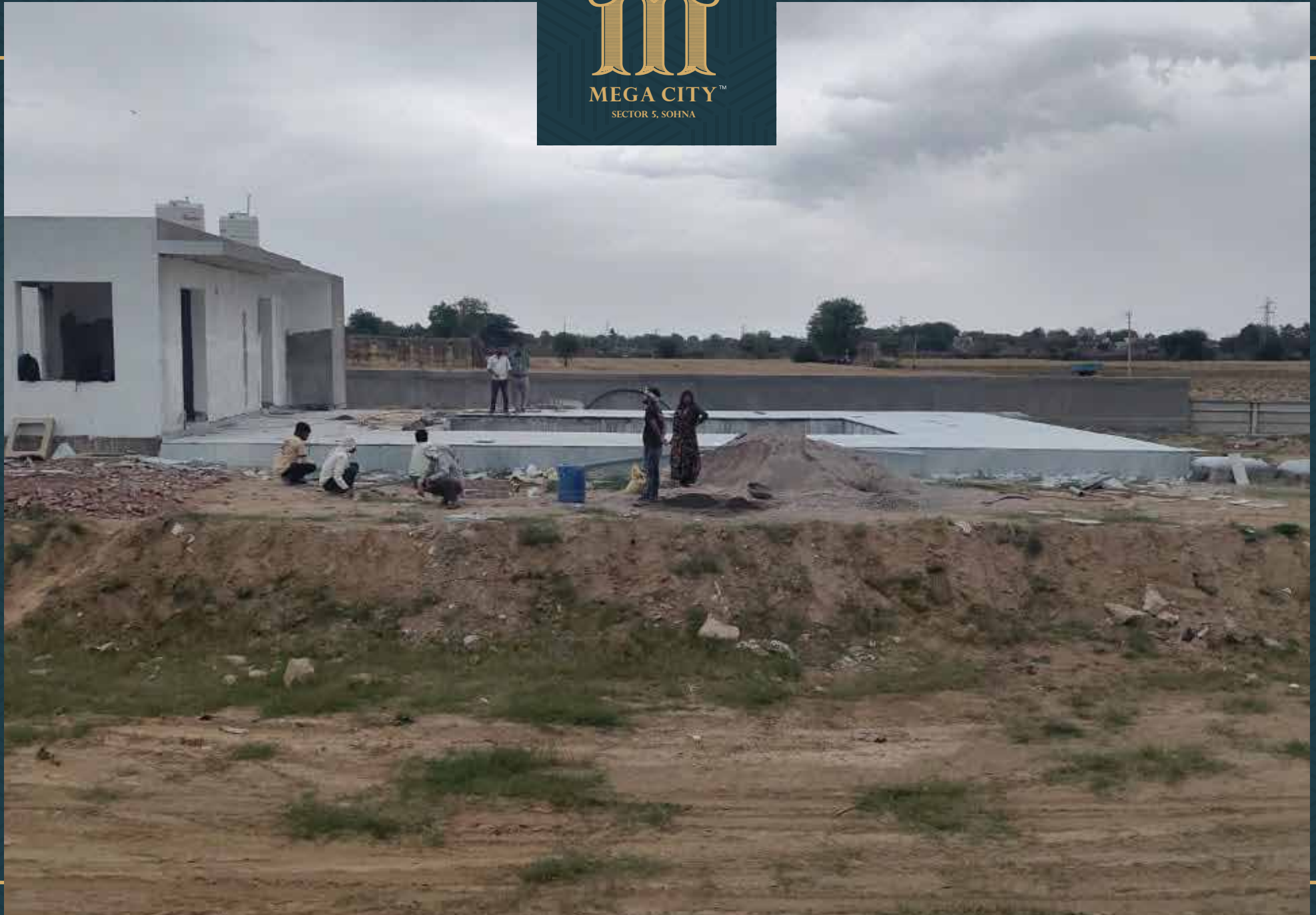
Swimming pool final finishing work in progress
