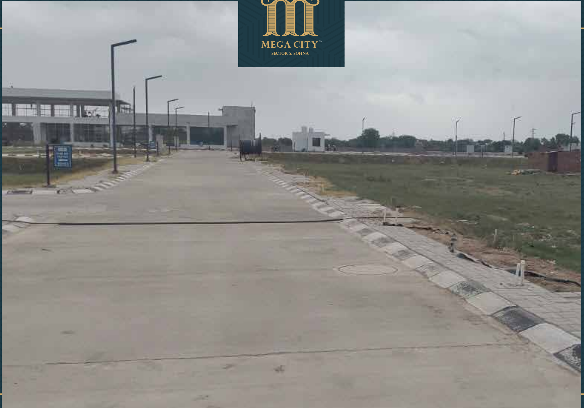
Road no. 7 development work completed including electrical cable lines
