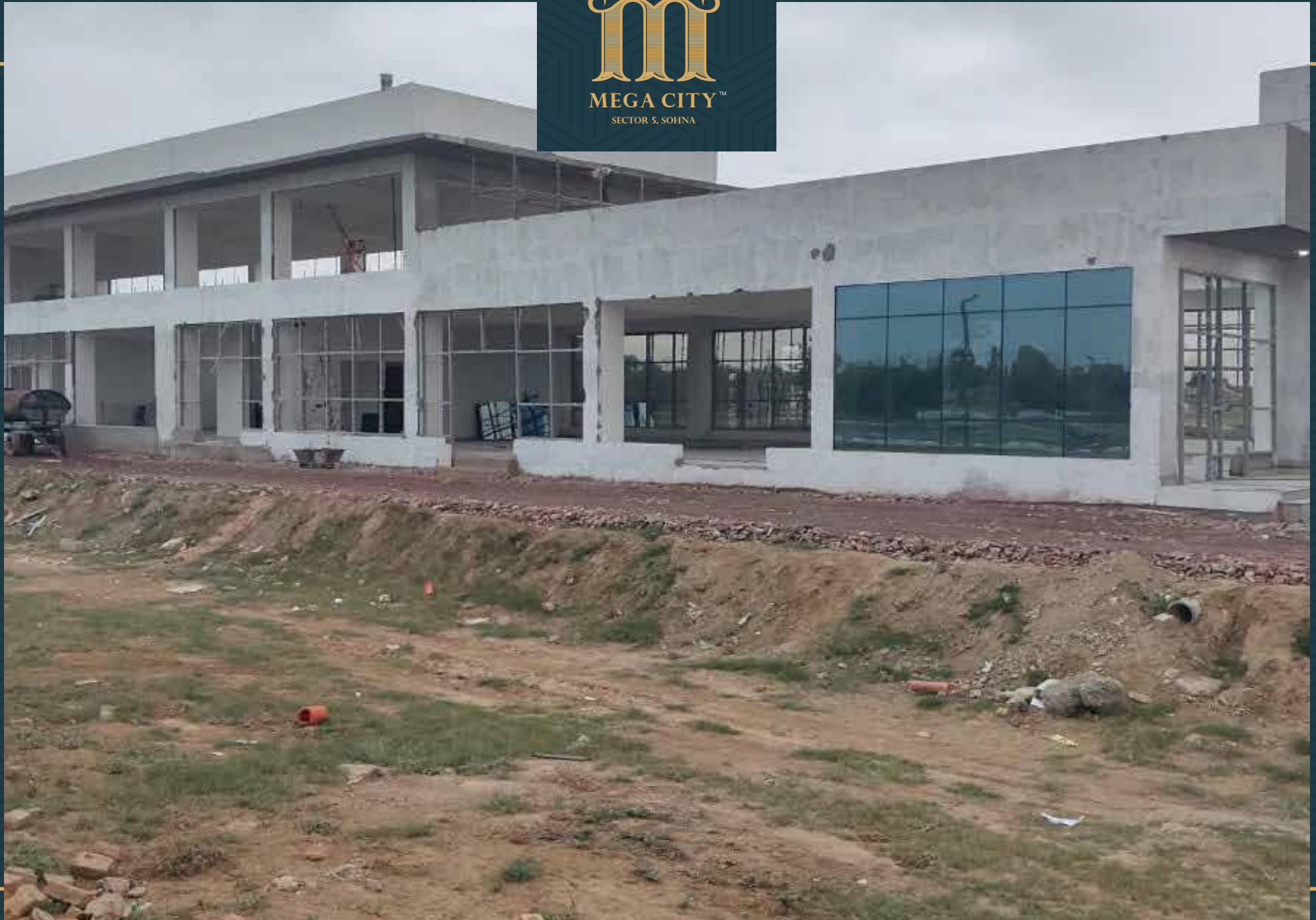
Club house final finishing work in progress
