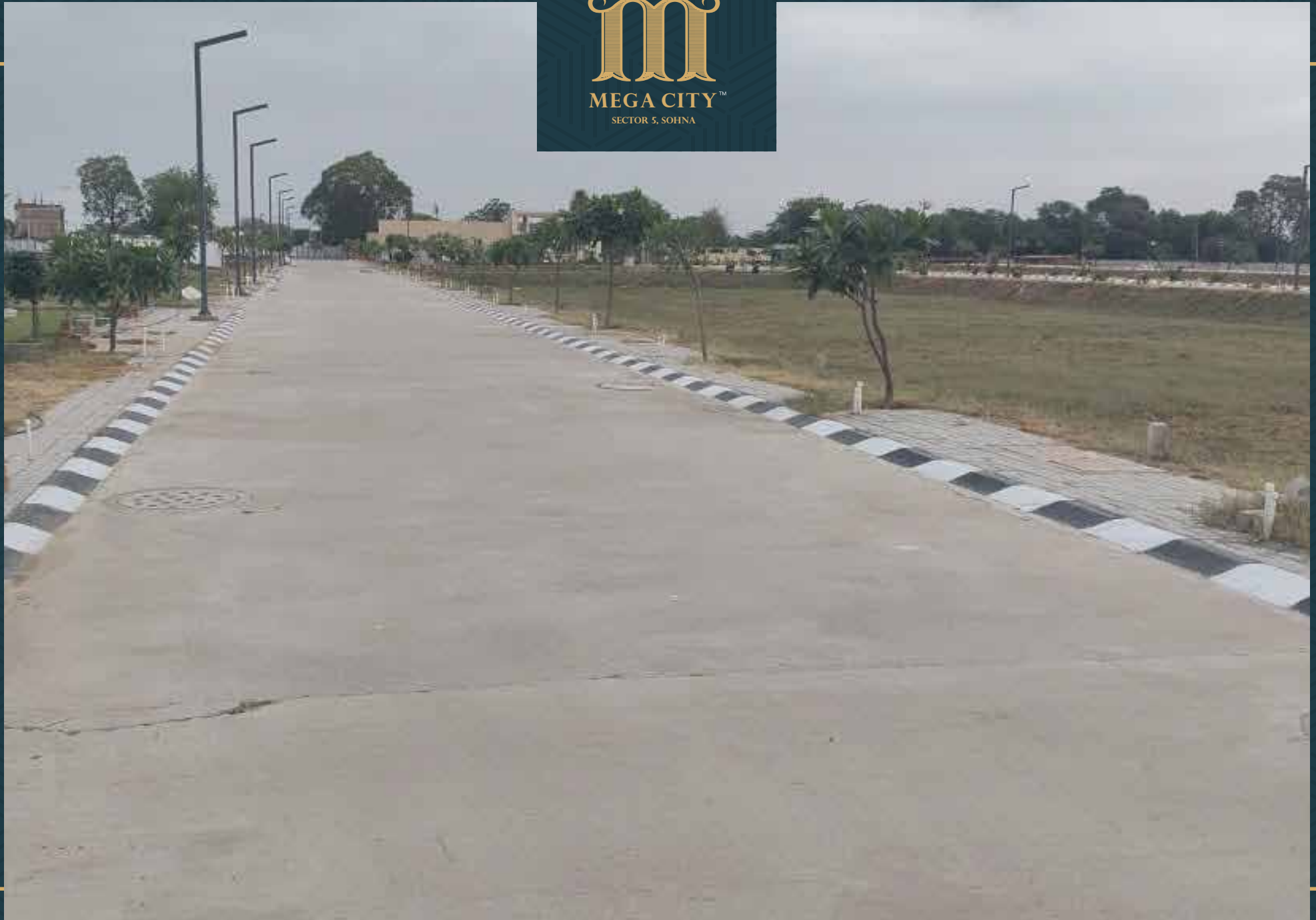
Road no. 3 development work completed including electrical cable lines
