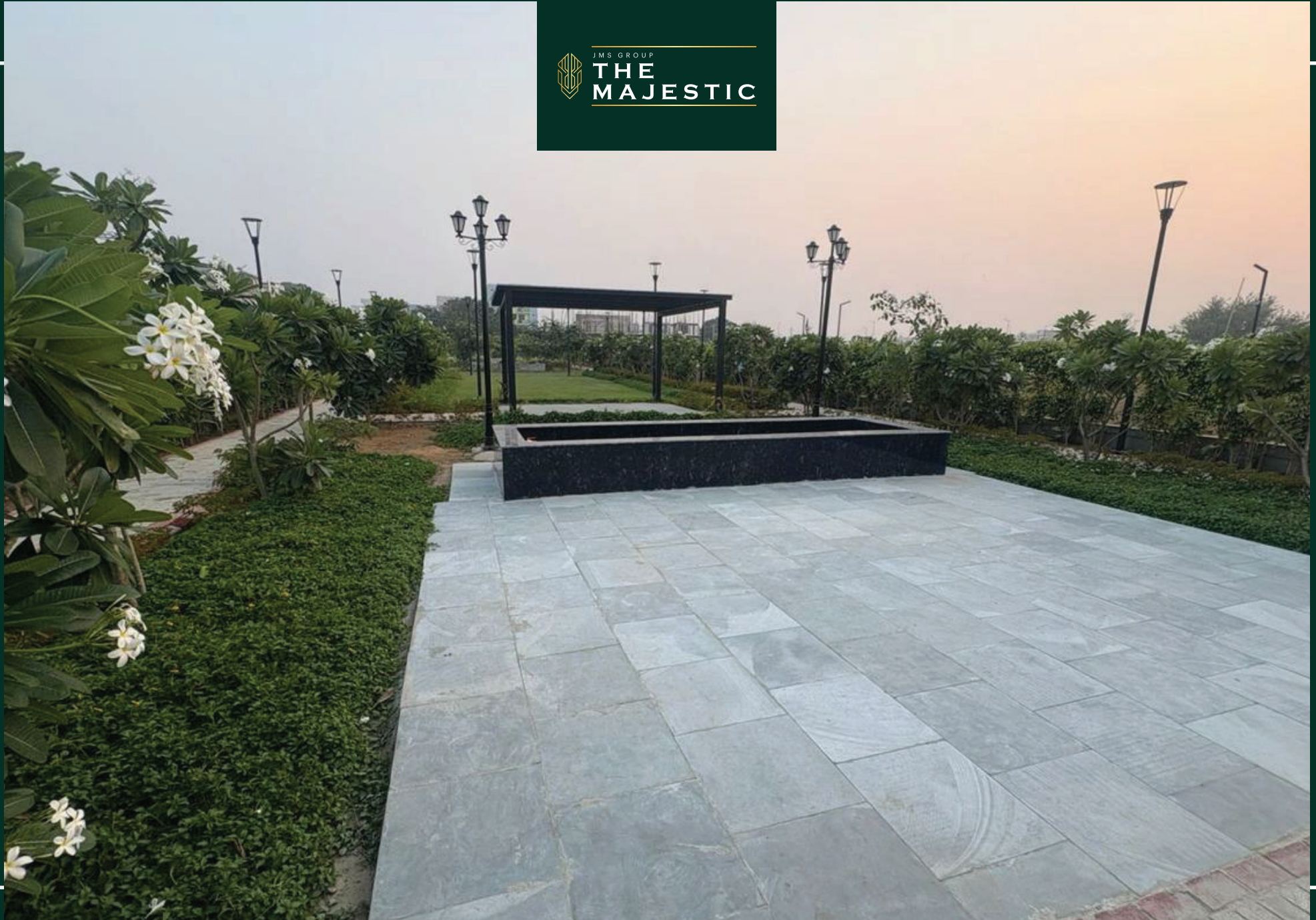
Park development work completed
