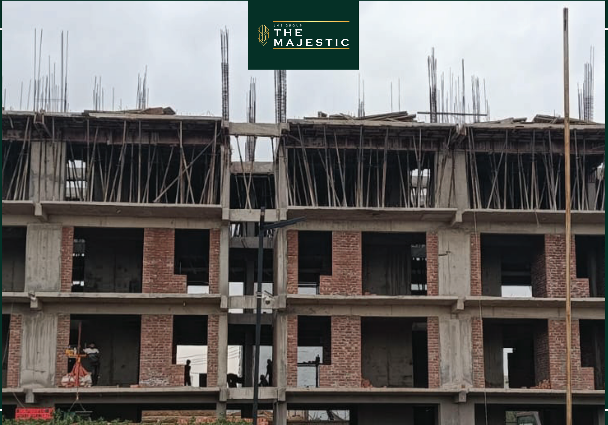
Plot no. 374-378 4th floor RCC casting completed
