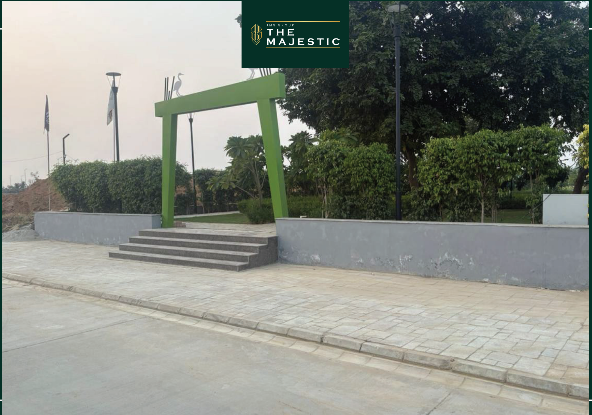
Park development work completed
