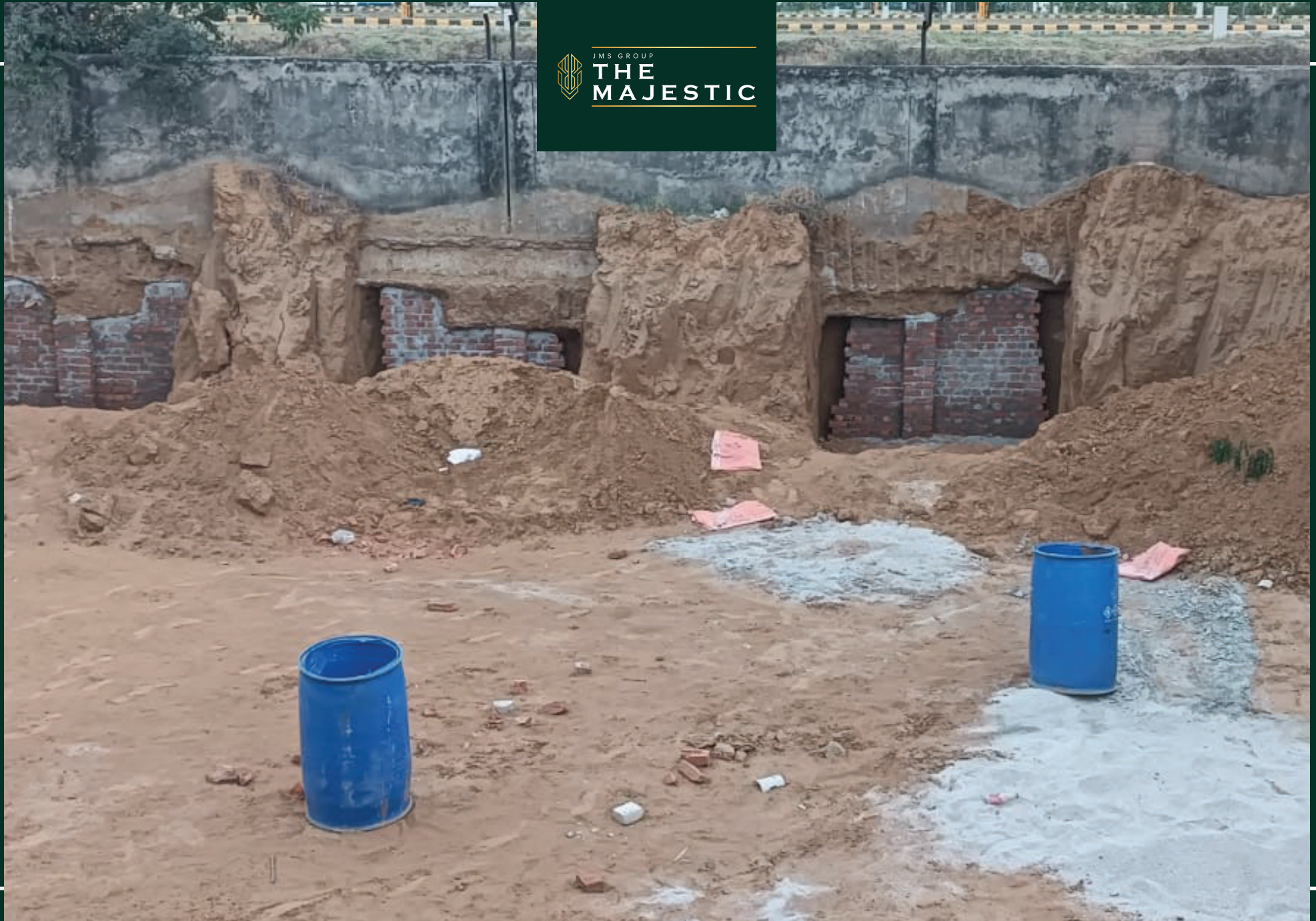
Plot no. 339-340 foundation brick work in progress
