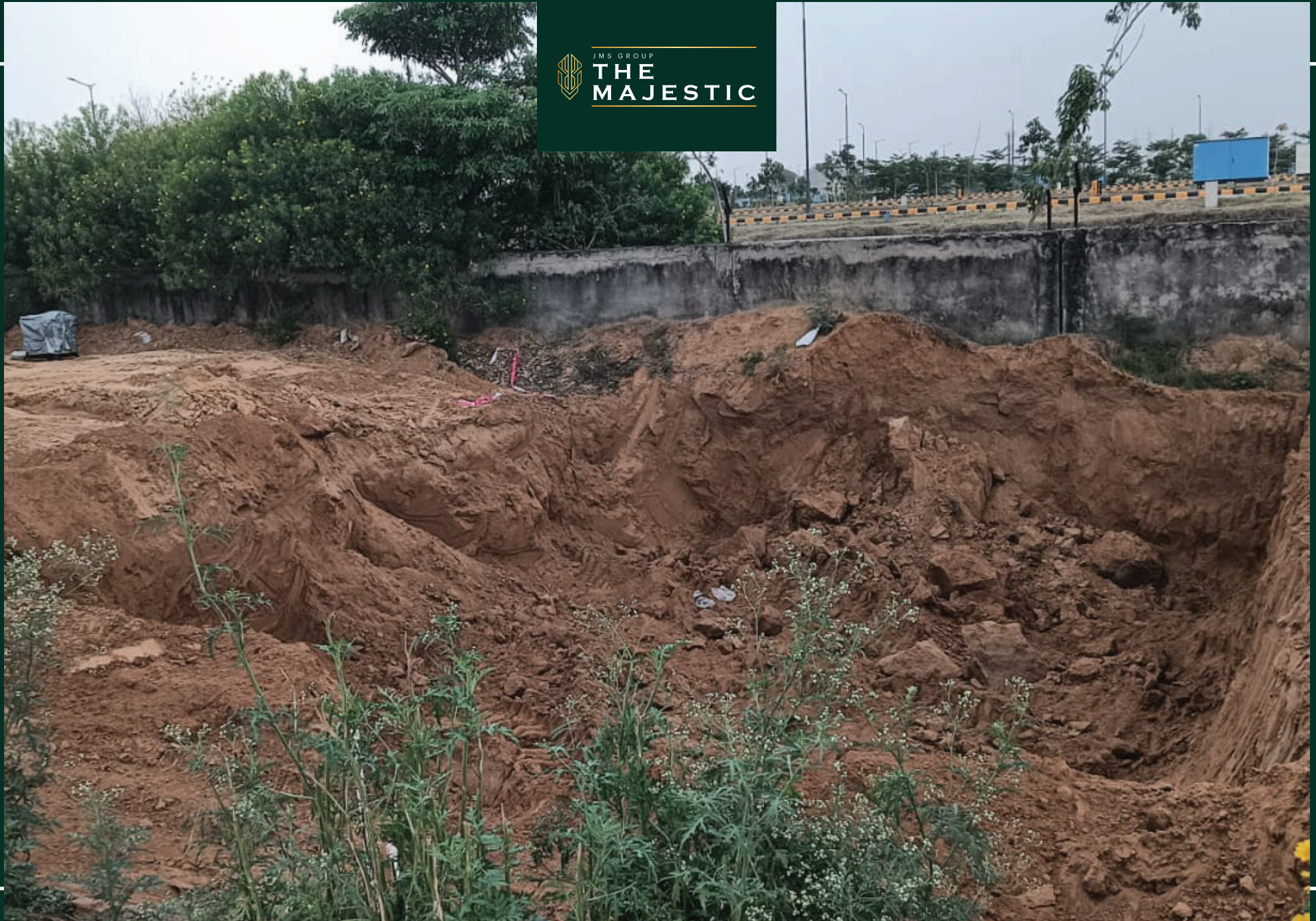
Plot no. 337 excavation work in progress
