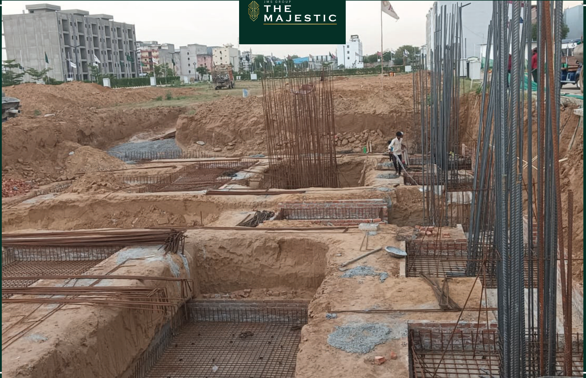
Plot no. 237-240 casting work in progress
