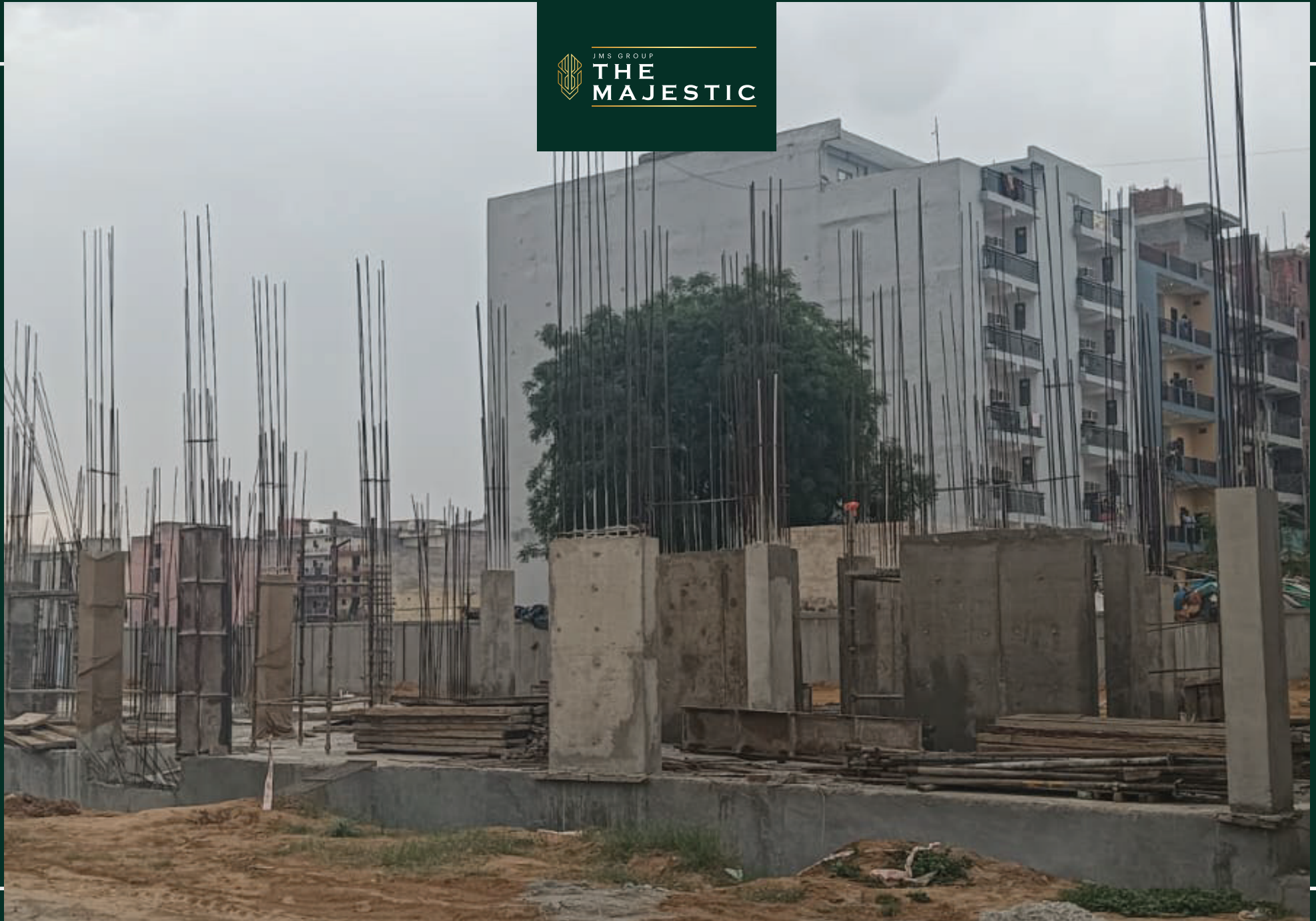
Plot no. 363-368 column casting and steel fixing work in progress
