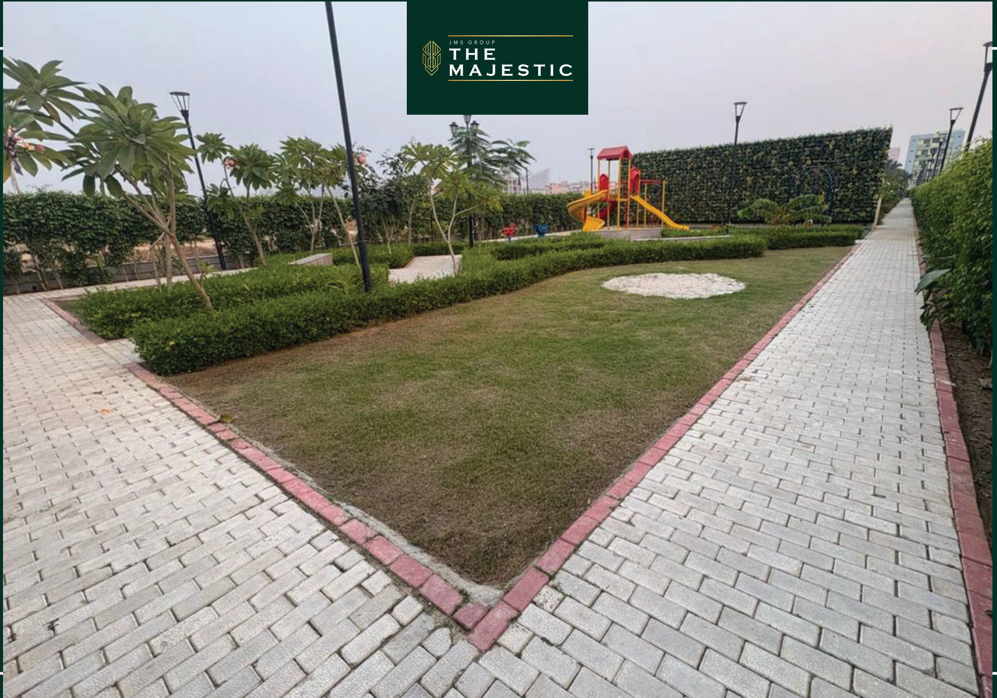
Park development work completed
