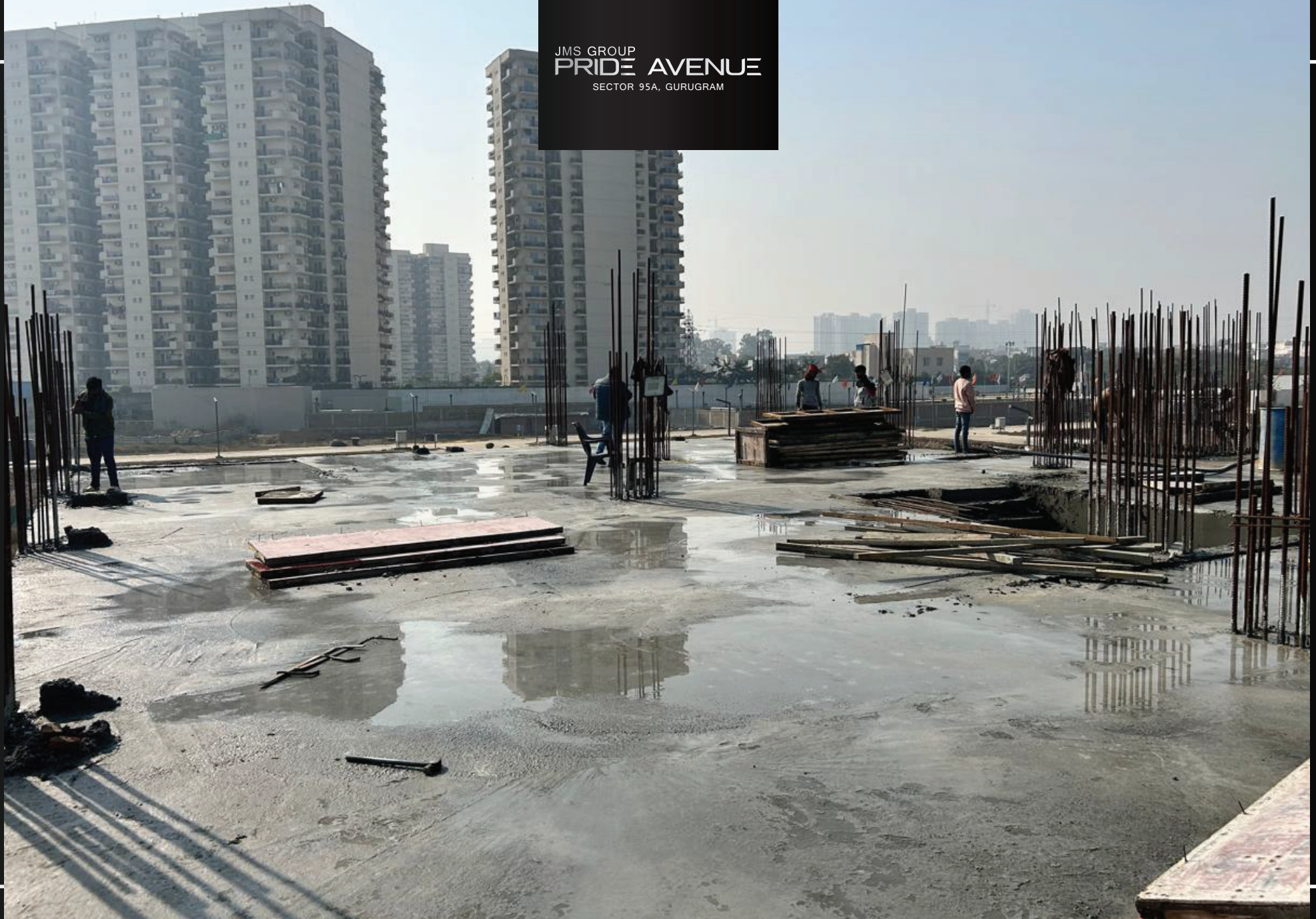
First Floor slab casting work completed
