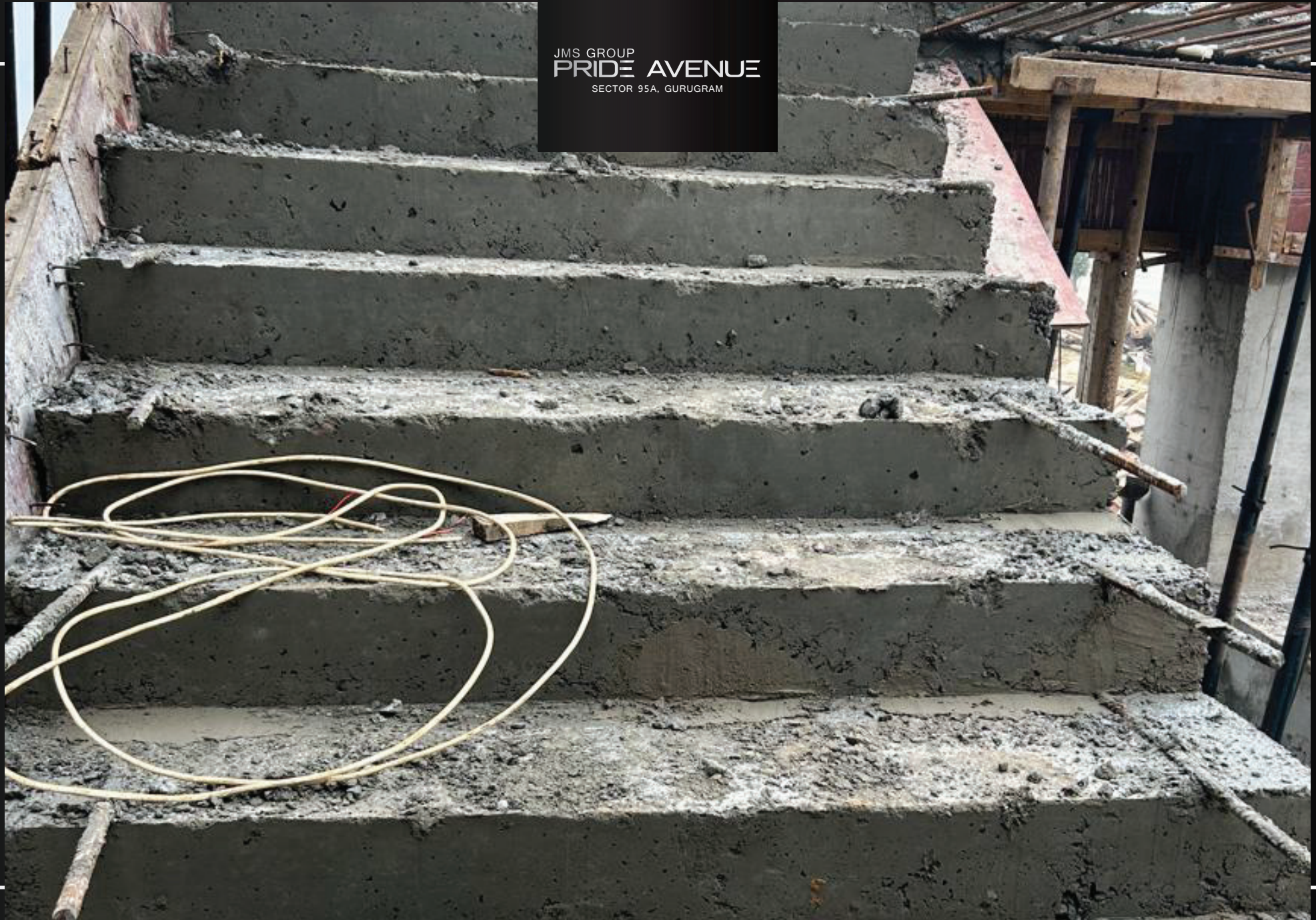
Staircase casting work completed
