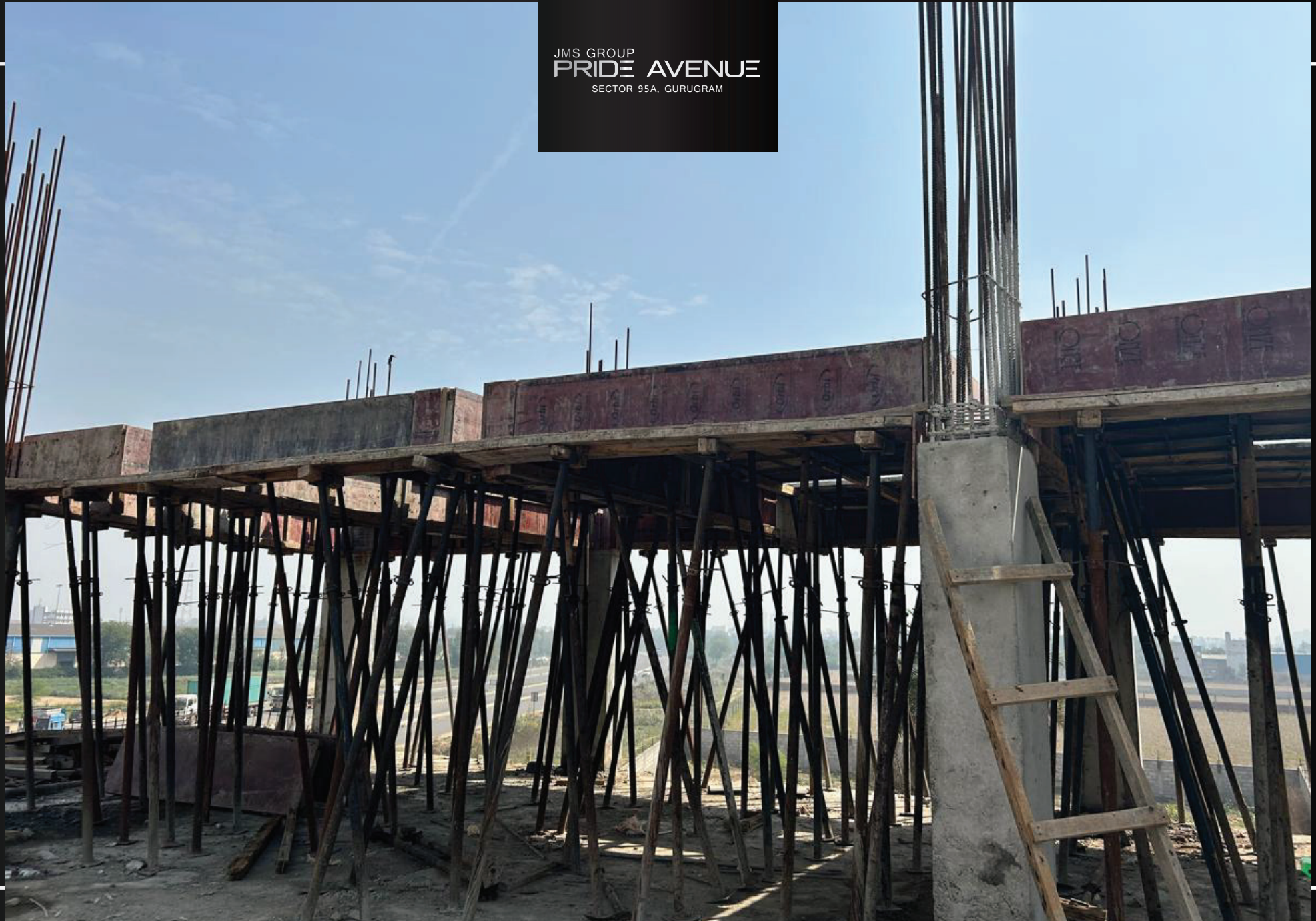
3rd floor slab shuttering work in progress
