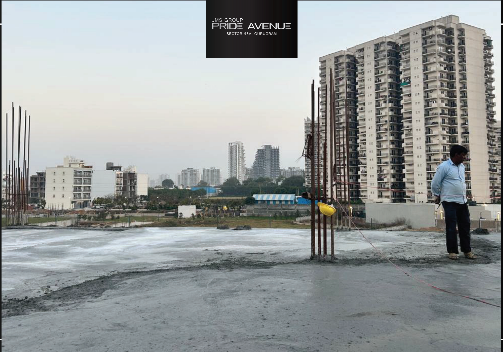
2nd floor slab casting work completed
