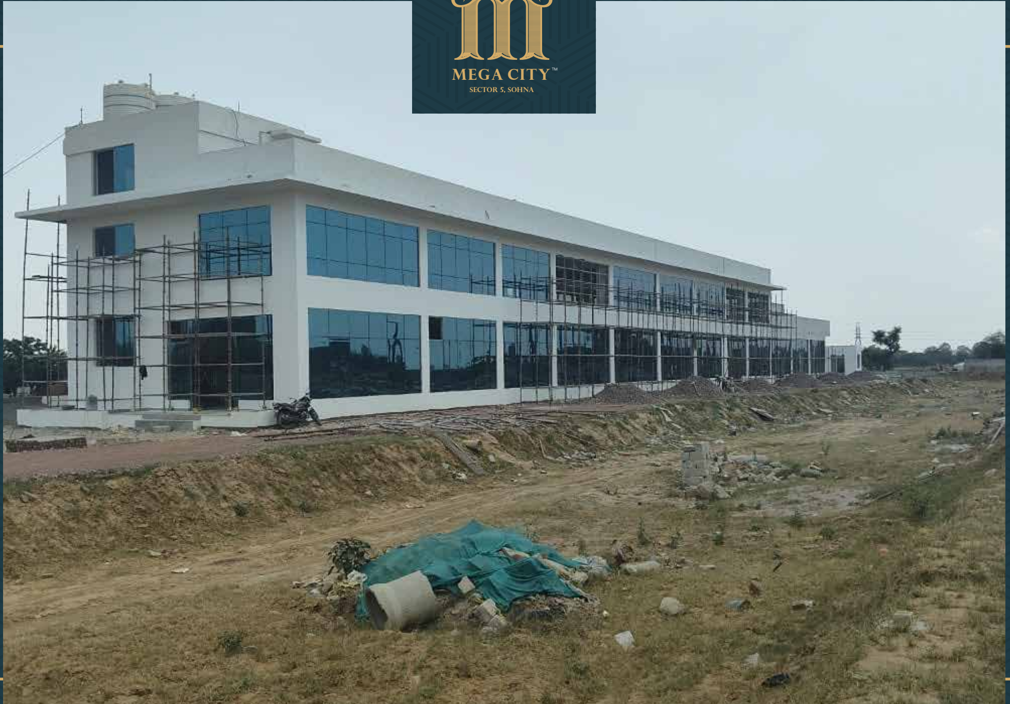
Clubhouse finishing work in progress
