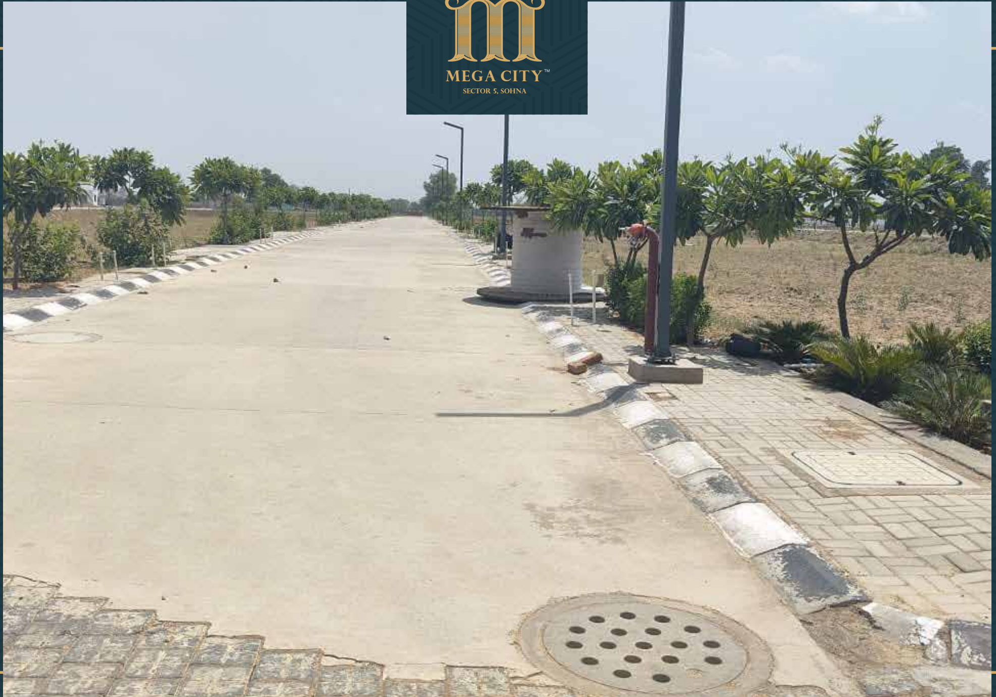
Road no. 4 development work completed
