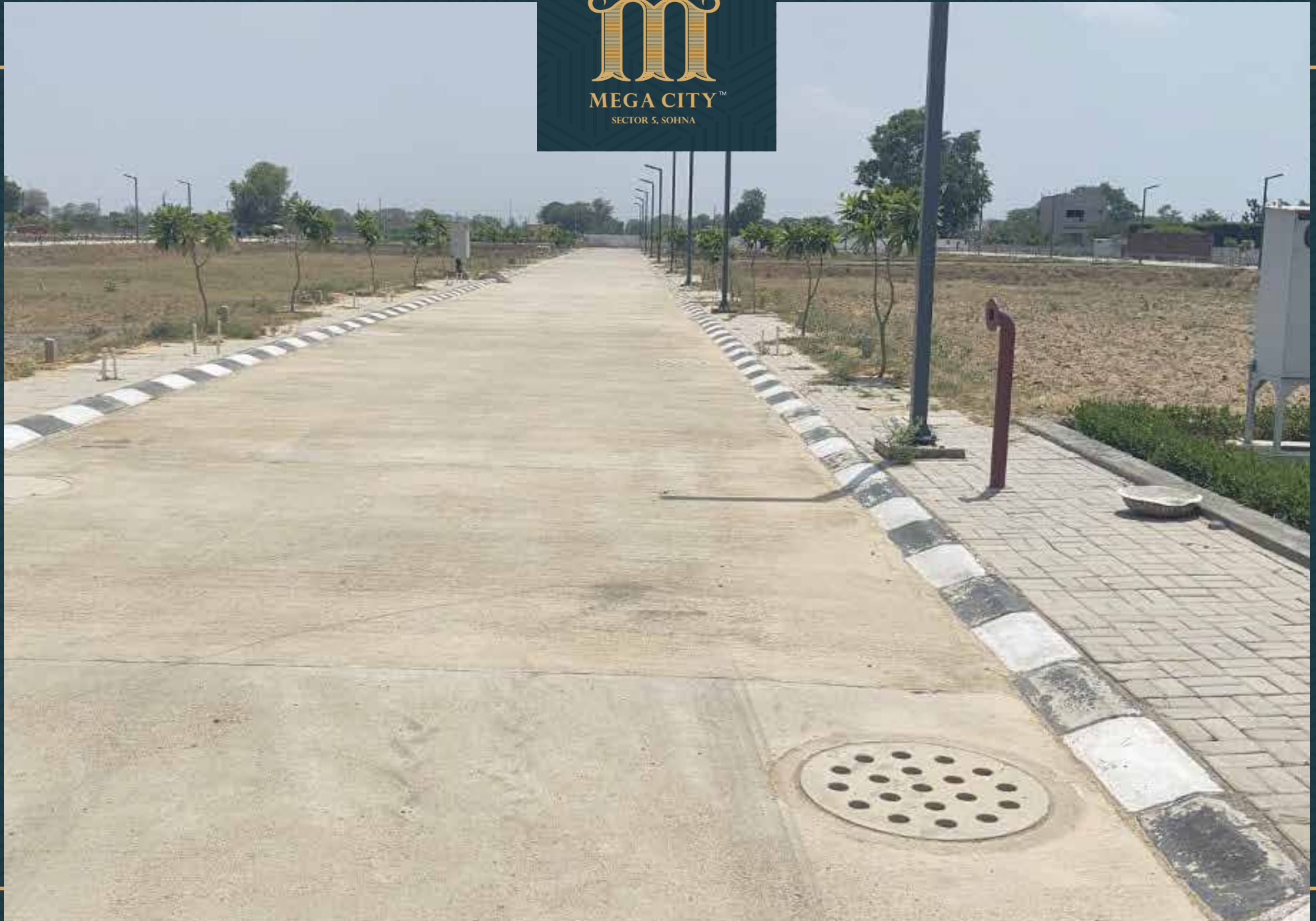
Road no. 2 development work completed
