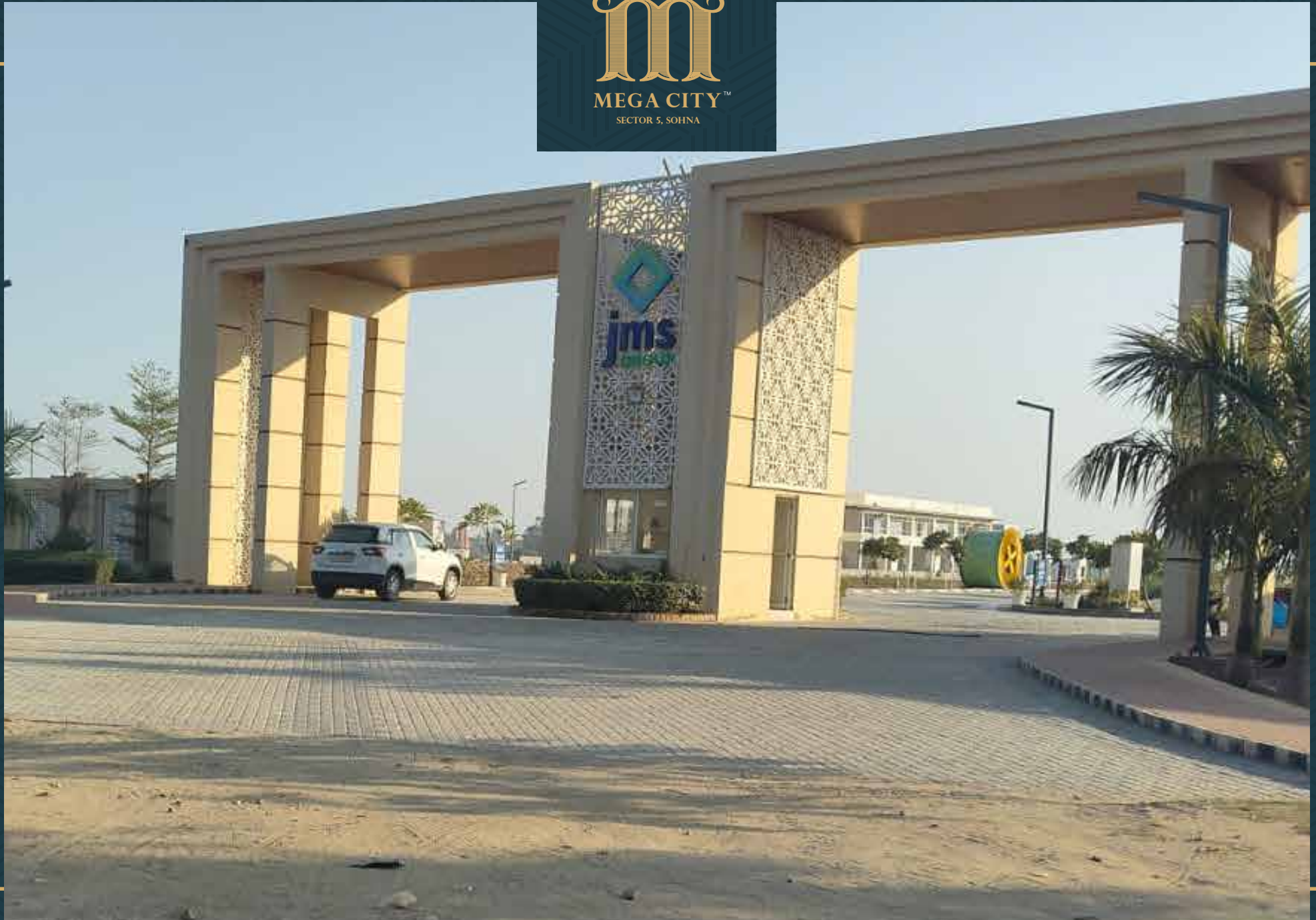
Entry Gate work completed
