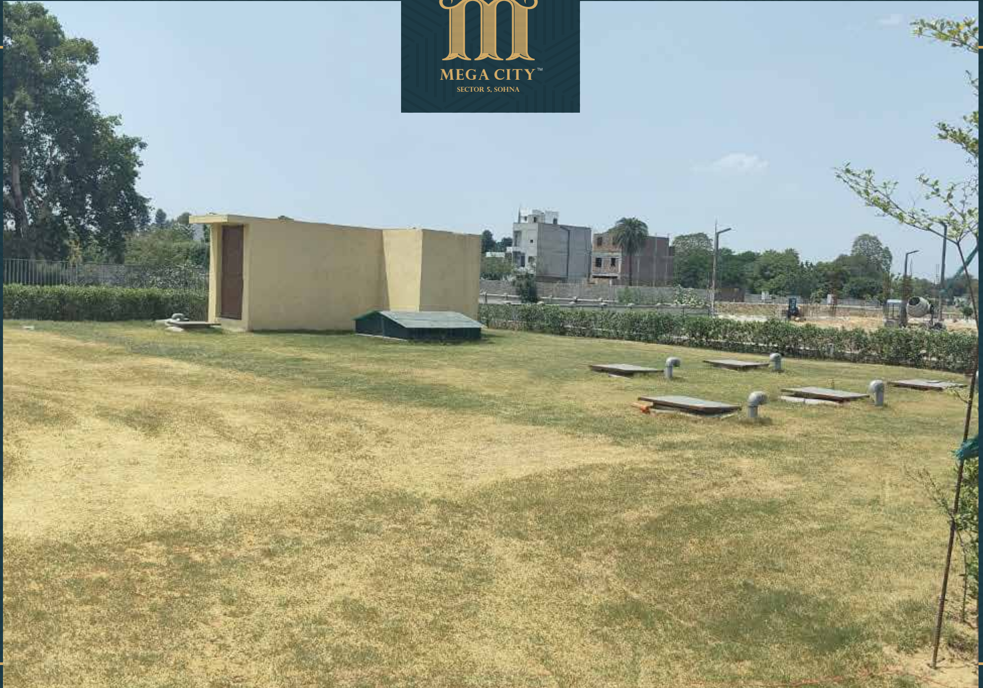
UGT construction completed
