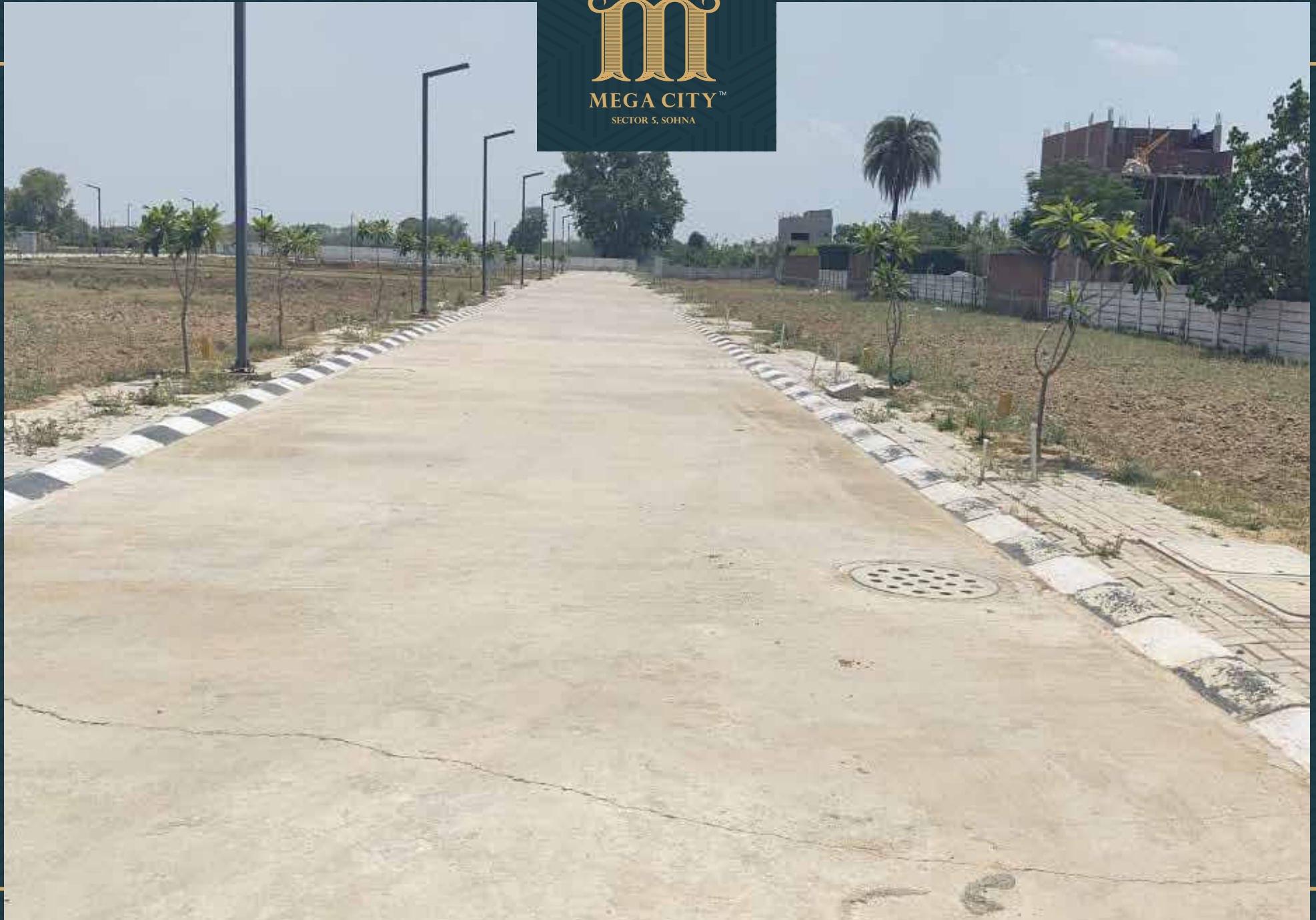
Road no. 1 development work completed
