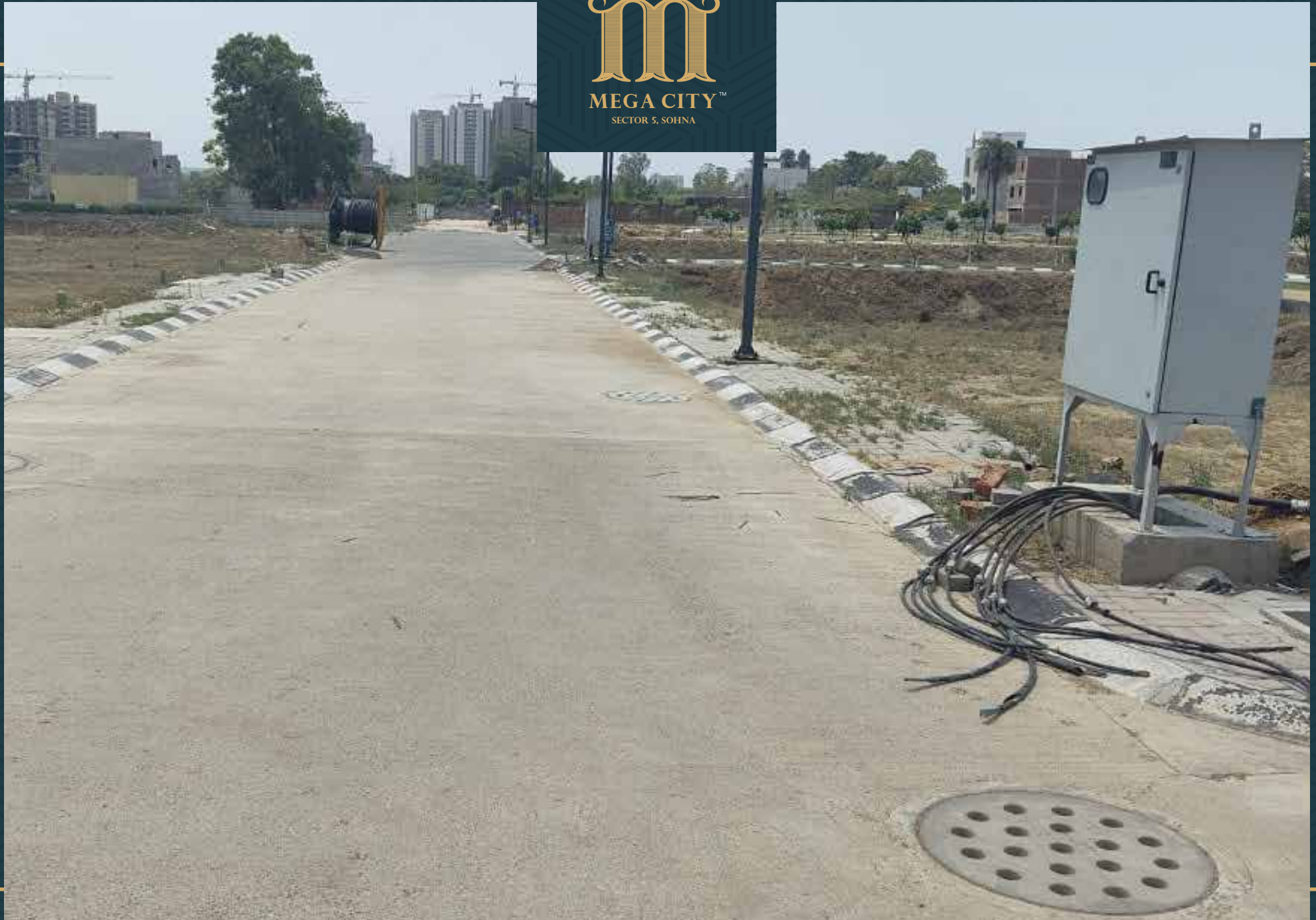
Road no. 7 development work completed and plantation work is in progress
