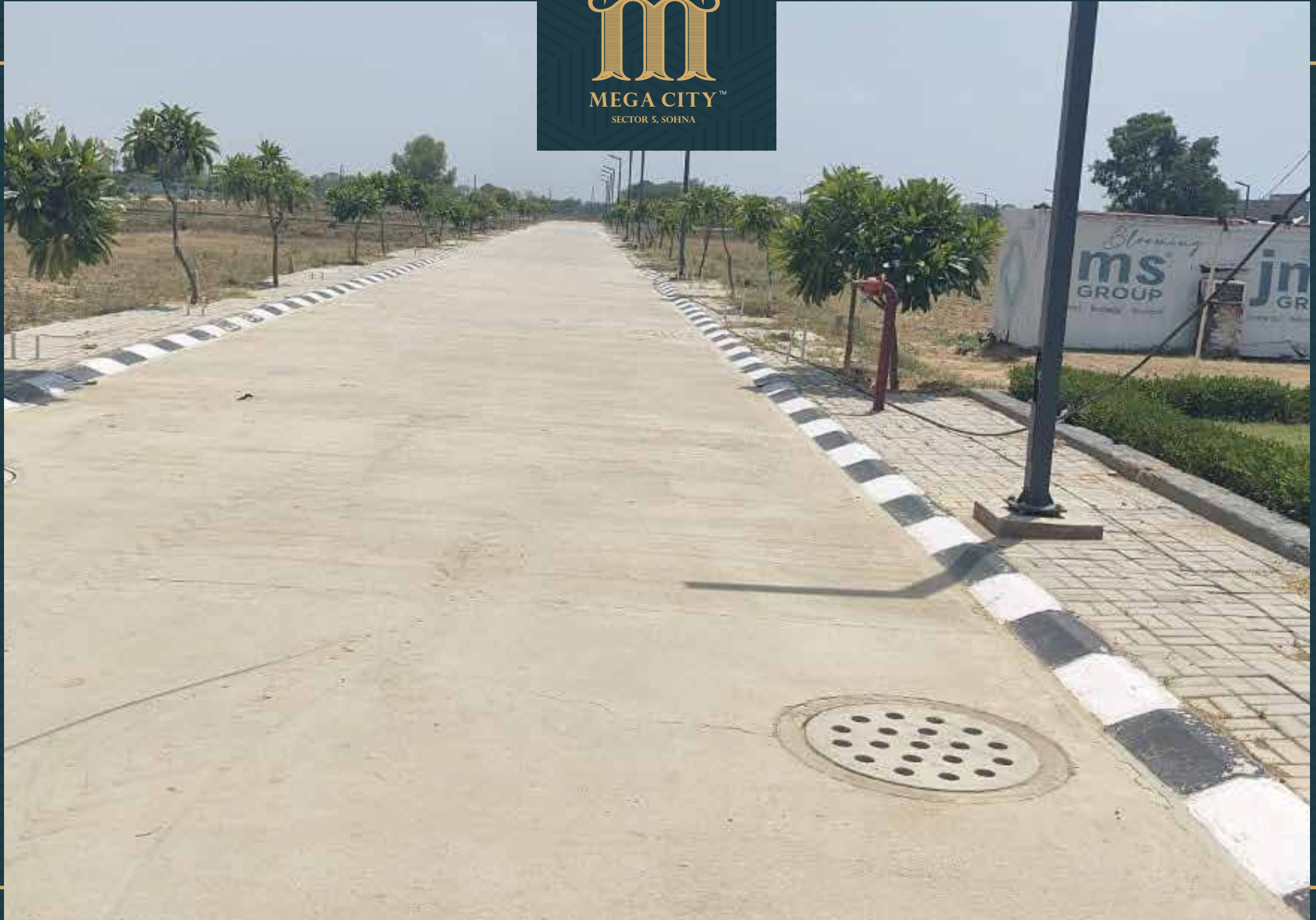
Road no. 3 development work completed
