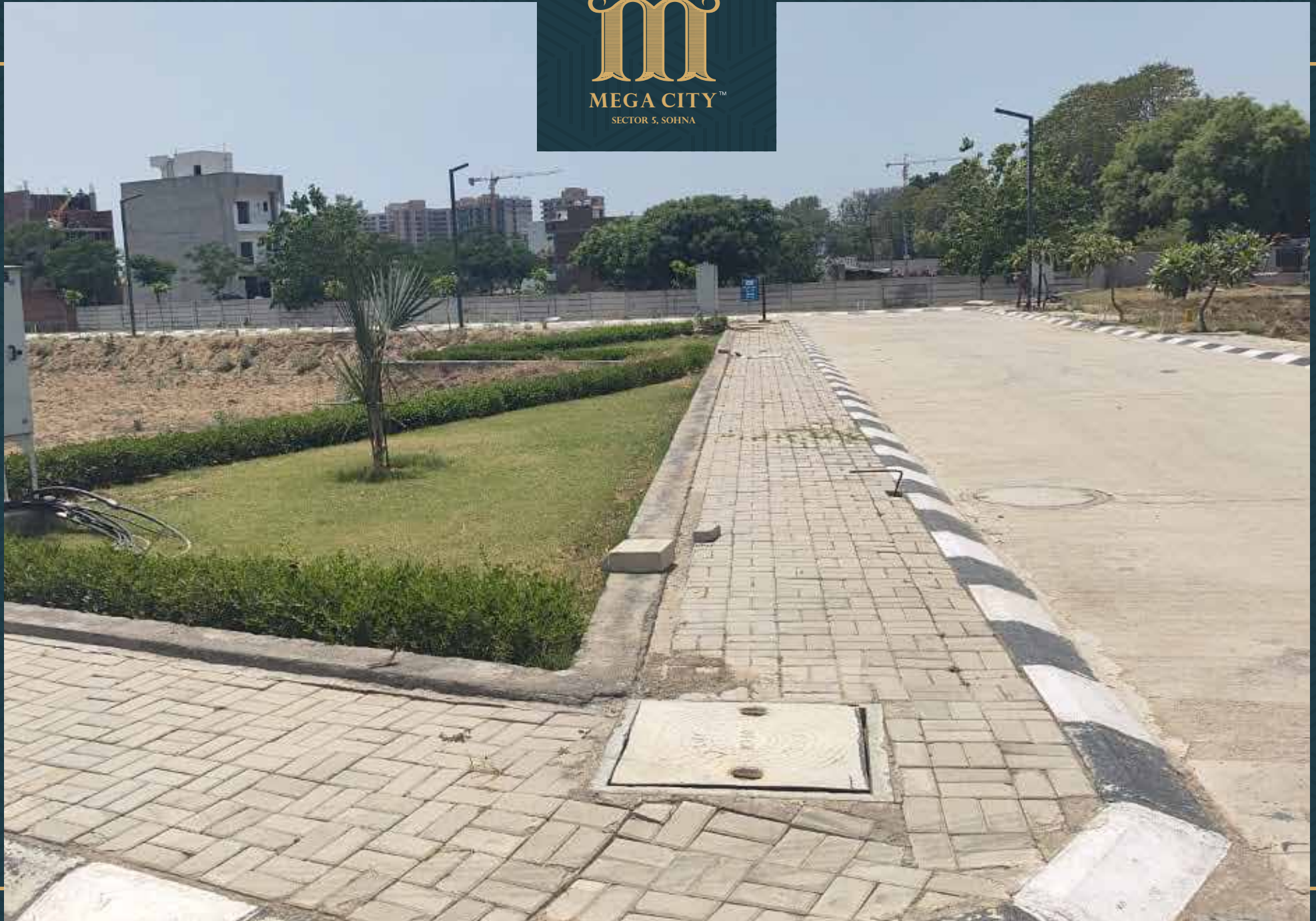
Green area development work completed
