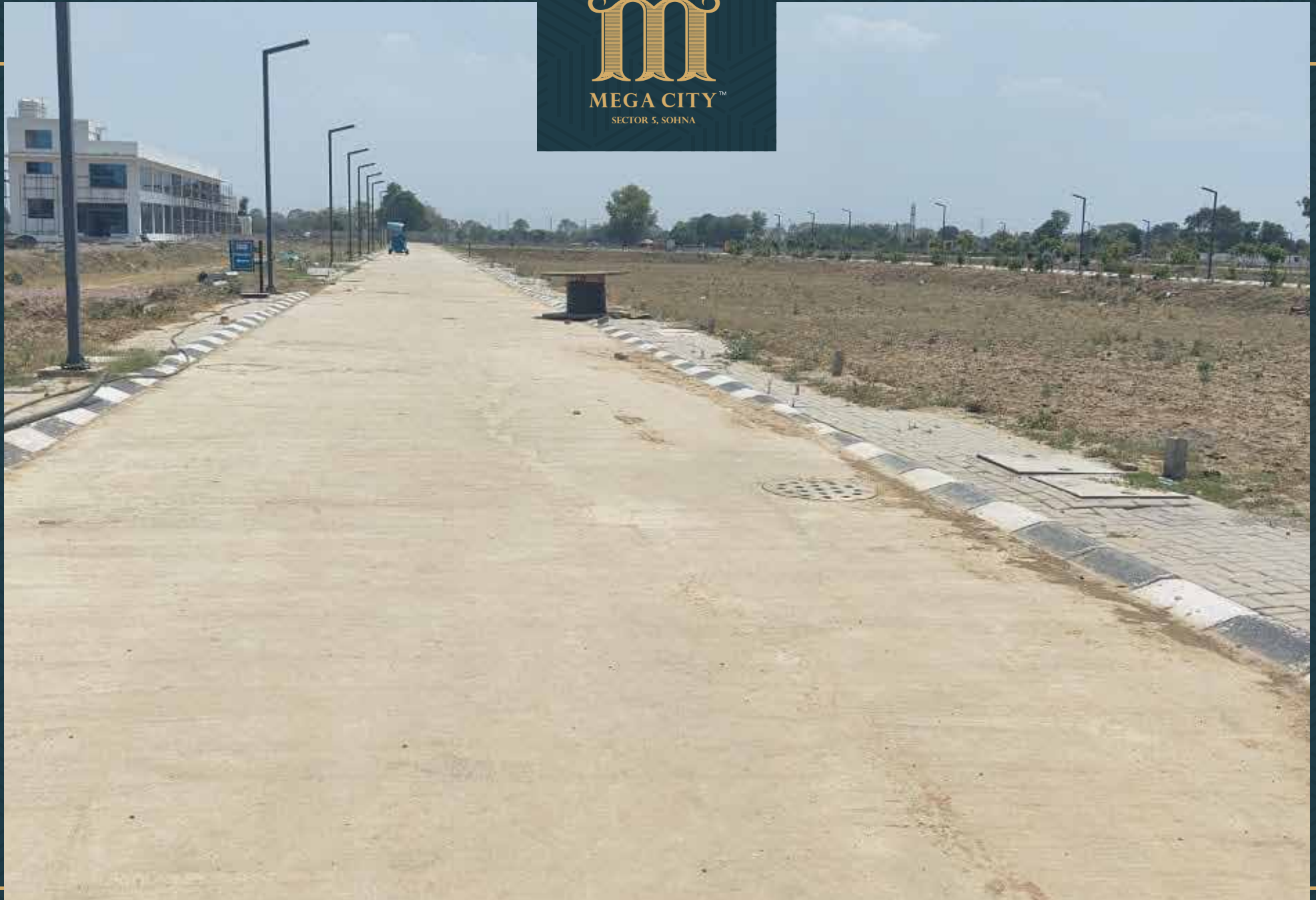
Road no. 5 development work completed and plantation work is in progress
