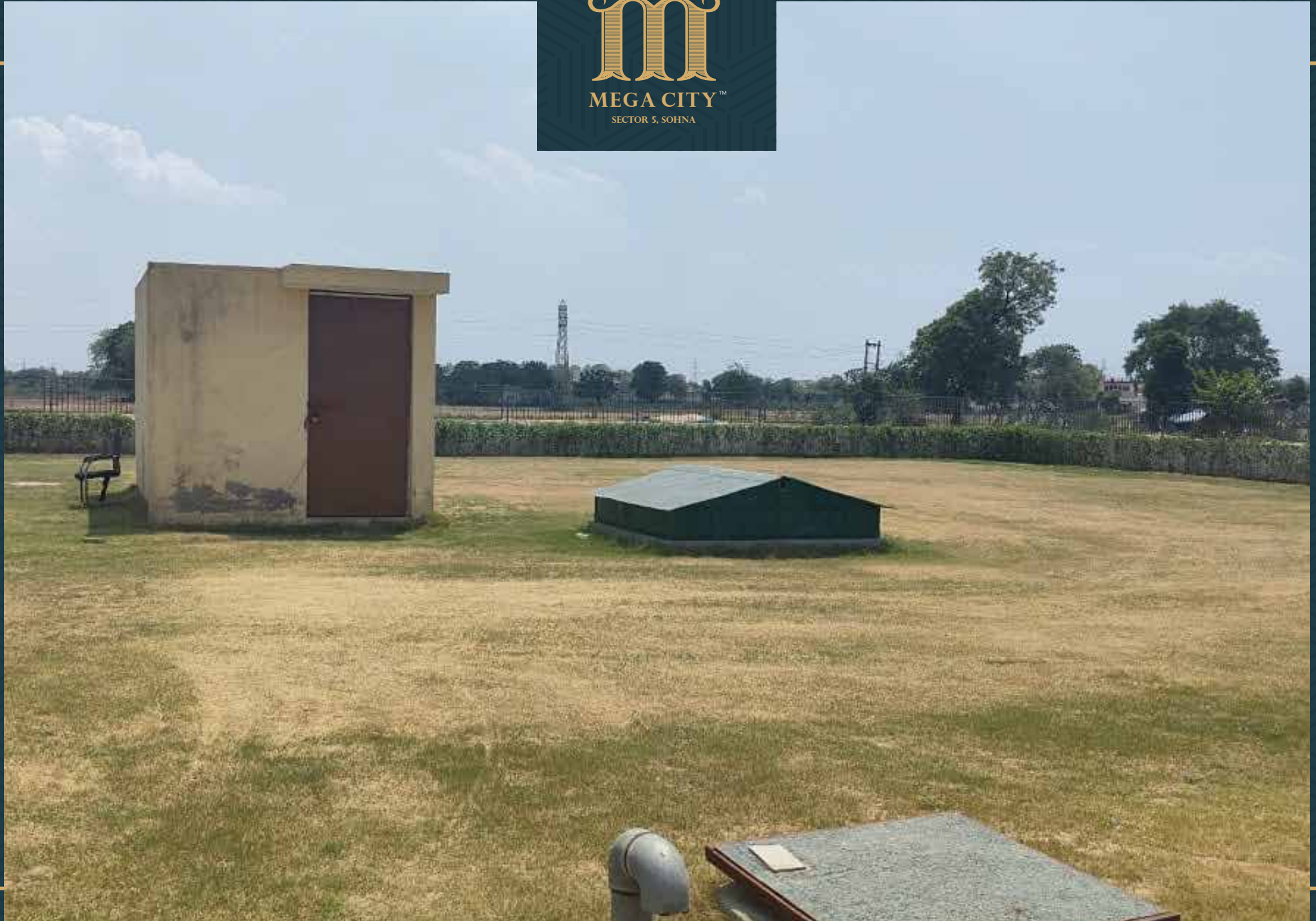
STP construction completed
