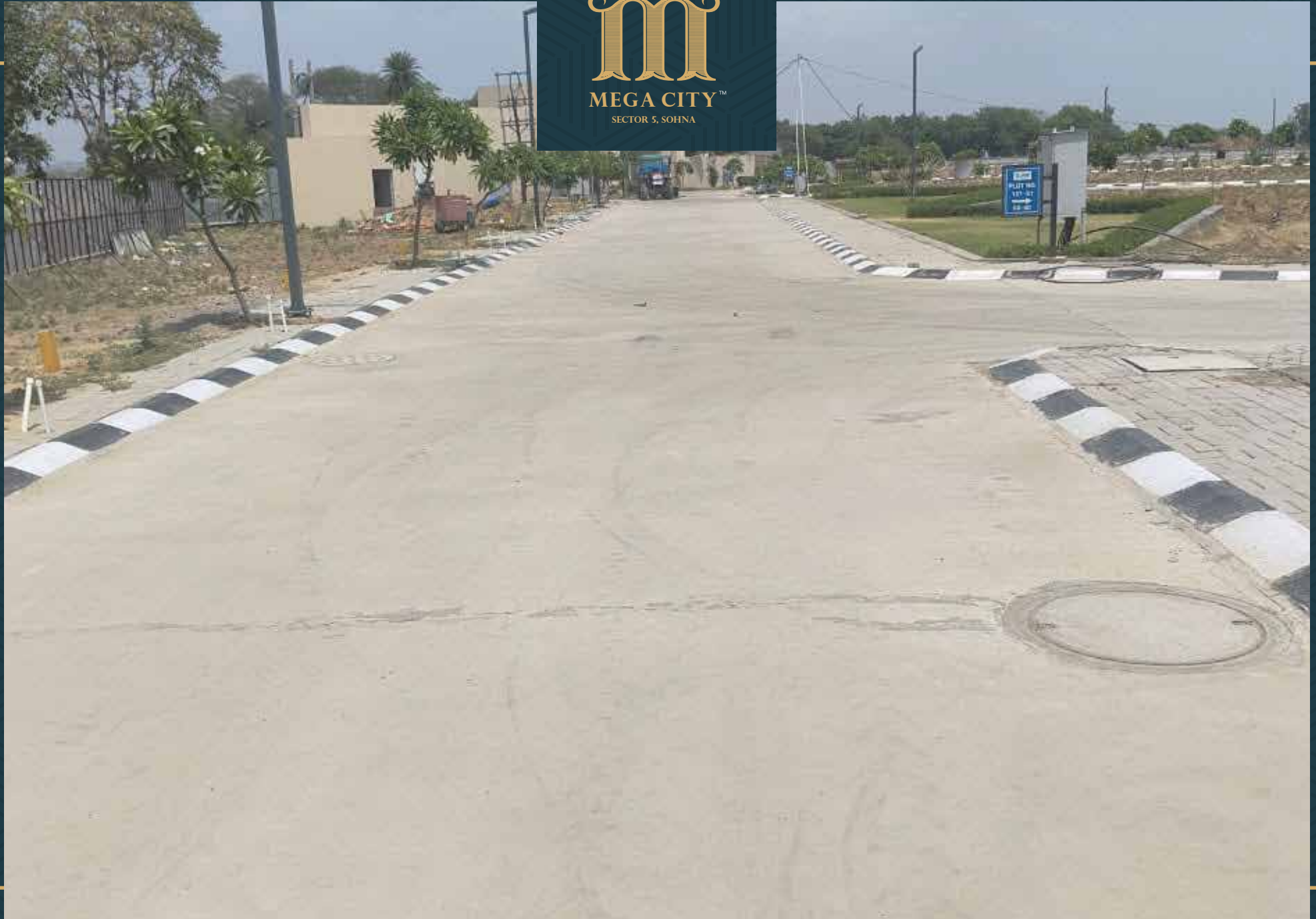
Road no. 6 development work completed
