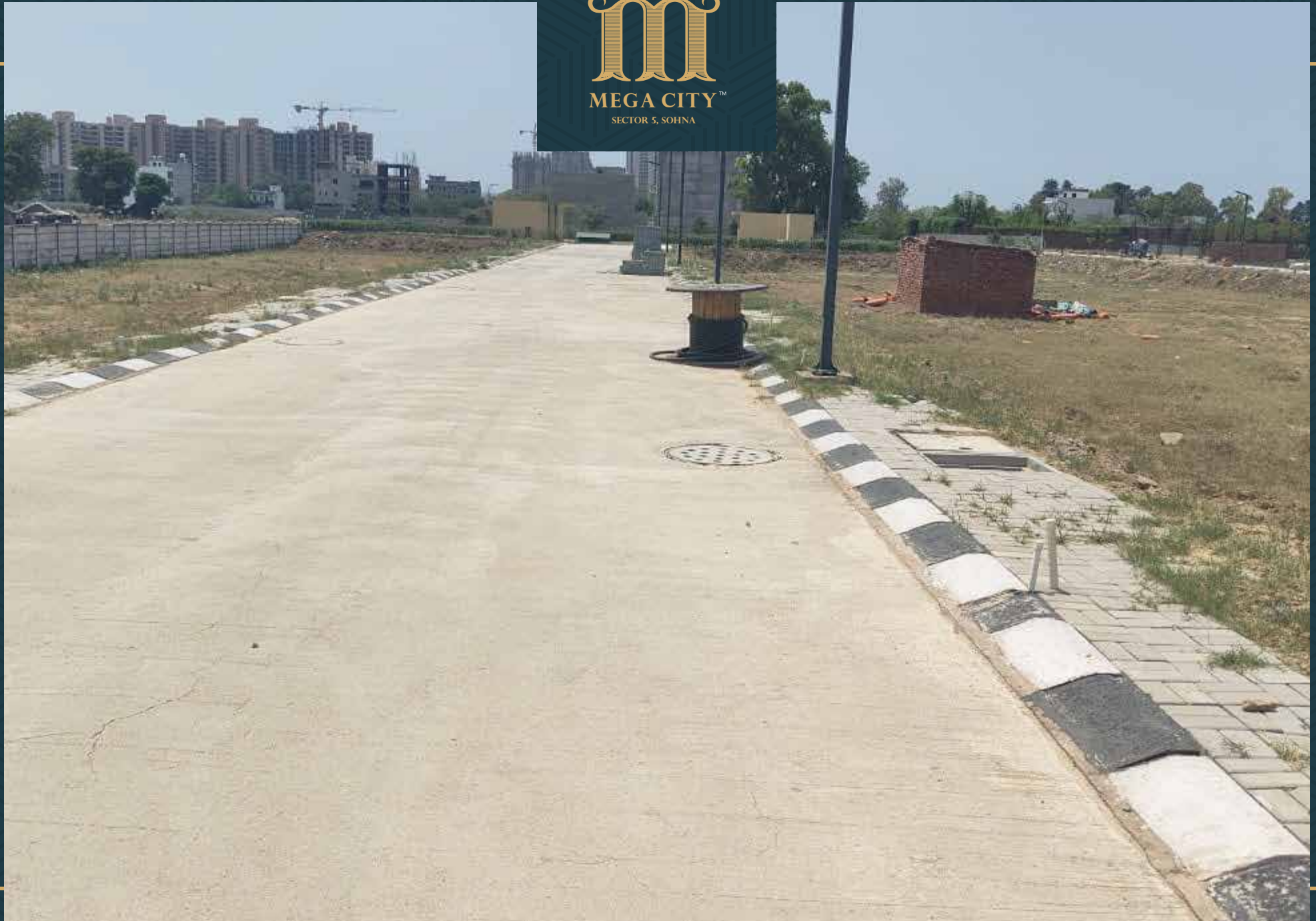
Road no. 8 development work completed and plantation work is in progress
