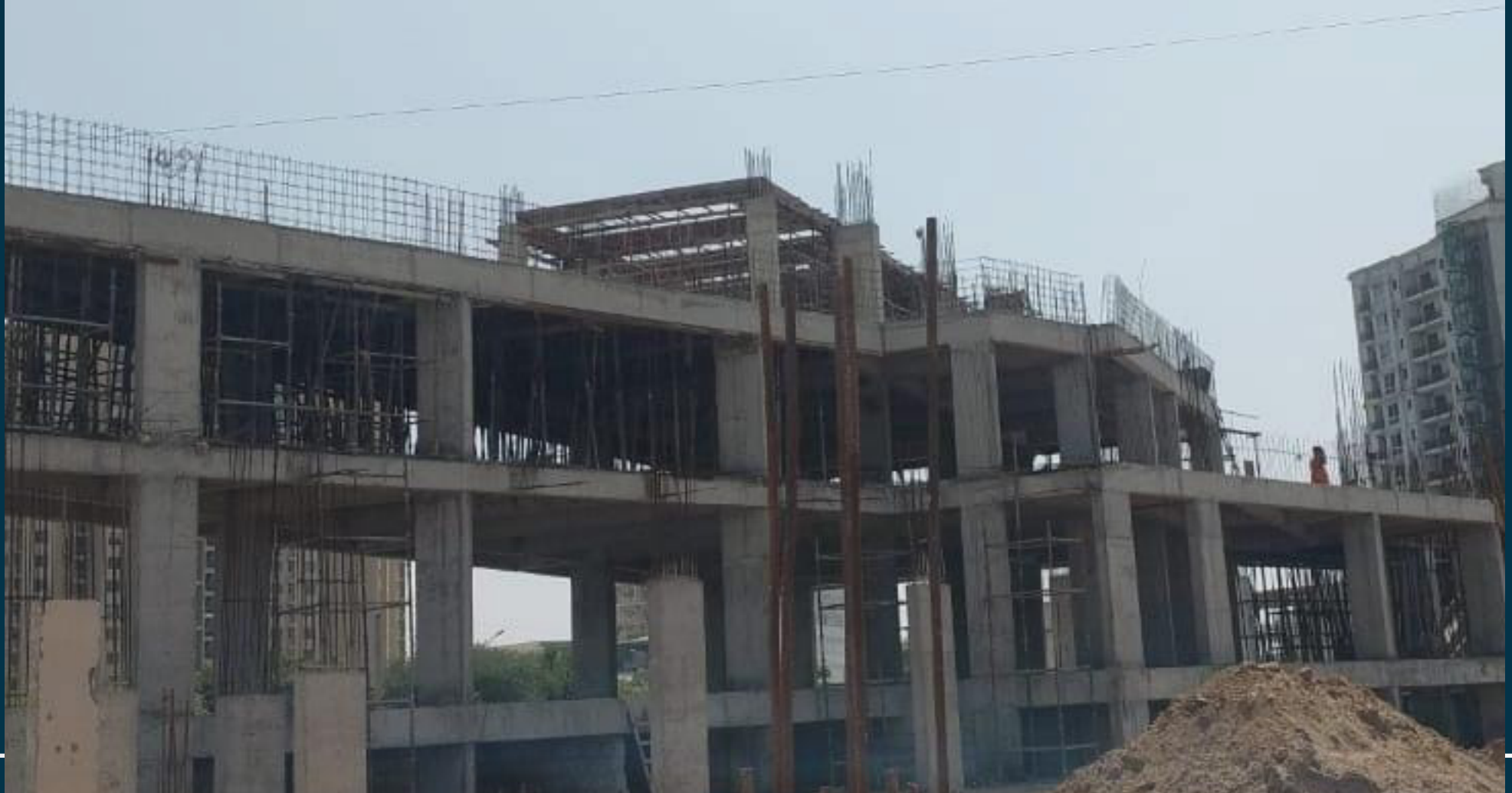
Block work in progress at lower ground floor level
