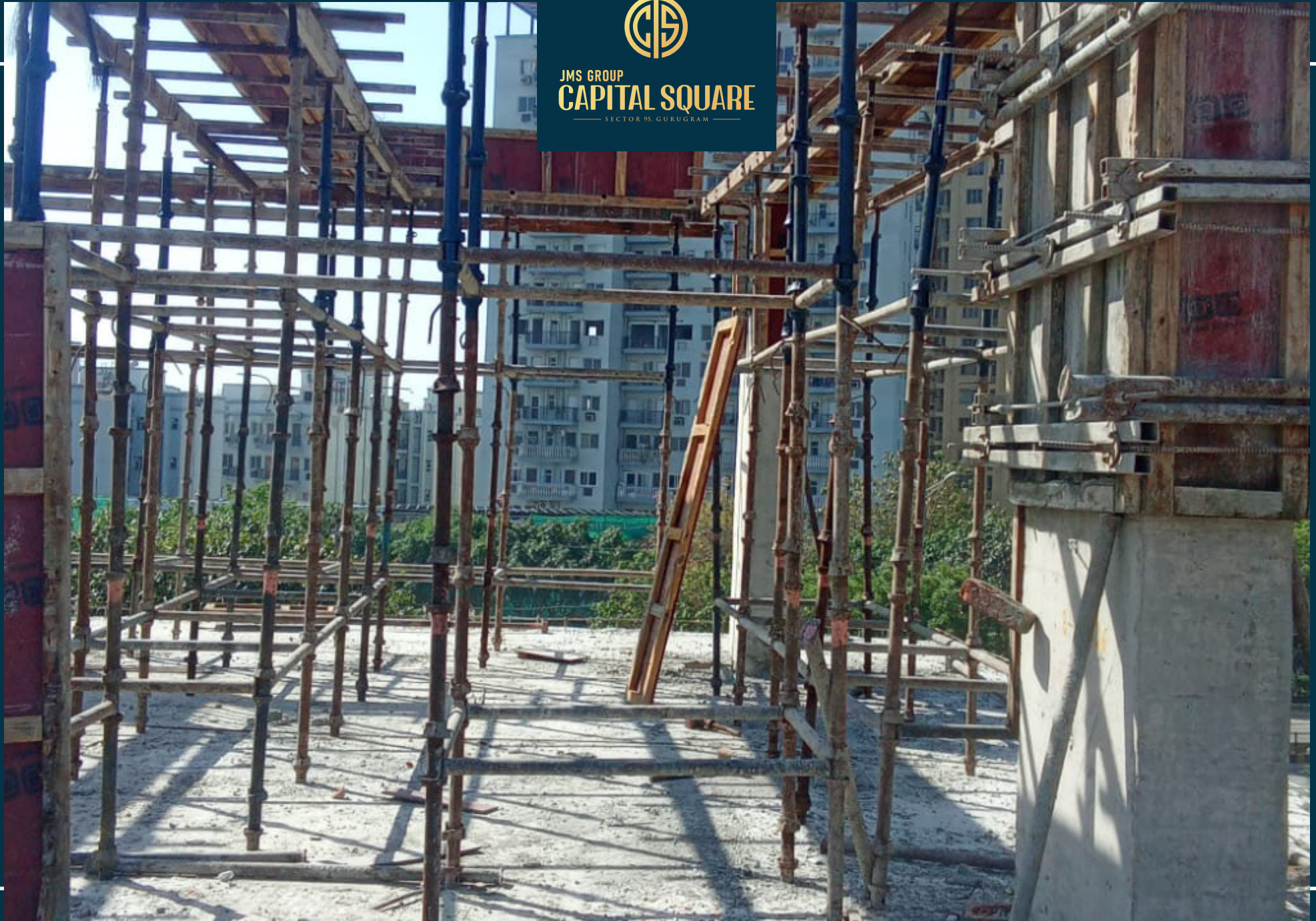
2nd floor roof slab shuttering work in progress
