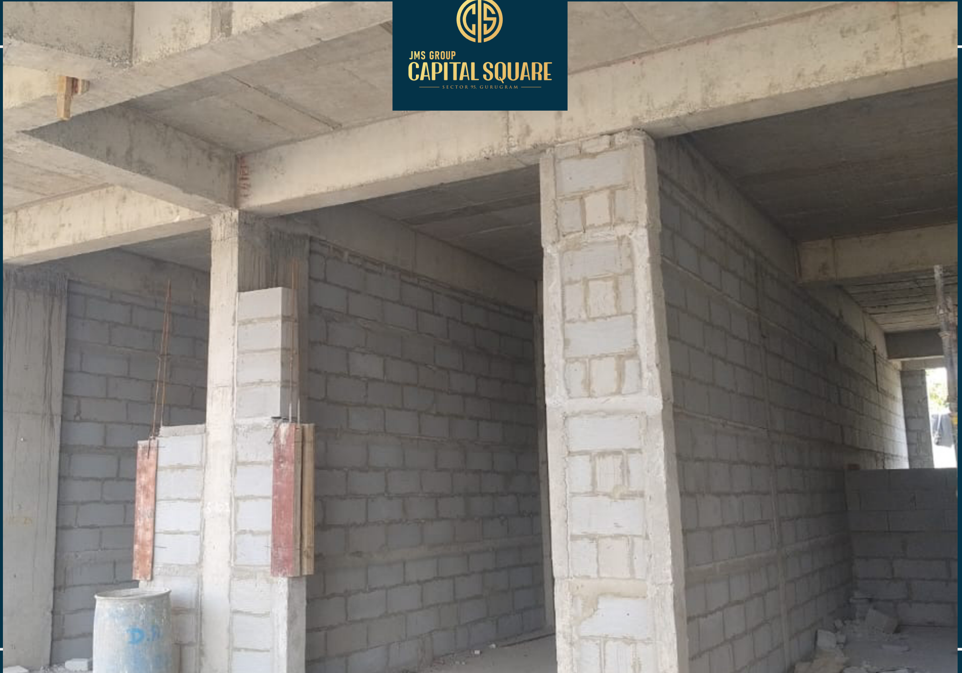
Block work in progress at lower ground floor level
