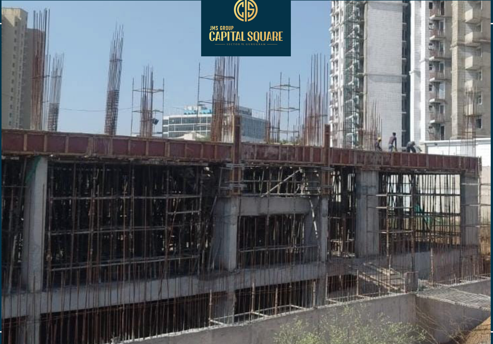
Underground floor level completed
