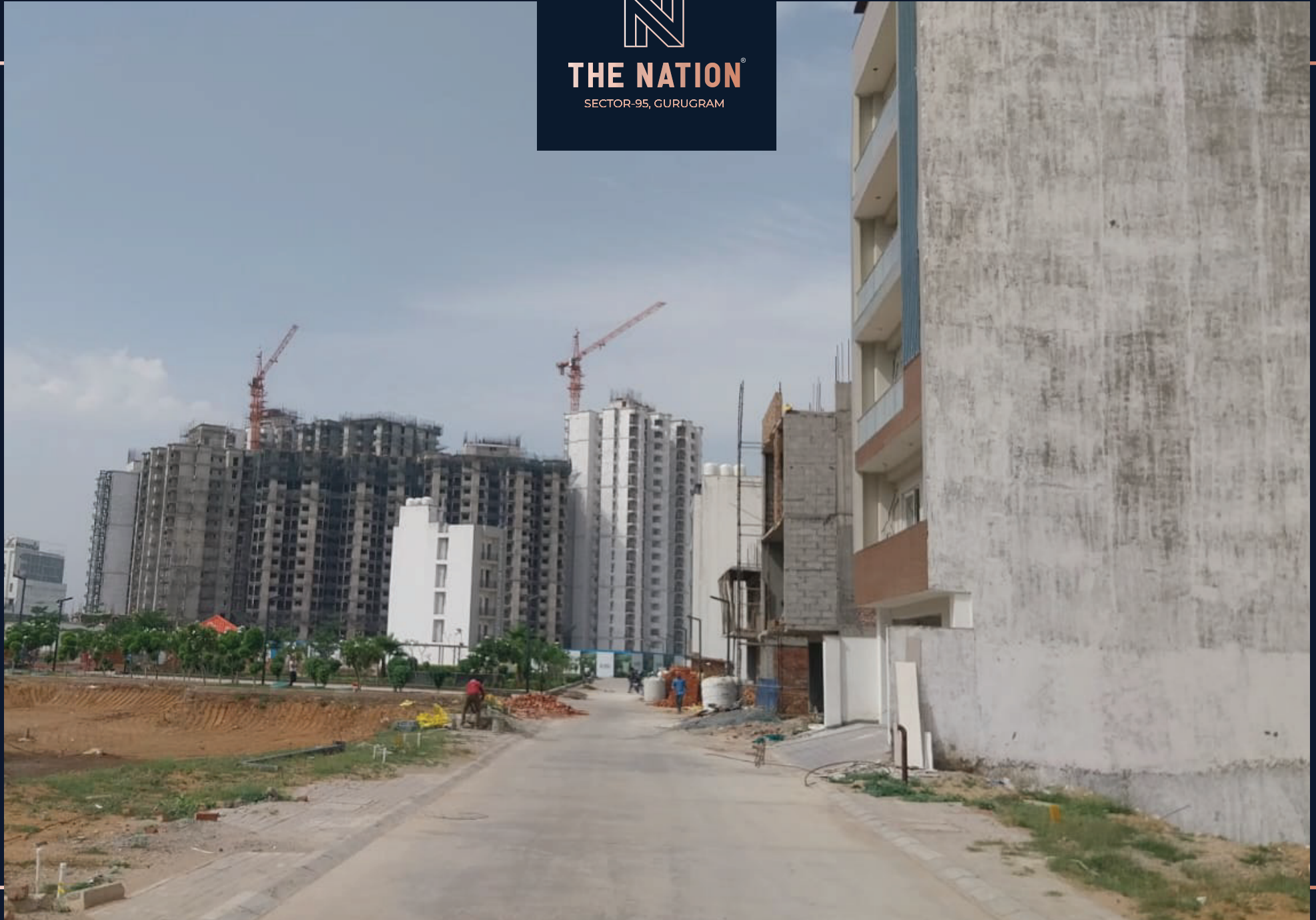
Construction of internal roads completed
