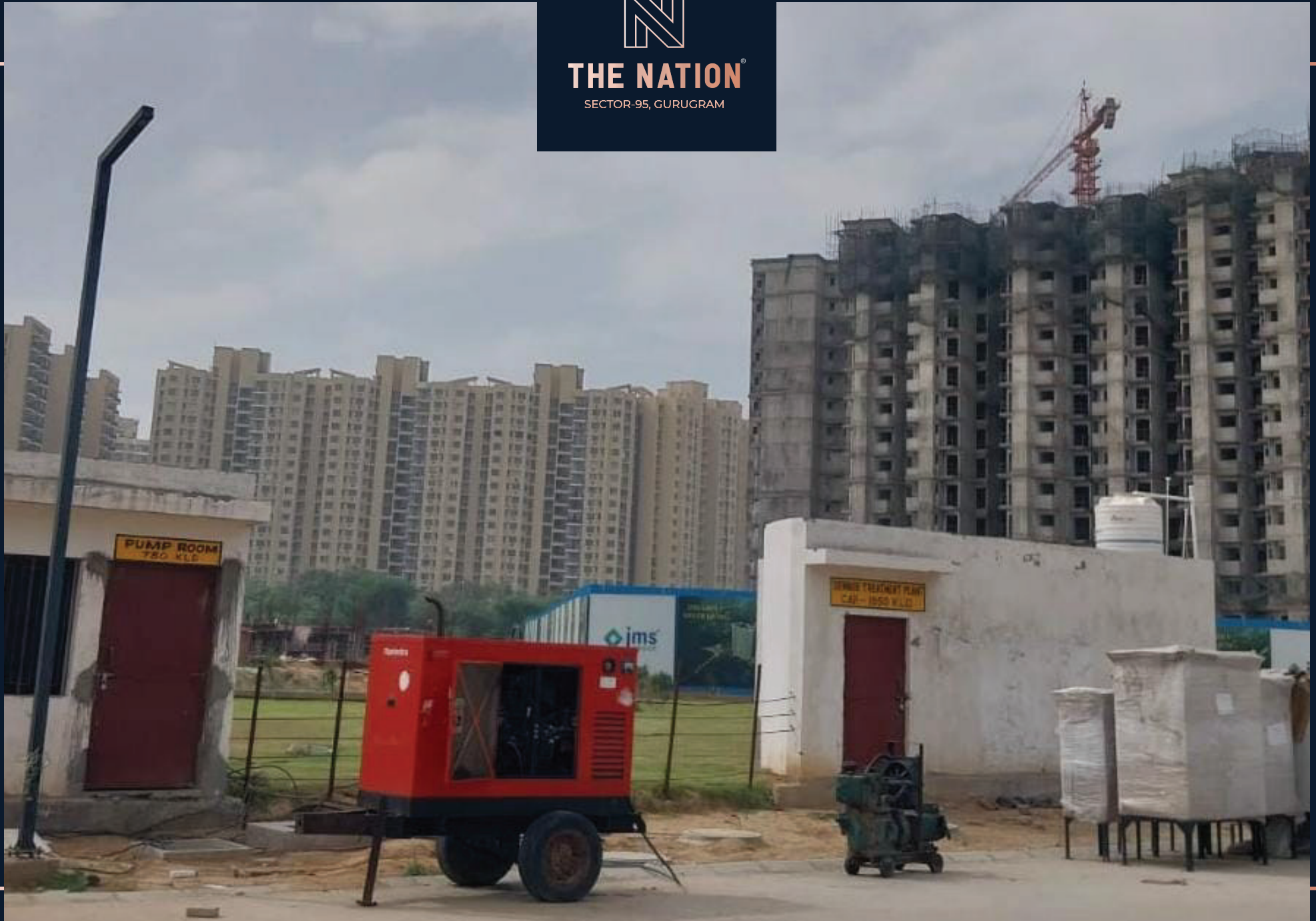
STP UGT construction completed
