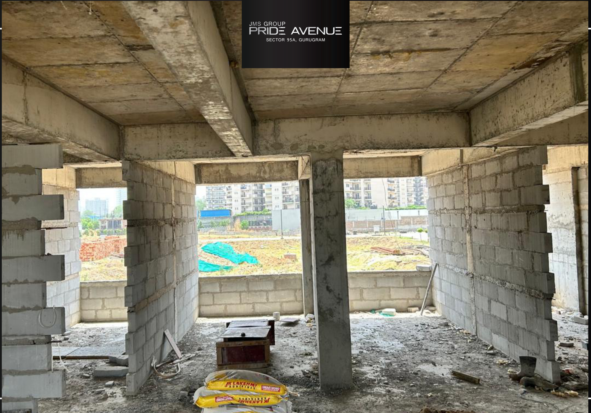
Ground floor block work in progress
