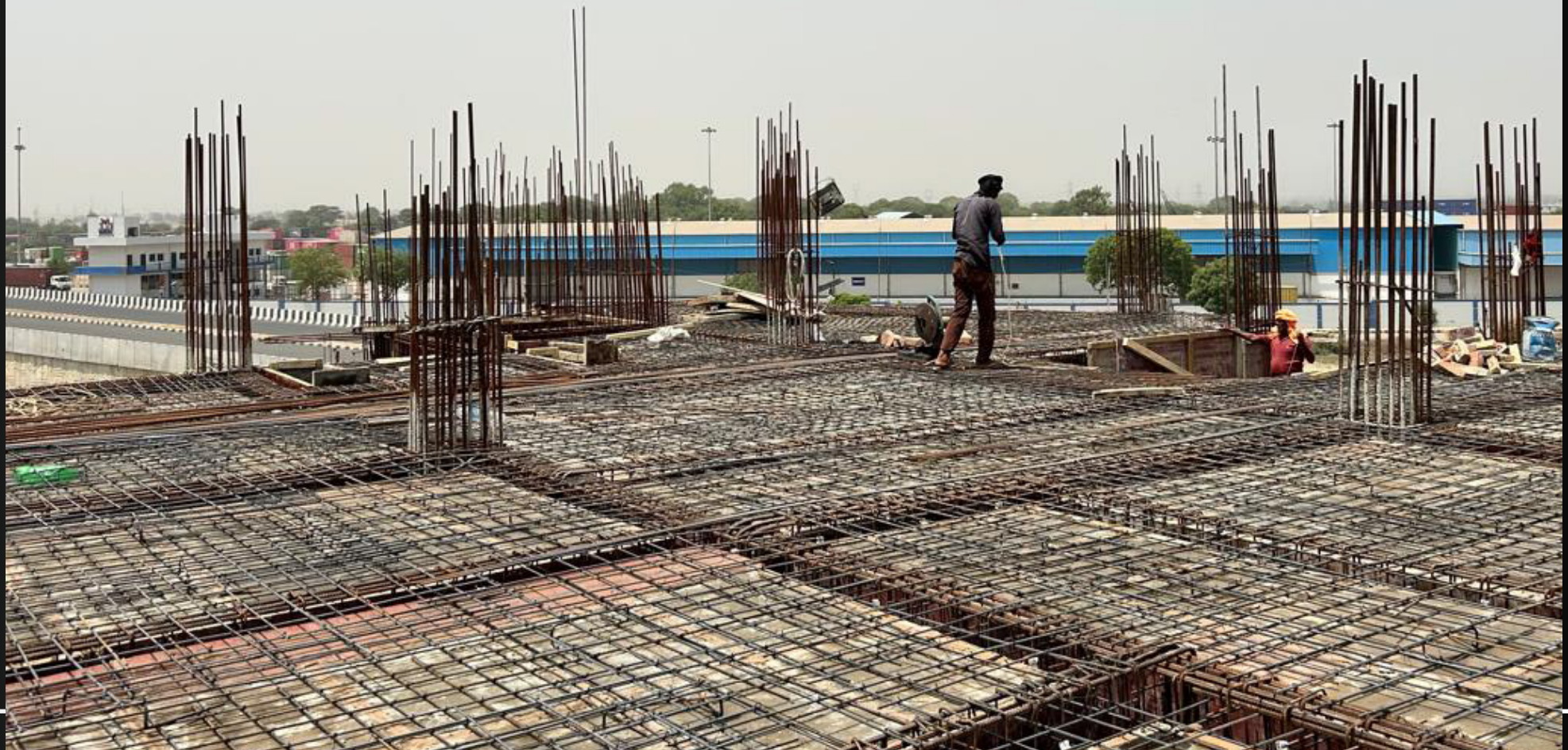
3rd floor slab reinforcement
