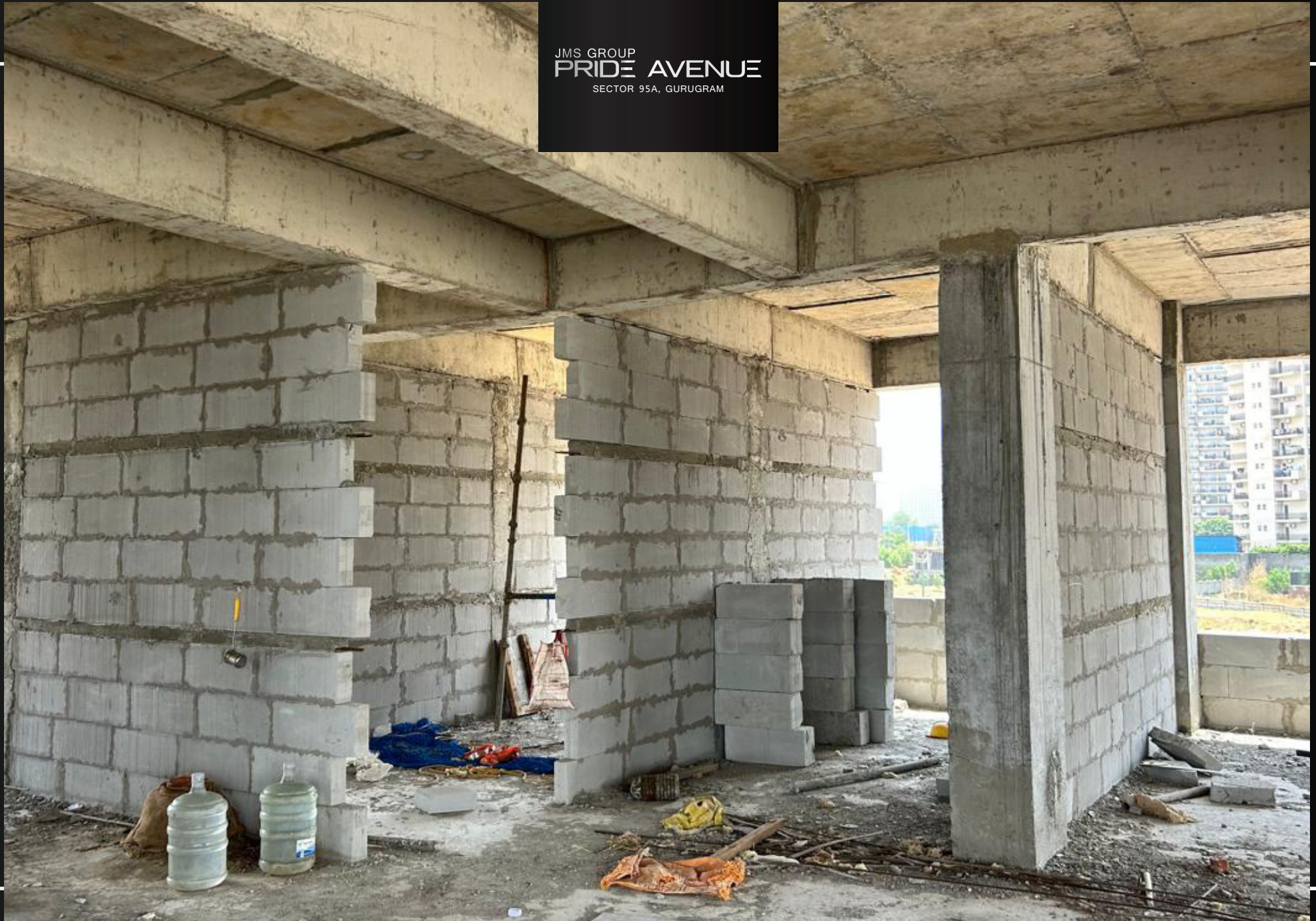
1st floor block work in progress
