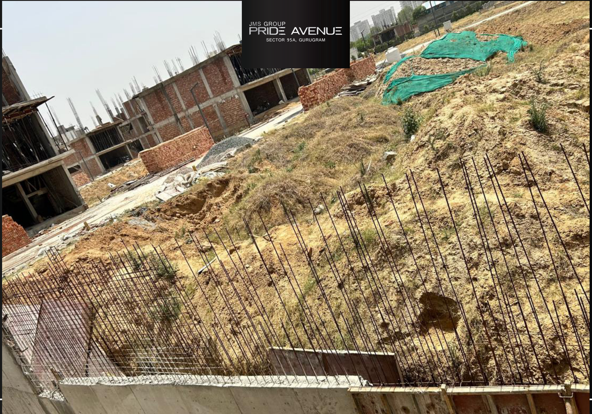
Outer retaining wall work in progress
