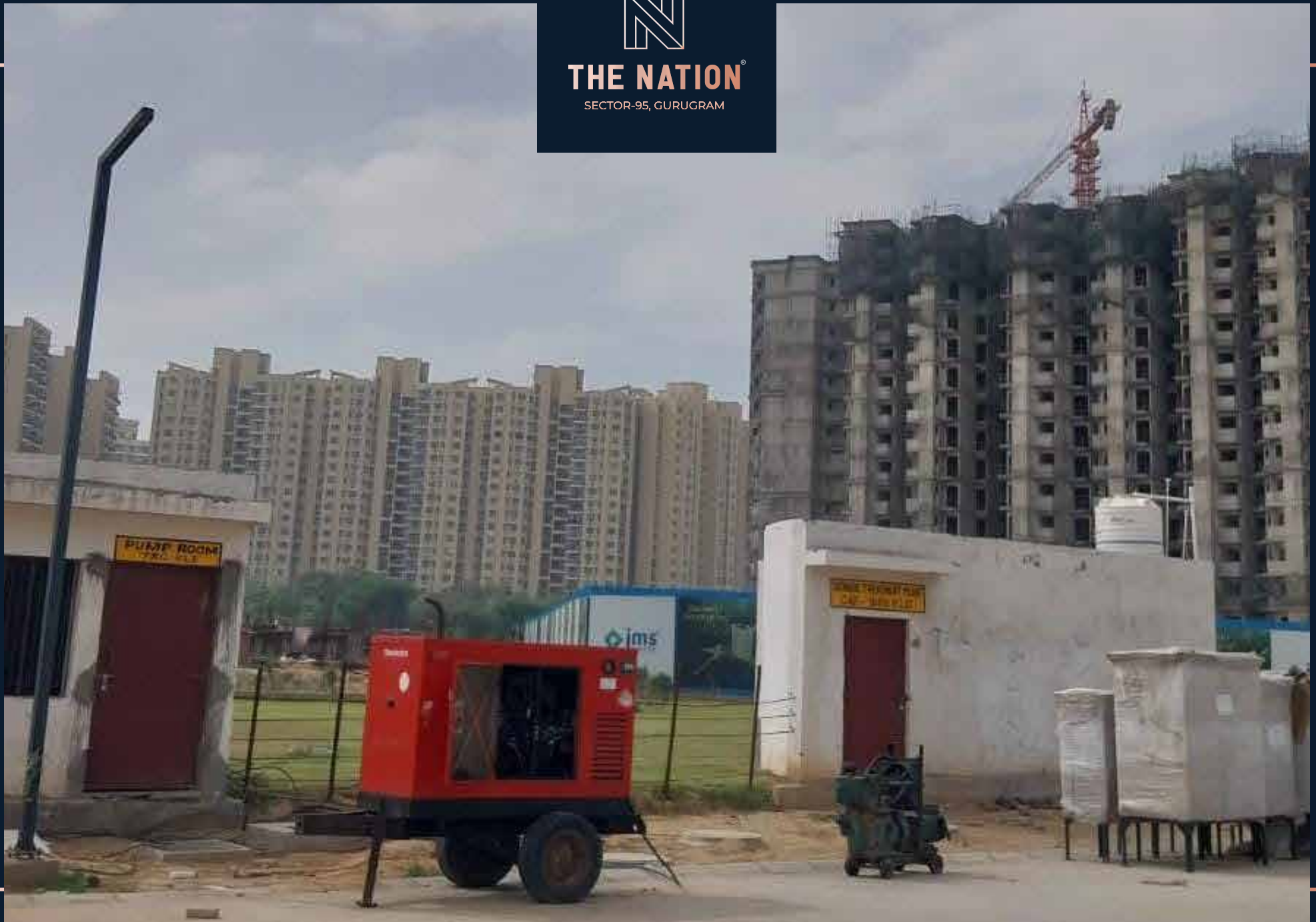
STP UGT construction completed
