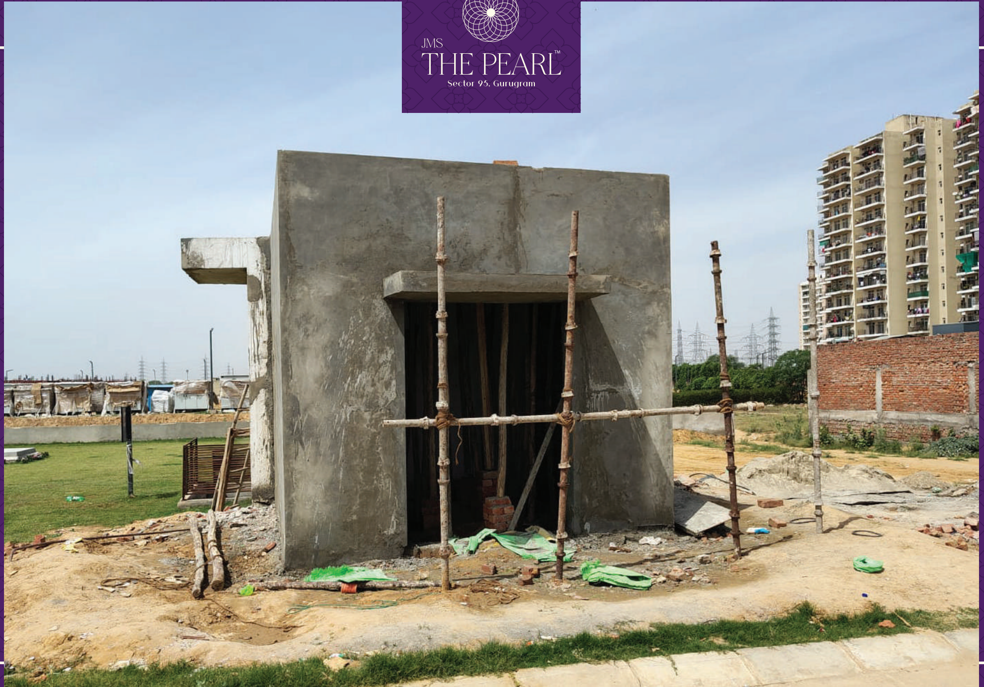
Meter room work in progress
