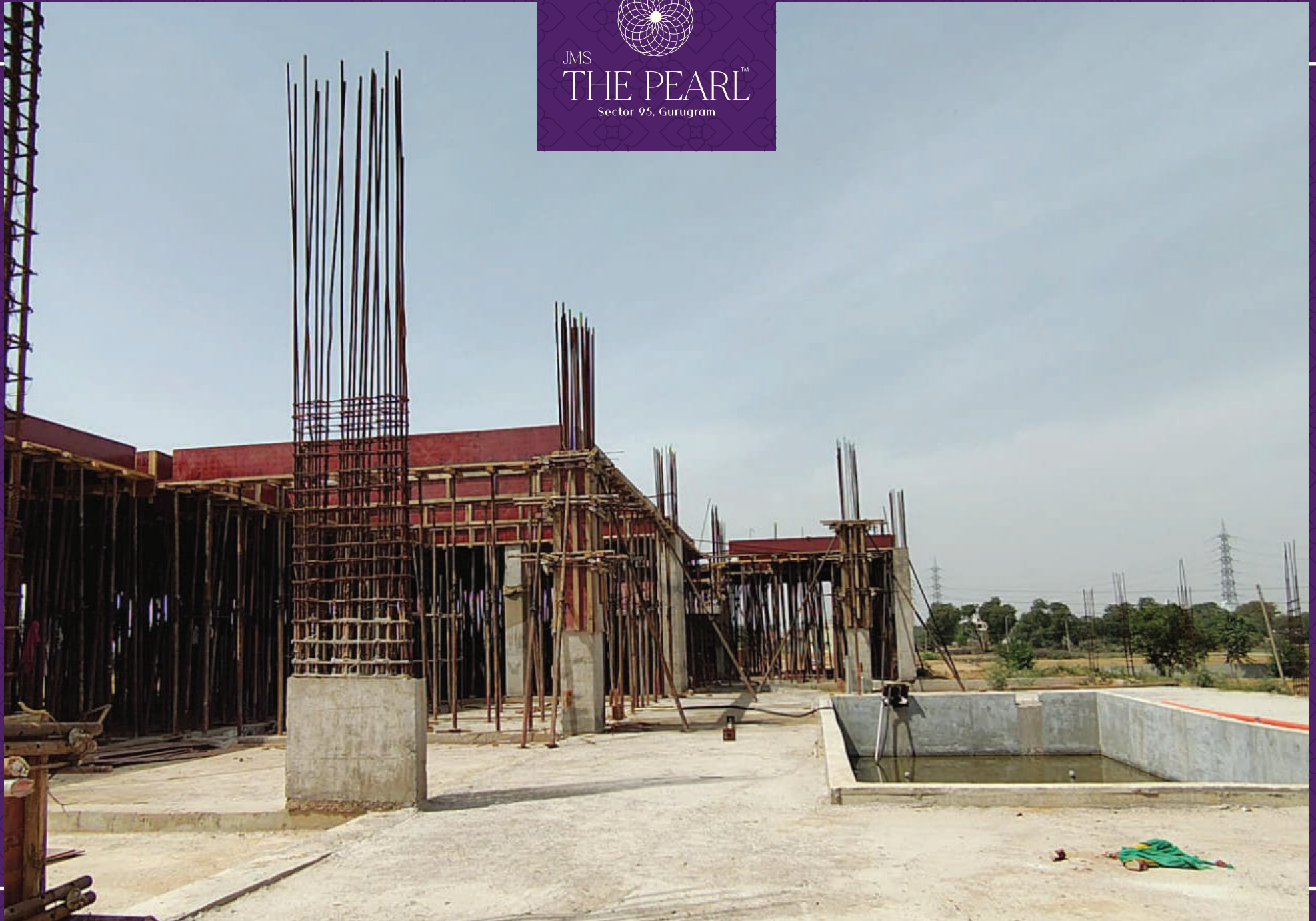
Clubhouse work in progress
