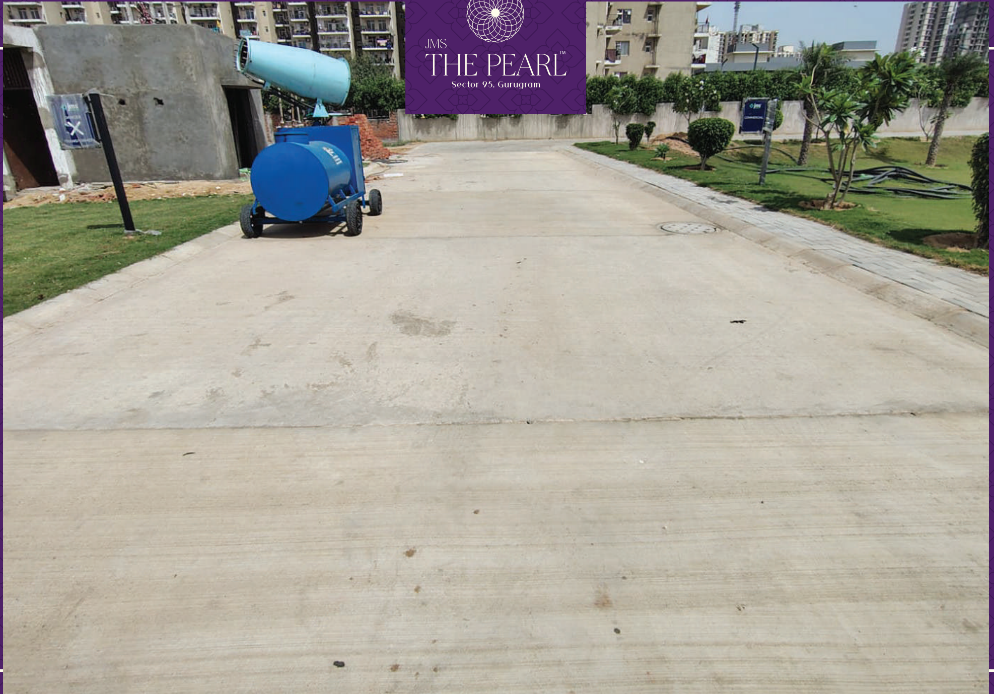
Construction of internal roads in progress
